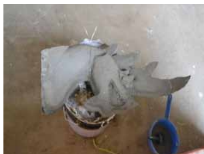
New dragon motif at the roof edge was produced using a mold of similar profile
