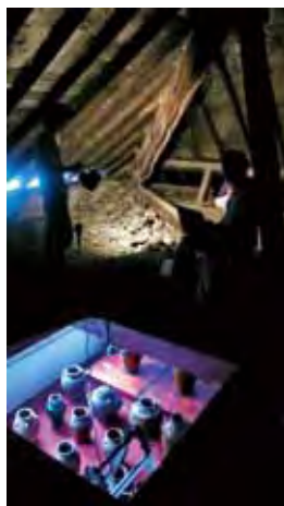
Photo 1. Survey on the roof
