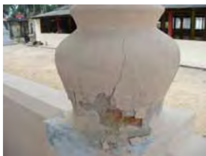
Dampness, broken plaster and termite infestation are some of the common building defects found at Ubosoth (Bothd)
