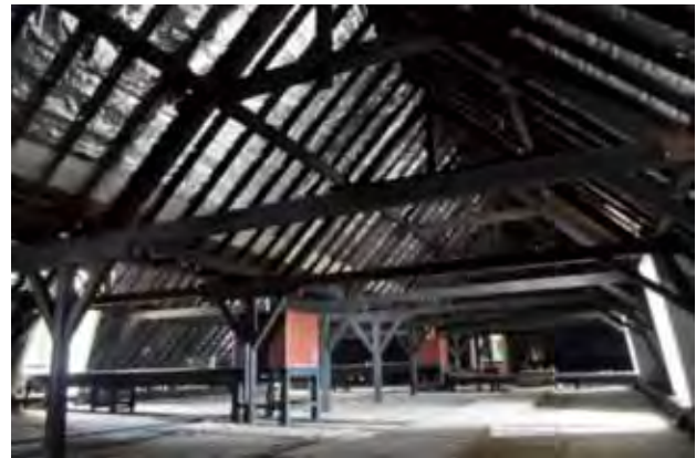
Photo 5. Trusses in the attic room
