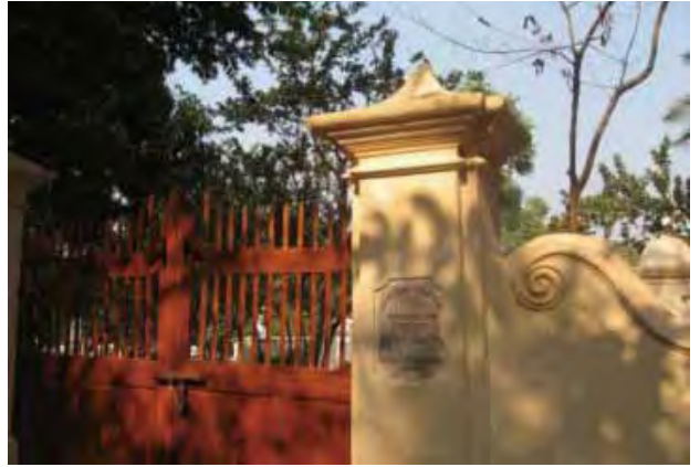
The new entrance gate and gateposts after restoration
