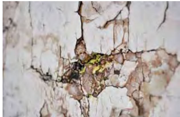
Photo 8. Decomposition on the wooden column
