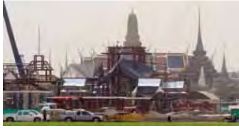
Fig. 13. The HRH Bejaratana's royal crematorium was under construction in 2012.
