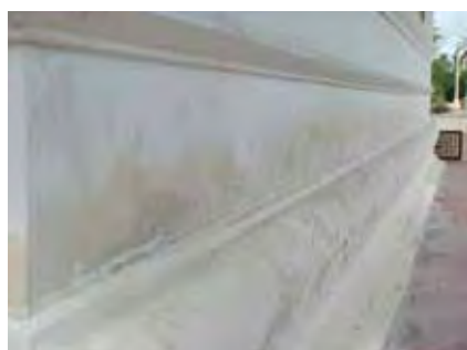
Dampness, broken plaster and termite infestation are some of the common building defects found at Ubosoth (Bothd)
