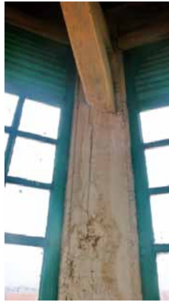
Photo 6. Defects on the tower column structure
