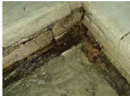
Timber blocks around the tank
