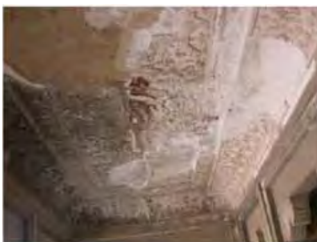
Restoration of stucco tracery work
