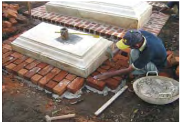
Construction of brick platforms in lime mortar where originals were missing
