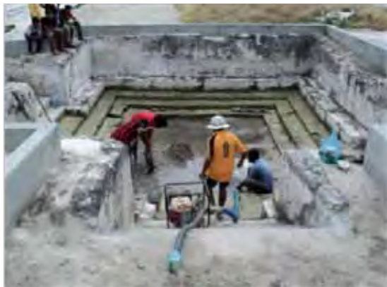
During excavation : pumping out water
