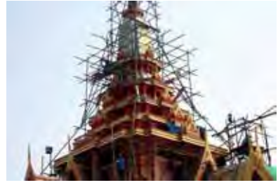
Fig. 14. The HRH Bejaratana's royal crematorium: The roof architectural ornament was assembled.
