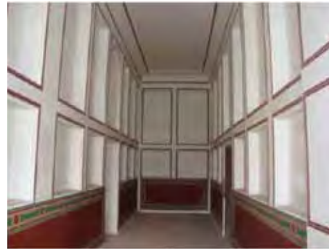
Restoration of glaze lime plaster fresco paintings
