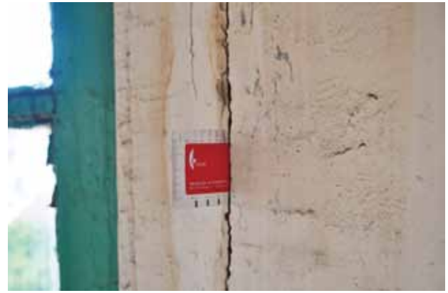
Photo 7. Cracks of 3 cm depth on the wooden column
