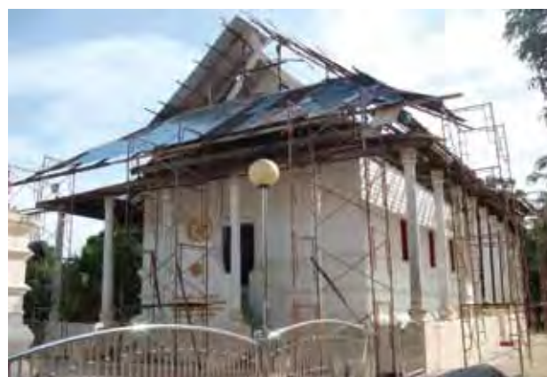
Temporary zinc-sheet roofing was built as a shelter to protect Ubosoth (Bothd) from heavy rainfall
