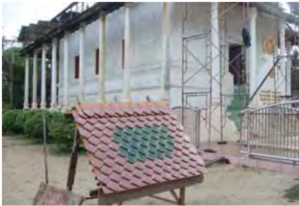
A roof mockup using new clay glazed tiles was set up at site for technical references
