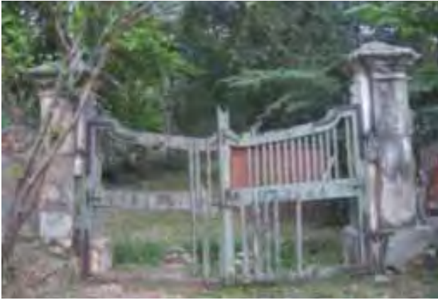
The wooden entrance gate and original gateposts before restoration
