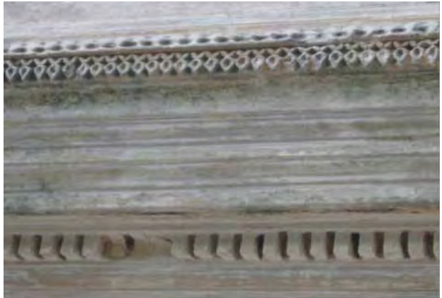
Layers of lime wash carefully scraped and embellishments in lime mortar exposed
