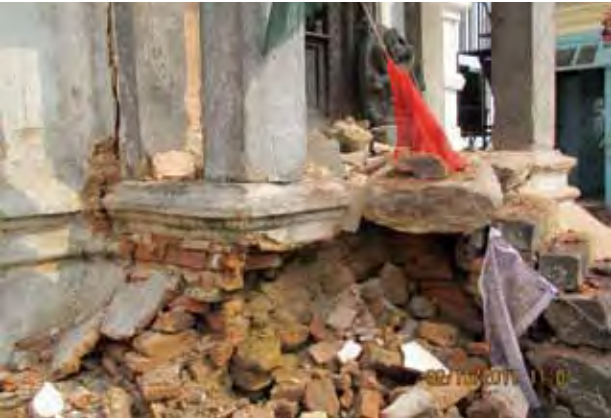
Severely damaged just above the foundation
