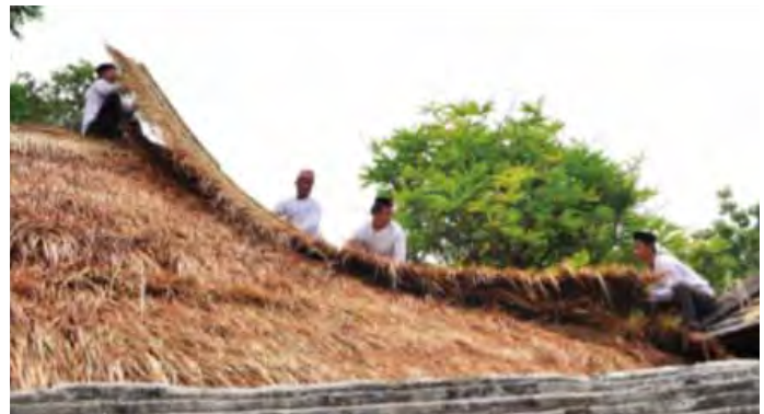
The reinstallation of hip ridge for finishing reroofing
