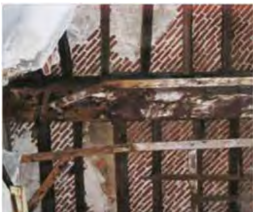
Delamination of ceiling plaster and exposure of terrace bricks, debonded joists and moisture laden primary wooden beam
