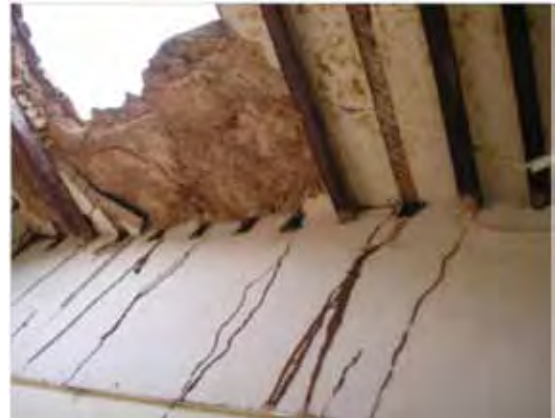
Extensive termite infestation led to deterioration in the wooden joists and eventual collapse of the roof
