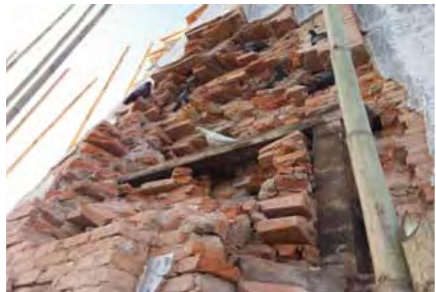
Damaged by the disaster
