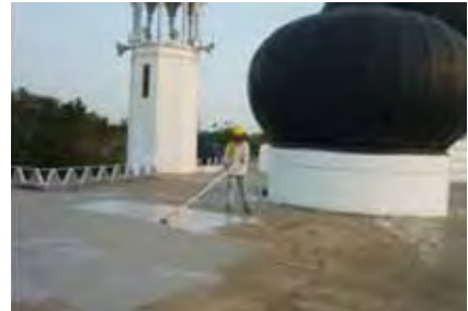
The application of moisture barrier coating (Duraflor NWB21) onto the concrete flat roofs of the Alwi Mosque.
