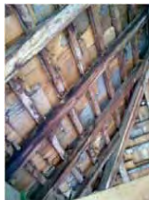
Building with wooden shingle roof ( sirap )
