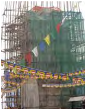
In the process of dismantling the temple
