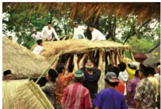
Raising and installing a part of the new thatched roof
