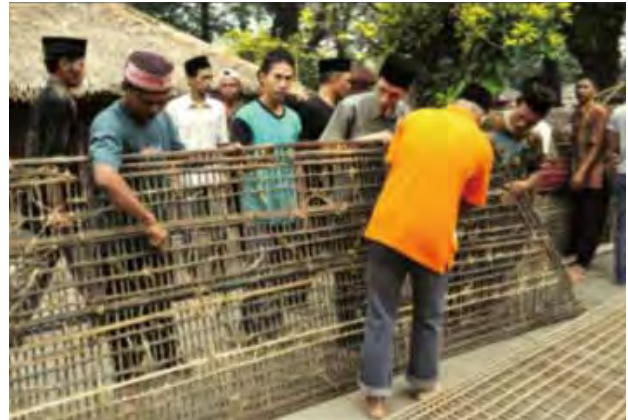
Some other men were releasing the old welit from the wooden frame and repairing it.
