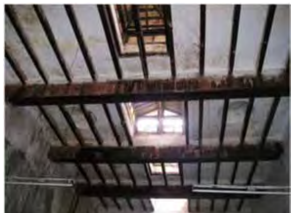
A typical Madras Terrace Ceiling with primary beams and secondary joists deteriorated due to water seepage and vegetation growth
