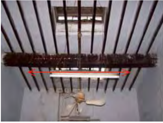
Deflection of primary beams and secondary joists as well as shear cracks can cause structural failures
