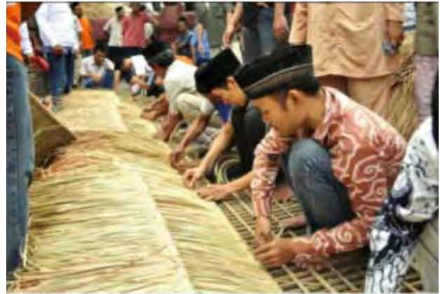
The installation of new welit to the old wooden frame
