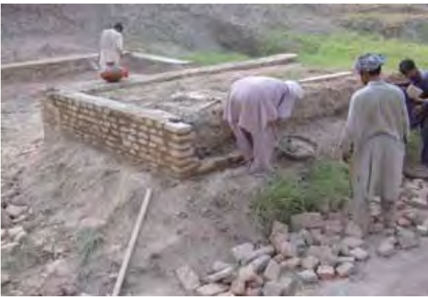
Figure 3. A. Conservation of existing structure in progress on great granary Mound F
