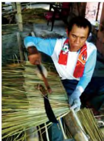
The wooven process of alang-alang using rambatan (small bamboo slat), jalon (bigger bamboo slat) and lulup (rope) done by the local inhabitants for five days on the spot near Omah Gede building which located outside Kabuyutan Trusmi Complex. The Omah Gede reroofing was held about one week after Memayu. The labour was all voluntary work.
