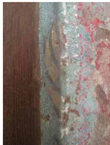
Fig. 4. The evidence of the original decoration of Ubosot corridor ceiling was found under several previous redecoration materials.
