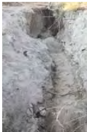
Fig. 22: Excavation trench along the runway of rainwater in the gully
