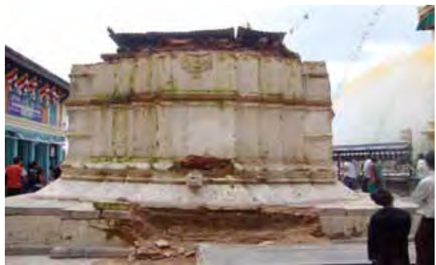
In the process of dismantling the temple
