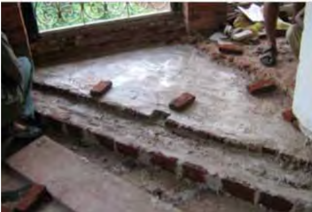
Laying of terrace bricks diagonally and along the edge
