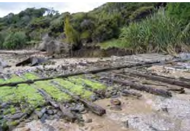
Figure 30. View of the slipway looking SW towards the workshop (NZHPT 2007). See Figure 17.
