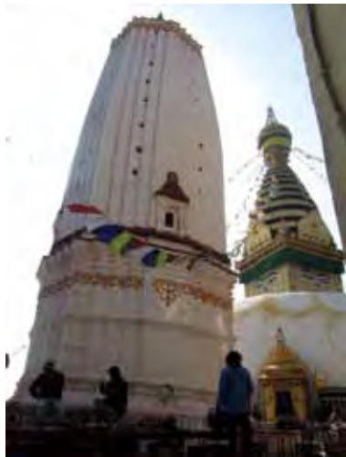
North east elevation after reconstruction of the temple
