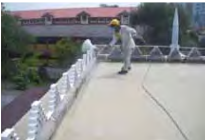
Under the controlled pressure, the concrete flat roofs were sprayed evenly with the epoxy primer (PolyVers PV 350) of elastomeric polyurea.
