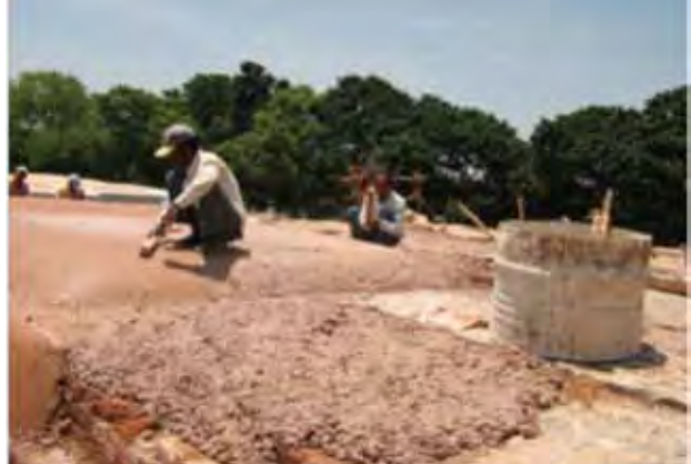
Waterproofing using brick bat and lime to required slopes
