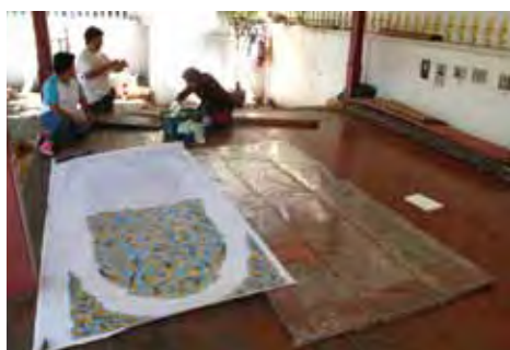
Fig. 5. Processes of corridor ceiling restoration work; Examination and record of each layer of decorations
