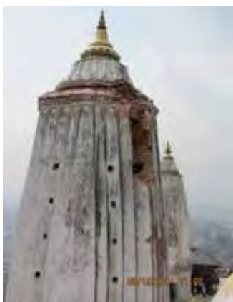
Damaged by the disaster
