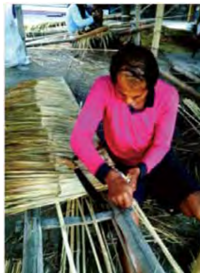
The wooven process of alang-alang using rambatan (small bamboo slat), jalon (bigger bamboo slat) and lulup (rope) done by the local inhabitants for five days on the spot near Omah Gede building which located outside Kabuyutan Trusmi Complex. The Omah Gede reroofing was held about one week after Memayu. The labour was all voluntary work.
