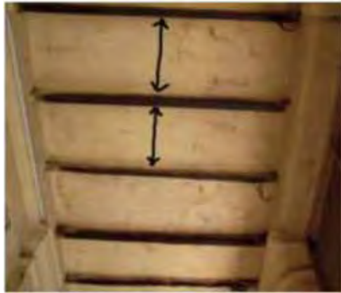
Where the primary timber beams have deteriorated beyond repair, I - beams of calculated dimensions can be inserted. Variation in interspacing causes eccentric loading
