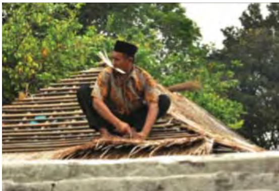
A man were installing the welit directly on the horizontal rafter of one building which has no plugged wooden frame of the thatched roof.
