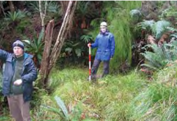
Figure 27. Foundations of the Winch House obscured by vegetation (NZHPT 2007). See Figure 17.
