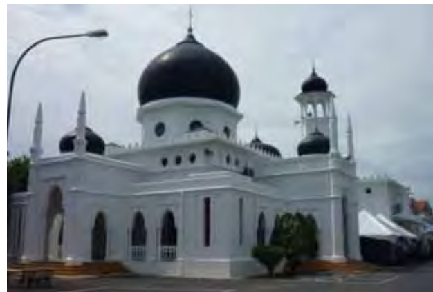
After restoration, the Alwi Mosque has been painted in its original colour which is white, whilst the copper domes in black.
