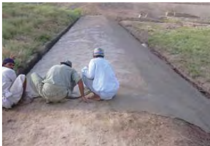
Figure 4. A. The ground level of trench in Mound F stabilized by surface dressing and mud plastering
