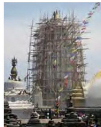
Prepared scaffolding for dismantling the temple
