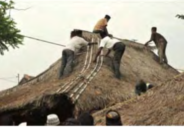
Dismantlement of the upper ridge ( bubungan ) and hip ( jurai ) before reroofing Only men who are descendants from Kyai were allowed to climb the roof.
