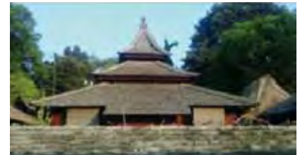
Building with sirap roof
