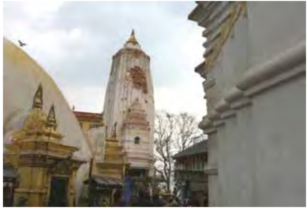
Damaged northwest part
