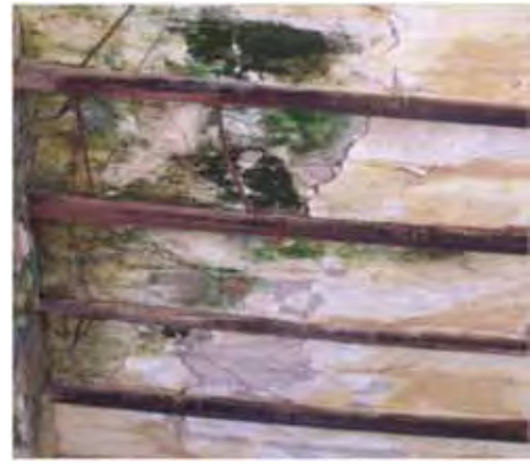
Vegetation growth and penetration of its roots allows seepage of water and debonds the joists from the ceiling
