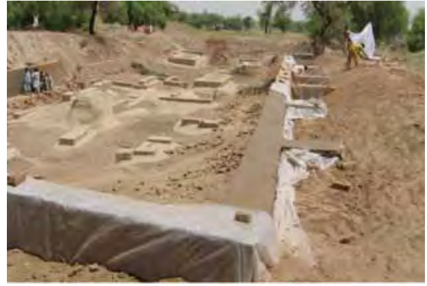
Figure 2. B. Construction of retaining walls in progress to protect sections of the trench. Mound F
