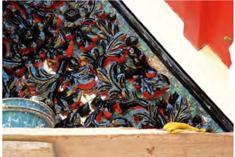
Fig. 8. The gable restoration work; The original materials in white and previous redecoration green glass mosaic were preserved under the new colour of white glass mosaic.
