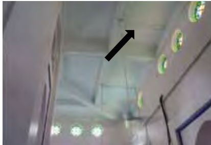
Falling dampness could be seen on the concrete-plastered ceiling of the Alwi Mosque.
