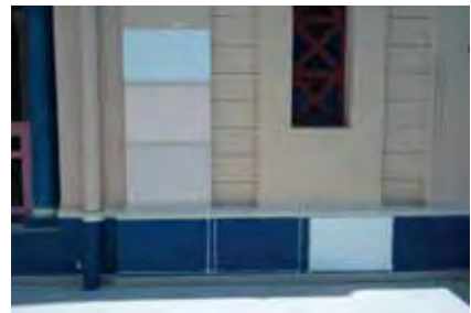
Prior to repainting works, several mockups of different types of off-white paints were set up on the exterior walls of the Alwi Mosque to determine the most suitable type of paint.
