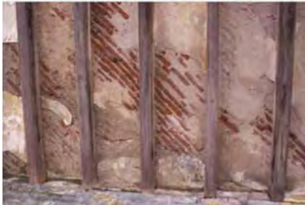
View of a Madras Terrace Roof ceiling
