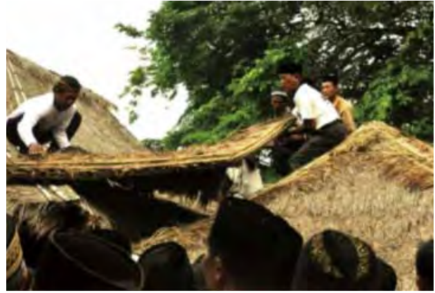
Dismantlement of a part of thatched roof together with the wooden frame
