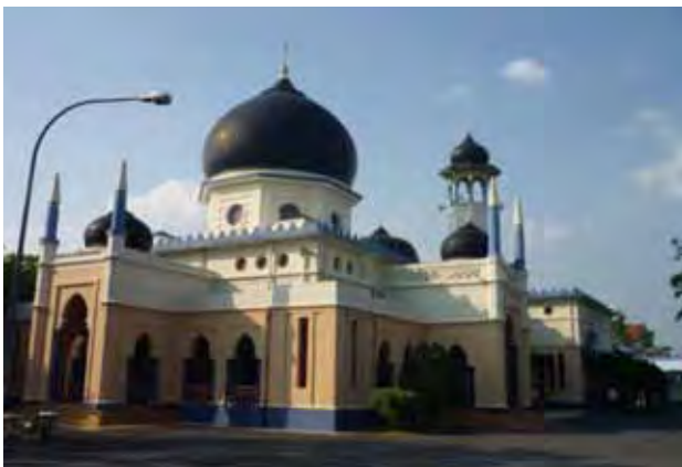
Before restoration, the Alwi Mosque has been painted in several layers of paint of different colours including blue, cream yellow, light orange, white and black.
