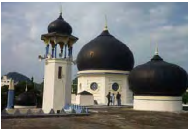
Due to severe leakages found on its flat roof, the Alwi Mosque faced two related building defects namely falling dampness; and cracks on concrete-plastered ceiling.
