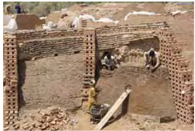
Figure. 3. B. Soil beneath a late Harappan wall strengthened by applying mud pusha Mound AB
