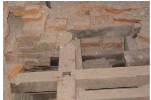
On the process of dismantling the temple
