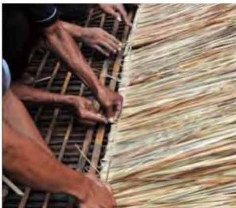
Knitting new welit to the wooden frame with rob made from young bamboo thin slat
