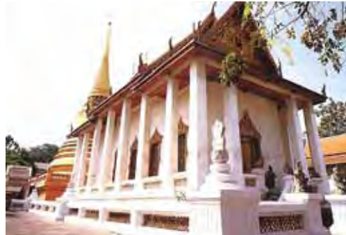
Fig. 2. The exterior decorations of Ubosot before restoration in 2009 (phase 1); corridor ceiling and its wooden frames panel was red and green. Gable and portico of windows and doors were decorated with gilt stucco and colour glass mosaic.
