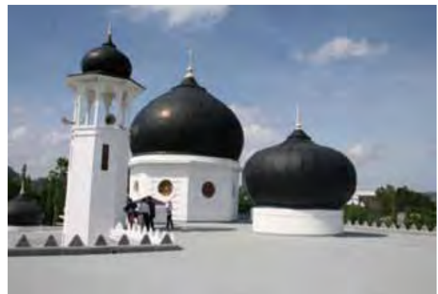
The Alwi Mosque showing its concrete flat roofs after the application of waterproofing system.
