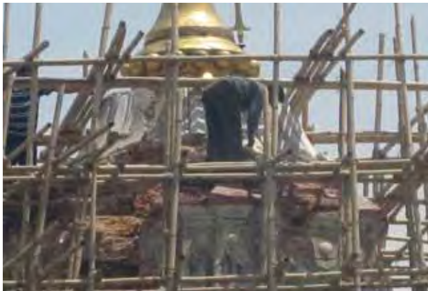
On the process of dismantling the temple on the top (Pinnacle)
