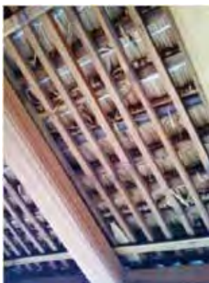
Building with thatched roof made from woven grass ( welit )
