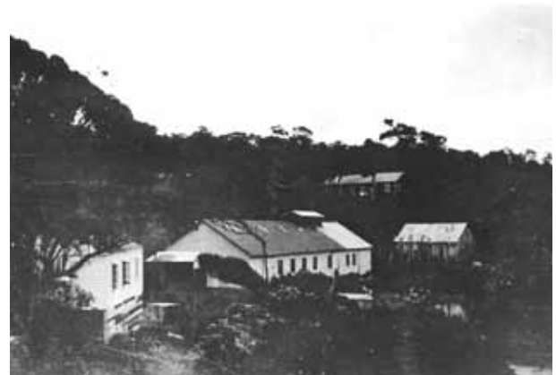
Figure 4. The Base ca. 1926-1932 showing the cookhouse (far left), workshop (centre), carpenter's shop (far right) and bunkhouse (top, in the bush above the working area of the base) (Photo: Southland Museum & Art Gallery).
