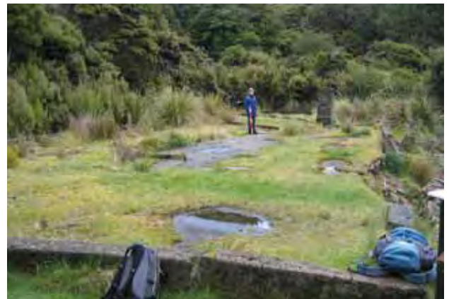
Figure 20. Foundations of the workshop (NZHPT 2007). See Figure 17.
