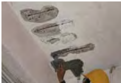
Crack repairs on the concrete-plastered ceiling involved the application of anti-corrosion coating to the exposed reinforced bars.
