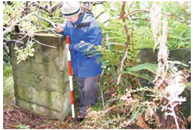
Figure 18. Foundations of the Managers' house showing the entranceway (NZHPT 2007). See Figure 17.
