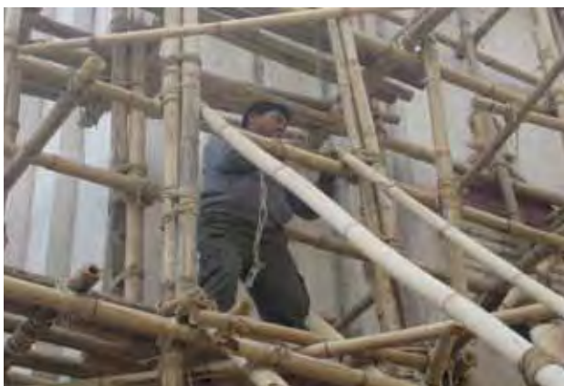
Preparing scaffolding for dismantling the temple
