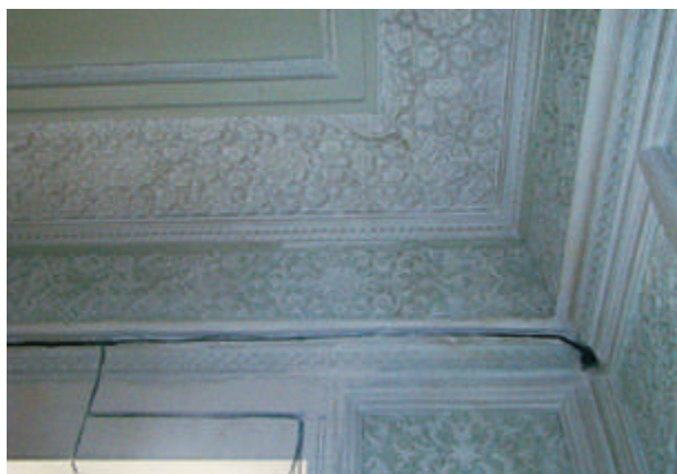
2. Cracks above cornice on the wall.
