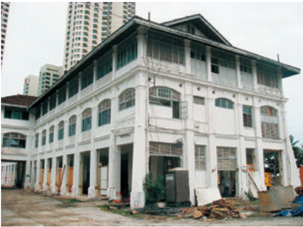
A buttress-type structure can be seen at each corner of the St. Joseph's Novitiate.
