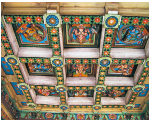
Before dismantling and removal of colored paint pigments
