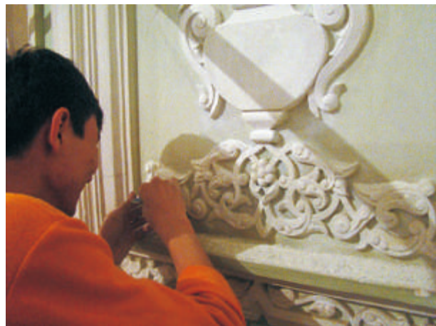
9. Process of restoration works.
