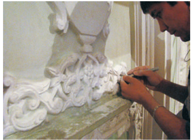
8. Process of removing color layer.
