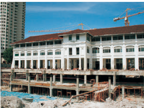
The construction of two levels of basement car parks underneath the St. Joseph's Novitiate was based on the underpinning process, a solution adopted to provide the new pile foundations.
