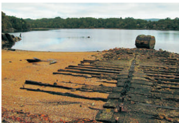
Figure 26. The slipway exposed at low tide showing the timber and concrete construction. The boiler from the workshop lies where it was abandoned in 1946 (Photo: NZHPT).
