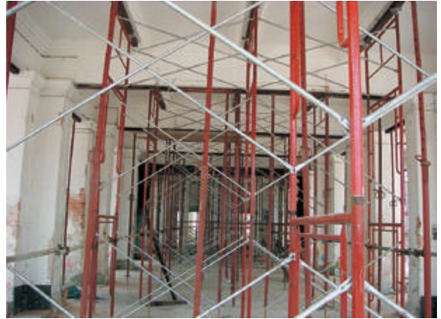
Temporary propping at the ground level of the St. Joseph's Novitiate during the construction of basement car parks.
