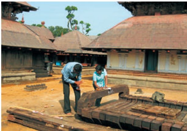
Condition assessment of the wooden members belonging to the sloped roof system
