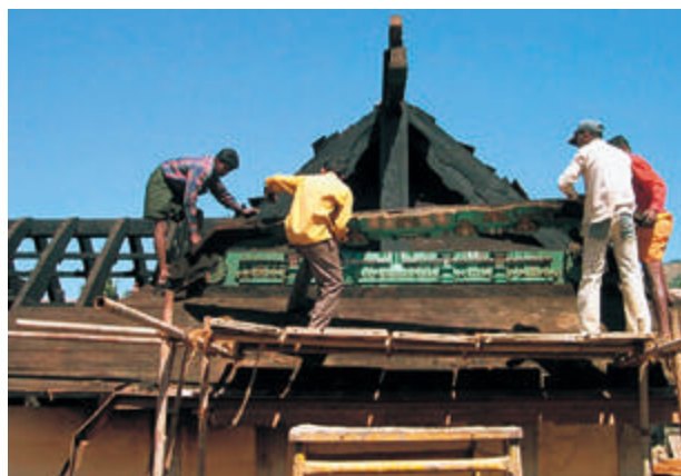
Dismantling of the gable after cataloguing under progress to re-carve /repair the members as well as remove oil paint
