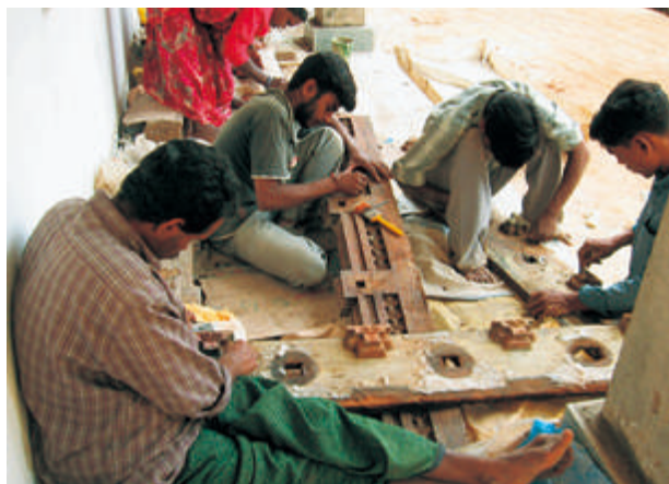
Cleaning of the ornamental details and removing the colored paint pigments
