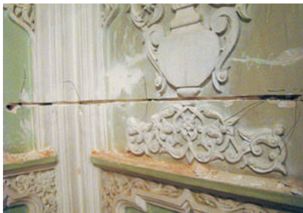
4. Part of ornaments and cornice with cracks.
