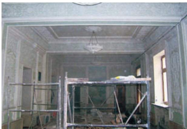
1. General view of Tashkent Hall before restoration.
