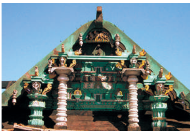
The elaborately treated gable ends of the sloped roof whose several members were deteriorated from inside due to insect attacks
