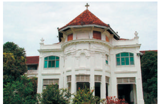
In 1925, the St. Joseph's Novitiate was further extended by the construction of a chapel attached to the middle section of the north elevation in a European Baroque style.
