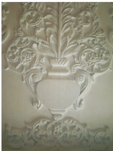
11. Part of Ganch panels after scrape.
