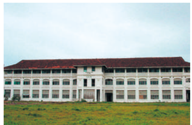
View of the south elevation portraying the repetitive windows, keystones and pilasters that reflect the image of an educational institution.
