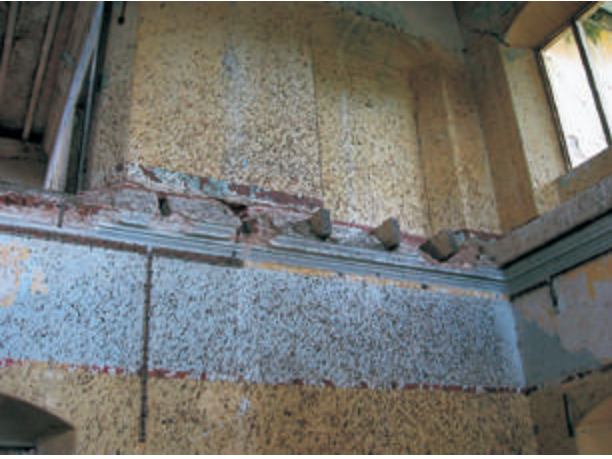
7. Timber Beams were stolen
