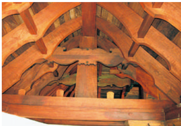
The wooden structural system of the sloped roof after restoration- repairs, cleaning, anti-termite treatment,
