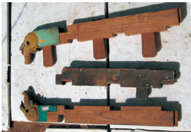
Retaining the original carved details and replacing only the dilapidated support system where necessary using original wood from other discarded larger members to retain authenticity
