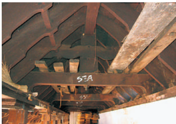
The wooden structural system of the sloped roof before restoration - an interior view
