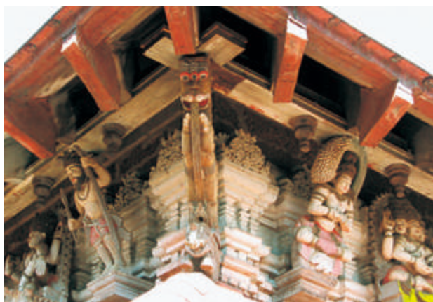
Wooden figures and figurines found below the sloped roof that required removal of paint and spot repairs
