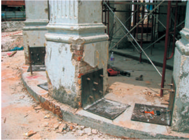
During the construction of basement car parks, L-shaped steel plates were bolted onto the existing column bases and the newly cast ground beams.
