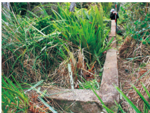
Figure 9. The foundations of the Managers House after vegetation clearance (Photo: NZHPT).
