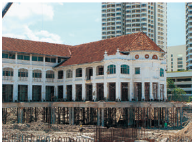
View of the St. Joseph's Novitiate standing independently in the middle of an open field supported by series of micropile shafts, a one-of-a-kind engineering feat in the country.
