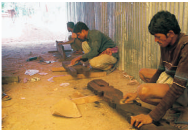
Carpenters recycling the original wooden members of the sloped roof system-cleaning, re-polishing and attaching new members to deteriorated portions maintaining the original joints
