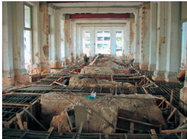
Prior to the construction of the new pile foundation, a new ground floor of concrete slab-and-beam system was introduced to support the existing brick columns.
