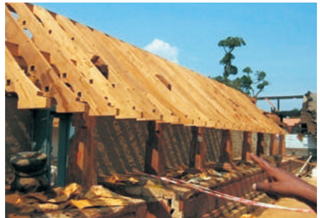
Parts of the inner prakara sloped roof system that is totally replaced by new wooden members
