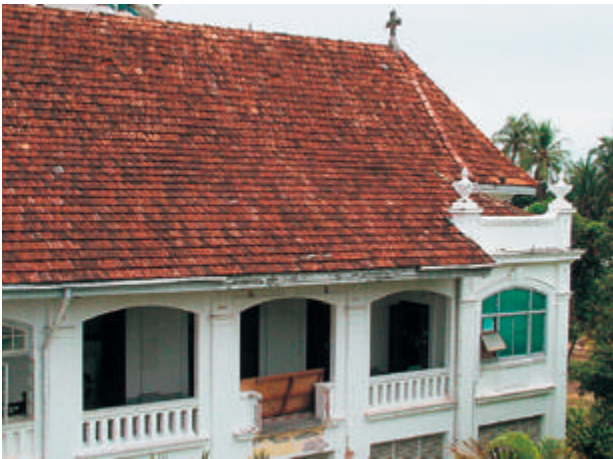
Condition of the Chapel before restoration.
