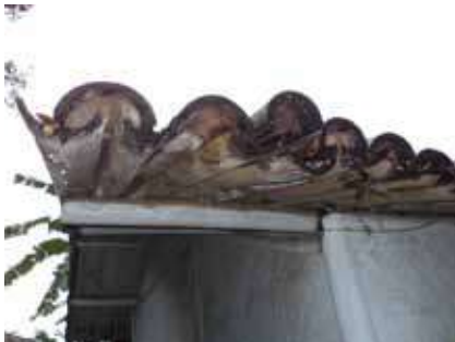
Detail of the bamboo construction on the roof (the talahap)(Documentation: BPCB Serang)
