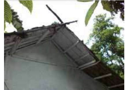
The roof cover consists of two layers. (Documentation: BPCB Serang)
