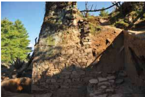
Fig. 11 Excavated area at main entrance
