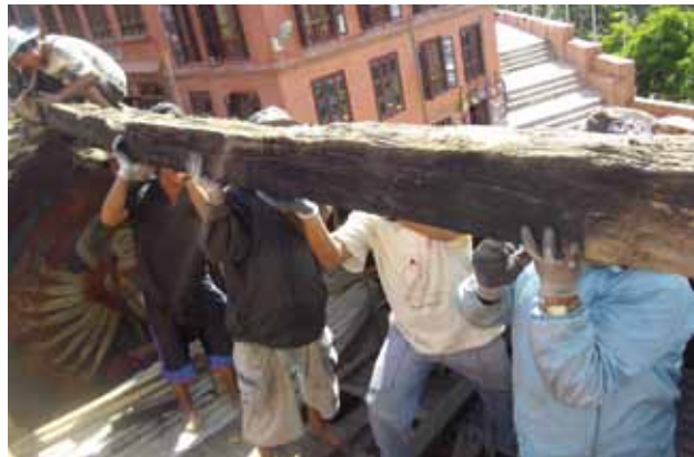
6. Rotten one of teh beams
