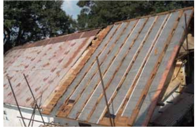
10. Using water proof material : just above the wooden planking
