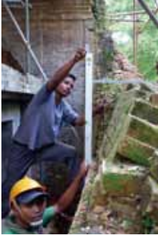
Fig 6. Structure survey (Photo: Hin Sophorn)
