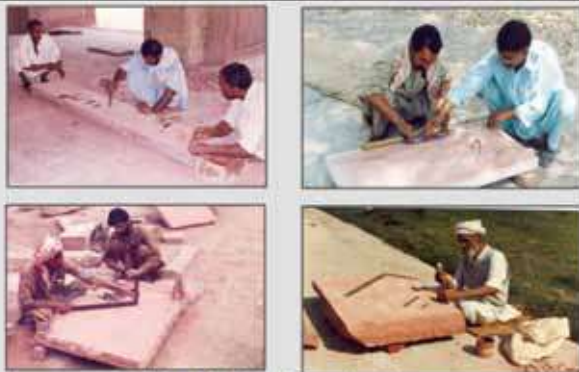
Traditional Method of Stone Leveling
