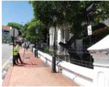
With a special coding system and symbol, external and internal target placements were scanned using stationed 3D terrestrial laser scanner.
