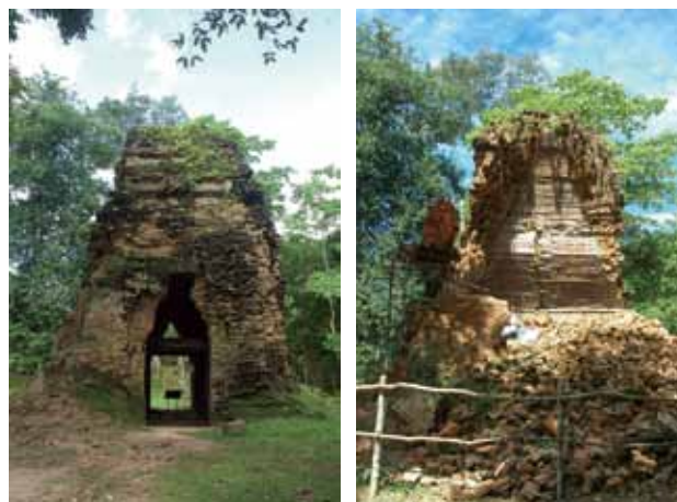
Fig 1 & 2. S2 Tower before and after collapse on July and August 2006 (Photo: Chan Vitharong/SCP)
