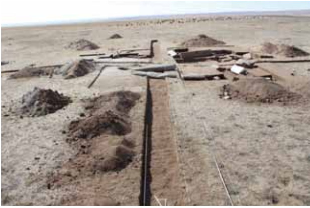
Fig. 4. Excavation trenches at the site
