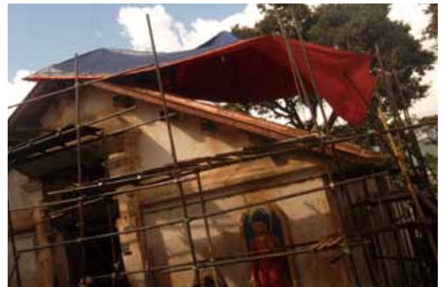
15. Two sides partially (one third) complete roof conservation work
