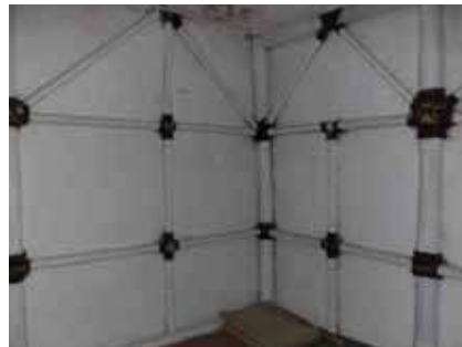
Construction of the wall (Documentation: BPCB Serang)
