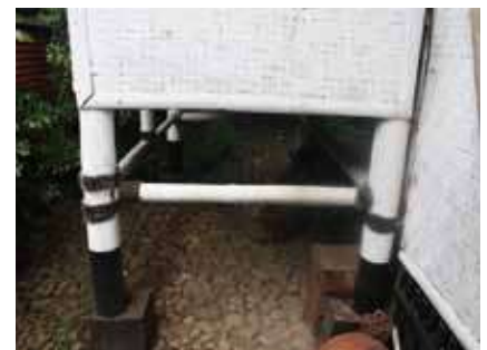
Detail of pillars on the bottom (Documentation: BPCB Serang)
