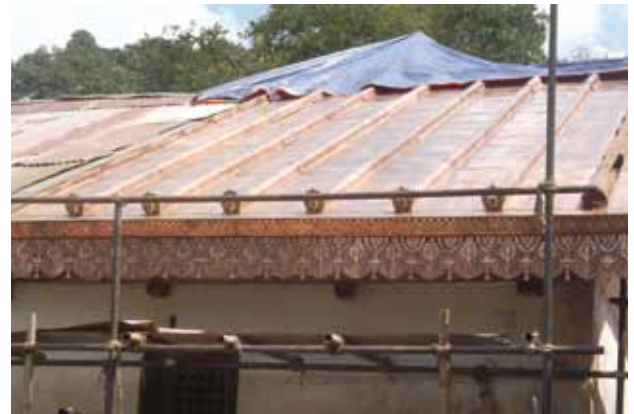
12. One side complete roof work
