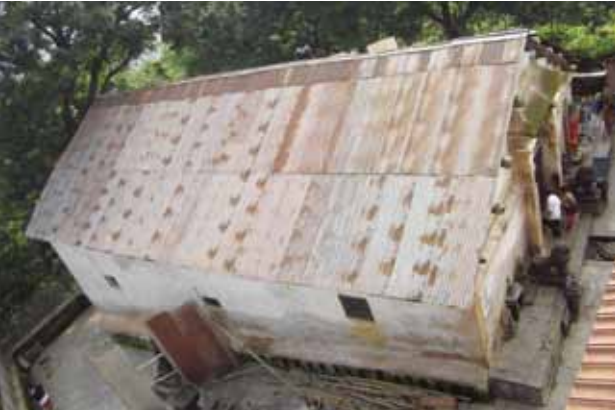
1. Before conservation of the roof
