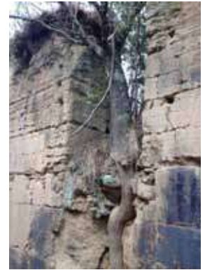
Fig. 10 Inner rammed earth walls
