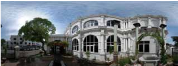
Panoramic photography technique was used to document the building as it captured everything at site.
