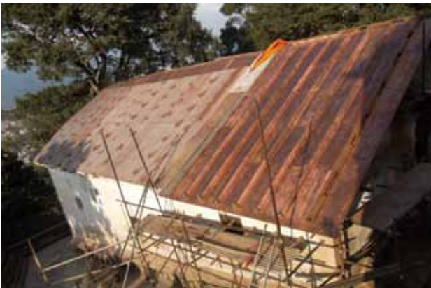
14. A partial completed roof conservation work
