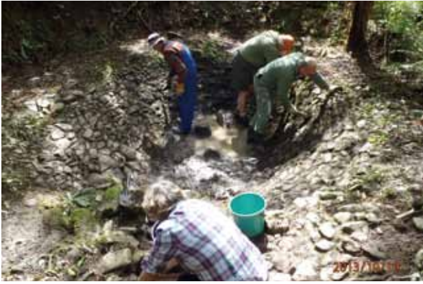
Figure 21. Excavation of the Lower Pond (Photo: NZHPT)
