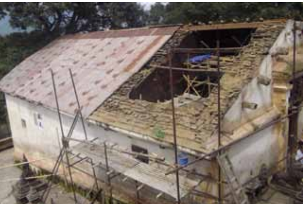
3. One part of the roof after taking off zinc sheets
