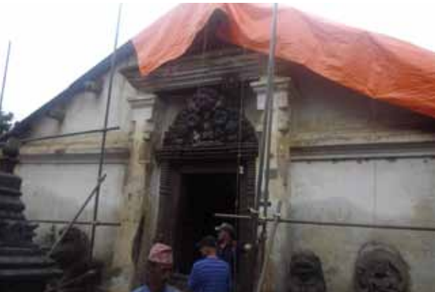
5. Covering to protect from rainwater: during conservation work
