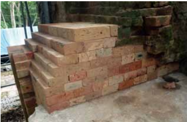
Fig 9. New brick materials have replaced to support the structure (Photo: Hin Sophorn)
