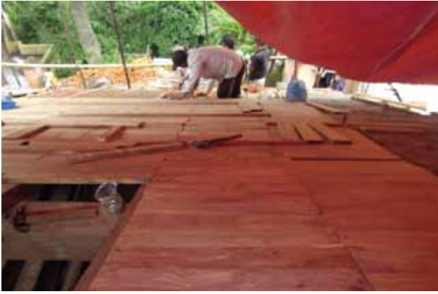
9. Wooden planking for copper sheet roof
