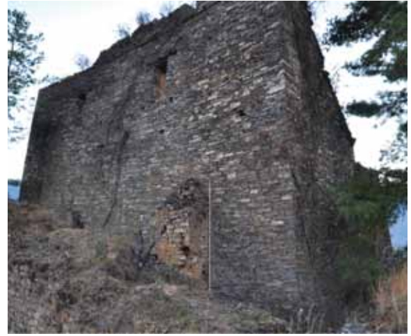
Fig. 5 View of Central tower (Utse)
