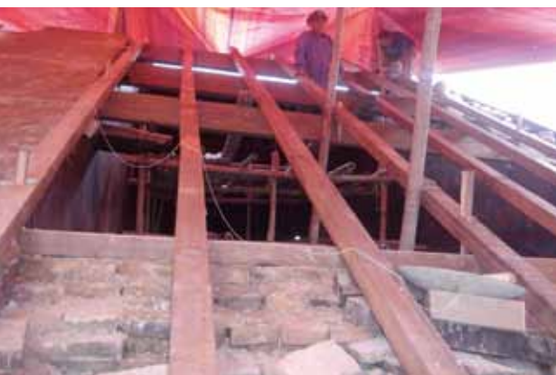
7. Preparing rafters for new roof
