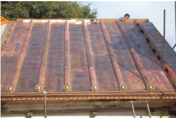
11. Copper sheets: final roof (above water proof material)
