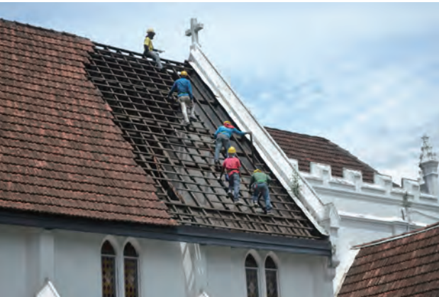
Existing Marseille roof tiles were carefully removed in batches, brought down and cleaned at site before they were re-installed on the roofs
