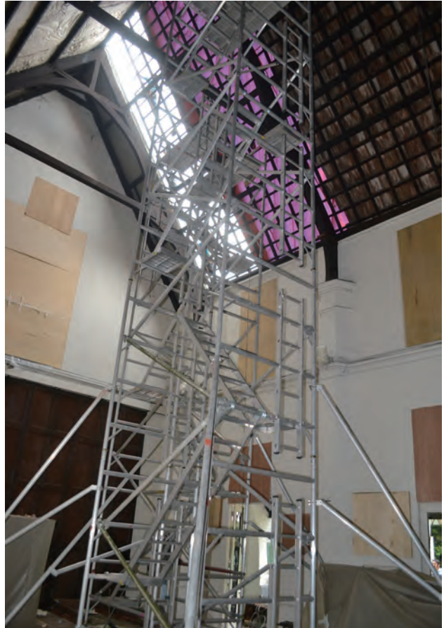
Mobile temporary scaffolding was set up inside the main hall to provide a strong working platform for installing a layer of acoustic treatment on the ceiling and for changing the rotten timber batten on the roof
