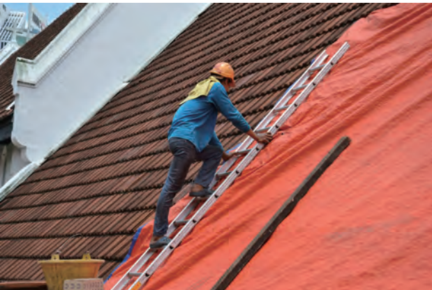
Waterproof plastic sheet covers were used to protect the exposed roof structures during rainy days
