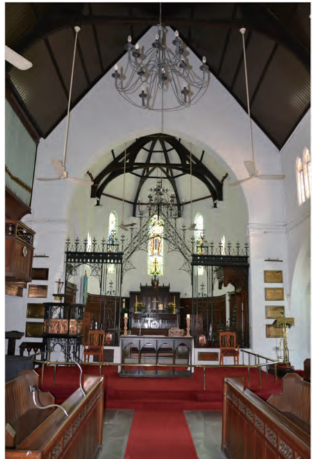
The interior of the main hall after conservation with the new acoustic control layer and metal strips linear ceiling
