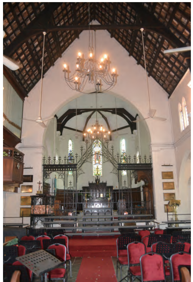
The interior of the main hall before conservation, with Marseille roof tiles and timber battens able to be seen from inside
