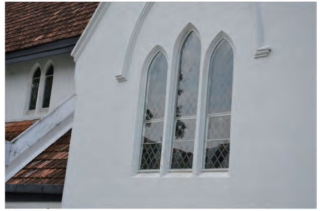
All stained glass lancet windows were fitted with an additional glass panel in order to minimise noise disturbances
