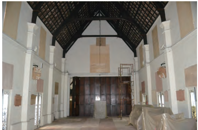
Prior to the conservation works, all furniture and electrical fixtures in the main hall were removed, the organ and pulpit were covered with plastic sheets and the interior floors were protected with plywood sheets to prevent any damage during construction
