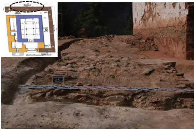
Fig. 8 Old remains of stone foundation discovered on the western side (2.8m thick wall)
