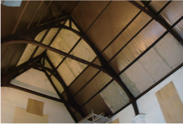
The installation of an acoustic control layer and metal strips linear ceiling at the main hall during construction
