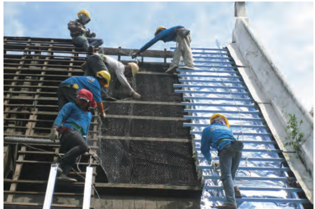
For energy efficiency and noise reduction, the roof structures were insulated with wire netting, rock wool and aluminum foil
