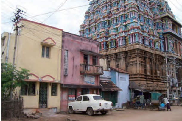
Houses and other public/private buildings encroach the historic monuments
