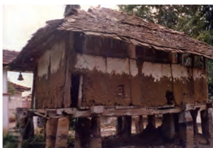
(Fig 1) Wattle and daub building, 19 th century AD
