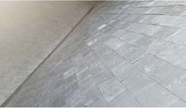
View of the pitched roof of the City Hall Building after the installation of the stone slate tiles.
