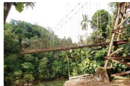
(Fig 125) Suspension bridge, Deraniyagala, 19th-20th centuries AD
