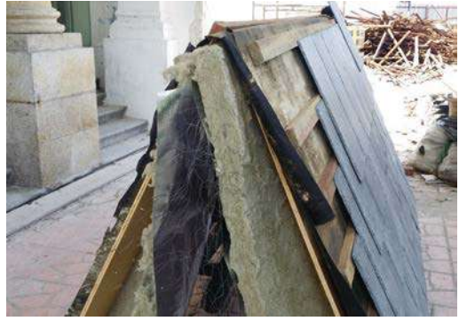
A full-size mock-up of a roofing system using timber structures and stone slate tiles was set up at the City Hall Building prior to any installation.
