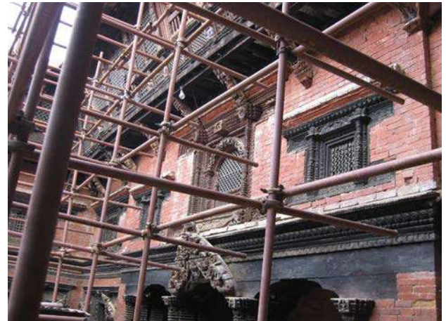
Scaffolding During Conservation
