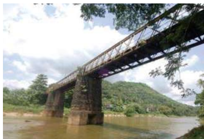
(Fig 124) Steel bridge, Yatiyantota, 19th-20th centuries AD
