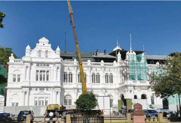
Once the installation of the stone slate roof tiles was completed, the temporary roofing was carefully dismantled and removed using a telescopic hydraulic crane.
