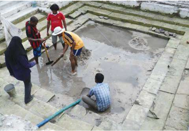
Figure 4: Removal of the spoil heap with spades after water has been drained out
