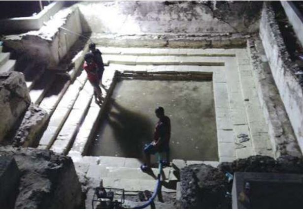
Figure 2: Condition of the bathing tank after DOH's excavation and cleaning
