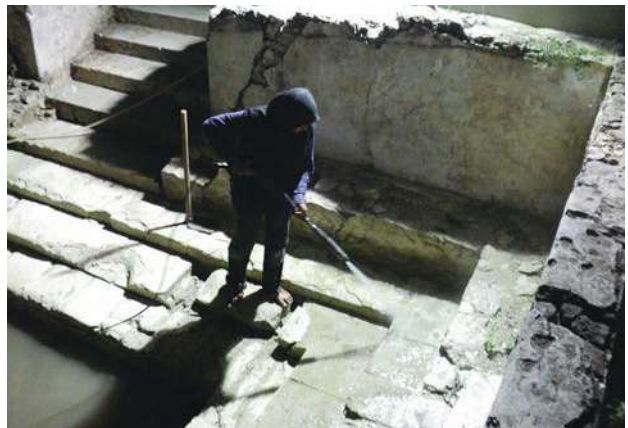
Figure 7: Cleaning the stones with a Karcher pressure washer
