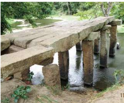
(Fig 121) Stone bridge, Malwathu Oya, Anuradhapura period
