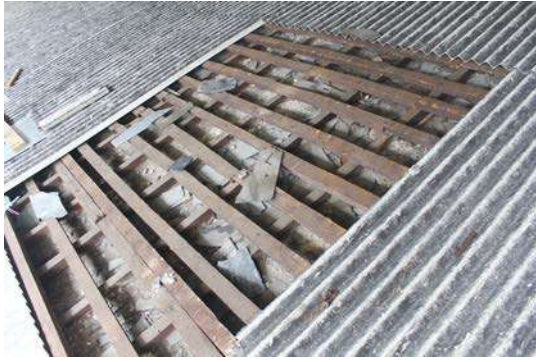
Once the corrugated asbestos sheets were removed, broken pieces of the original stone slate tiles were found scattered on the timber planks.
