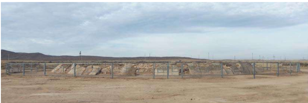
View after finish of work
