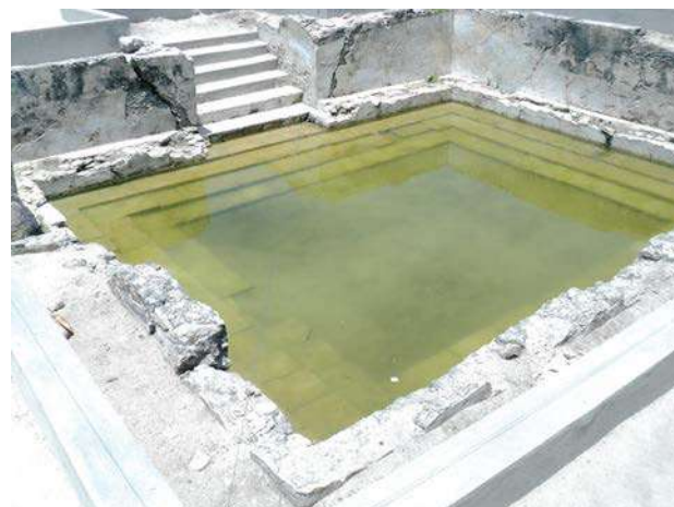
Figure 1: Condition of the bathing tank after MNDF's excavation
