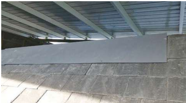
Powder-coated galvanised iron, in a grey colour similar to the colour of the stone slate tiles, was used for the roof ridge cap.
