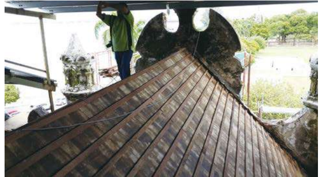
New 2.5 cm x 5.0 cm battens were fixed at 17.5 cm intervals, starting from the lowest end of the roof, over the new roofing felt (bitumen).
