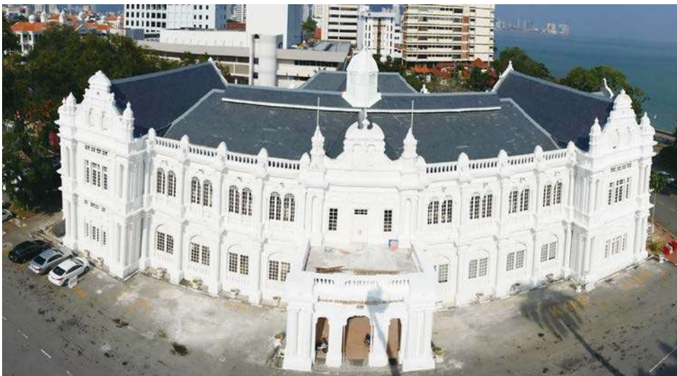
Aerial view of the City Hall Building after installation of the stone slate roof tiles.
