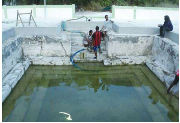
Figure 3: Preparation and placing of water pump to drain the water out
