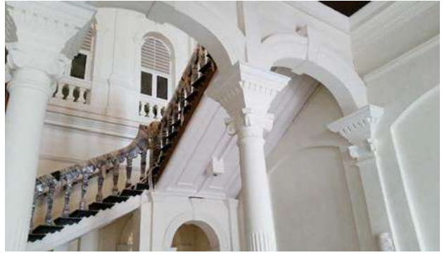
Interior view of the City Hall Building after restoration.
