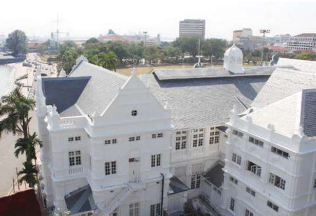
Aerial view of the City Hall Building showing the newly installed stone slate roof tiles and back elevation after restoration.
