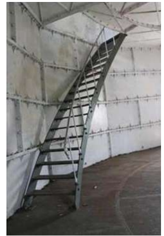
Stairs that connect the floors (Documentation: BPCB Serang)
