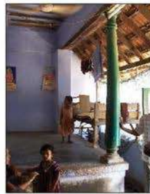
WOODEN COLUMN WITH STONE BASE
