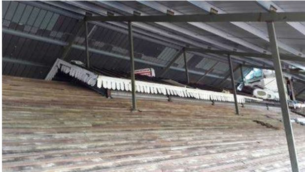
The restoration of the roofs began with an inspection of existing timber planks, rafters, battens and plywood boards once the existing corrugated asbestos sheets were dismantled and removed.
