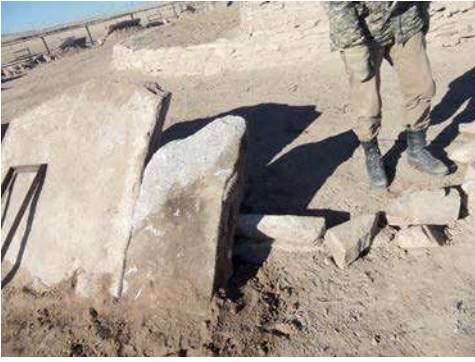
Installing panels for fence No 1
