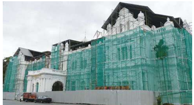
View of the City Hall Building showing its temporary roofing during restoration.
