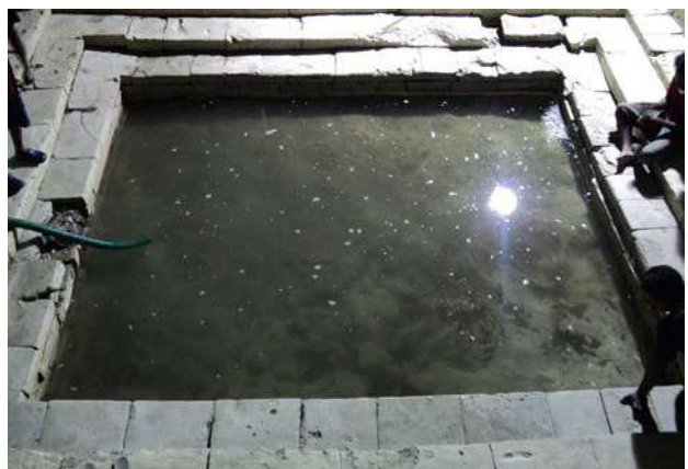
Figure 9: Stones and water after cleaning.
