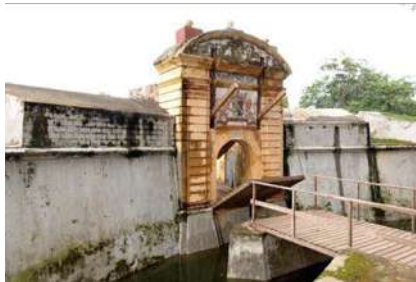
(Fig 98) Timber Draw Bridge, Matara Star Fort, 18th century AD
