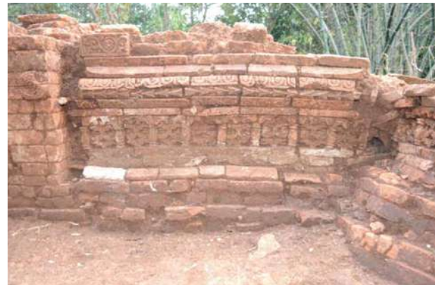
Northern wall: close up view
