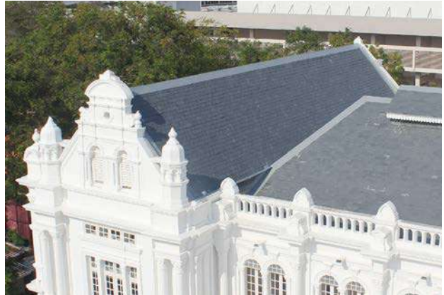
Close-up view of the newly installed stone slate roof tiles at the City Hall Building.
