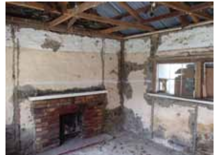
Figure 25. Interior of main cottage bedroom 1 and 2 showing modern fire but 19 th century style window on the right wall (Photo: Matthew Schmidt).
