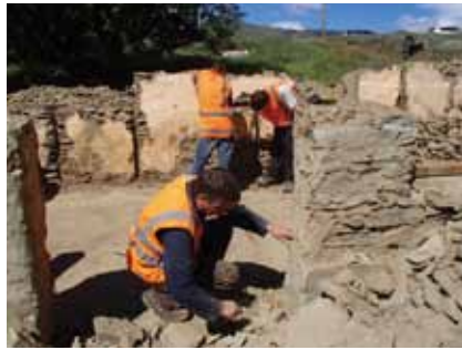
Figure 33. Stonemasons preparing the walls (Photo: Matthew Schmidt).
