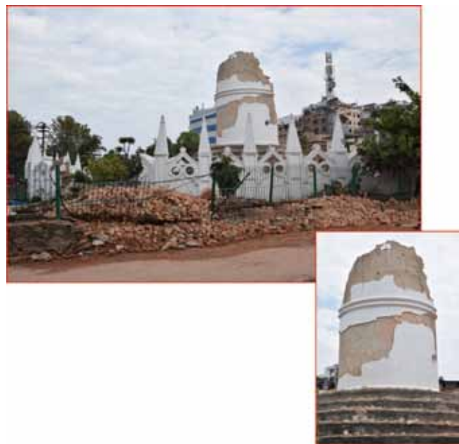
Collapsed Dharahara during the first earthquake on 25 th april 2015— outside the boundary of a World Heritage Property in the Kathmandu Valley
