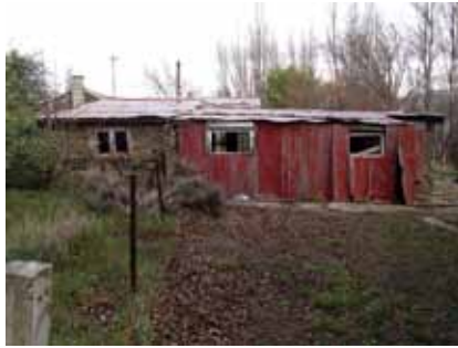
Figure 21. Back of later stone lean to and corrugated iron 'store' (Photo: Matthew Schmidt).
