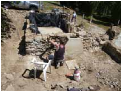
Figure 45. Repointing underway on one of the back walls of the main cottage (Photo: Steve Holmes).
