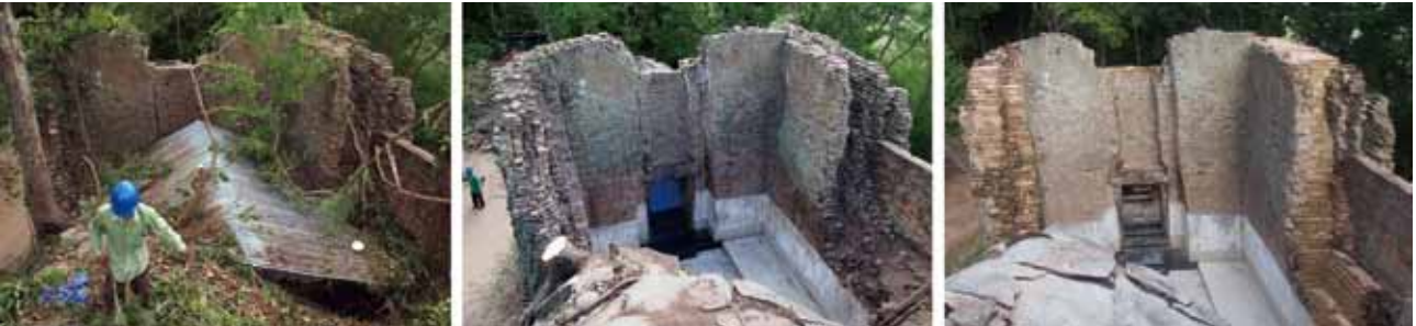
Fig. 10: The interior wall before and after restoration work
