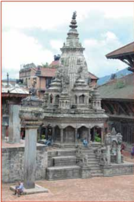
Vatsala Temple before earthquake—Bhaktapur PMZ
