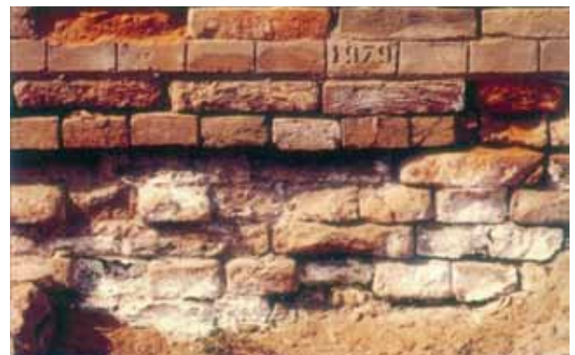
Base of a Wall showing the horizontal damp-proof course at Moenjodaro
