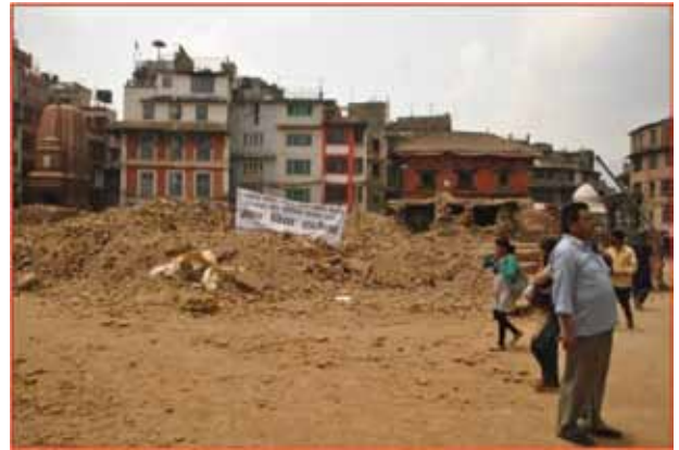
Completely collapsed Kasthamandapa due to the earthquake—hanumandhoka PMZ
