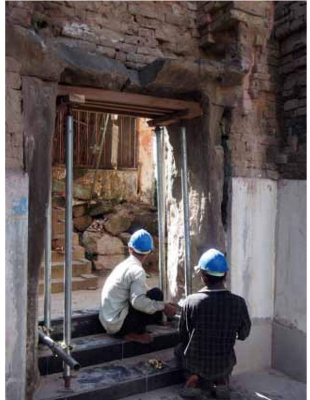
Fig. 6: Emergency support installation for the doorway
