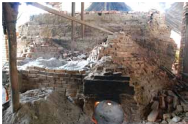
The roof clay tiles are stacked in several layers above the ground in the earthen kiln, which is also covered with bricks to retain heat.
