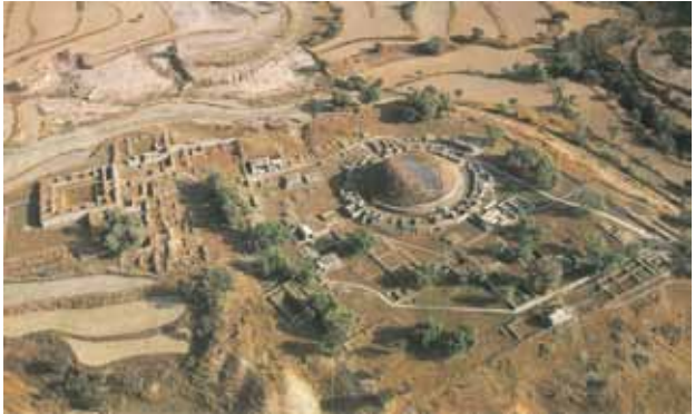
Dharmarajika stupa after conservation work
