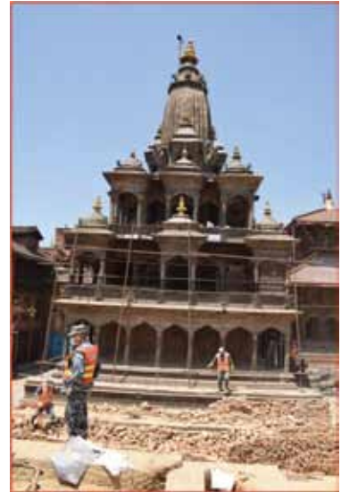
Completely collapsed Narasingha Temple due to earthquake, close to Krishna Mandir— Patan Durbar PMZ
