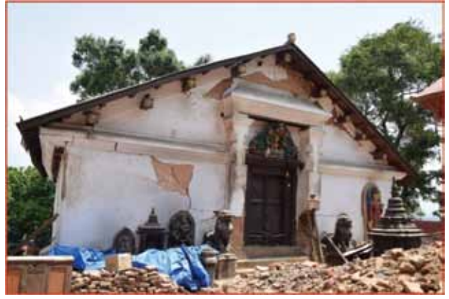
Partially damaged Shantipur Temple due to the earthquake—Swayambhu PMZ
