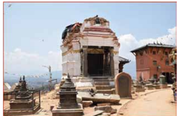
Partially collapsed Anantapur Temple due to earthquake—Swayambhu PMZ
