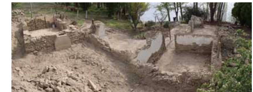
Figure 39. View over site from behind Main cottage and Bedroom 1 & Living room after partial demolition and vegetation clearance completed. Ready for stonework. (Photo: Matthew Schmidt).
