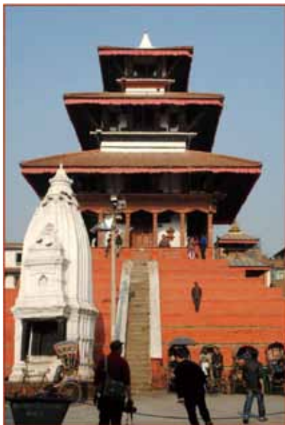
Maju Dega before earthquake—Hanumandhoka PMZ
