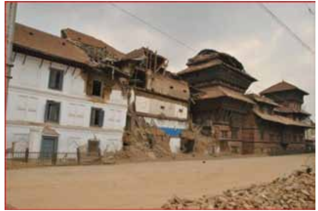
The buildings of Hanumandhoka Palace Complex after earthquake
