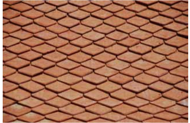
The overlapping arrangement and repeated pattern of Singgora roof tiles resembling fish scales.
