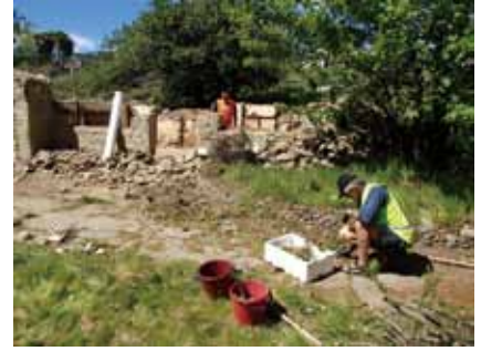
Figure 31. Stonework being prepared and vegetation being cleared during partial demolition (Photo: Matthew Schmidt).
