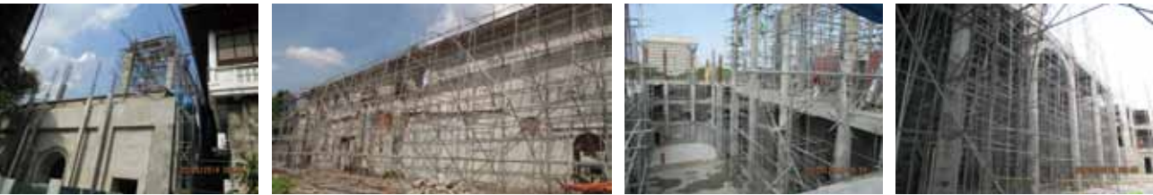
Reconstruction of the façade, exterior, and interior walls of the church (2014, IA Photos)
