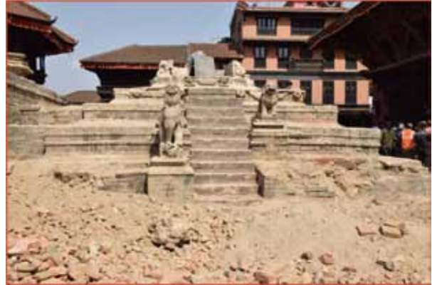
Vatsala Temple after earthquake—collapsed due to earthquake
