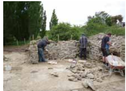
Figure 46. Repointing underway on the main cottage (Photo: Steve Holmes).
