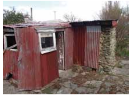
Figure 22. Later corrugated iron framing added to original 19 th century schist stone 'store' room (Photo: Matthew Schmidt).
