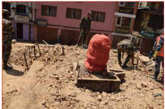
Char Narayan Temple completely collapsed in the earthquake—Patan Durbar PMZ
