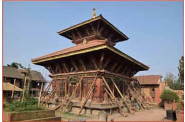
Changunarayan Temple still surviving during and after the earthquake—immediate protection was needed—Chanagunarayan PMZ
