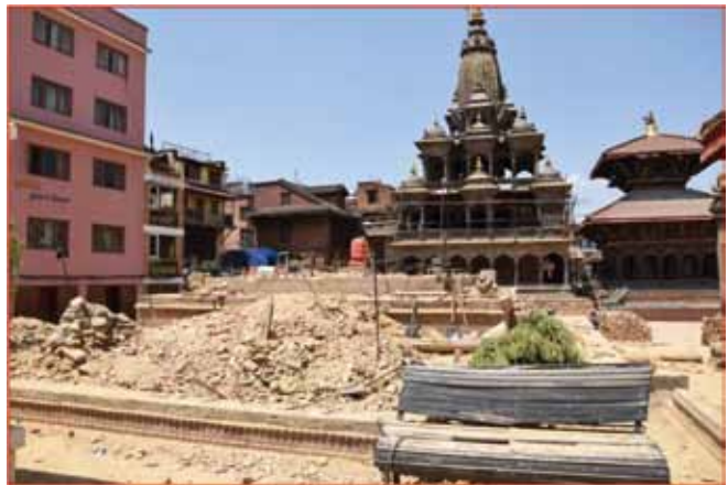
Completely collapsed Hari Shankar Temple due to earthquake at Patan Durbar PMZ
