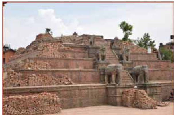
Fasidega collapsed due to earthquake—Bhaktapur PMZ
