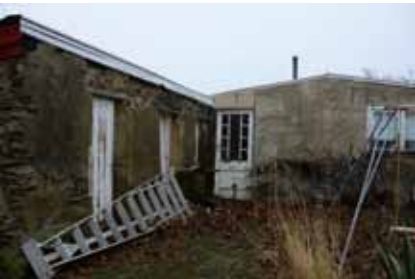
Figure 23. Front of 'store' and 20 th century wooden and rendered living room/kitchen (Photo: Andrew Winter, Jackie Gillies & Assoc's).
