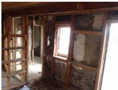
Figure 27. Interior 'store' looking at original stone work right of photo (Photo: Matthew Schmidt).
