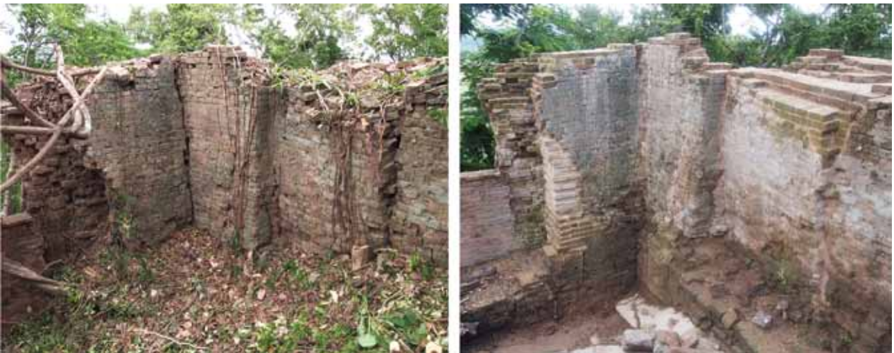
Fig. 11: The east corner of the north wall before and after restoration work
