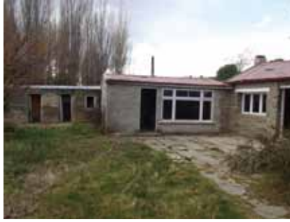
Figure 18. Centre of photo later addition made of timber, far left outbuilding same age as main cottage (Photo: Matthew Schmidt).
