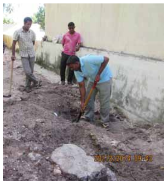
Fig 3: Excavation of Trench 1 by the locals of the island
