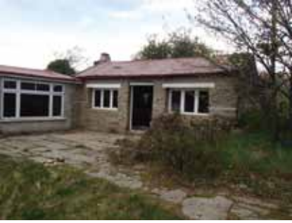
Figure 17. Beattie's cottage before partial demolition. View to main cottage centre and Living room/kitchen to the left (Photo: Matthew Schmidt).
