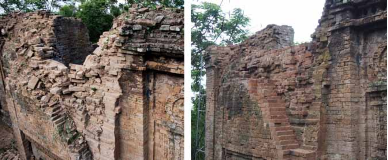
Fig. 9: The front pediment before and after restoration work
