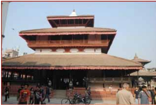
Kasthamandapa before Earthquake
