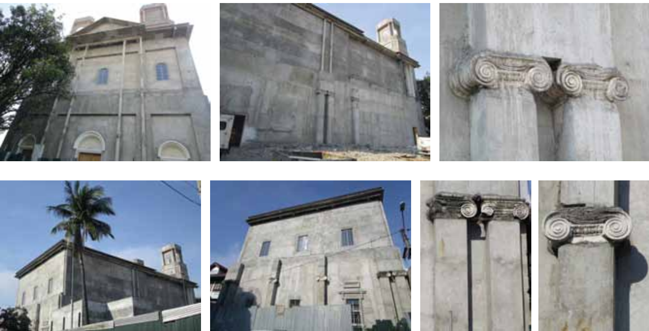
These are recent exterior photos of the church taken by the author (2015). The original columns have been preserved.
