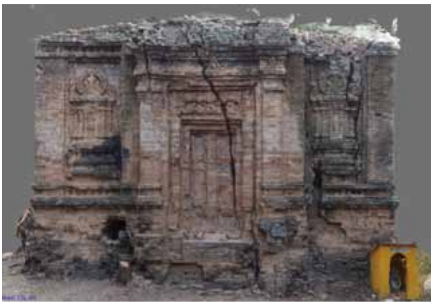
Fig. 5: East façade (before restoration work) created by PhotoScan
