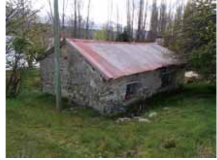
Figure 19. The back wall of the main cottage (Bedroom 2 & 3) before partial demolition.
