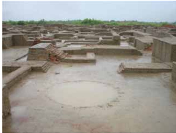
Rainwater penetration into the structure at Moenjodaro
