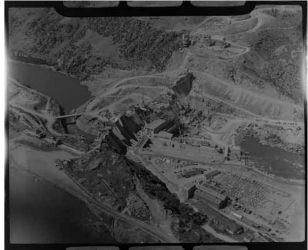
Figure 4. The Roxburgh Dam under construction in 1955. All areas along the river margins were gold mined and gold miners hut sites were present in the rocky landscape. Otago. Whites Aviation Ltd (Photo source: Alexander Turnbull Library Wellington, New Zealand. ref WA-39231-F).
