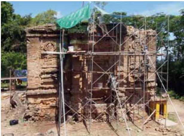
Fig. 7: East façade during restoration work
