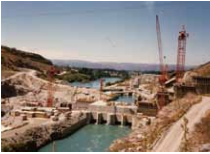
Figure 7. The Clyde Dam under construction, 17/01/1983 (RW Murray Collection held by Matthew Schmidt).
