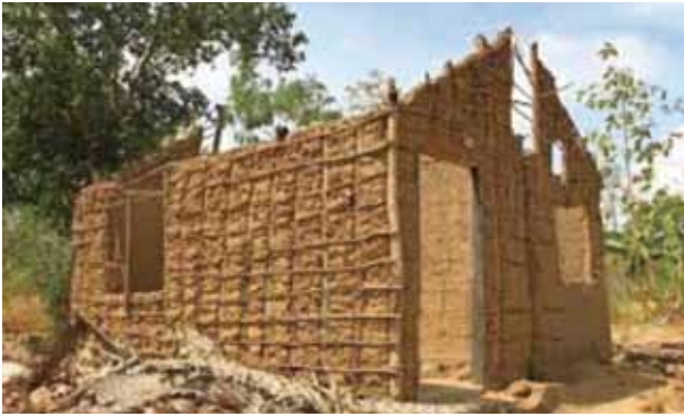
Fig. 6: Wattle and daub construction
