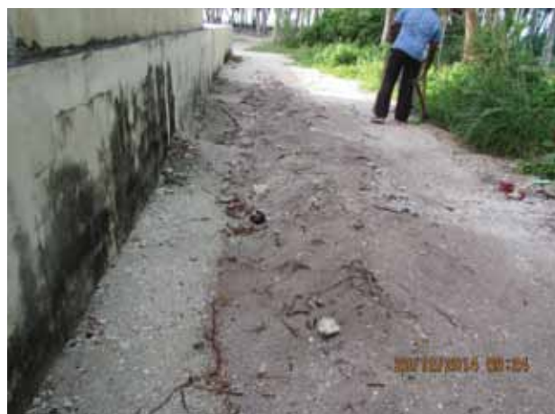
Fig 2: Area before excavation
