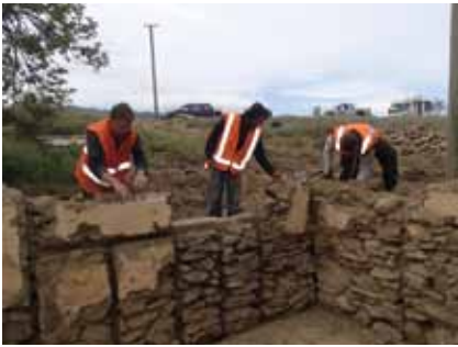
Figure 32. The stone mason class and expert stonemason Steve Holmes preparing the stonework (Photo: Matthew Schmidt).
