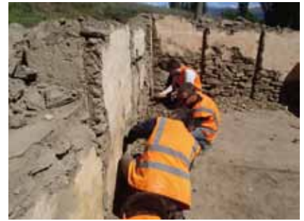
Figure 34. Stonemasons preparing the walls (Photo: Matthew Schmidt).
