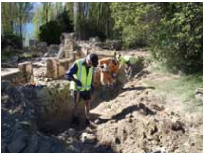
Figure 35. Clearing debris from behind the back wall of the main cottage (Photo: Matthew Schmidt).
