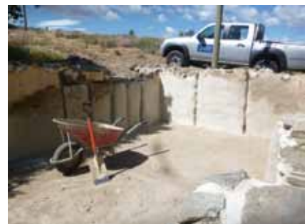
Figure 48. Rendering of the inner walls of the main cottage as they would originally have been. A tougher mortar is used as these walls will now be exposed to the weather (Photo: Steve Holmes).
