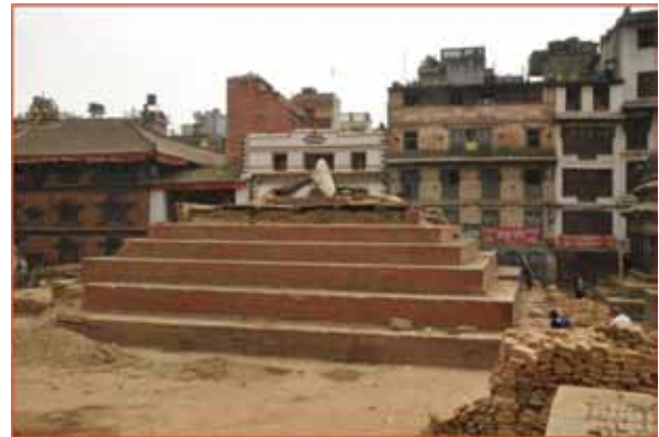
Completely collapsed Narayan Temple due to the earthquake—Hanumandhoka PMZ
