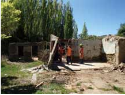
Figure 29. Partial demolition underway (Photo: Matthew Schmidt).
