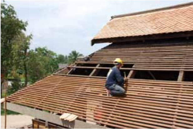
The use of Singgora roof clay tiles during the restoration of Kedai Mulong Mosque, Kota Bharu, Kelantan.
