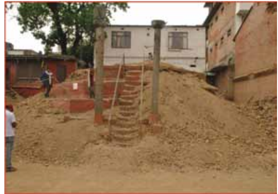
Completely collapsed Chyasing Dega (Krishna Mandir) due to the earthquake—Hanumandhoka PMZ
