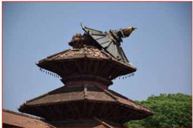
Broken pinnacle of Taleju Temple at Patan Durbar during earthquake
