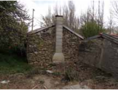
Figure 20. Left side of main cottage showing modern concrete stacked chimney, later stone lean to (right) and 20 th century concrete shuttering to support walls.
