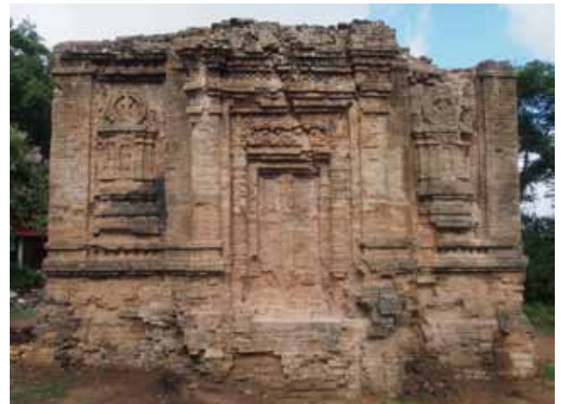
Fig. 8: East façade after restoration work
