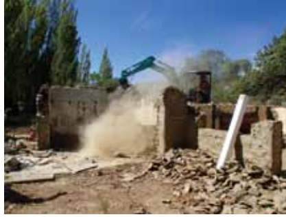
Figure 30. Partial demolition underway (Photo: Matthew Schmidt).
