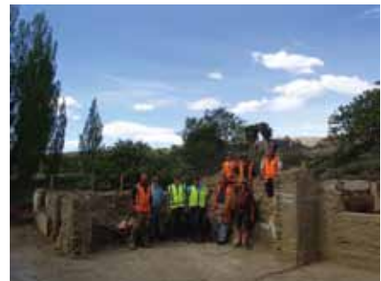
Figure 28. Contractors/Volunteers who worked on the preservation project (Photo: Matthew Sole).
