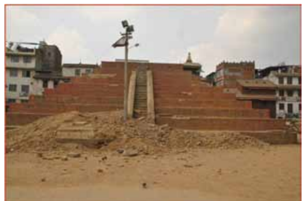
Completely collapsed Maju Dega due to the earthquake— Hanumandhoka PMZ
