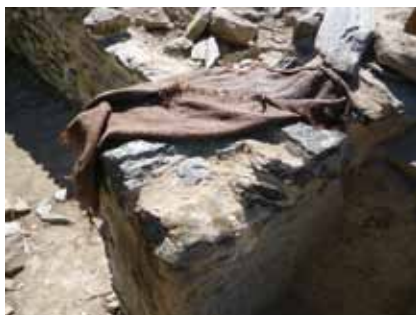
Figure 47. Capping of the stone walls using a hard mortar and pieces of schist (Photo: Steve Holmes).
