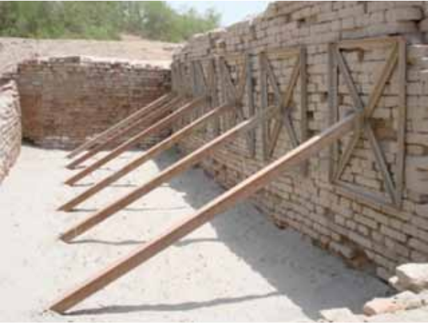
Leaning walls being protected with steel supports at Moenjoaro
