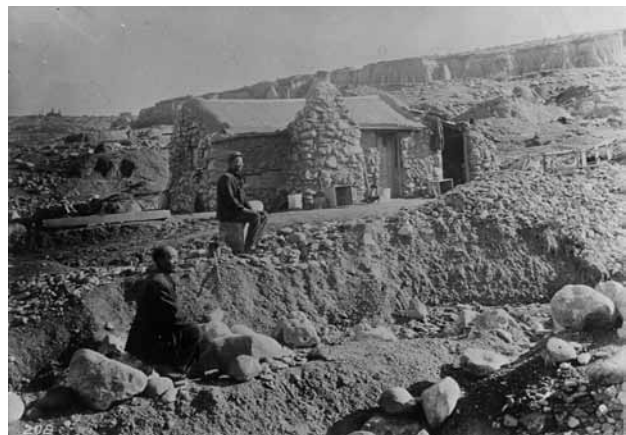
Figure 6. Chinese gold miners in the 19 th century in the Roxburgh Gorge. Settlements such as this were buried under Lake Roxburgh. (Alexander Turnbull Library, Wellington, New Zealand Lib ref 1-4-009945-G).
