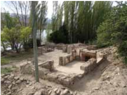
Figure 41. The main cottage (Bedroom 1 and 2) ready for stonework (Photo: Matthew Schmidt).
