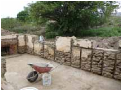
Figure 44. Main cottage walls being prepared for pointing by the stonemasonry class (Photo: Steve Holmes).
