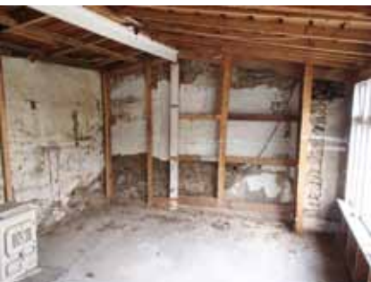
Figure 26. Interior of later wooden living area and kitchen showing earlier schist stone wall in background (Photo: Matthew Schmidt).
