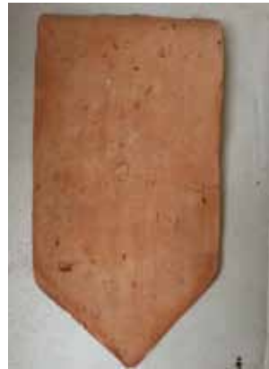
Top view of the rhomboid-shaped Singgora roof clay tile.
