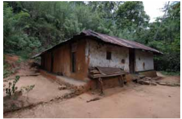
Fig. 3: Ancient house in Meemure village in Central Province – 9 th century. An inability to find traditional roofing materials and in the interests of easy maintenance and durability, galvanized sheets were added during a later period.
