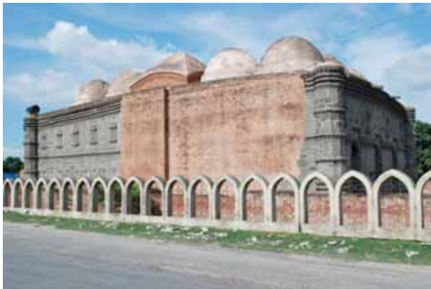
Western wall of the mosque
