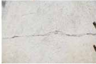
Some cracks developed in the dome of Swayambhu Mahachaitya due to the earthquake—Swyambhu PMZ
