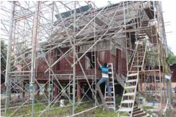
Dismantling the Bugis house.
