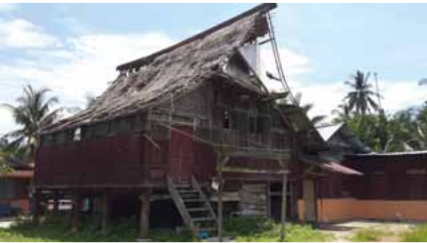
View of the Bugis house in 2014 after it was left abandoned and had deteriorated rapidly due to decayed timber structures, termite infestation, roof leakage and poor maintenance.
