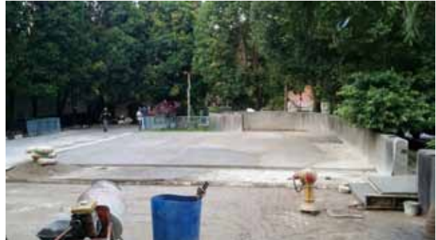
Reconstruction of the Bugis house in the grounds of the Sultan Alam Shah Museum began with the construction of a concrete-mix foundation floor to create a level surface.
