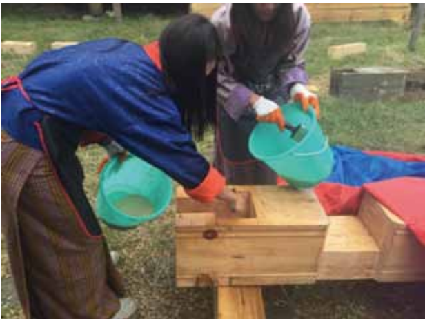
Fig.11 Applying fermented persimmon liquid to new timber components
