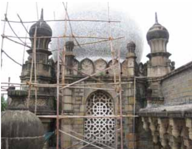
Discoloured masonry wall surface with dirt grime and salt deposits on the left and a cleaned clear surface on the right
