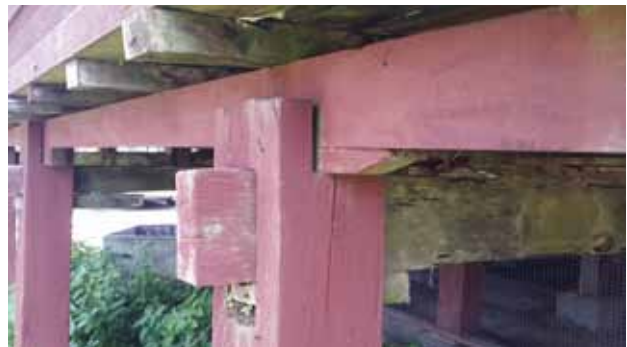
The entire Bugis house was constructed without the use of a single nail but it was locked using timber peg frames and wedges.
