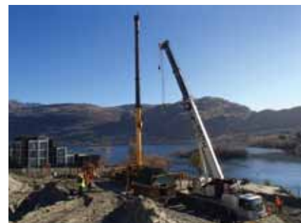
Figure 22. The cranes ready to lift the 59 ton Meat Shed (photo: Matthew Schmidt, HNZPT, 2016).
