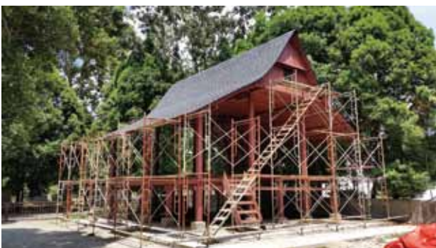
View of the Bugis house during reconstruction.
