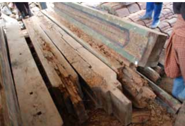
Fig.7 Decayed timber components which were not exposed to the air
