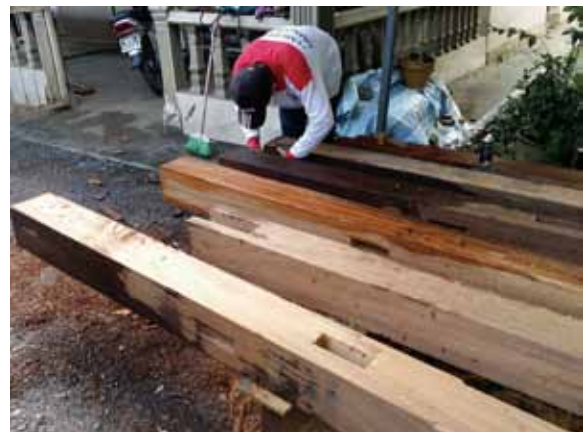
All new and old timber structures were treated against termite infestation.
