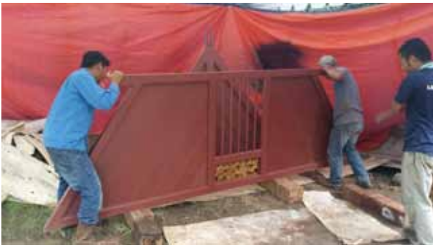
Carpenters handling a newly restored gable end.
