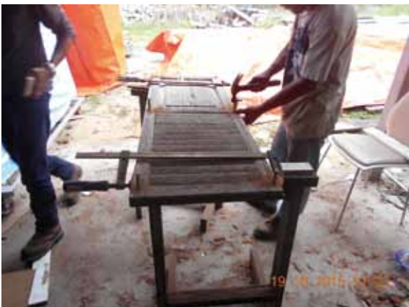
Restoration of casement window panel in progress.
