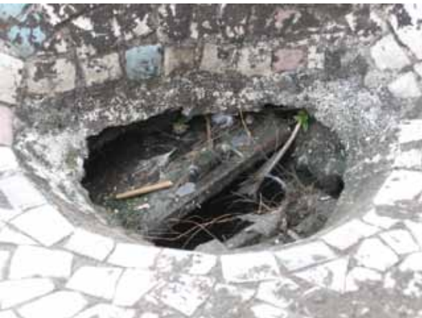
Clogged drain-mouths on the terrace surface that had prevented complete drainage of surface runoff rainwater
