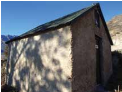
Figure 15. The Dairy building showing the entrance doorway. The schist is hidden by a cement render (photo: Matthew Schmidt, HNZPT, 2016).
