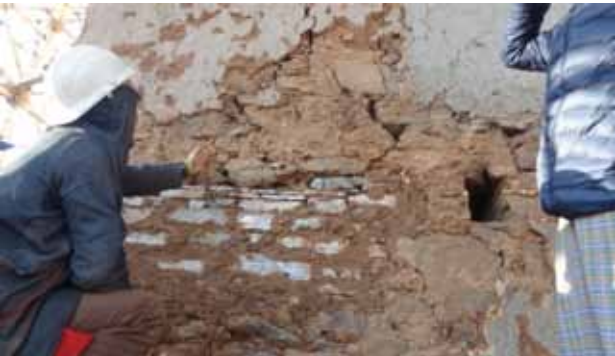
Fig.5 New wall constructed to stitch cracks on old wall
