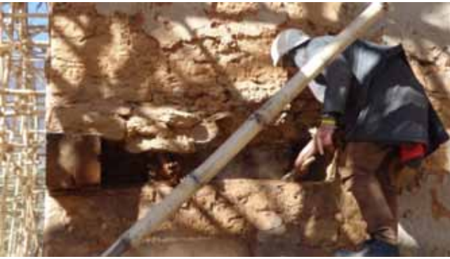
Fig.3 Surface being prepared for wall stitching
