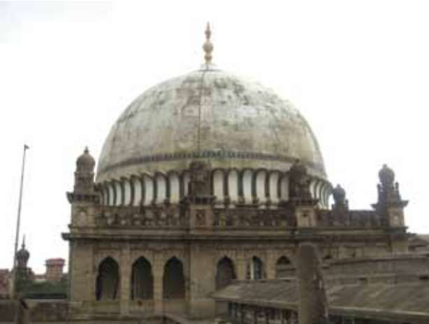
The discoloured main central dome with dust and grime deposits
