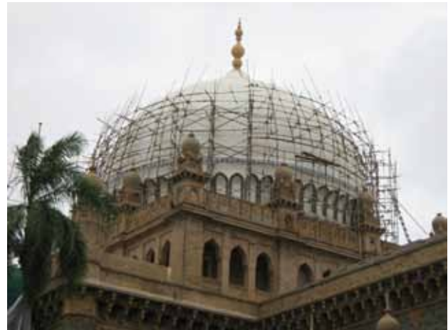
The original shine on the white dome after the non-abrasive and non-chemical cleaning process
