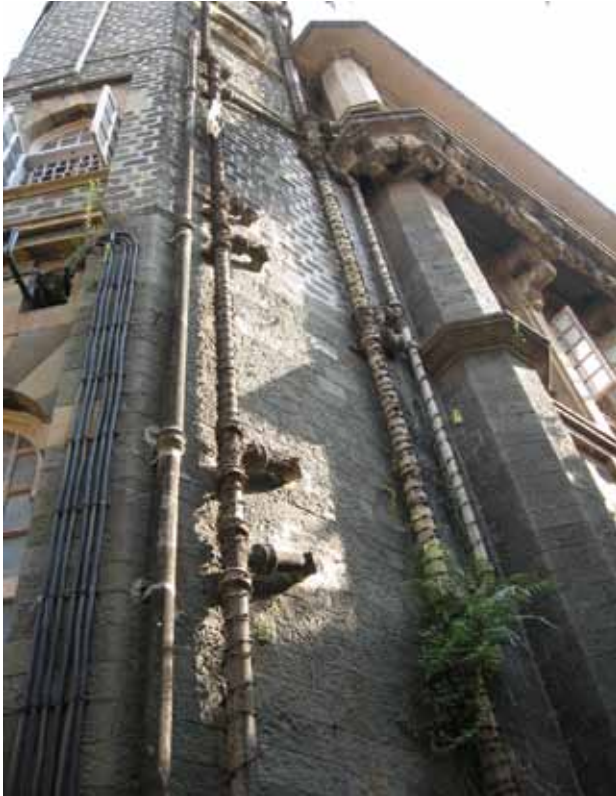
Leaking water pipes give rise to ficus growth and seepage of water into the masonry surface
