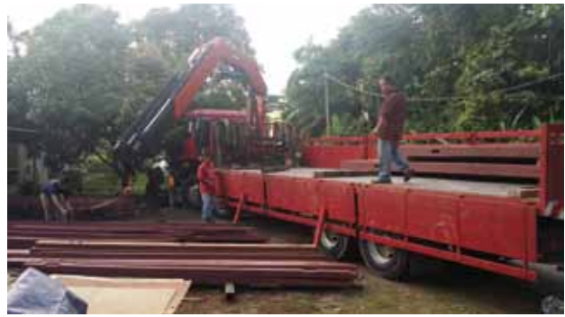
Treated timber structures and elements were loaded onto a truck at the sawmill before being transported to the new site.
