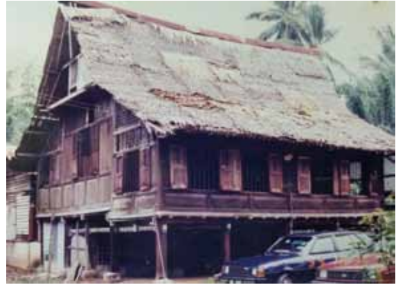
The front view of the Bugis house in 1999 revealing building defects such as a missing gable end, broken carved lattice panels and decayed thatched attap roof made of palm leaves.
