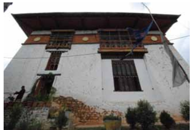
Fig.1 Front facade (East) of the Lhakhang before renovation
