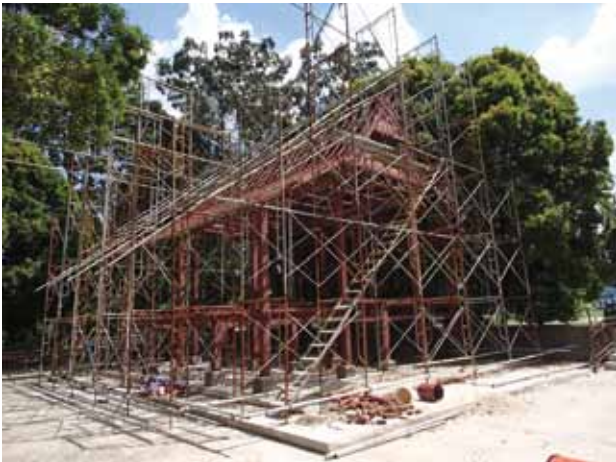
During reconstruction of the Bugis house, scaffolding was erected to support the building structures and elements, installation of new roofing materials and repainting.
