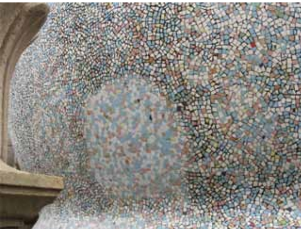
The China mosaic dome during the cleaning process
