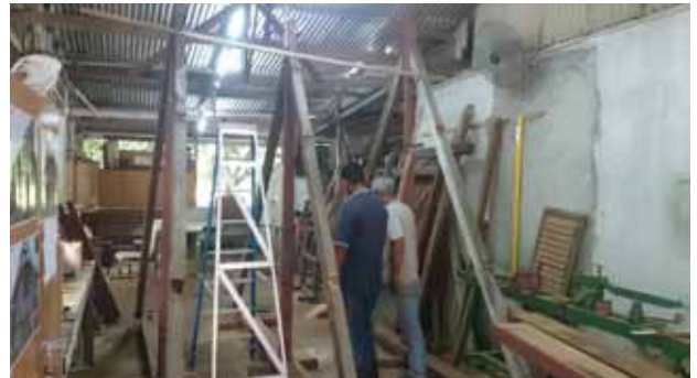
Timber structures and elements were repaired, replaced and replicated at a sawmill in Kampung Padang Jawa, Kelang, Selangor.
