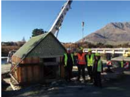
Figure 26. Some of the moving team, from left: Lou Robinson of Hadley & Robinson, Scott Sutherland of Civil Construction Ltd, Matthew Schmidt of Heritage New Zealand Pouhere Taonga and Jackie Gillies of Origin Consultants Ltd (photo: Matthew Schmidt, HNZPT, 2016).
