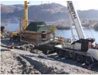
Figure 23. The Meat Shed successfully lifted and the beginning of the slow move over to the moving truck (photo: Jackie Gillies, Origin Consultants Ltd, 2016).
