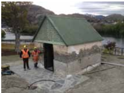
Figure 29. Landscaping works underway around the Meat Shed as well as initial repairs to the building. Pictured from left are Scott Sutherland of Civil Construction Ltd and Dean Kirk who undertook the repairs (photo: Matthew Schmidt, HNZPT, 2016).
