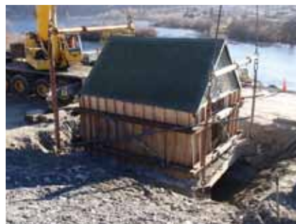
Figure 21. The Meat Shed all braced with crane straps connected to the lifting corbels (photo: Matthew Schmidt, HNZPT, 2016).
