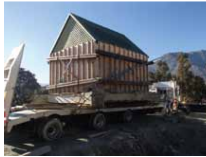
Figure 24. The Meat Shed on the house moving truck on its way to the new location 50m from its original location (photo: Matthew Schmidt, HNZPT, 2016).
