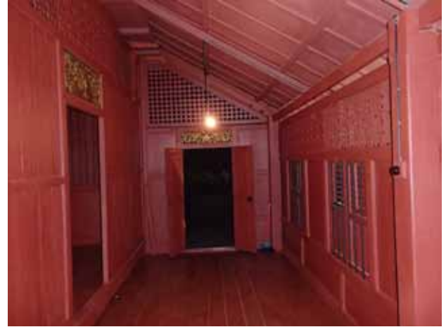
Interior view of the verandah after reconstruction.
