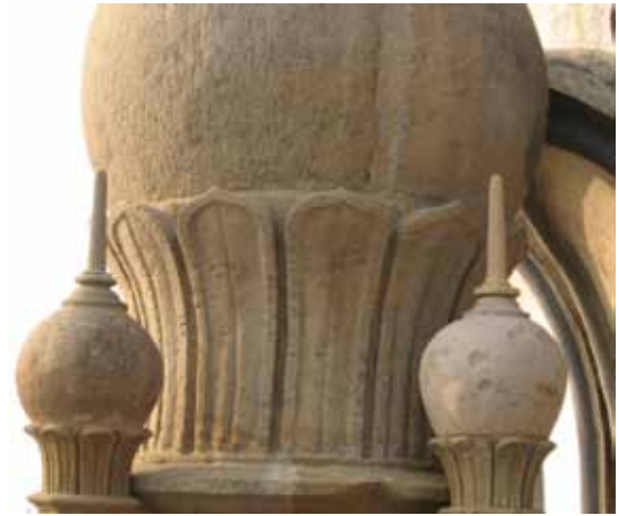
A newly carved guldasta dome and finial fixed beside an original and existing one
