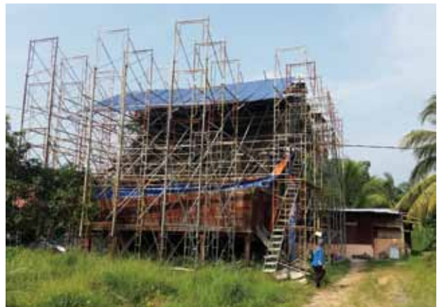
During the dismantling stage, scaffolding was erected around the Bugis house to support the building structures, while temporary roofing was constructed above the house to protect the interior from heavy rainfall.
