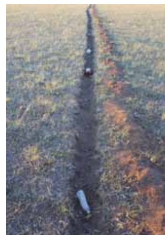
Fig. 23: Trench for base. From the south
