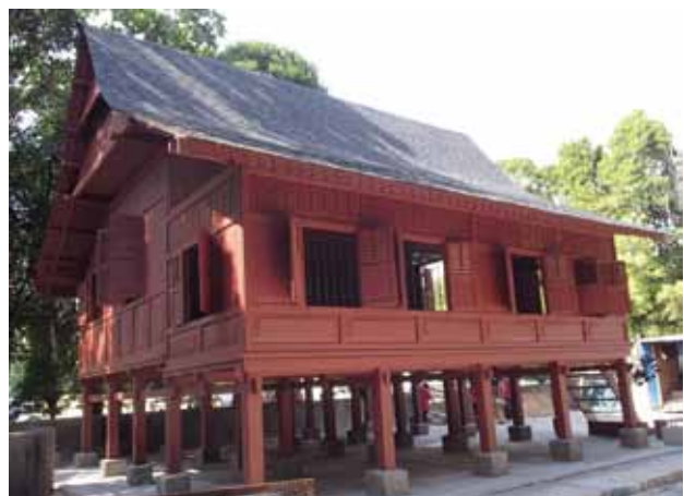
Front view of the Bugis house after reconstruction.
