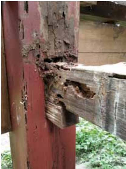
Decayed timber stilt and floor beam due to natural decay and termite infestation.
