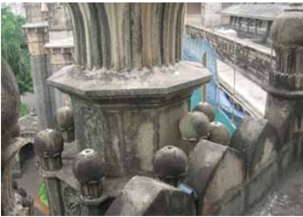
The domes and finials of the guldastas were in a damaged condition. The fallen domes were collected and refixed again
