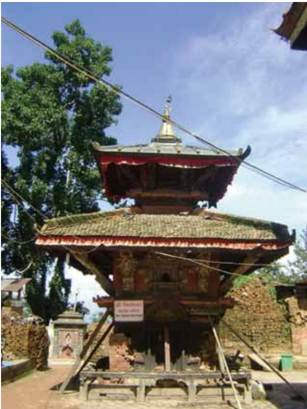
1. Kileshwor Temple, Changu Narayan Damaged by the Earthquake
