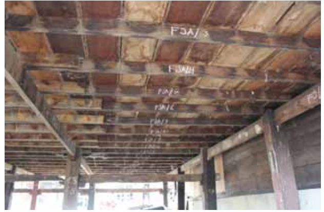
All timber structures including stilts, floor beams and floor joists were marked and coded for reference.
