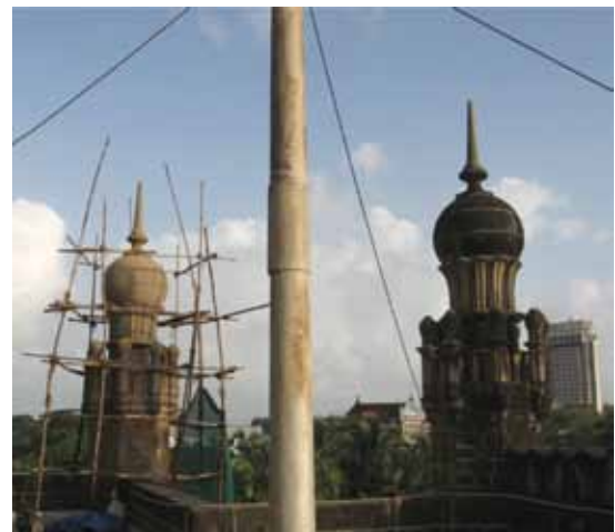
Discoloured urns and finials and other decorative elements with dirt grime and salt deposits on the right and a cleaned and repaired surface on the left
