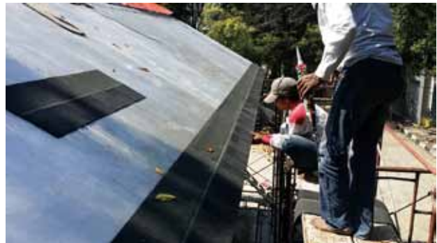
Installation of asphalt shingles on the roof.
