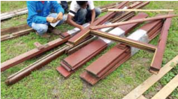
All dismantled timber structures and elements were transported to a sawmill for the process of timber selection and classification.
