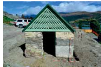
Figure 19. The Meat Shed prior to preparation for moving (photo: Ben Teele, Origin Consultants Ltd, 2016).
