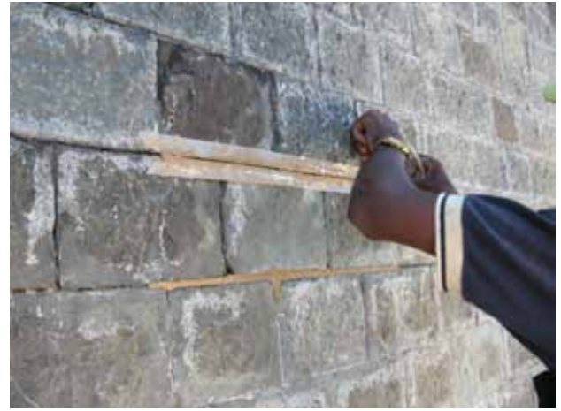
Re-pointing in lime mortar after covering the sides with masking tape
