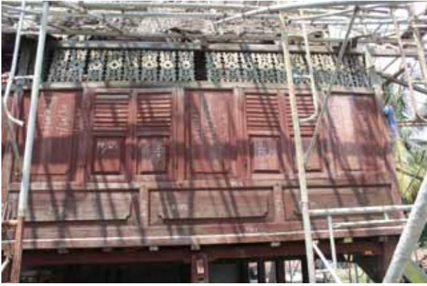
Special codes were marked on timber elements before dismantling and salvaging.
