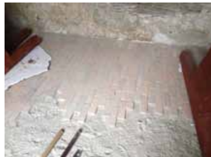
Figure 30. The brick floor of the Meat Shed being reinstated (photo: Matthew Schmidt, HNZPT, 2016).
