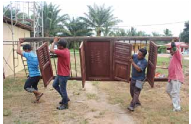
Dismantled louvered casement windows were taken down to the ground for investigation and salvaging.
