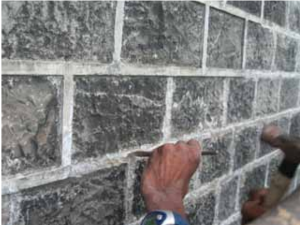
Removal of ribbon cement pointing
