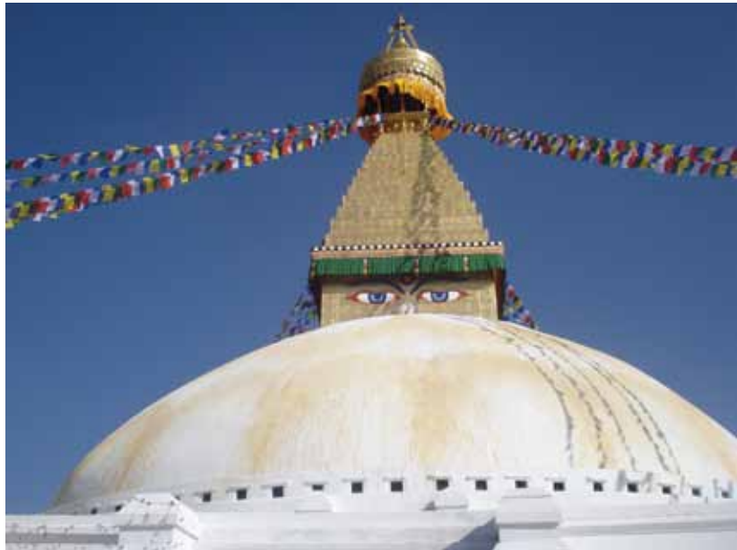
6. Completion of Conservation Work of Bouddha Sutpa After Earthquake 2015
