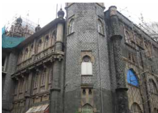
The ribbon cement pointing seen on the upper half of the corner tower has been added, while the original lime mortar pointing can be seen on the lower half
