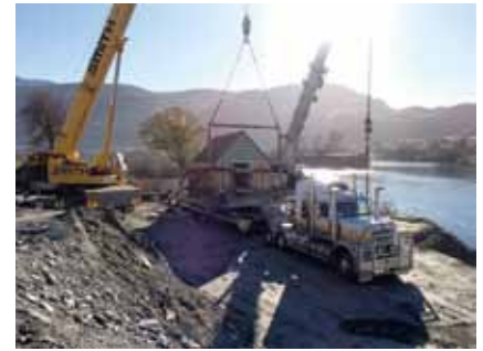
Figure 25. The Meat Shed being backed into place next to its new location (photo: Matthew Schmidt, HNZPT, 2016).
