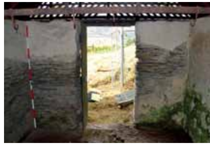
Figure 13. The interior of the Meat Shed showing the schist walls (parts rendered), timber roof, meat hanging bars and hooks and the doorway (photo: Ben Teele, Origin Consultants Ltd, 2015).
