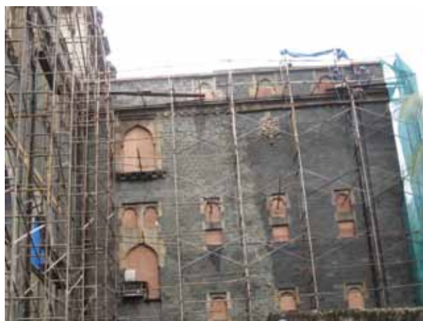
Masonry walls with ribbon cement pointing removed, re-pointing done in lime mortar, and washing using the misting technique after blocking all openings temporarily using plywood boards
