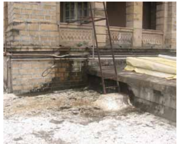
Leaking rainwater pipes and poorly managed storm water drainage on the terrace
