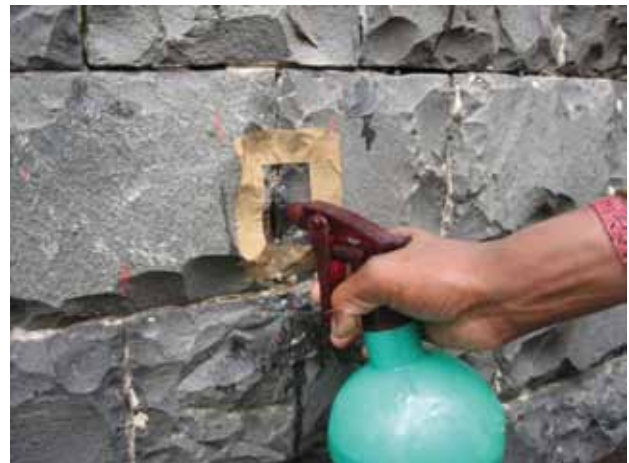
Removal of ficus growth and application of chemicals in the crevices to kill roots and prevent further growth
