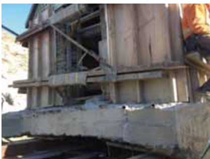
Figure 20. Close view of the concrete beam strip foundation and other bracing prior to the move (photo: Matthew Schmidt, HNZPT, 2016).
