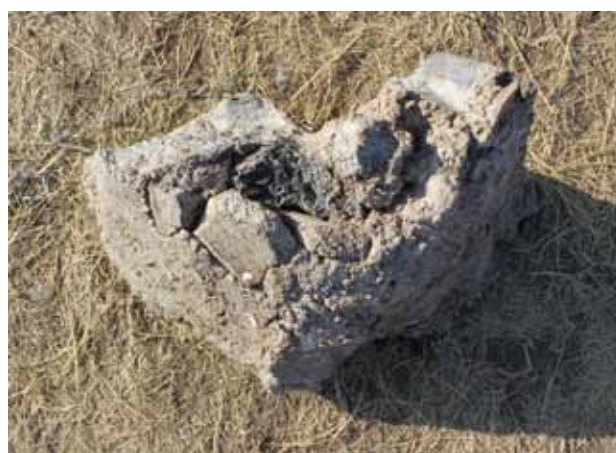
Fig. 4: Post-hole cement with roof-tile pieces
