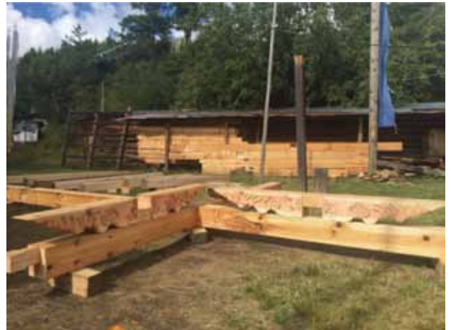
Fig.12 The timber components being allowed to dry after application of the persimmon liquid
