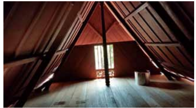
Storage attic featuring double-layered gable end, small opening and pitched roof ceiling after reconstruction.
