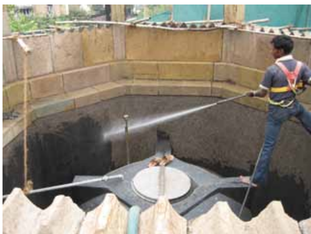
Cleaning discoloured surfaces using the water misting technique with a calibrated pressure pump and nozzle
