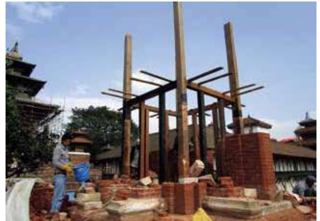
The corner timber posts are tied together at regular intervals with timber tie beams for seismic strengthening. The upright posts on either sides for the sanctum entry are also provided. Such timbers are embedded inside brick masonry and are under constant threat of moisture penetration; to avoid such conditions necessary barriers are provided. (Photo: 2017-06-11)
