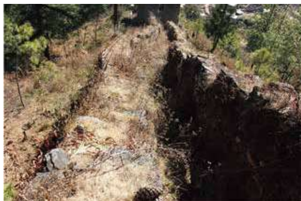
Fig. 6 Fortified pathways and watch towers (above and below). Source: DCHS
