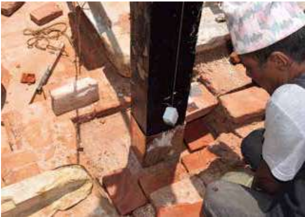
The bottoms of the timber upright posts to be embedded within the masonry were coated with bituminous paint and wrapped with copper sheets for protection against moisture. (Photo: 2017-05-25)
