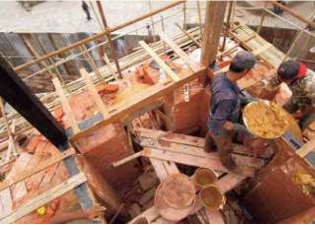
Constructing the arches above the entry to the main sanctum. (Photo: 2017-06-15)
