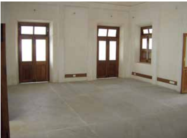
The installed doors and windows
