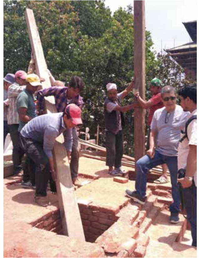
Upright timber posts were erected at four corners of Shikhara. The portion of timber embedded within the brick masonry was coated with bituminous. (Photo: 2017-05-25)
