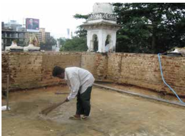
Cleaning of the terrace in progress
