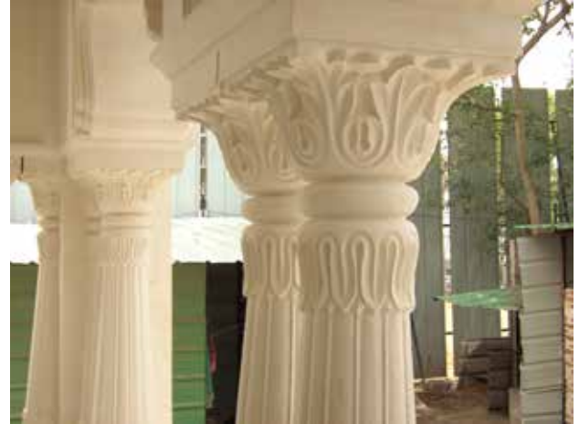
The column capitals before and after strengthening and finishing
