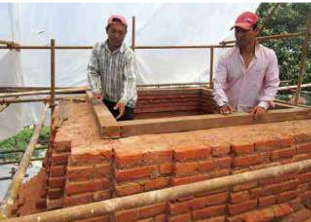
Timber wall plates provided at important levels of the Shikhara. (Photo: 2017-07-17)
