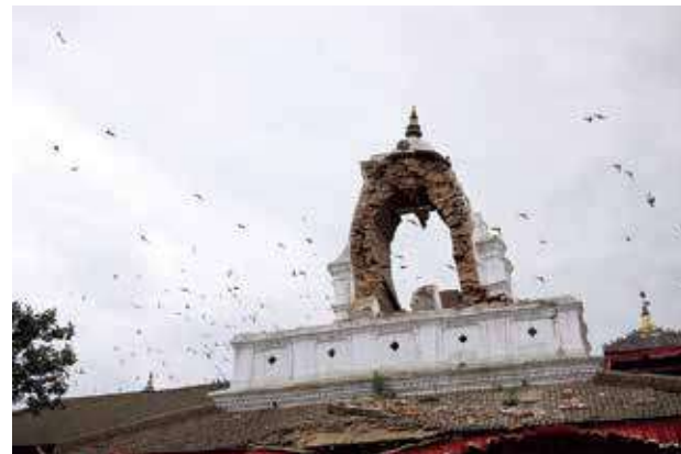
Kageswor Mahadev Temple during the April 25th earthquake. (Photo:2015-04-25)
