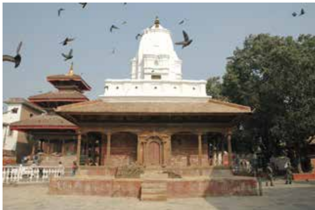
Kageswor Mahadev Temple before the April 25th earthquake. (Photo:2005-11-25)
