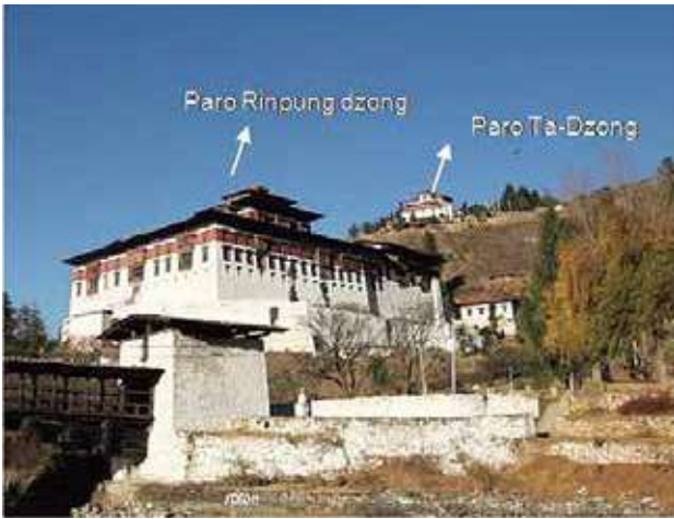
Fig. 7 Paro Rinpung dzong (left) and Paro Ta-dzong (right) showing the location of the main dzong and watch tower. Source: DCHS
