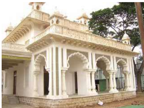
The verandah after restoration
