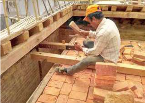
Carpenters preparing the new timber sections on site, which shall replace the affected and non-reusable timber sections. (Photo: 2017-03-31)
