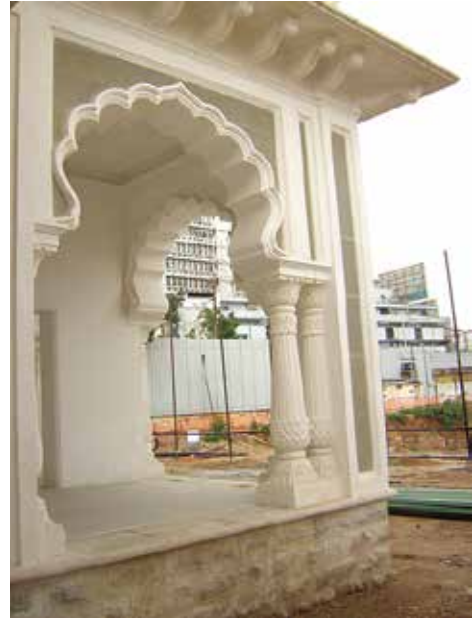
The revamped brackets of the chajja over the verandah before and after restoration
