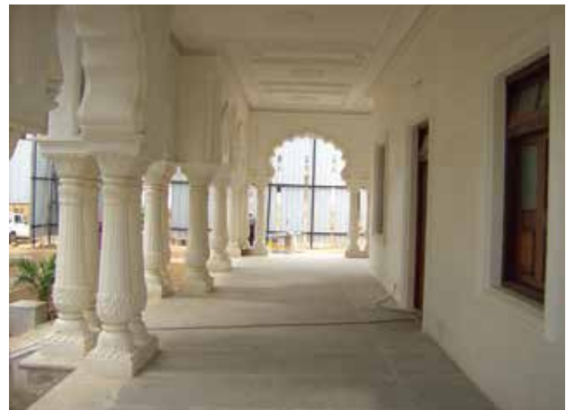
The finished verandah
