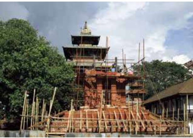
Shikhara structure turrets construction continued with rafters on the skirt roof below. (Photo: 2017-06-26)
