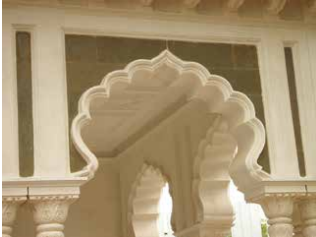
The cusped arch façade with Shahbad stone before and after restoration
