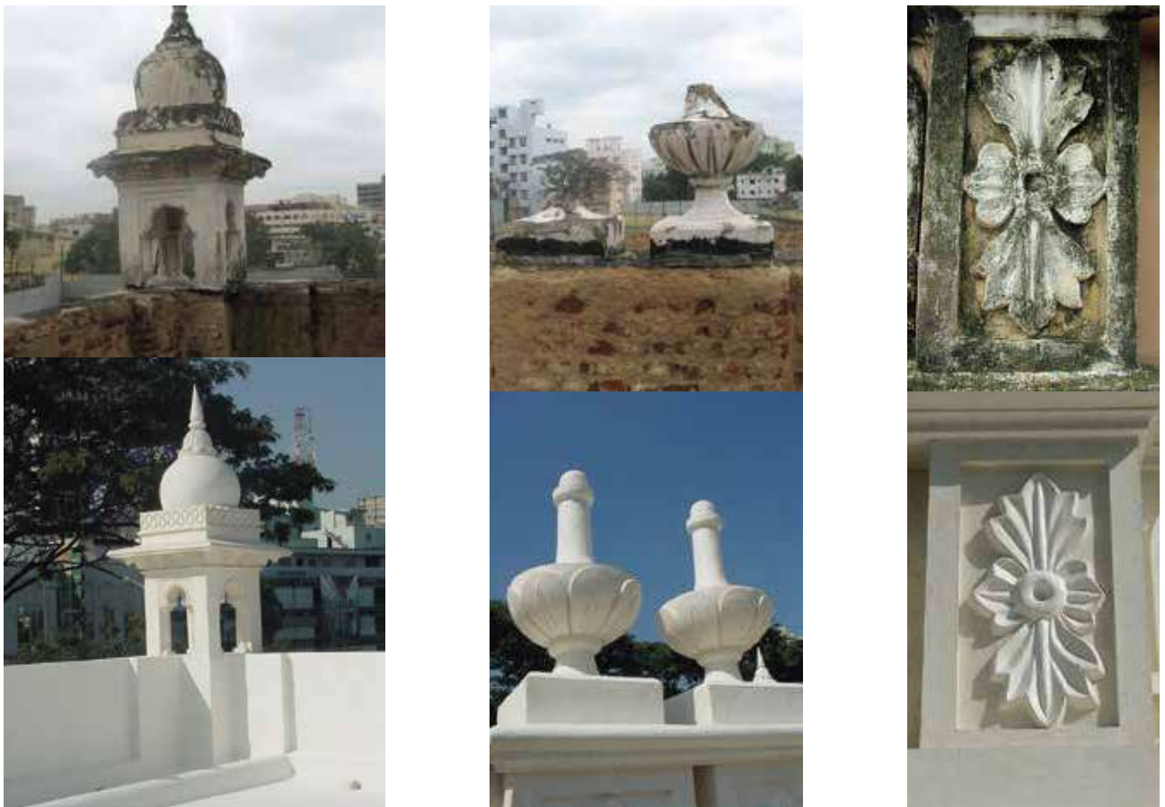
Kiosks, bowl-shaped finials and parapet wall detailing before and after restoration
