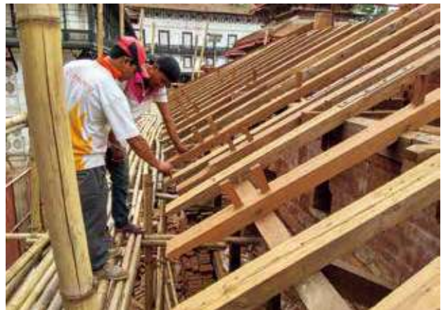
New timbers were used for rafters of the skirt roof. Each rafter is properly aligned and fixed in place using wooden pegs. (Photo: 2017-06-30)
