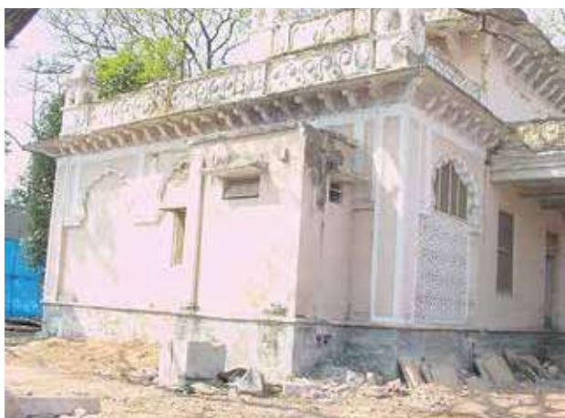
Enclosed verandah before restoration
