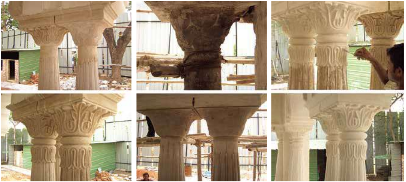
The column ornamentation before and after the lime finishing works
