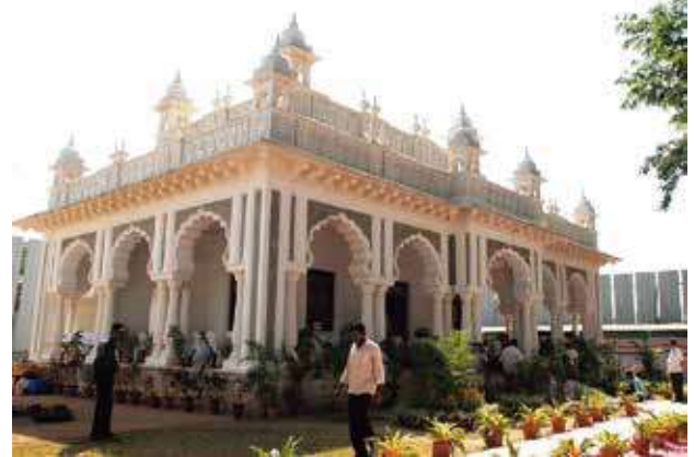
The conserved structure and completed landscaping with walkways
