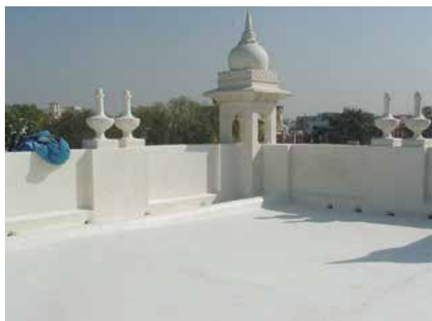
Waterproofed and finished terrace
