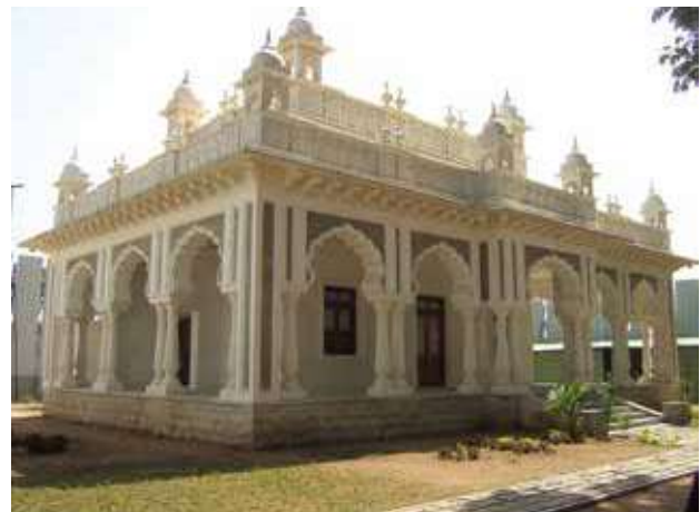
The CIB building restored
