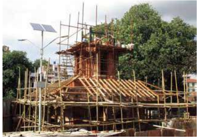
South-west view. The skirt roof rafters are being laid while the shikhara structure continues to rise. (Photo: 2017-06-26)
