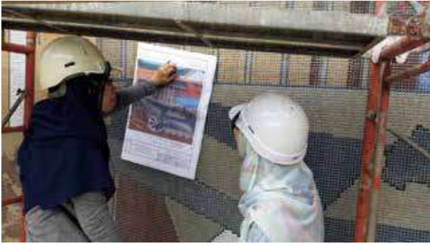
It was important to check the reinstalled mosaics which were positioned according to the grid system.
