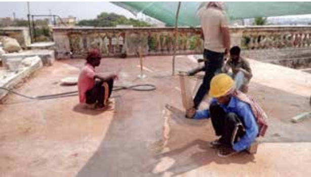
Ramming the terrace with wooden kurchi
