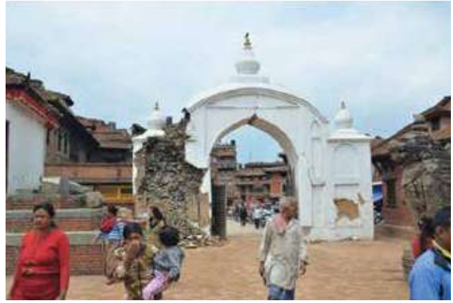
2.1.2 City Entrance Gate, BKT after earthquake
