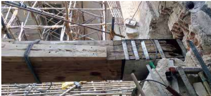
Consolidation and SS capping at both ends of the beam FFB1 in situ
