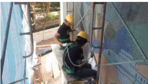
The reinstallation of mosaics began from the bottom left, moving upwards and sideways.
