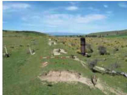
Figure 18. One of the huge earth walled gold mining water reservoirs. The pipework to control the flow of water out of the reservoir and into a 'header' race to the mining area is intact (Photo: Briden & Schmidt 2007).
