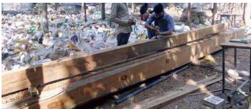
Planing and processing the teak wood for the new FFB2 beam
