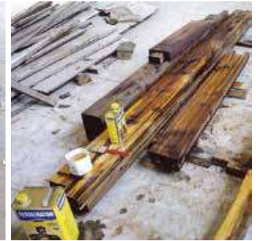
Application of anti termite coating on the new FFB2 and old FFB2
