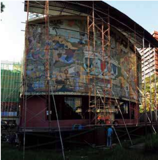
Before reinstallation of the mural, scaffolding was erected on the platform and temporary roofing was fixed on the roof for the entire period of the mural reinstallation works.
