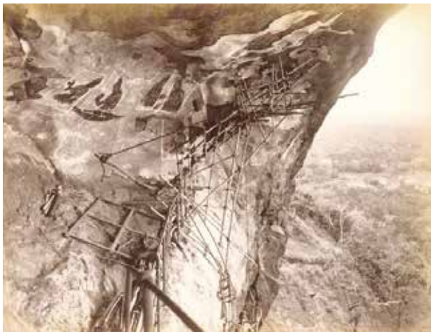
Documentation of Sigiriya and erecting iron platforms
