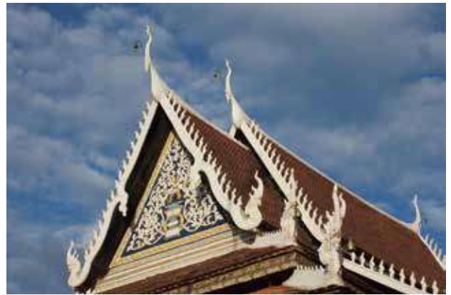
Fig 25. Southwest view of adorned roof elements after restoration
