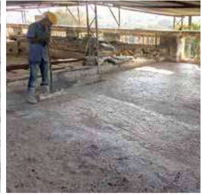
After the second layer of kappi was laid, it was levelled with a wooden or aluminium member and further flattened by ramming
