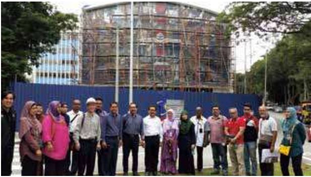
Regular site inspections were jointly conducted by the Public Works Department (JKR HQ and JKR WPKL), Department of National Heritage, Dewan Bahasa dan Pustaka, consultant architect, consultant building conservator and contractor team members to ensure that the project was completed on schedule.
