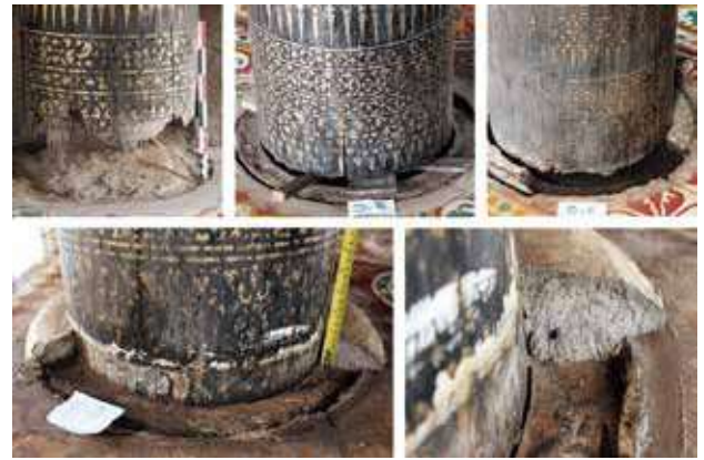
Fig 8. Condition of the bottom of columns
