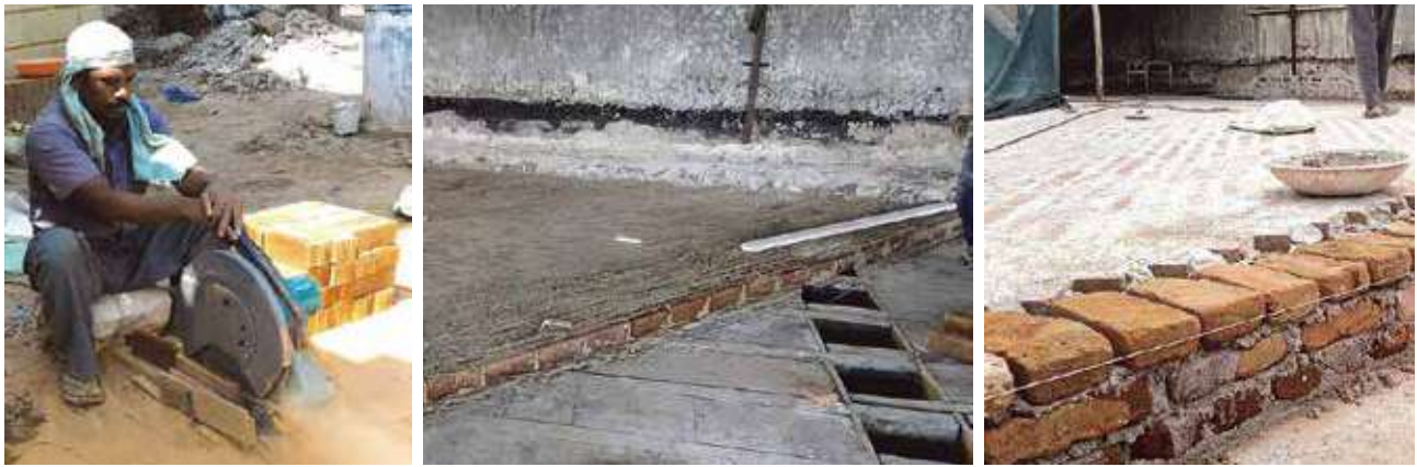
Standard size bricks were finely machine cut into the required size and laid at a 45 degree angle to the joist. Finally, the gap between the teak wood joists on the ceiling was plastered and painted.
