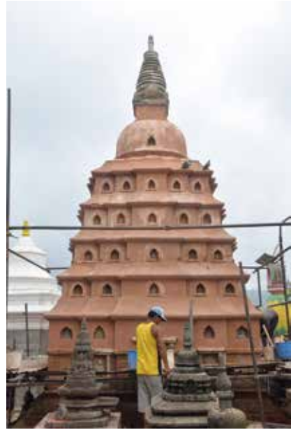
5.2.3 Tashi Gomang Stupa, Swayambhu after reconstruction
