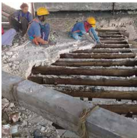
Carefully dismantling the deteriorated lime concrete and later additions on the roof
