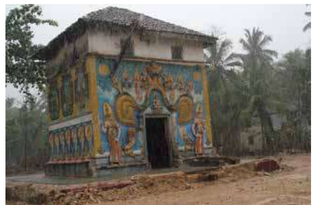
Disaster caused by the tsunami
