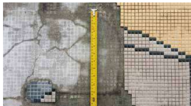
A dilapidation survey was conducted to determine the condition of the DBP mosaic wall, as well as common mural defects and their causes.
