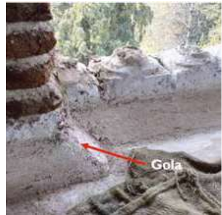
The edges of the terrace roof sealed with gola in lime concrete
