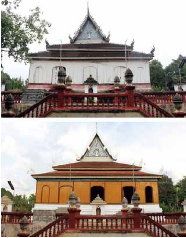
Fig 22. West view: before and after restoration
