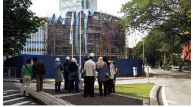
Removal of the plastic sheets and dismantling of scaffolding after reinstallation of the mural mosaics.
