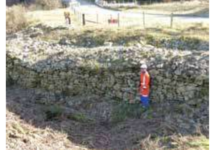
Figure 43. The beautiful dry schist stone walling of the roadside tailrace at Site 1 after vegetation clearance. This is the same tailrace obscured by vegetation in Figure 35. The stone has originated from the piles of gold tailings which used to fill the space next to it. Skilful experienced miners would have built this wall (Photo: Dougall Campbell, Transpower).
