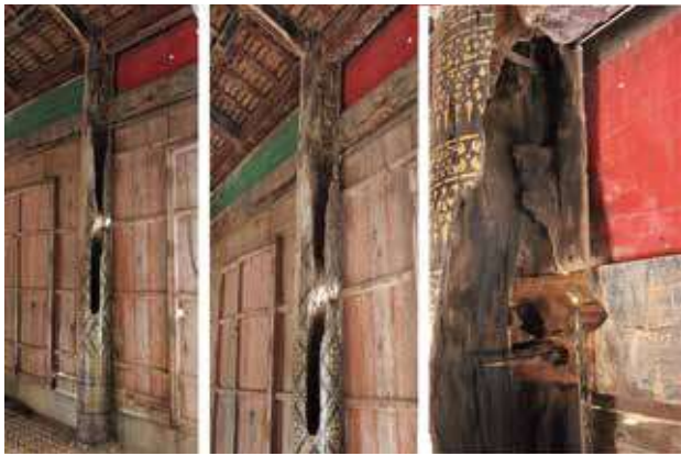
Fig 7. Column condition and detail
