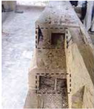
New sections of wood with tenons were fixed into mortise grooves made in the existing FFB2 beam
