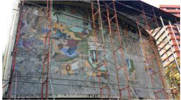
An important stage in the conservation works involved the removal of all mosaics before treating the wall substrate.
