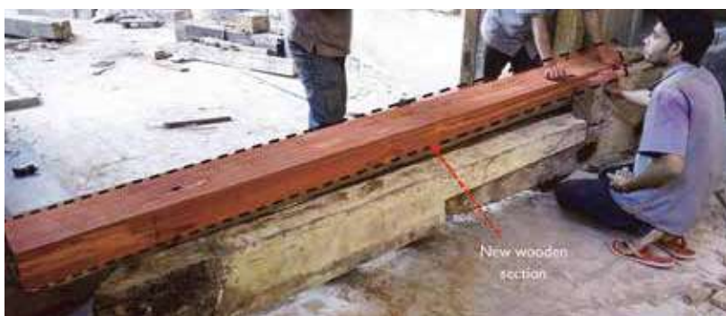
Wooden members of various sizes used to fix the beam FFB2 to replace UGB2
