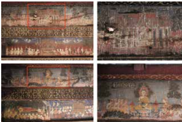
Fig 9. Condition of the upper wall mural paintings
