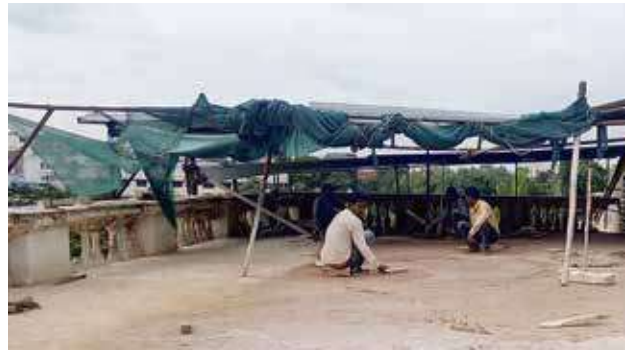
The completed lime concrete roof over the Madras terrace roof, above the oval room
