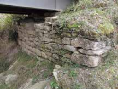
Figure 23. 19 th century schist bridge abutments. These are from the bridge that can be seen in Hart's ca. 1877 photograph of the Kyeburn Diggings in Figure 4 (Photo: Matthew Schmidt).
