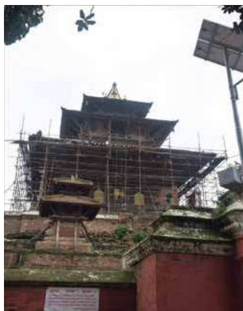
1.4.3 Taleju Temple – ongoing conservation
