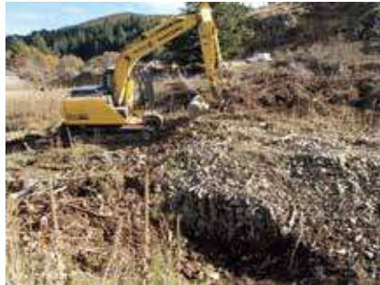
Figure 39. Vegetation being removed from the stone-lined tail race at Site 1 during restoration works by Heritage New Zealand & Transpower. Note the stone revetting (Photo: Matthew Schmidt).
