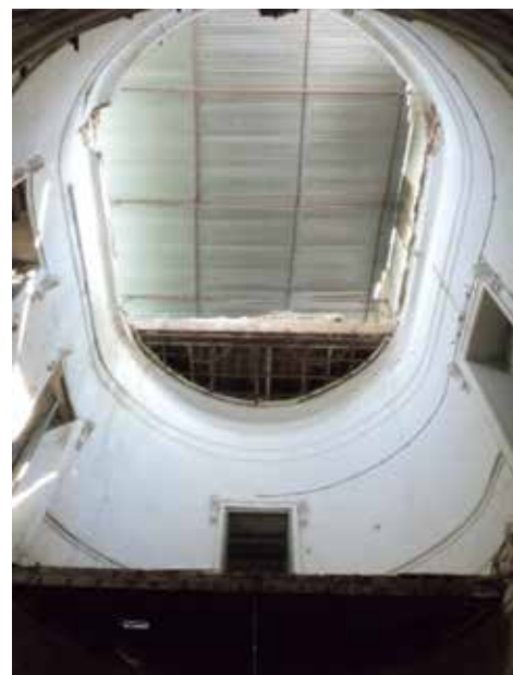
A worm's eye view of the oval room with the exposed temporary sheet roof, after careful dismantling of the Madras terrace roof components and primary beam FFB2. The FFB1 beam remained intact.
