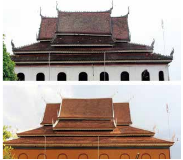
Fig 23. South view of the roof: before and after restoration
