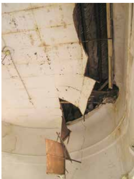
Thin rusted ornamental sections of iron sheets that had detached themselves from the wooden rafters of the oval room ceiling, above which rests the madras terrace roof
