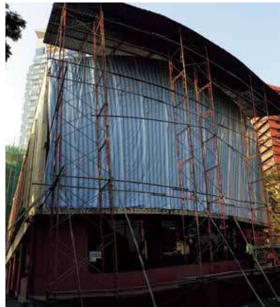
The mural surface was covered with plastic sheets to protect it from direct sunlight and heavy rain.
