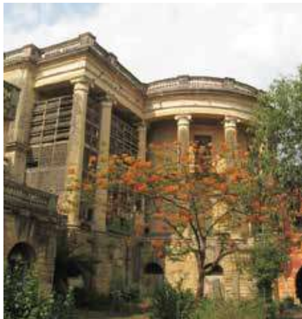
Palladian rear view of the British Residency
