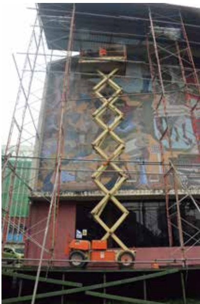
A scissor lift was stationed on the platform for the high resolution photography process.
