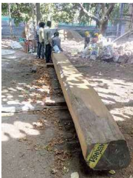
The teak wood procured for the new FFB2 beam
