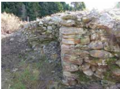
Figure 44. A close view of the dry schist stone wall stonework seen in Figure 43 (Photo: Dougall Campbell, Transpower).
