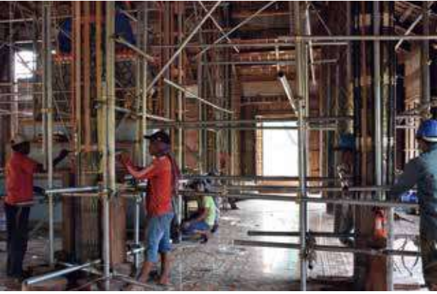
Fig 14. The setting for lifting up the columns
