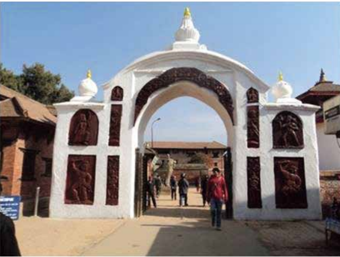
2.1.3 City Entrance Gate, BKT after reconstruction
