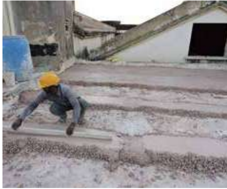
After the second layer of kappi was laid, it was levelled with a wooden or aluminium member and further flattened by ramming
