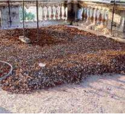
Brick bat cobba and burnt lime ( kappi ) before mixing, laid to achieve the required slope
