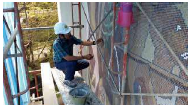
The mosaics were reinstalled based on the grid system established from the captured mural image.
