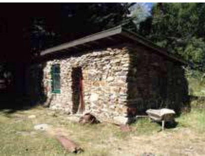
Figure 26. The 'Schist House' at Site 2 as indicated on Survey Map SO 785 from 1918 in Figure 8 (Photo: Matthew Schmidt).
