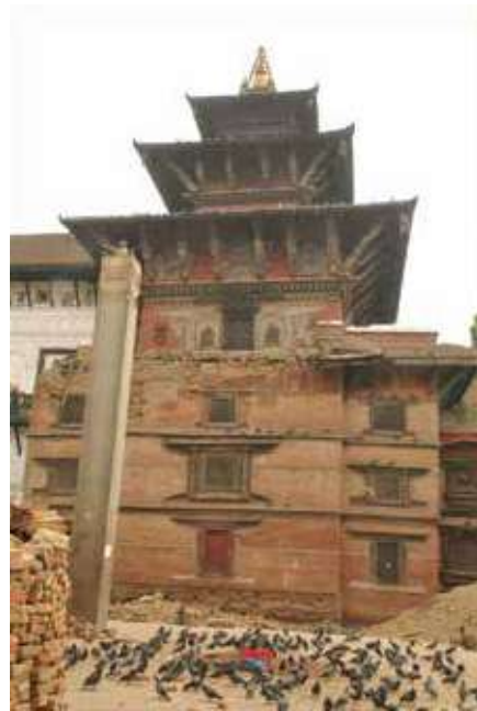
1.2.2 Degu Taleju after earthquake
