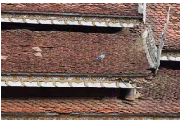
Fig 5. Broken adorned roof elements
