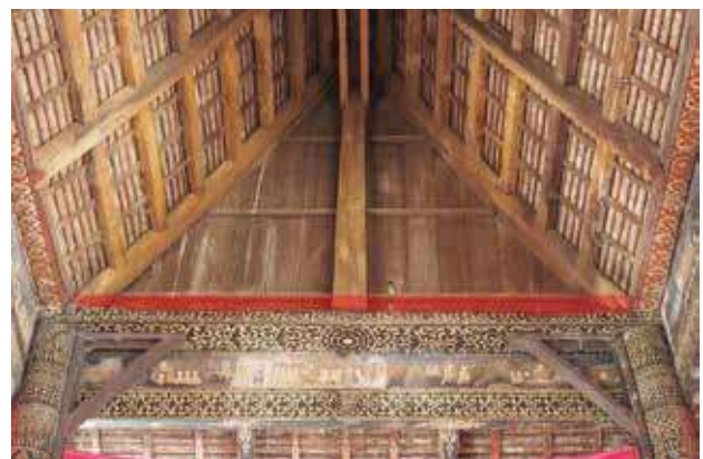
Fig 6. The broken main beam
