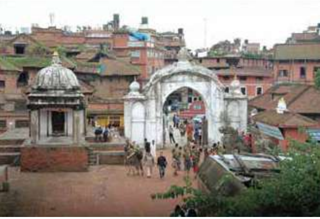
2.1.1 City Entrance Gate, BKT before earthquake
