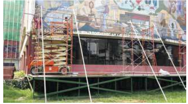
During site preparation, a suitable location was identified on site to build a sturdy working platform to place the scissor lift and scaffolding.
