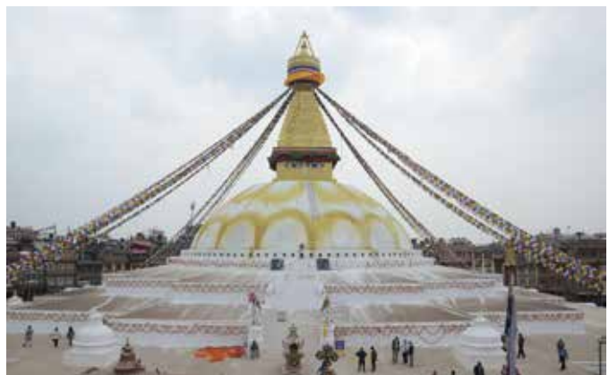
4.1.3 Bouddha Stupa, Bouddha after renovation
