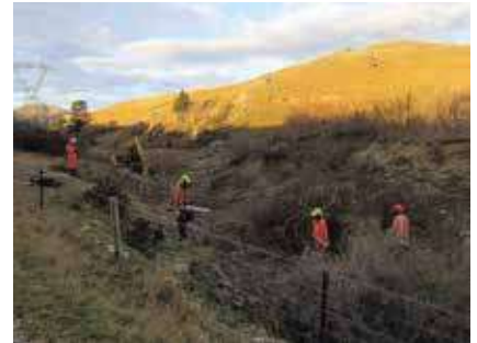
Figure 40. Vegetation clearance work being undertaken by Electric contractors at Site 1 (Photo: Matthew Schmidt).
