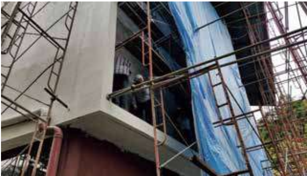
All cracks on the wall substrate were repaired before resurfacing the wall substrate with the same material as the existing one.
