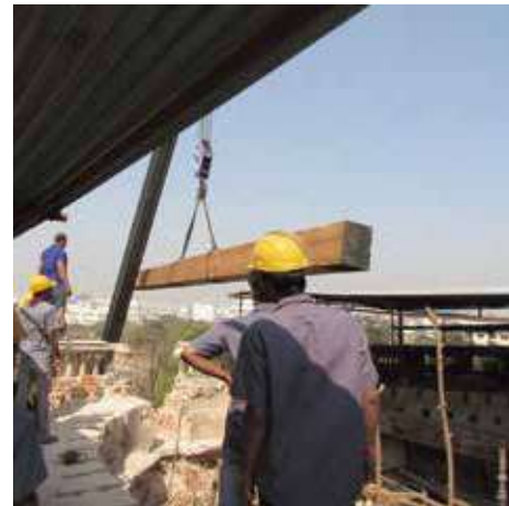
Lifting the new FFB2 beam over the terrace and placing it in position
