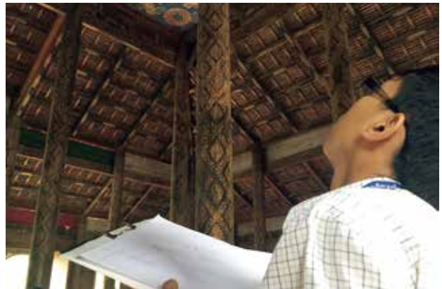
Fig 19. Checking the construction structure
