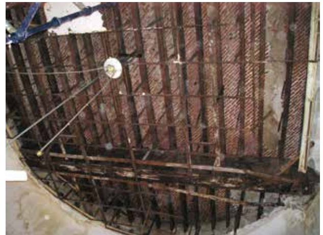
The exposed Madras terrace roof after removal of the false ceiling tin sheets with the deteriorated primary beam
