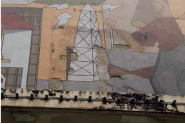
The dilapidation survey revealed that some of the mosaics were loose, detached, broken, missing or had fallen off.
