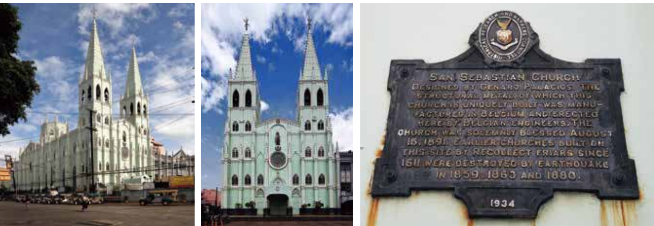
A 1934 marker can be seen in the facade of the San Sebastian Basilica. It reads: "San Sebastian Church was designed by Genaro Palacios. The structural metal of which this church is uniquely built was manufactured in Belgium and erected here by Belgian Engineers. The church was solemnly blessed on August 15, 1891. Earlier churches built on this site by the Recollect Friars since 1611 were destroyed by earthquake in 1859, 1863, and 1880."
