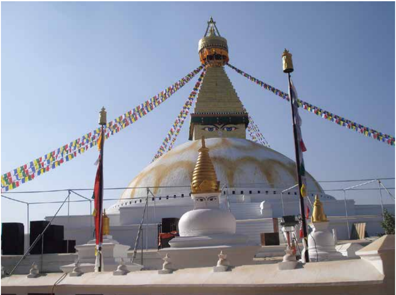
After completion of renovation of Stupa
