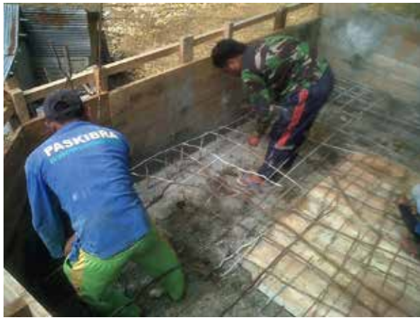
Concrete reinforcement assembly
