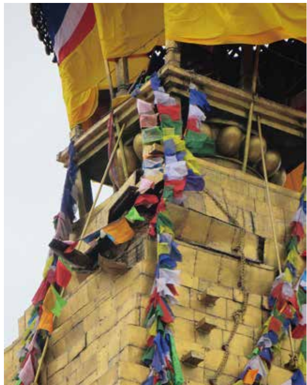
Damaged upper parts of sutpa-trayodasha bhuvana
