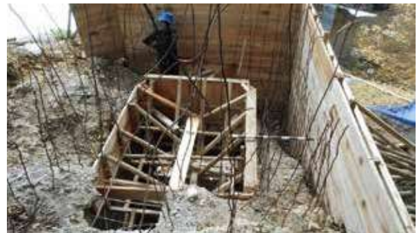
Wall framework installation
