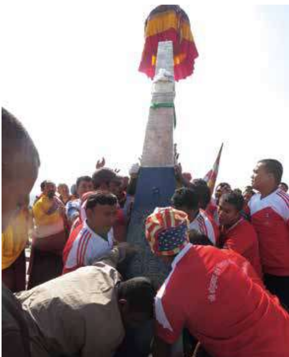
Reinstalling the soksing ( yesthi ), the central shaft beam which is the main vertebra of the stupa after performing religious activities
