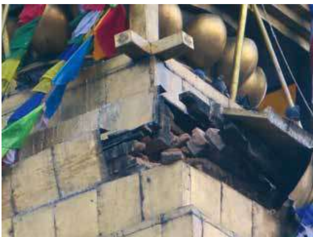
Damaged due to Earthquake 2015
