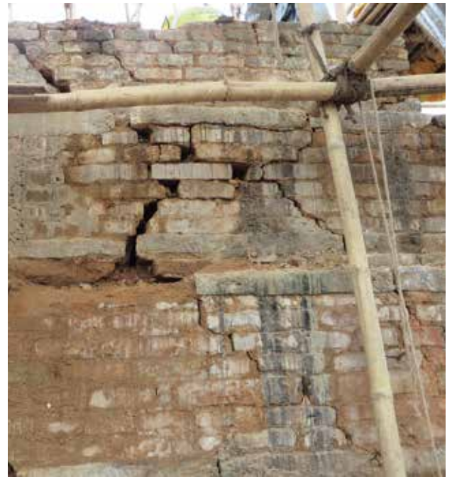
Damaged parts of harmika , explored after removing the copper sheets
