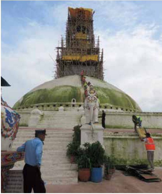
Bamboo scaffoldings prepared for renovation work in the beginning
