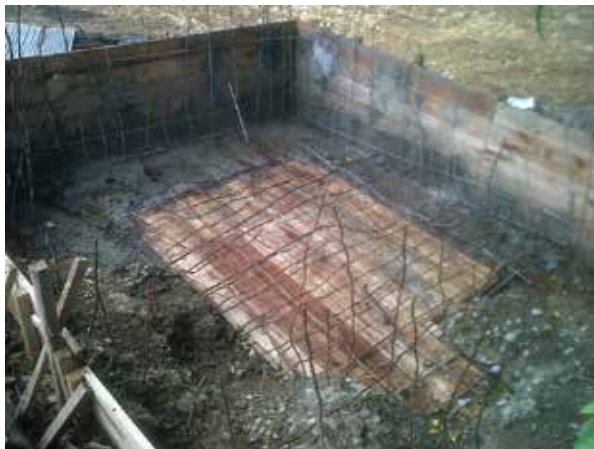
Details of wall framework and concrete reinforcement
