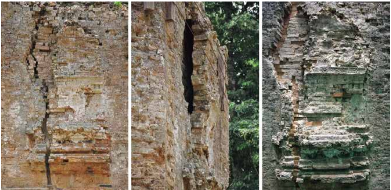
Example: The 'flying palace' wall carving of S8 tower and its state of conservation (left & middle: before; right: after)
