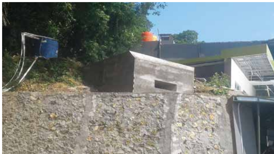
The result of the bunker reconstruction
