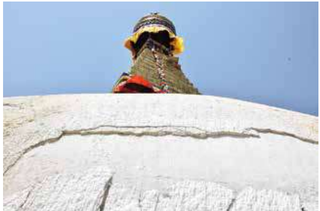
Damaged due to Earthquake 2015
