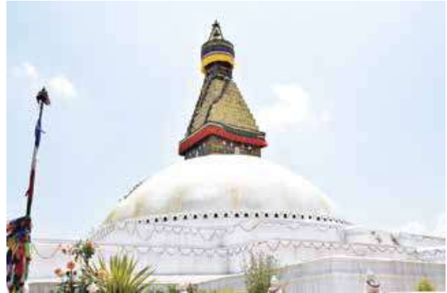
Damaged Bouddha Stupa due to Eartquake 2015
