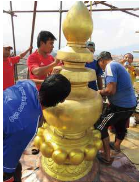
Topmost part, gazur-finial of Stupa, almost finalizing the renovation of upper part
