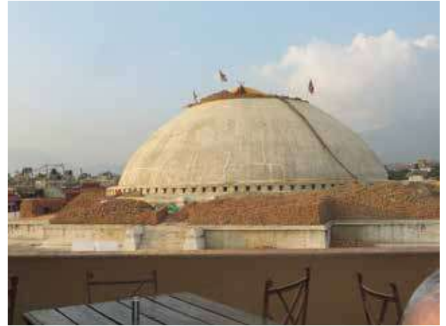
Stupa after opening the severely damaged upper parts to renovate
