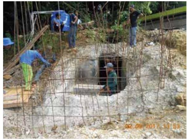
Concrete reinforcement assembly
