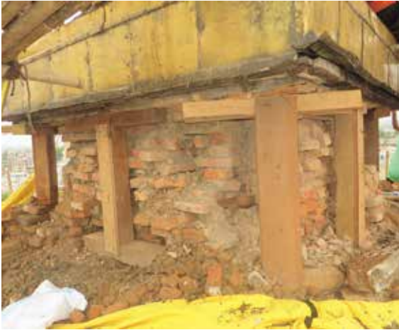
Damaged parts of harmika , explored after removing the copper sheets with new support
