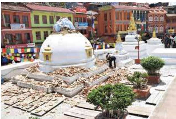
The damaged associated stupa within Boudha Main Stupa
