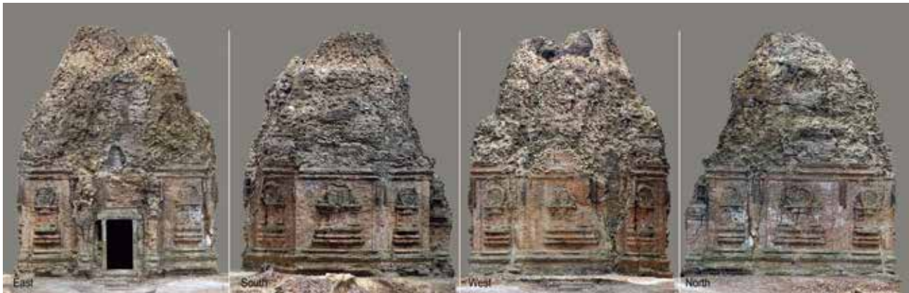
Photoscan images of elevations of the S11 tower before restoration
