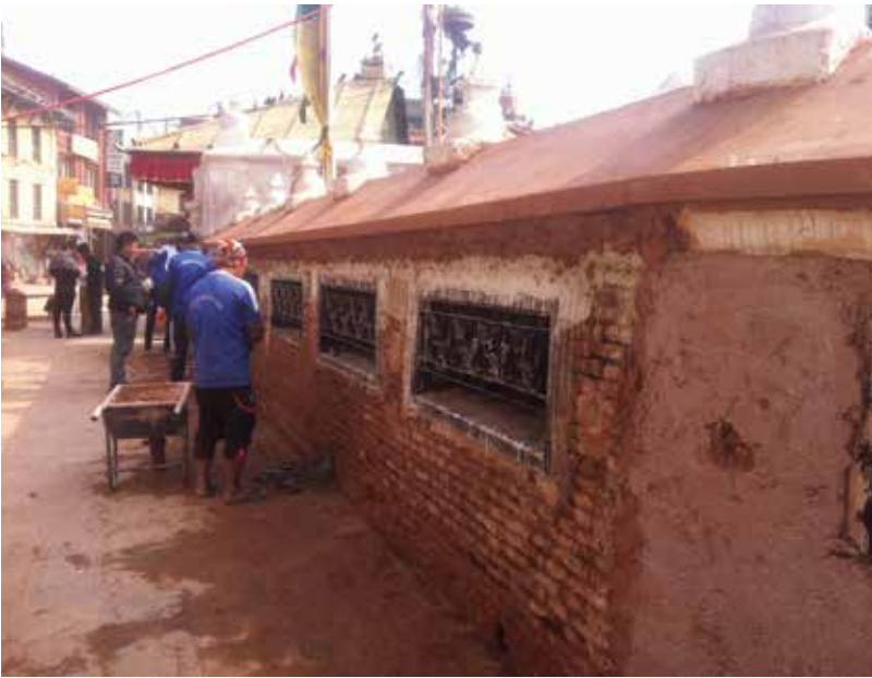
Finalizing the renovation of stupa-plastering with lime surkhi in the lower parts of Stupa
