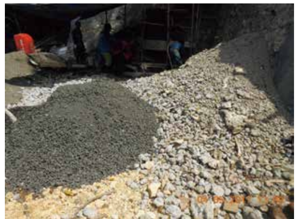
Sand and gravel for making the concrete
