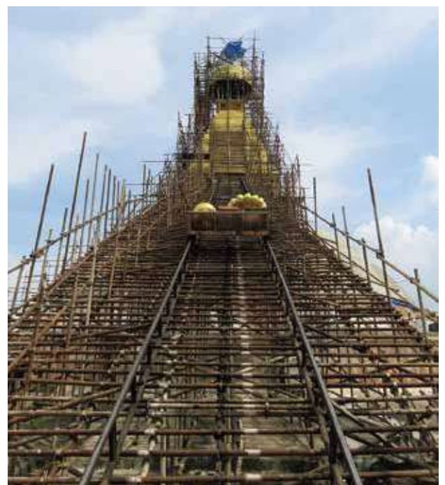
Metal scaffoldings to work easily on the upper part of the stupa
