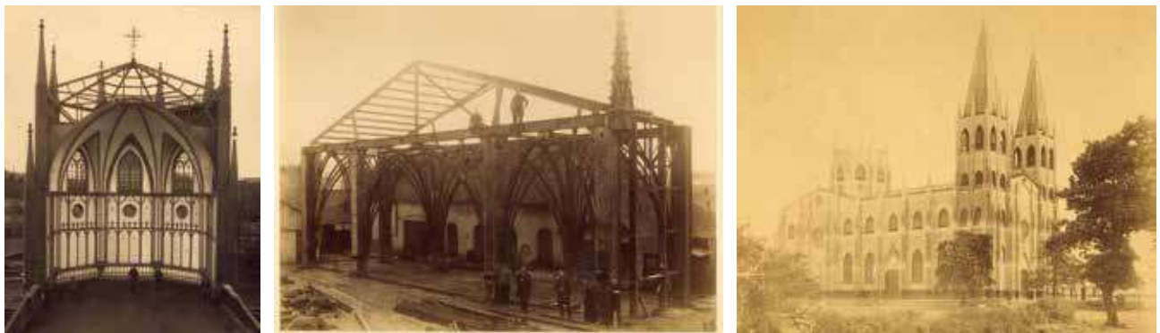
The first two photos above (from left) were taken in Belgium when they were doing trial mounts of the prefabricated pieces before disassembly and shipment to the Philippines. They had to make sure of the correct measurements before shipping the parts. The San Sebastian Basilica consists of 1,500 tons of metal. The first shipment arrived in 1888 and the first column was erected on September 11, 1890. The basilica has one dome, two towers, 132 columns and 64 spires.
