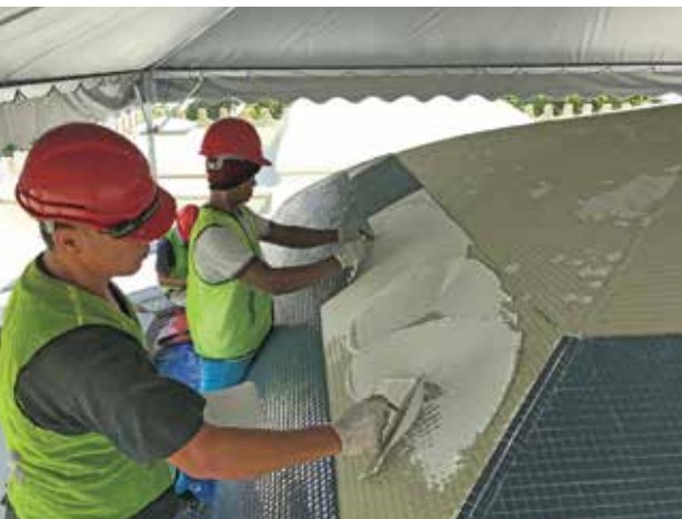
Spreading the tile adhesive on the surfaces of the dome by using a notched trowel before layering the sheet of glazed porcelain mosaics.
