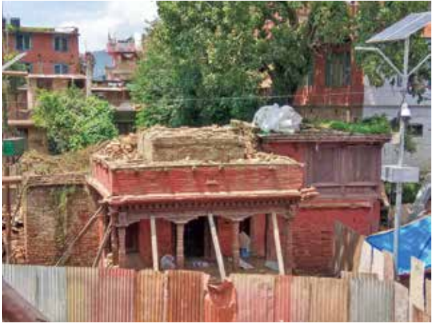
Fig 9. A view of the temple after removal of the roof rafters. The inner sanctum wall on the first-floor level can be seen (2017-08-27).
