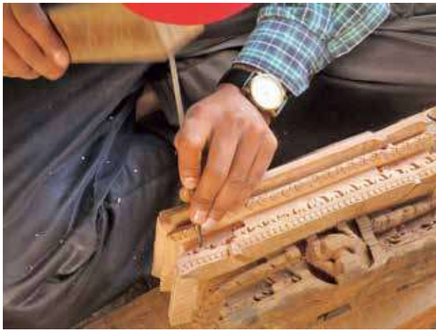
Fig 12. A new timber added to the lion base of the main door threshold being carved. The details are as per the originals (2017-10-26).
