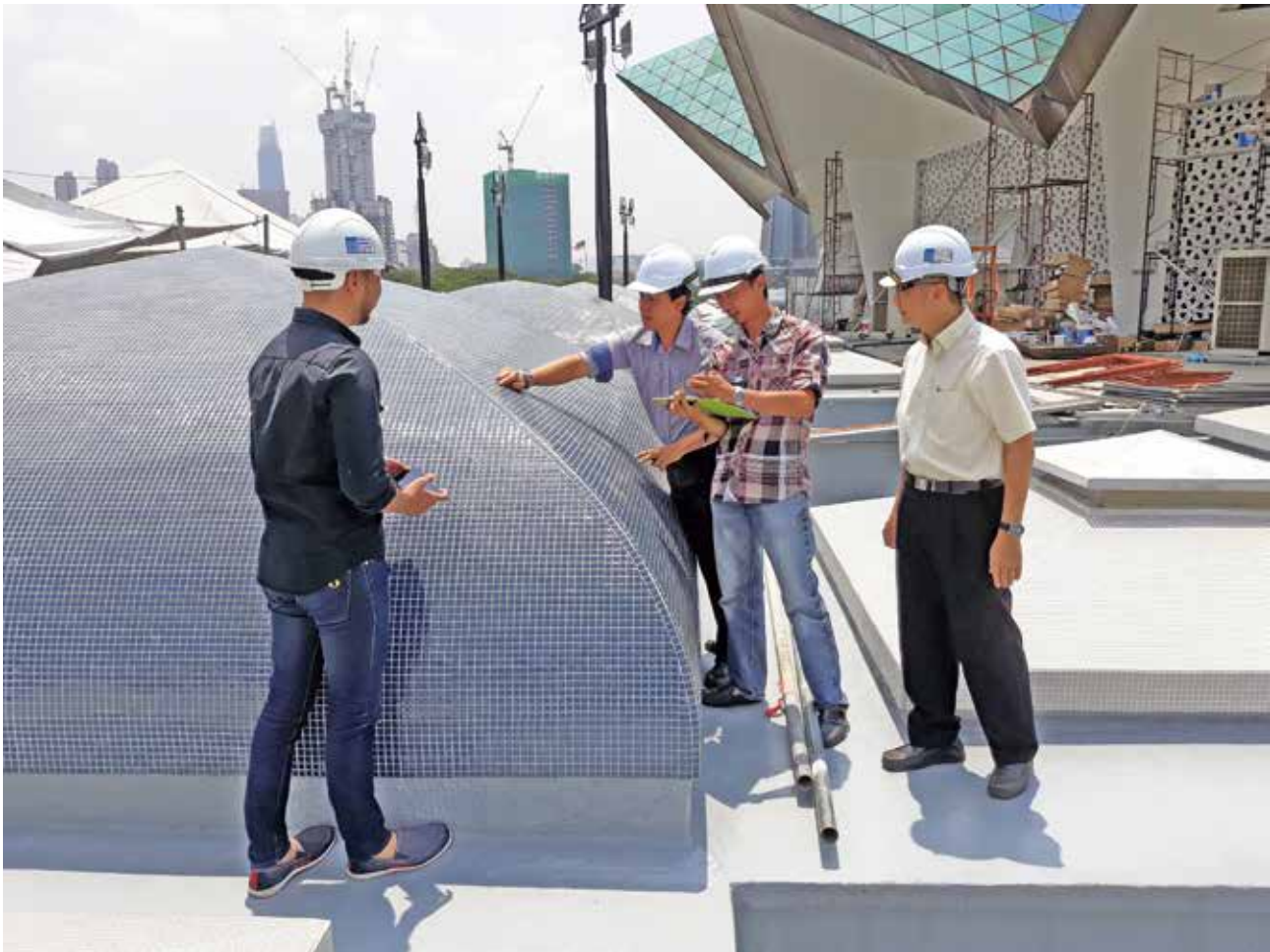
Regular inspections were carried out by all parties to ensure the quality of workmanship after the installation of glazed porcelain mosaics and the application of waterproofing coating on the flat roofs of the National Mosque.
