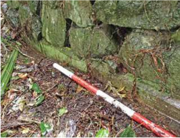
Figure 21. The strip concrete foundation onto which the stone rough stones walls were built, 29 April 2018 (Photo: Matthew Schmidt).
