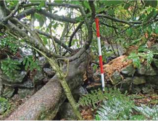
Figure 15. Damage to a wall from a collapsed tree (Photo: Matthew Schmidt).
