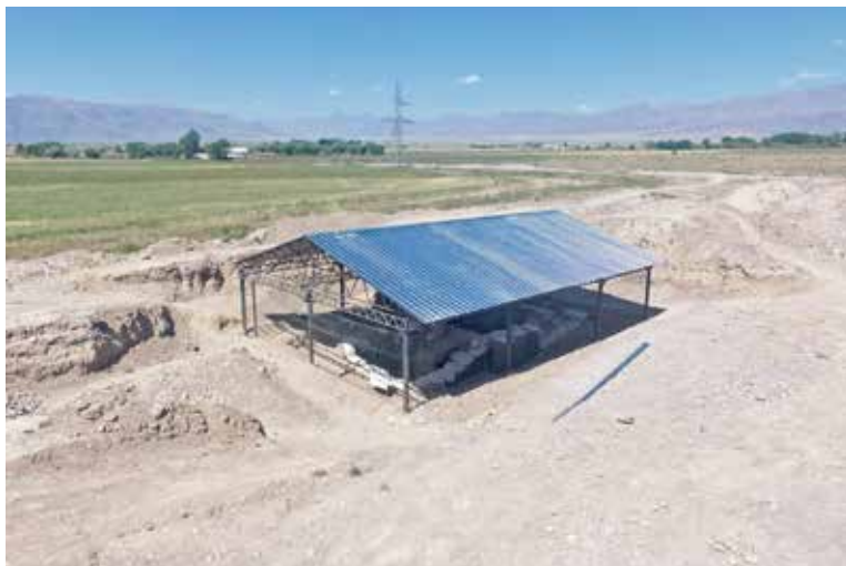
Fig. 6. The metallic shed over the Kyok-Tash mausoleum.
