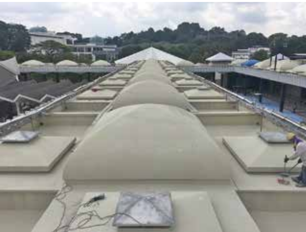
The flat roofs of the National Mosque covered by polyurea waterproofing coating.
