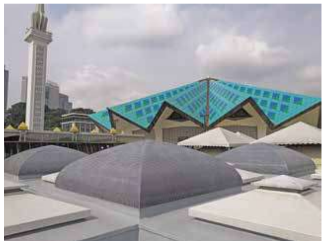
The domes and pyramid roofs of the National Mosque after the installation of new glazed porcelain mosaics.
