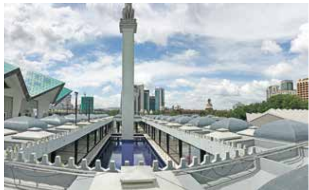
Upon completion, a total of 13,482,953 new glazed porcelain mosaic pieces were used to cover 95 domes and 270 pyramid roofs on the flat roofs of the National Mosque.
