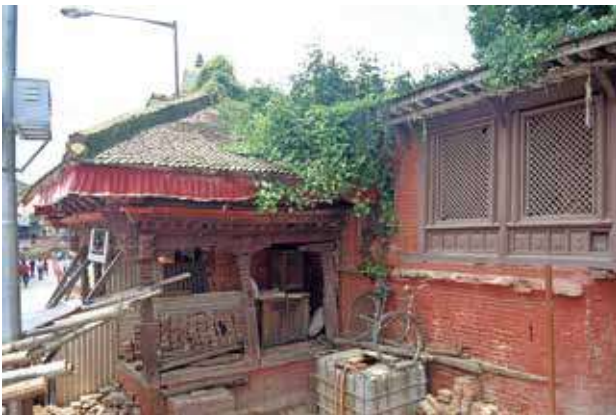
Fig 7. A view from north. The temple is attached to the boundary wall along the western edge. The desolate rear garden and heavy vegetative growth and ground moisture are taking its toll on the temple structure (2017-07-25).
