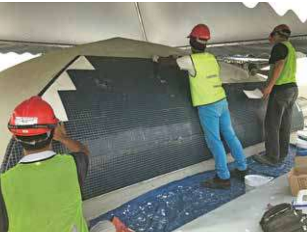
The installation of new glazed porcelain mosaics on the dome was carried out from the bottom layer and working upwards.
