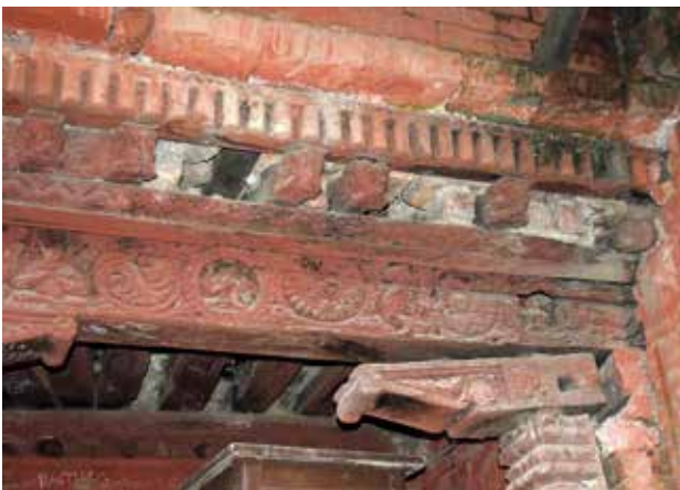
Fig 8. Dhalin khva above the nina are in a critical state due to a long period of exposure to wet rot. The faces carved in dhalin khva are not recognizable. The corner post and meth are dislocated (2017-07-25).
