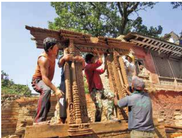
Fig 13. Installing the main sanctum door in its proper position. Such carved doors are assembled from many complex smaller carved members which are correctly put together by master carvers (2017-11-7).
