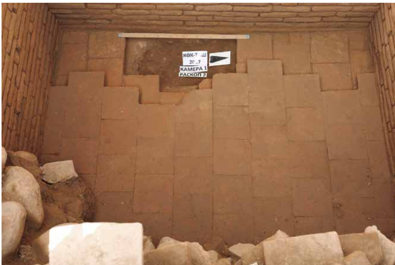
Fig. 4. The floor of the first room of the Kyok-Tash mausoleum.
