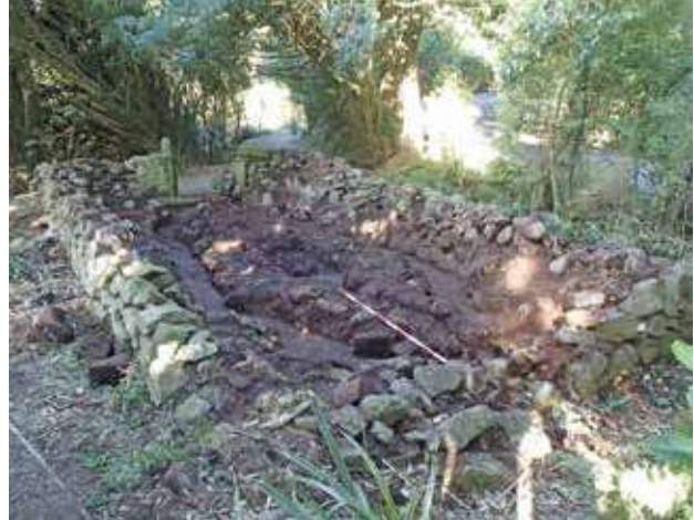
Figure 30. The fernery after the 26 August 2018 excavation showing the layout of the structure. The entranceway is in the background, the pond in the centre and the path leading part way round the fernery interior, 26 August 2018 (Photo: Matthew Schmidt).
