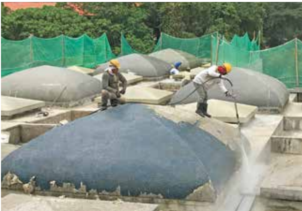
Removal of the existing layer of waterproofing coating on domes by using an 11,000 psi high pressure hydro jet, revealing the original glazed porcelain mosaic in blue.
