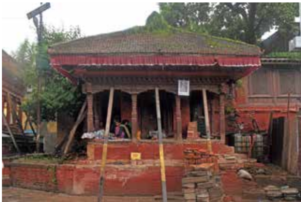
Fig 2. The east elevation of the temple. Raking shores are provided to support the temple roof (2017-07-26).
