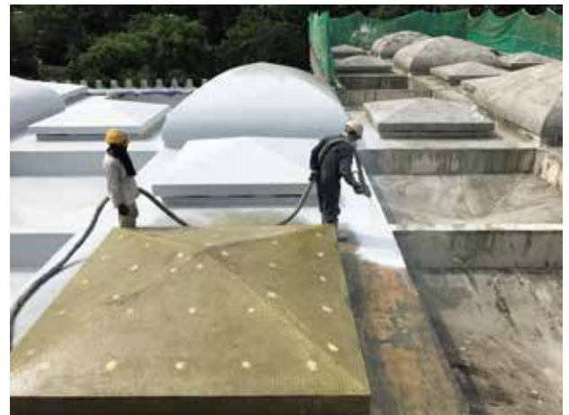
The spraying of 2 mm-thick polyurea waterproofing coating on the primed surfaces of the domes and pyramid roofs.
