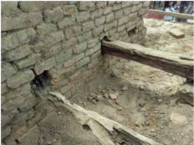
Fig 10. Almost all of the floor joists on the first-floor level were decayed due to wet rot (2017-08-29).
