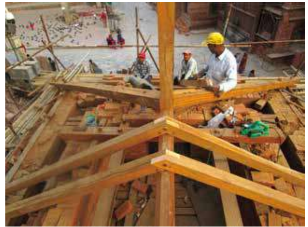
Fig 15. Carpenters laying the roof rafters (2018-1-31).
