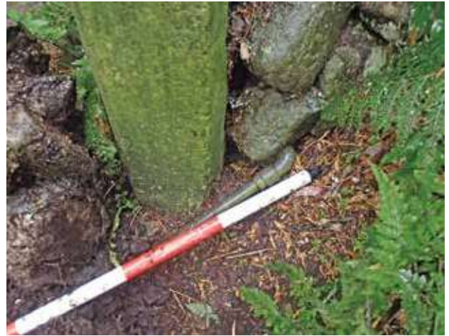
Figure 24. Water pipework coming into the fernery from an exterior water source (Photo: Matthew Schmidt).
