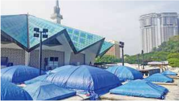
Canvas sheets were used to cover the domes and pyramid roofs after the outer-most layer of glazed porcelain mosaics had been removed. This was to protect the exposed surfaces from water penetration.
