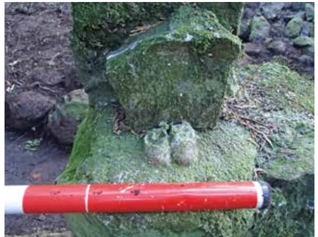
Figure 36. Small concrete boots from a missing statuette which used to be on top of the Oamaru stone entranceway pillars (Photo: Matthew Schmidt).
