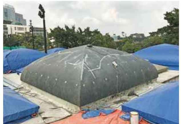
The dome after completion of work using the "Helifix-DryFix" stainless steel helical pinning system.
