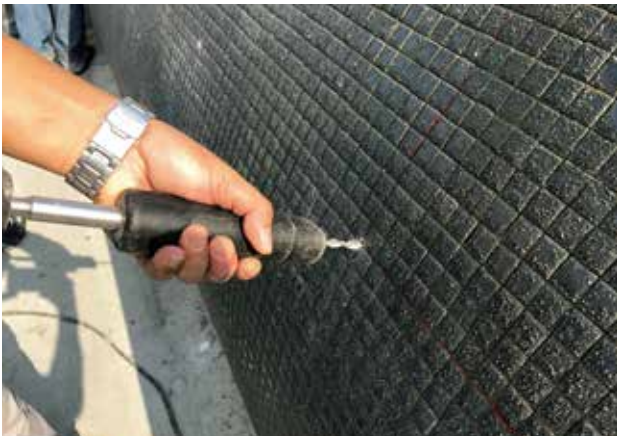
Rehabilitation of the reinforced concrete structure or substrate of the domes was carried out by driving 8 mm-diameter "Helifix-Dryfix" stainless steel helical pins through the pilot holes and into the reinforced concrete structure or substrate.
