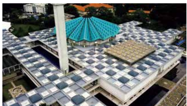
An aerial view of the National Mosque with its newly conserved flat roofs.
