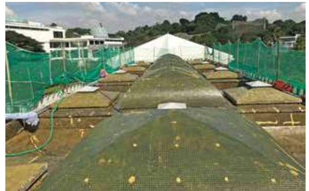
The domes and pyramid roofs were primed with epoxy scratch coat after application of the helical pinning system.
