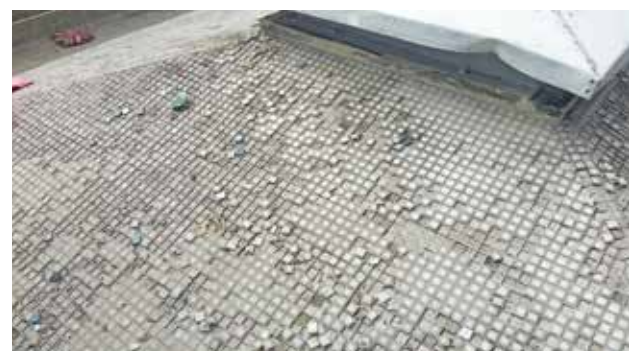
Similar to the domes, the glazed porcelain mosaics on the pyramid roofs were found to be either missing, detached, loosened or to have fallen off, exposing the old layer of waterproofing coating.
