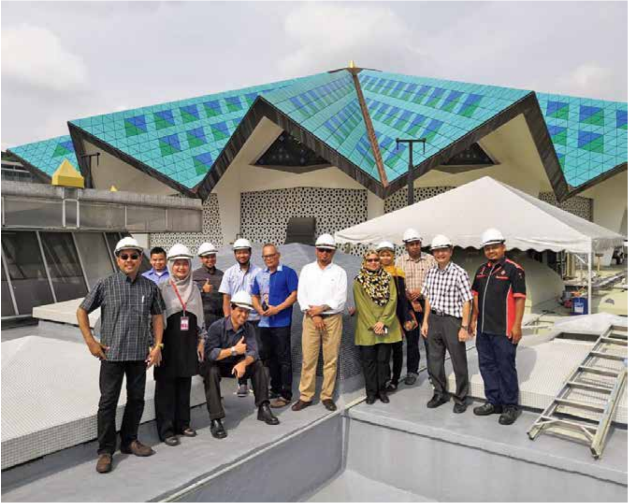
The conservation of the flat roofs at the National Mosque represents an outstanding masterpiece of well-orchestrated efforts by all consultants, building contractors and government agencies involved in the project.
