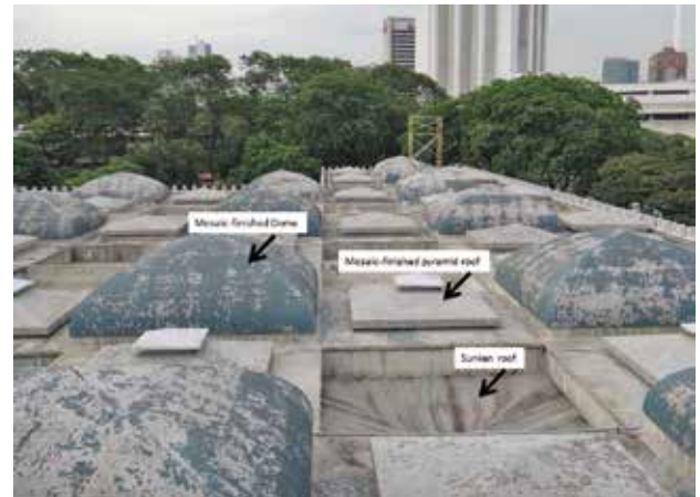
The flat roofs of the National Mosque accommodate mosaic-finished domes, mosaic-finished pyramid roofs, sunken roofs and skylight roofs. Each roof type measures 4 m x 4 m at the base. The height of the dome is 1.8 m, the pyramid roof is 0.8 m and the sunken roof is 1.3 m deep.
