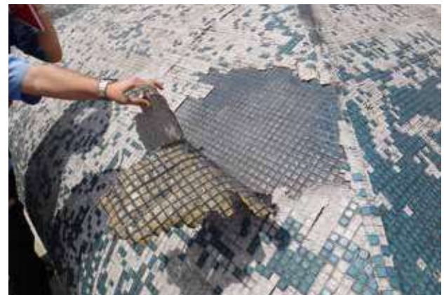
The ageing top layer of glazed porcelain mosaics on the domes of the National Mosque were found to be either missing, detached, loosened or to have fallen off, exposing the old layer of waterproofing coating and the original mosaics. This condition had caused water penetration, trapped moisture and roof leakage onto the prayer halls and other spaces underneath the flat roofs.
