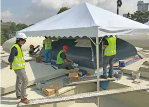
Temporary tents were erected to cover each dome and pyramid roof during the mosaic installation stage in order to protect them from direct sunlight and heavy rain.
