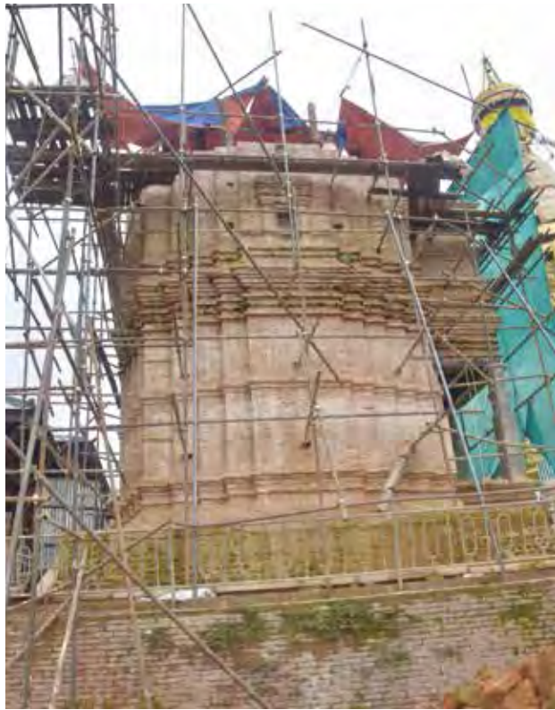
Anantapur Temple during the rehabilitation process
