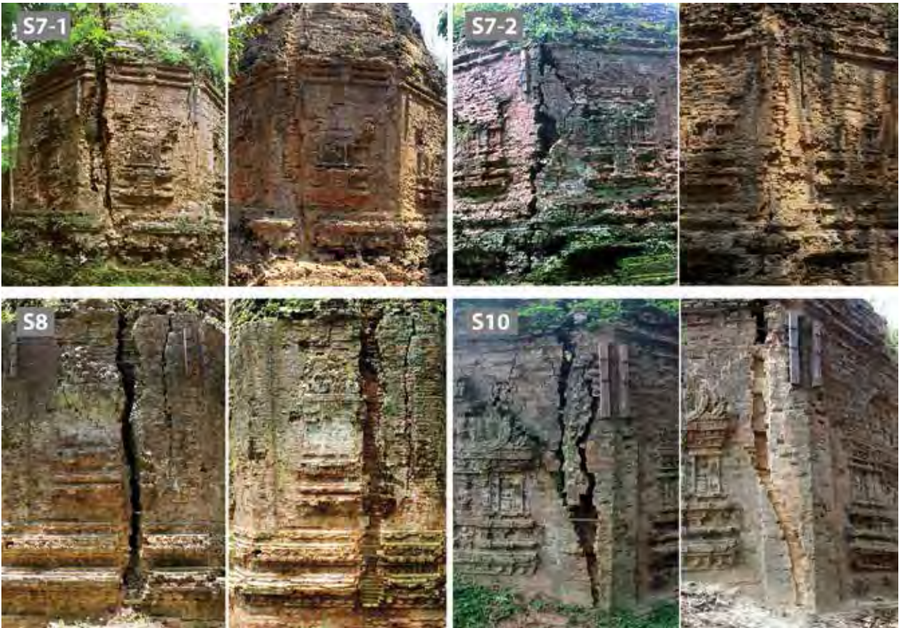
Examples: Partial emergency conservation, before and after conservation.
