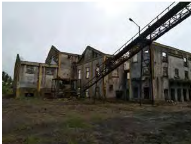
Figure 2: Salak Power Plant Complex in Salak Power Plant Compound (in Area A) (Copyright Owner: Prita Wikantyasning)
