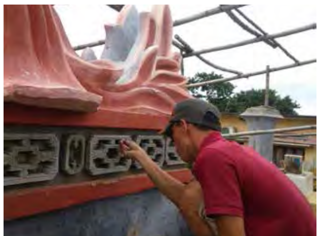
20. Decorative patterns re-installed in their original positions
