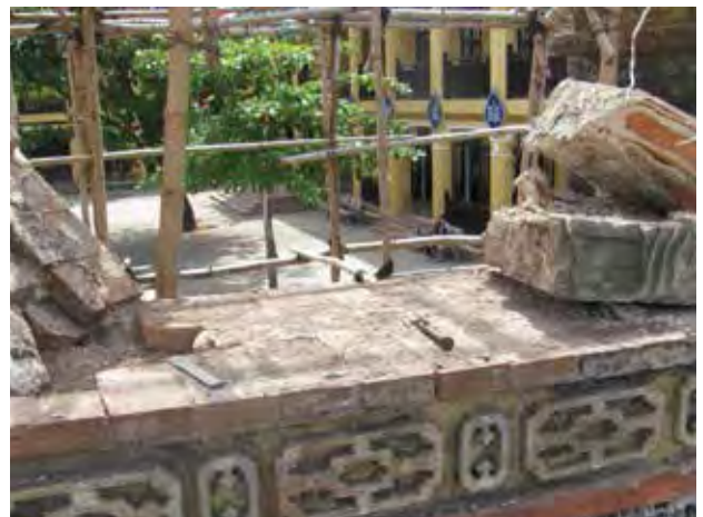
14. Cleaned and reinforced broken elements
