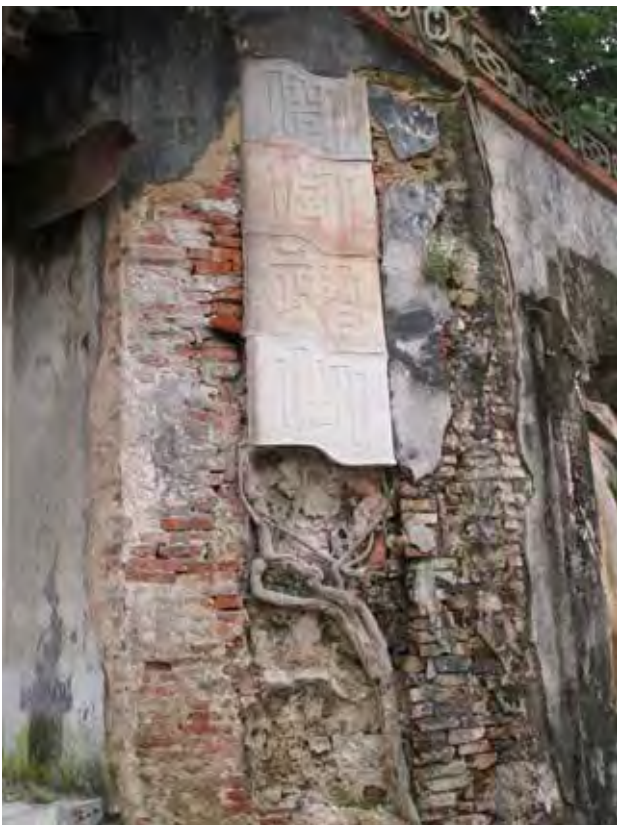
5. Some components had fallen off the wall.
