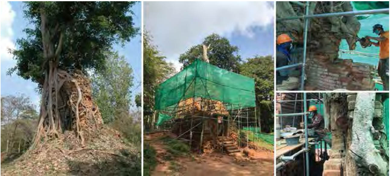
The S3 gate before, and during restoration and activities.
