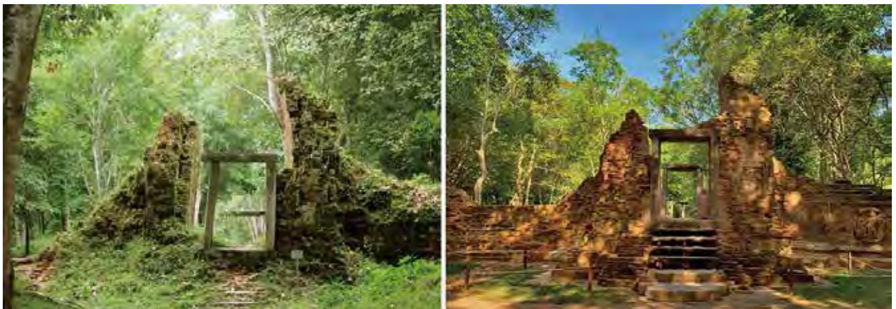
The S5 gate before and after restoration.
