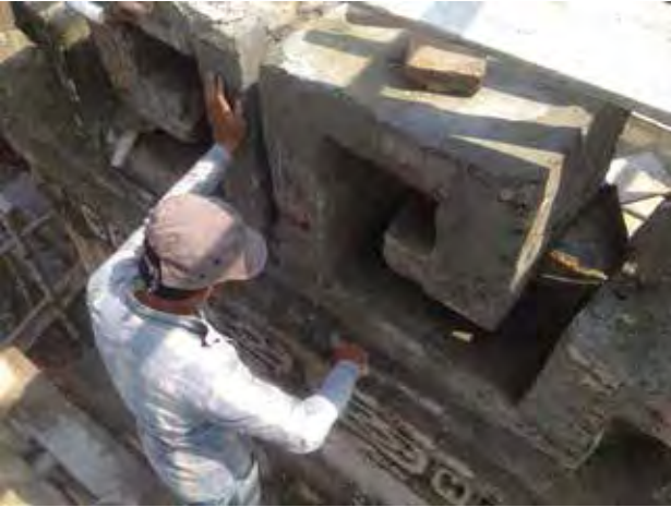
15. Attached, patched broken elements being placed back in their original position
