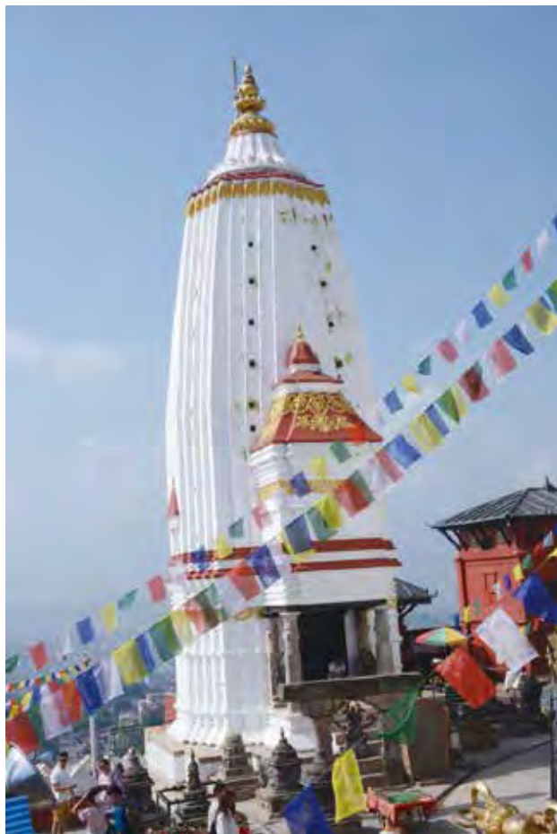
Anantapur Temple after rehabilitation
