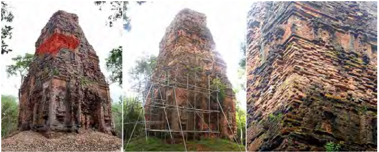
Example: Z1 tower: Partial emergency conservation, before (left), during (middle) and after conservation (right).
