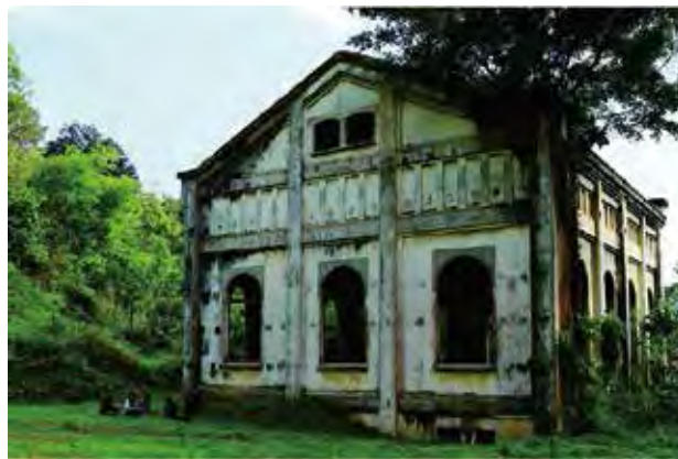
Figure 1: The Compressor Building is one of significant objects in Doerian Mining Pit Compound (in Area A) (Copyright Owner: Office of Cultural Affairs, Historical Remains Museum of Sawahlunto Municipality)
