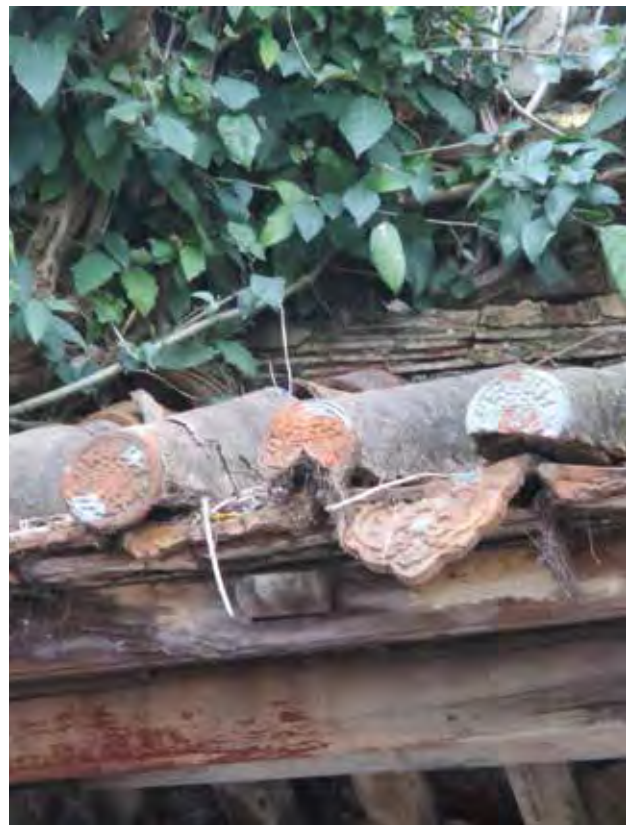
6. The majority of wooden frames had rotted.
