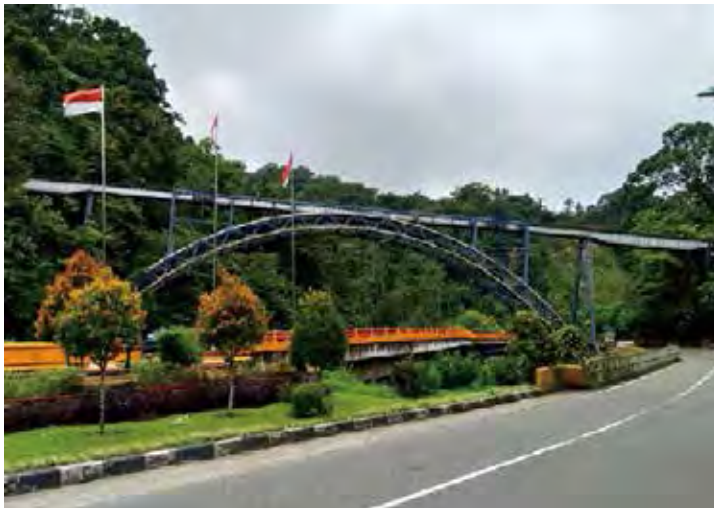
Figure 4: Tinggi Bridge (in Area B) (Copyright Owner: Prita Wikantyasning)
