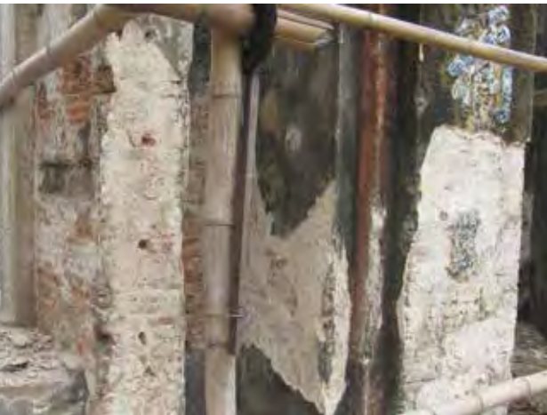
17. Flaked lime mortar walls were taken out.
