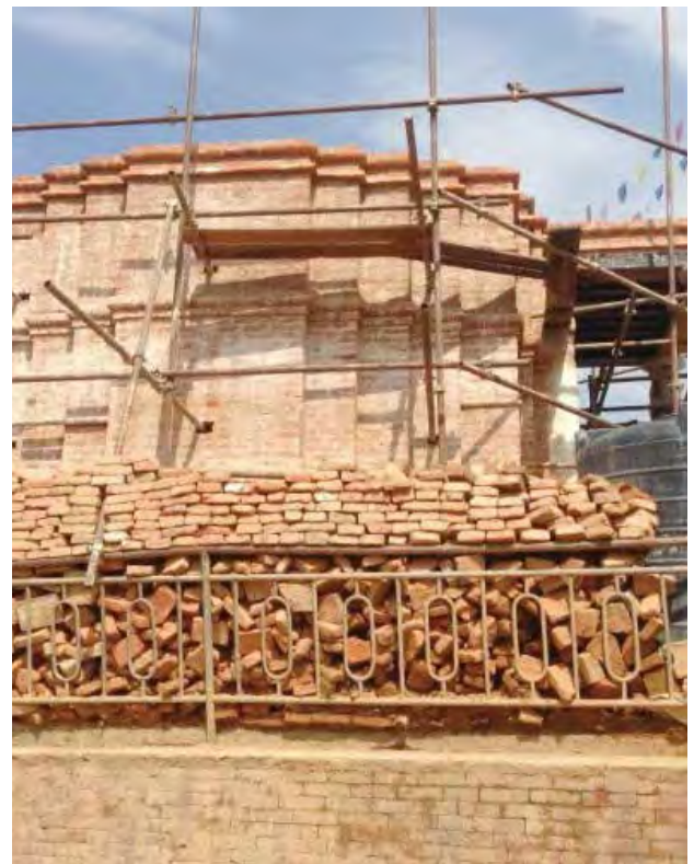
Anantapur Temple during the rehabilitation process
