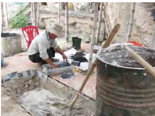
25. Experienced worker mixing traditional lime mortar
