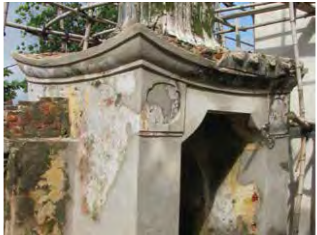
18. Wall rendered with lime mortar
