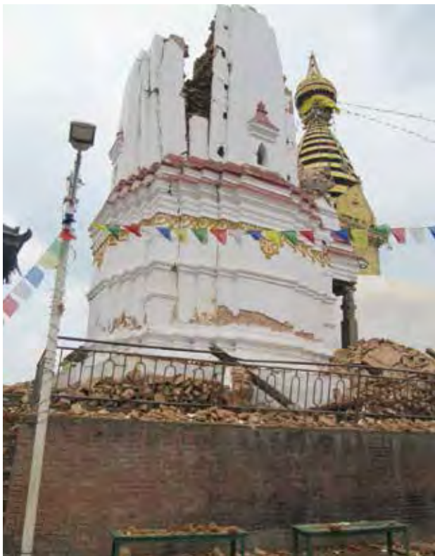
Anantapur Temple damaged by the 2015
