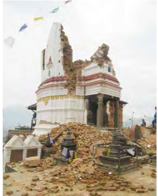
Anantapur Temple damaged by the 2015
