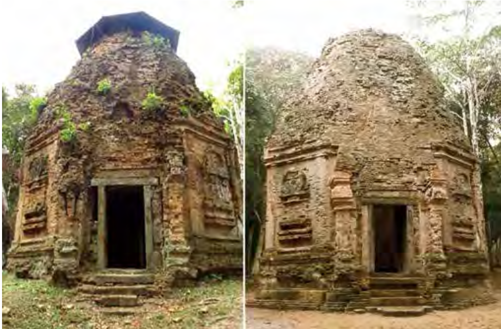
The S11 tower before and after restoration.
