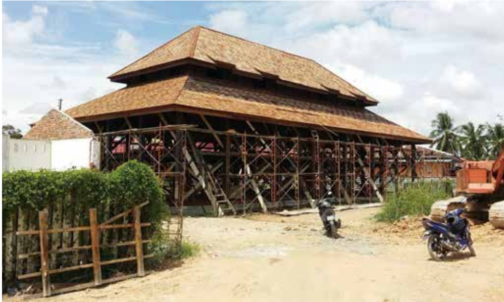
Exterior view of Fort Lili during conservation.
