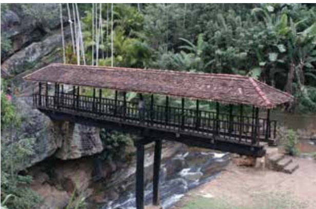
Bogoda wooden bridge
