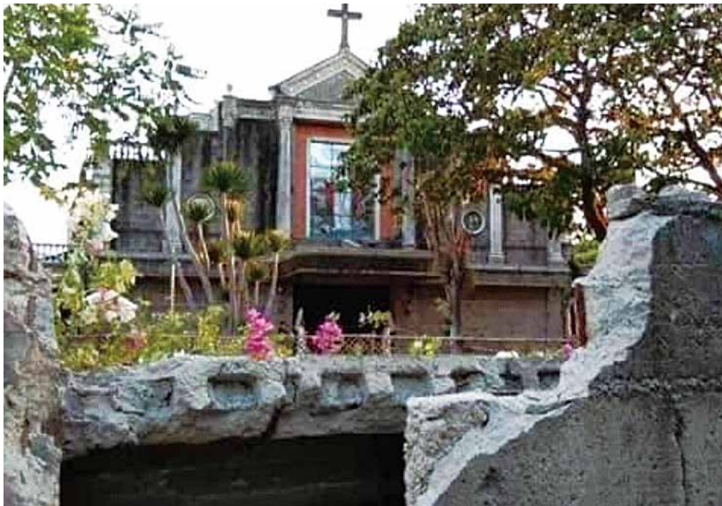
Fence cracks at Monasterio de Santa Clara, Betis
