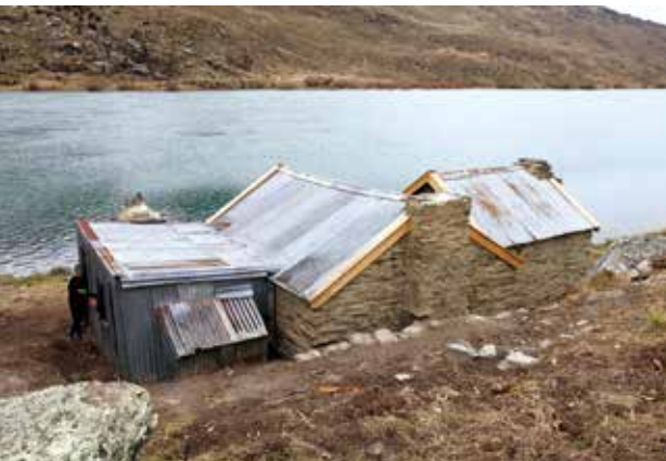
Figure 33. The back of the cottage showing barge boards and capping repaired and replaced, and iron roofing mostly left in place as it was water tight (Photo: Matthew Schmidt).
