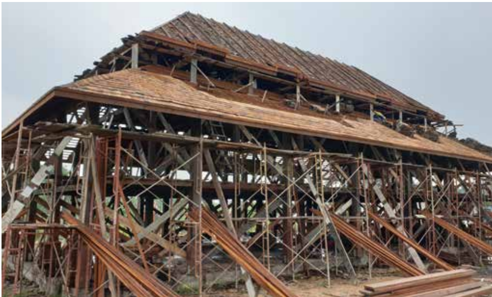
During the conservation works, Fort Lili underwent major refurbishment and restoration including the dismantling of building structures, salvage of building materials, storage, conservation treatment and reconstruction.
