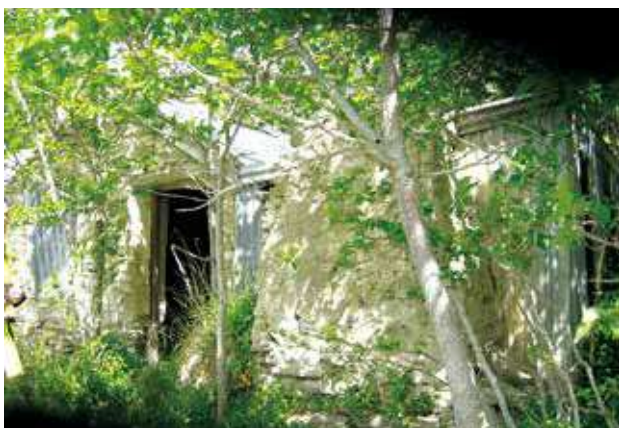
Figure 9. The cottage completely overgrown along the front (Photo: Matthew Schmidt).
