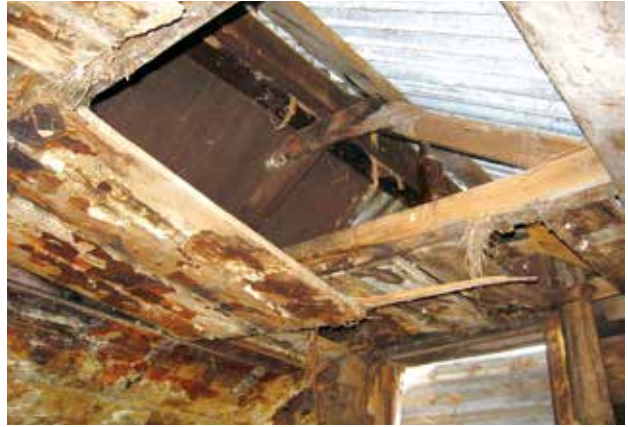
Figure 12. The tongue and groove timber ceilings were in a poor condition but repairable (Photo Matthew Schmidt).
