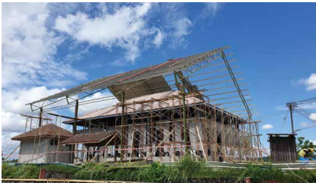
Temporary roofing was installed to protect Fort Emma during conservation.
