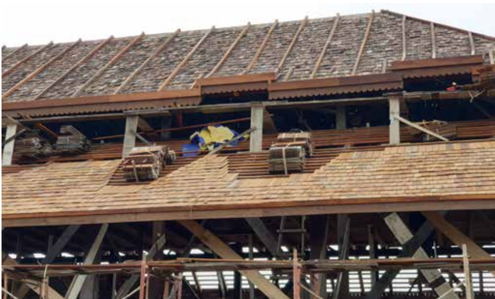
During the conservation of Fort Lili, a double-layered roofing system was introduced to allow the installation of proper insulation while maintaining the visibility of the underside of the belian shingles.
