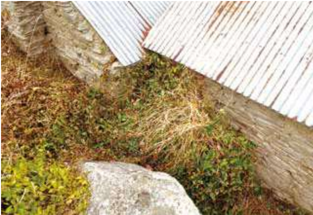
Figure 21. The back of the centre and south stone bays just before the 2019 conservation works (Photo: Matthew Schmidt).
