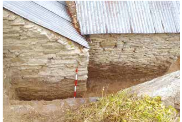
Figure 22. The back of the centre and south stone bays after fill removal in May 2019 works. Note the dark areas on the stonework indicating the level the earth fill came up to behind the cottage creating the damp back walls (Photo: Matthew Schmidt).
