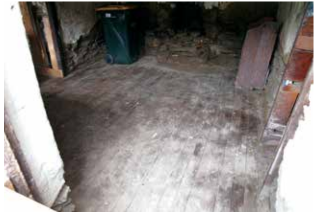
Figure 30. Centre Bay floor cleaned with only minor repairs required (Photo: Matthew Schmidt)
