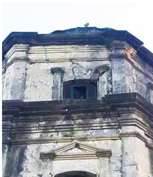
Cracks at belfry of Santa Rita de Cascia Parish, Sta. Rita
