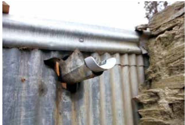
Figure 32. Stormwater gutting repaired using original and new elements to take water away from the cottage (Photo Matthew Schmidt).
