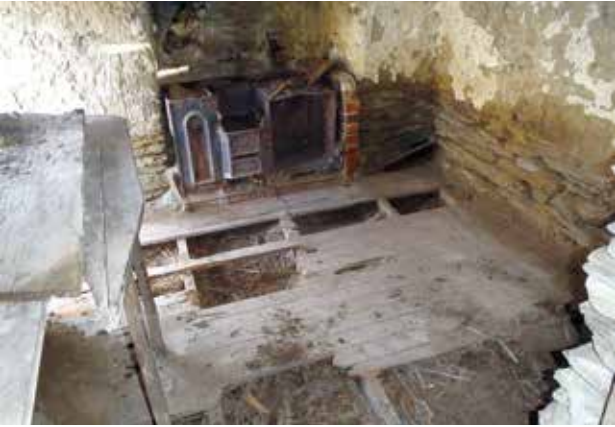
Figure 11. The cottage interior, South Bay shown, was relatively dry with various debris and holes in the floor. South Bay shown (Photo: Matthew Schmidt).
