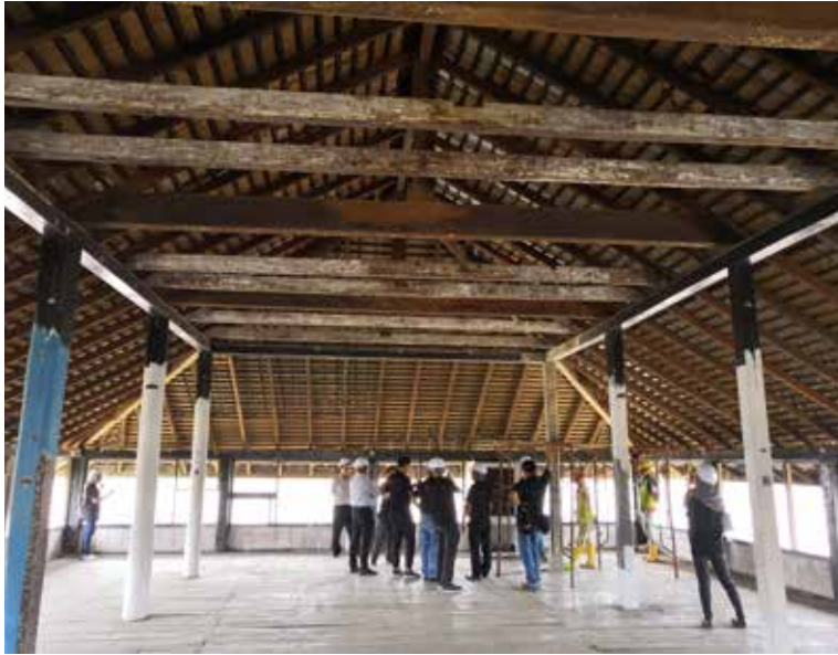
Interior view of Fort Emma during conservation.
