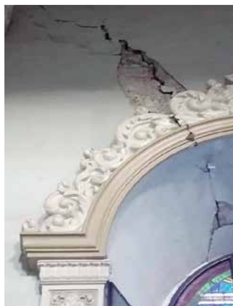
Wall cracks at the Holy Rosary Church, Angeles Parish
