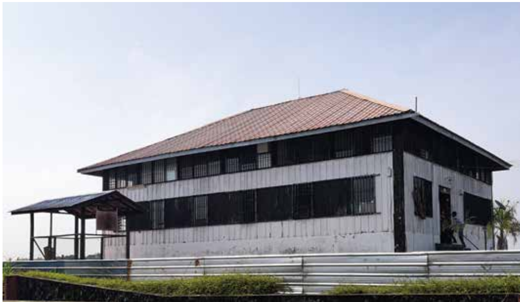
Exterior view of Fort Emma before conservation.
