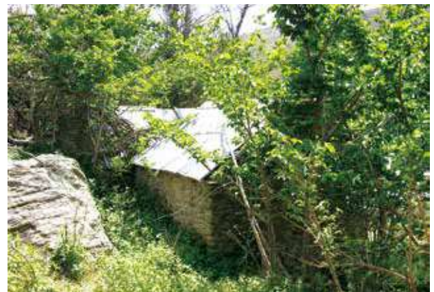
Figure 8. The cottage completely overgrown along the back with a fallen tree lying on the cottage (Photo: Matthew Schmidt).
