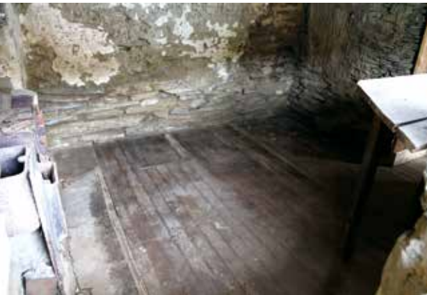
Figure 31. South Bay room floor repaired and room cleaned (compare to Figure 11) (Photo: Matthew Schmidt).
