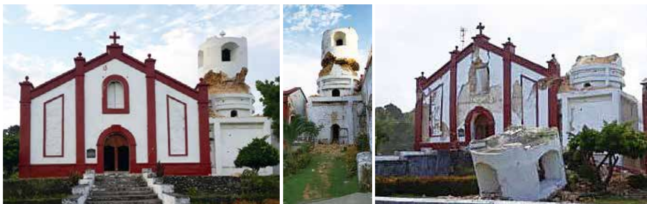
Itbayat Church: The bell tower fell after a series of earthquakes and aftershocks in July 2019
