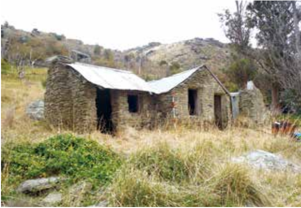
Figure 19. Front of cottage just before the 2019 conservation works (Photo: Matthew Schmidt).
