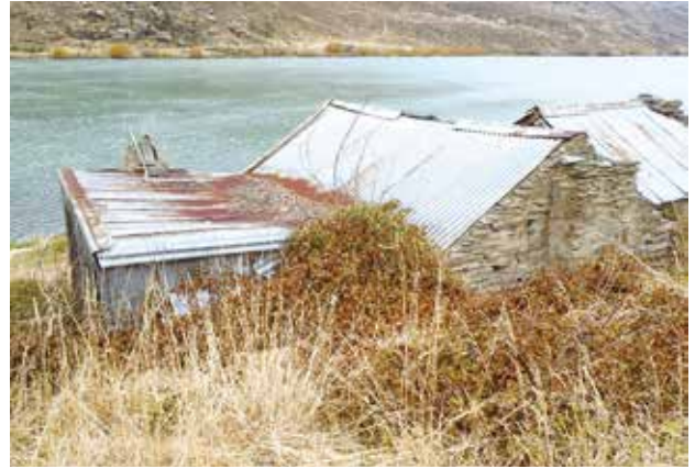
Figure 20. The back of the corrugated iron north bay (20th century) and central stone bay (ca. 1863) just before the 2019 conservation works (Photo: Matthew Schmidt).
