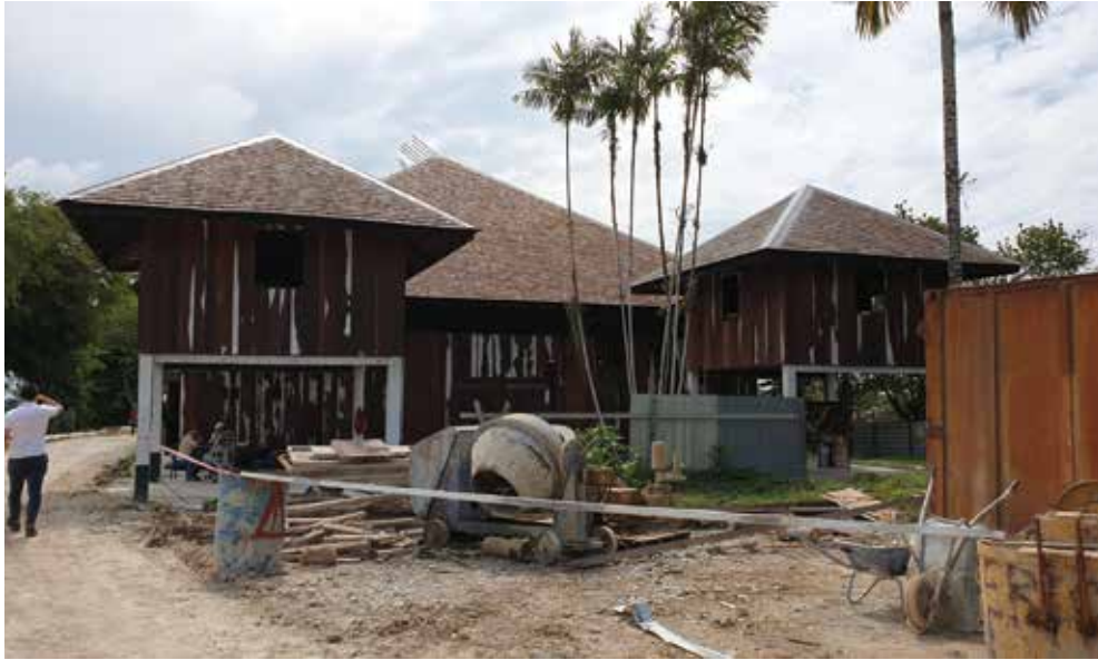
The back view of Fort Hose during conservation.
