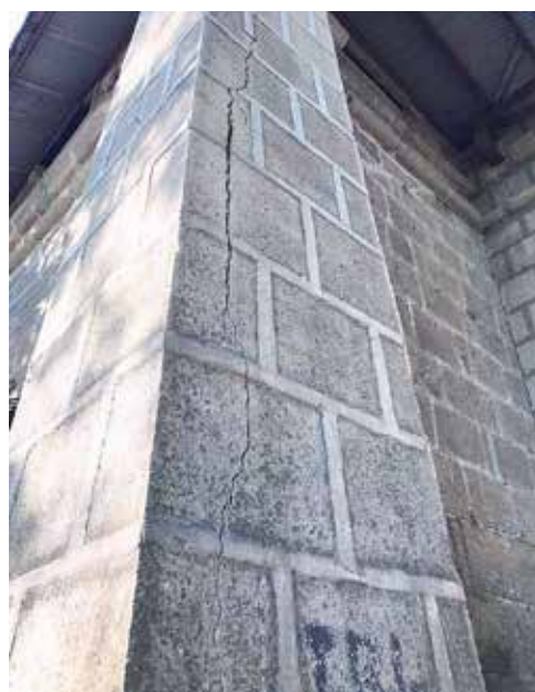
Cracks on wall at Santa Monica Parish
