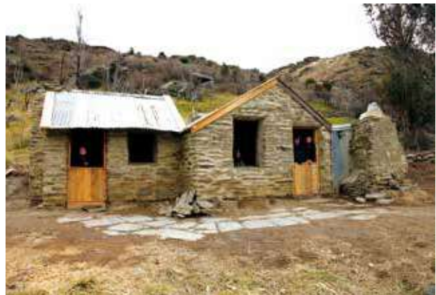
Figure 34. Stonework, carpentry and excavations around the cottage completed. Note the self-closing doors to stop sheep entering the building. Visitors enjoying the cottage (Photo: Matthew Schmidt).
