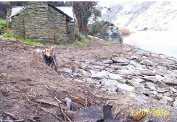
Figure 17. The wave wall to protect the cottage from erosion soon after completion (Photo: Daniel Druce).
