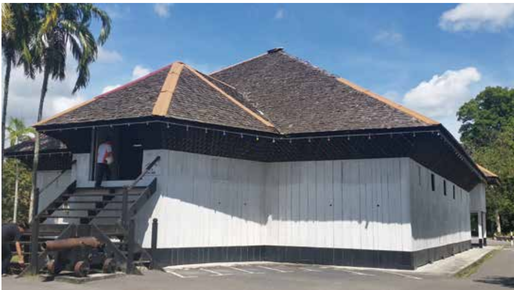
Front view of Fort Hose before conservation.
