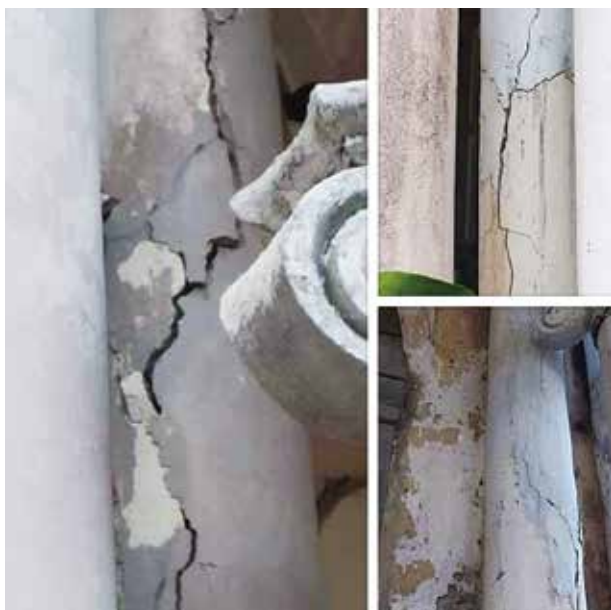
Cracks on columns at St. James de Apostle Parish, Betis, Guagua
