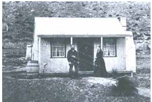
Figure 26. A miner's dwelling mid-19th century from the Otago Goldfields showing a wooden barrel to store fresh water (Image: Hocken Collections ref Kawarau Gorge 1241 01 002A).
