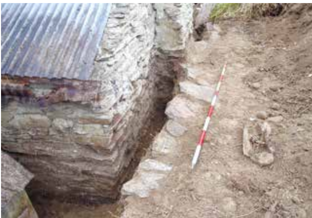
Figure 23. The back of the central stone bay (ca. 1863) after fill removed in May 2019 (Photo: Matthew Schmidt).
