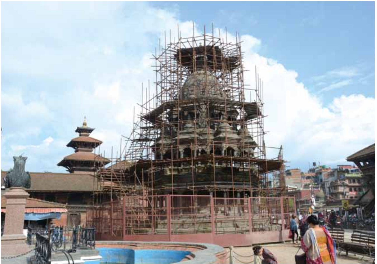
2-11 Radha Krishna (Octagonal) Temple, work on going
