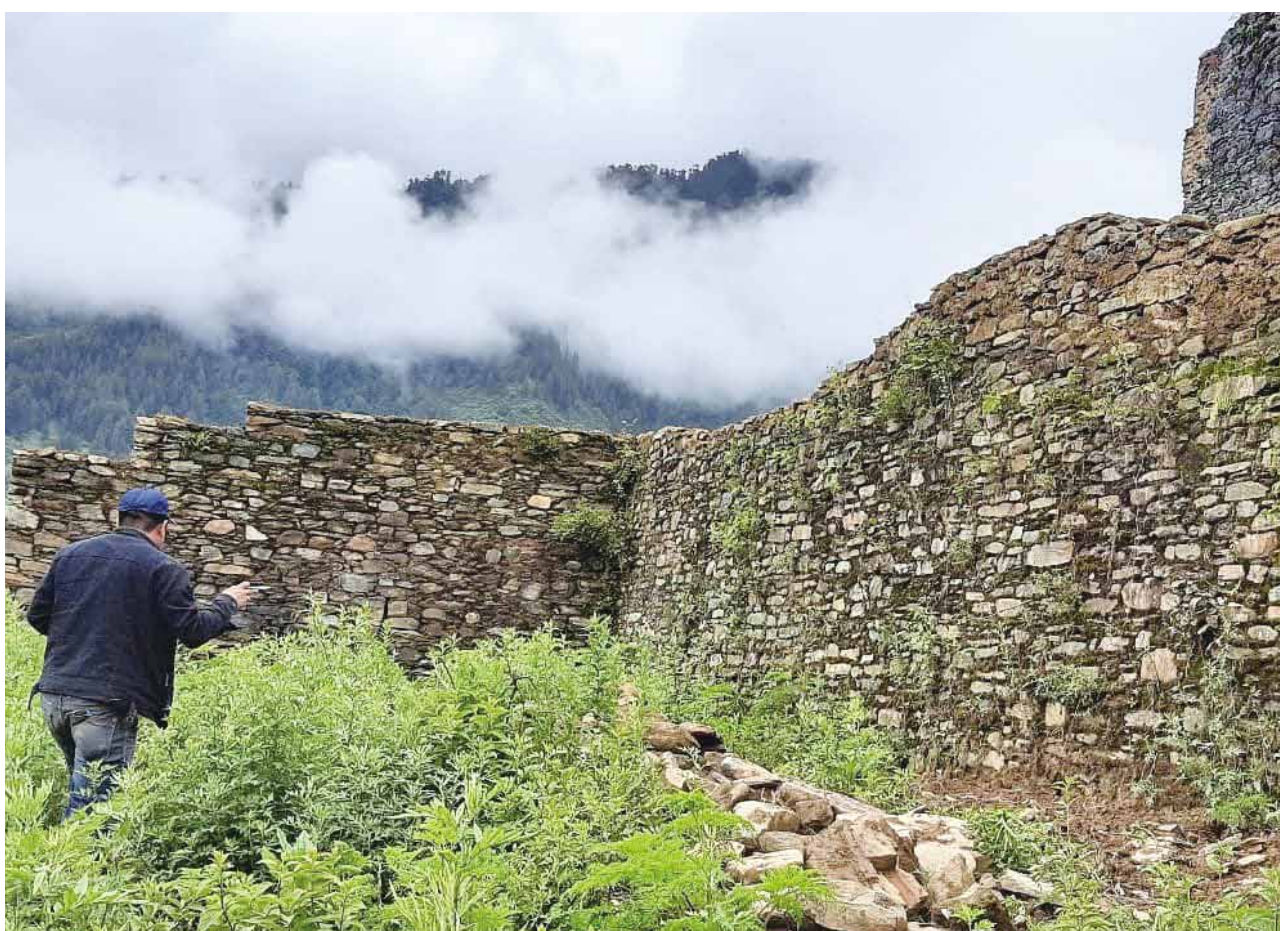
Fig. 5 After consolidation works of shabkhor (surrounding) structure
