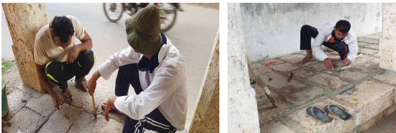
Fig. 18 & Fig. 19: Pointing work before conservation
