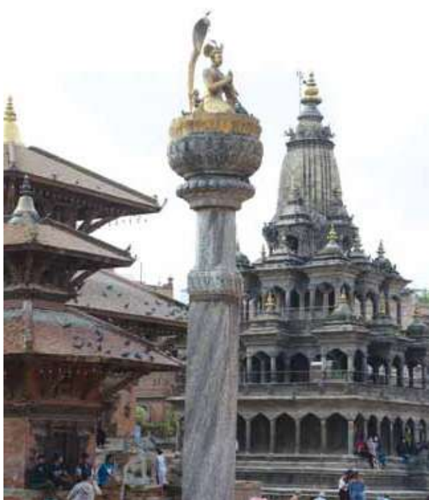
2-8 Yognarendra Malla Pillar after rehabilitation
