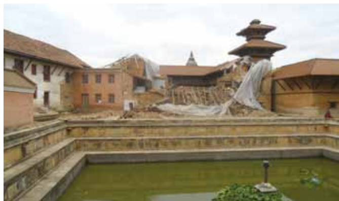
1-1 Sundari Chowk, collapsed by the earthquake
