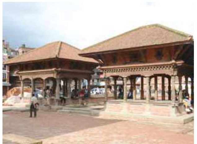
2-5 Maniwandapa after rehabilitation
