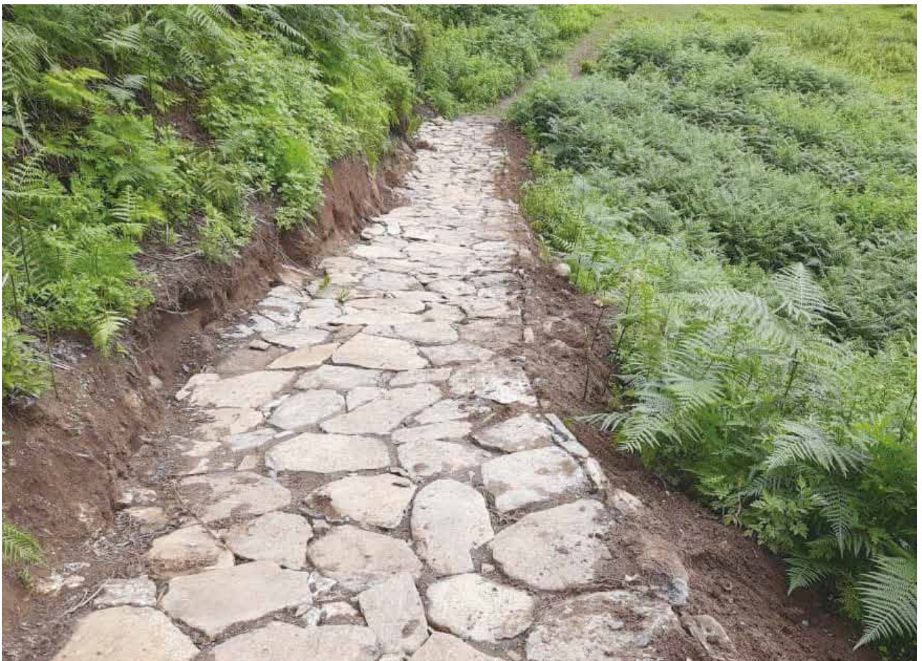
Fig. 11 Construction of the new footpath to the site
