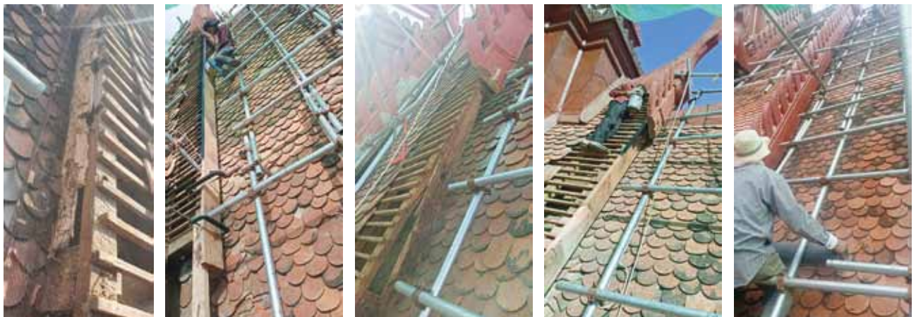
Damaged timber before and after restoration
