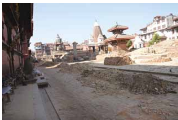
1-3 Harishankar Temple (behind the stone pillar), collapsed by the earthquake
