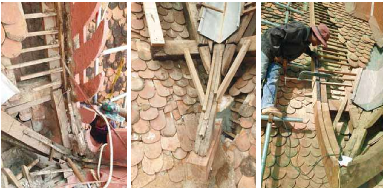
Damaged timber before and after restoration
