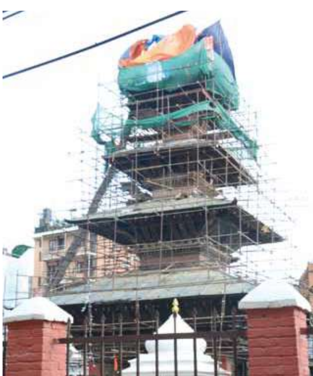
2-10 Kumbheshwar Temple, work on going
