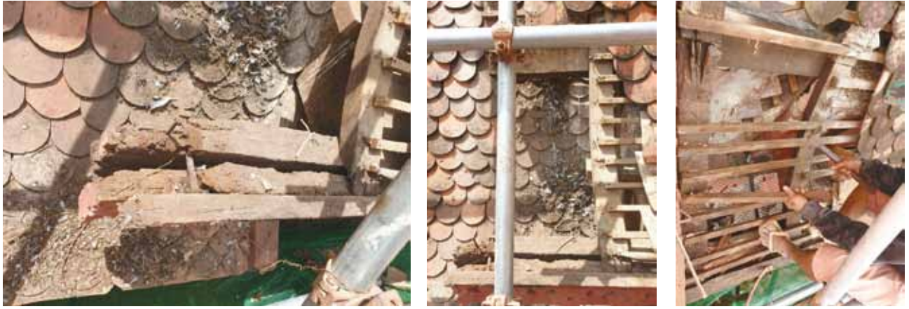
The pigeon nest and droppings on the roof
