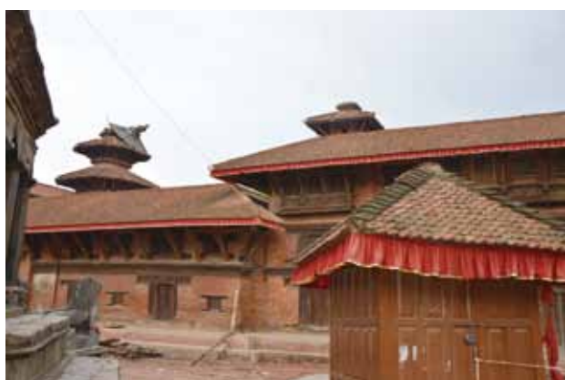
1-6 Taleju Temple, collapsed by the earthquake
