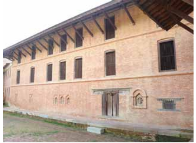
2-1 Sundari Chowk-East after rehabilitation
