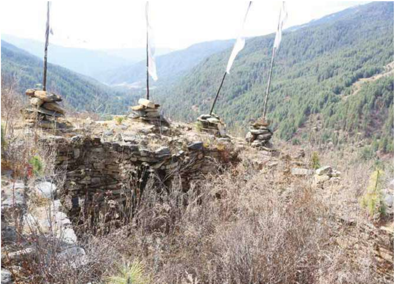
Fig. 6 Before consolidation works
