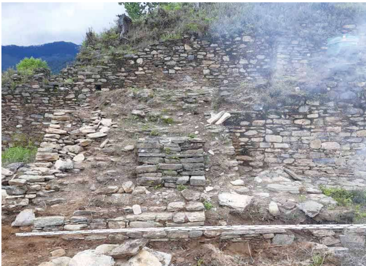
Fig. 8 Before consolidation of main entrance steps to the fortress
