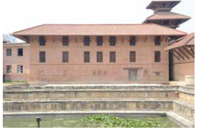
2-1-1 Sundari Chowk-East after rehabilitation
