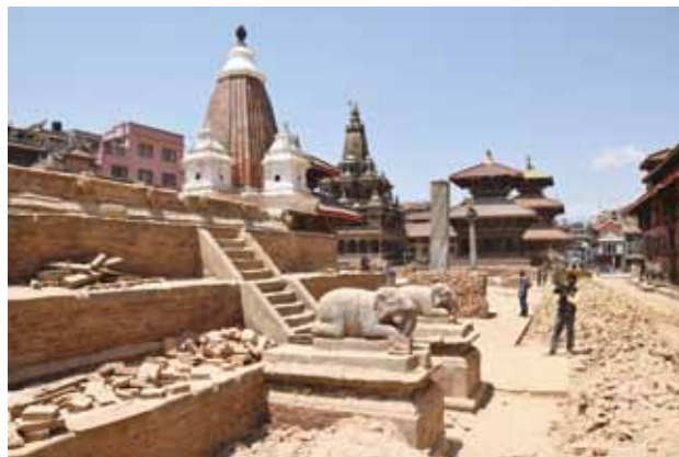
1-7 Vishweshwor Vishwanath, collapsed by the earthquake
