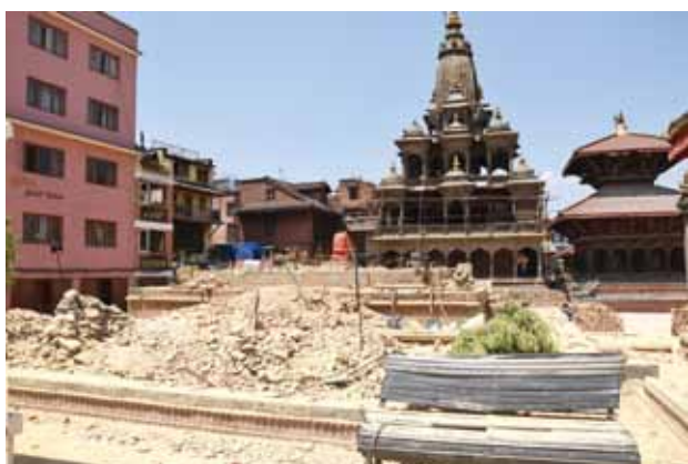
1-2 Char Narayan Temple, collapsed by the earthquake
