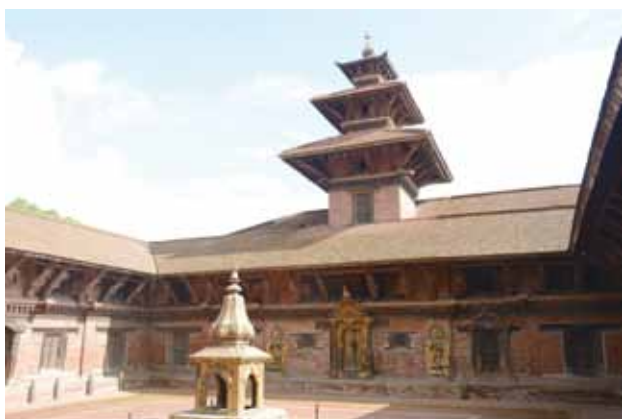
2-6 Taleju Temple after rehabilitation
