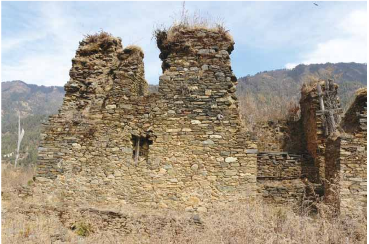
Fig. 2 Before consolidation works of Utse
