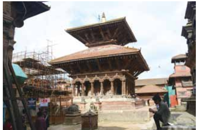
2-3 Harishankar Temple after rehabilitation
