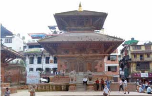
2-2 Char Narayan after rehabilitation
