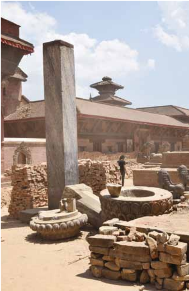
1-8 Yognarendra Statue, collapsed by the earthquake
