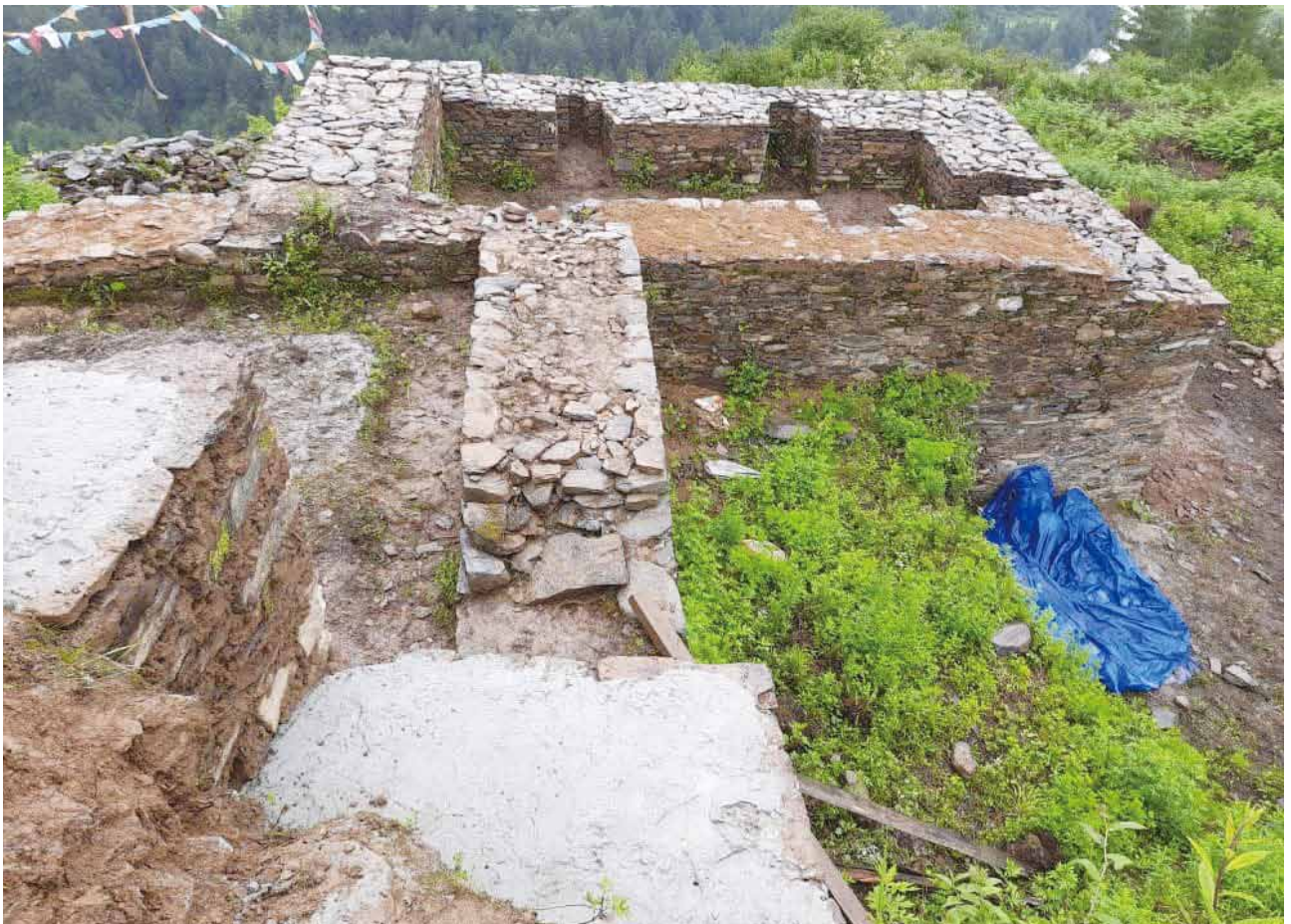
Fig. 7 During consolidation works
