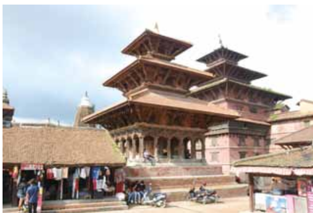
2-7 Bishweshwor Temple after rehabilitation
