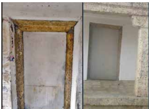
Fig. 20: Before & After, door conservation work
