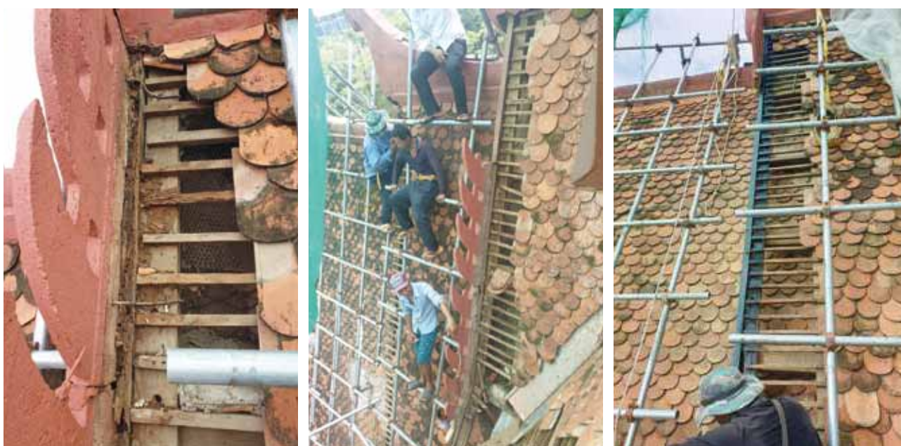
Damaged timber before and after restoration
