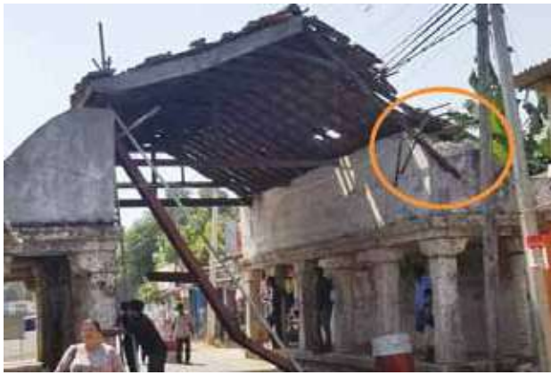
Fig. 5: Madam in 2019—After being damaged
