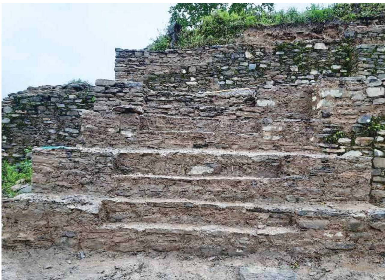
Fig. 9 After consolidation of main entrance steps to the fortress
