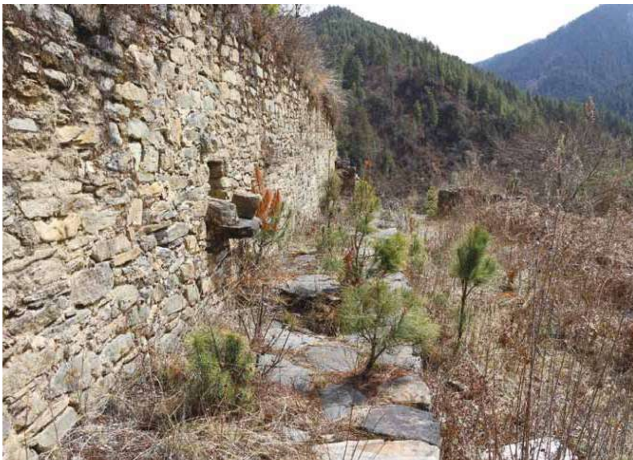
Fig. 4 Before consolidation works at the main entrance of shabkhor (surrounding) structure
