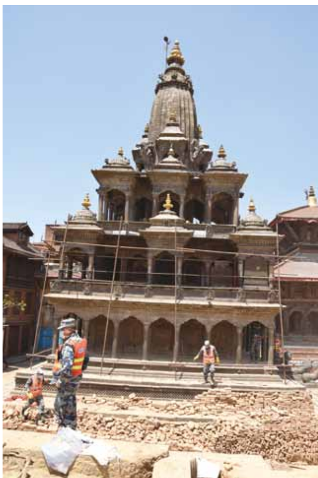
1-4 Krishna Mandir, collapsed by the earthquake
