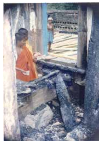
Figure 6. Floor totally burnt
