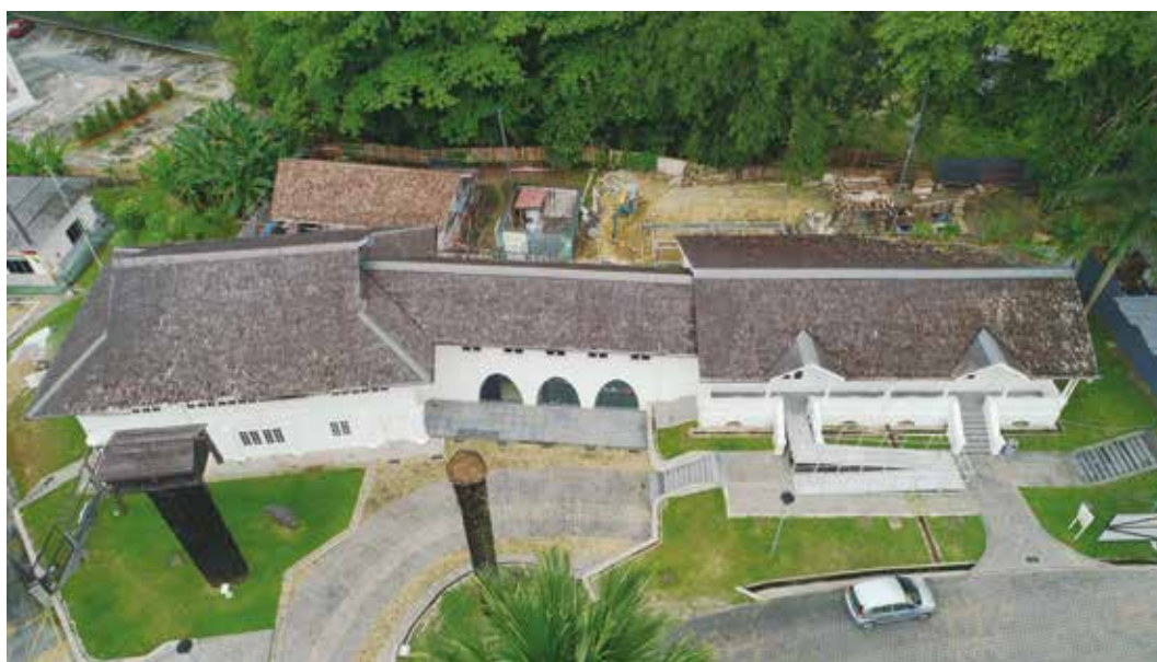
An aerial view of the Curator's House (far right) before installation of the temporary roof system
