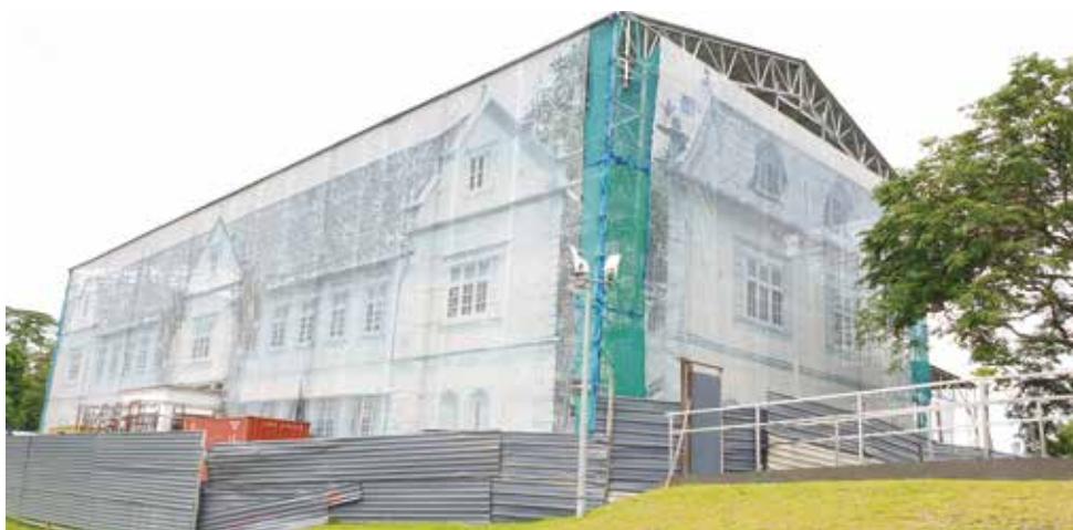
Printed netting or inkjet-mesh tarpaulin, displaying images of the Old Sarawak Museum building facade, installed to cover the building throughout the construction period. This was the first such printed netting introduced in a heritage building conservation project in Sarawak.
