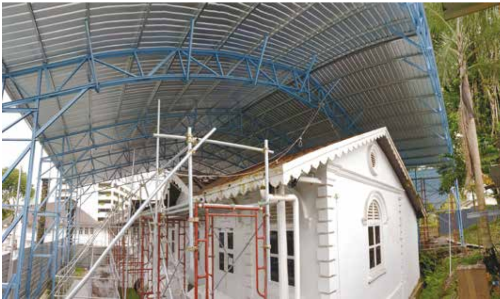
A panoramic view of the Curator's House showing its wide-span temporary roof system
