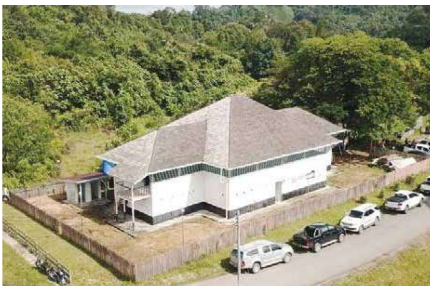
Aerial view of Fort Brooke before the installation of the temporary roof system
