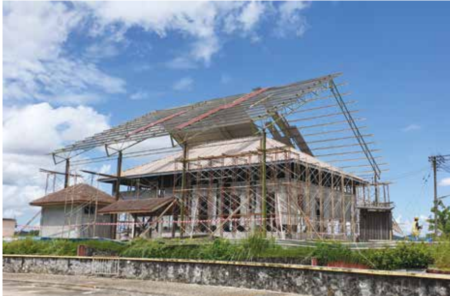
A scaffold roof system 10.5 metres high was erected for the temporary roof at Fort Emma.
