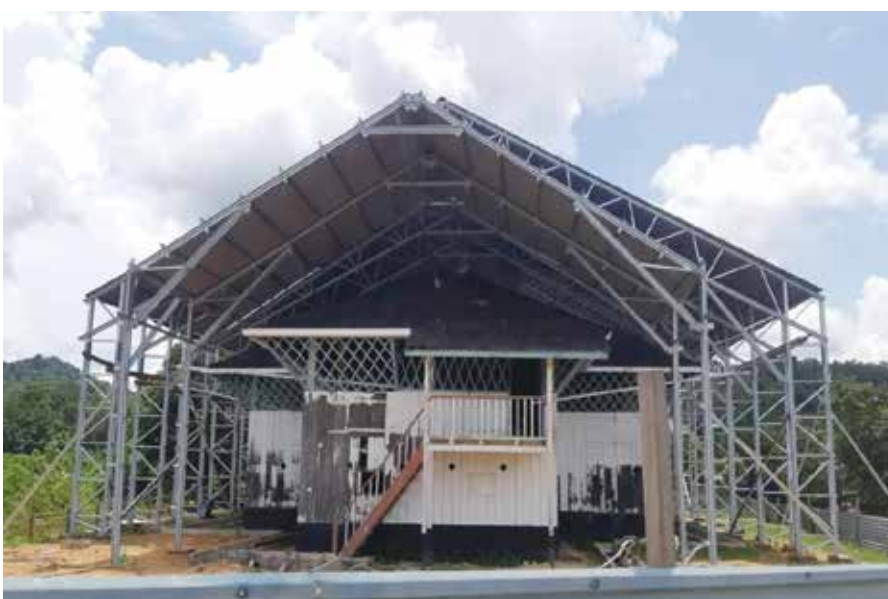
Steel truss frames of 12 metres in height were erected for the temporary roof system at Fort Brooke.
