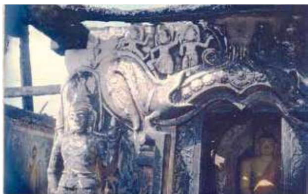
Figure 7. Damage to murals and paintings
