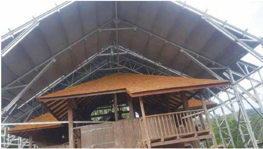
Throughout the construction period, the temporary roof system protected the roof structure of Fort Brooke from harsh weather, dust, and environmental damage.
