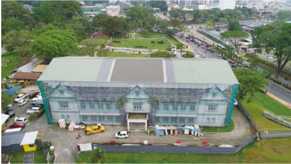
An aerial view of the Old Sarawak Museum showing its long-span temporary roof system
