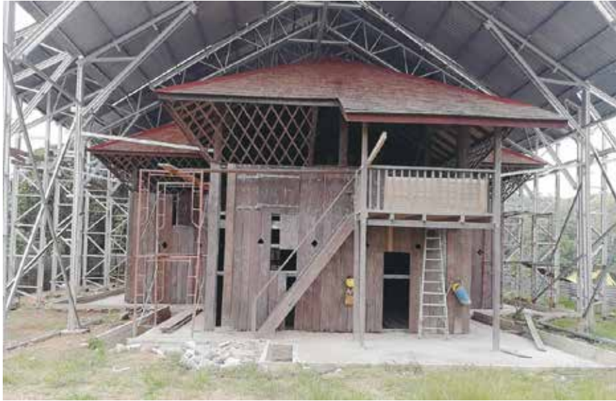
The temporary roof system at Fort Brooke provided a comfortable working environment, particularly during the installation of belian (ironwood) roof shingles.
