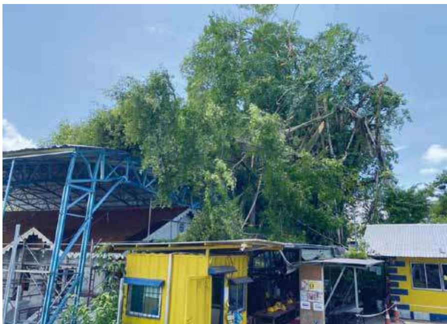
In the evening of 22 August 2020, the temporary roof saved the Curator's House from destruction when a nearby tree fell down during a heavy rainstorm.
