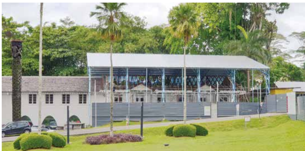
During the conservation of the Curator's House, a temporary roof 6.5 metres high using a portal framed roof system was installed.
