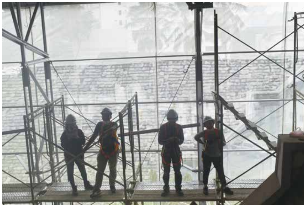
The portal framed roof system at the Old Sarawak Museum incorporated concrete footings, galvanised light-weight steel frames, and fly-bracing cables.
