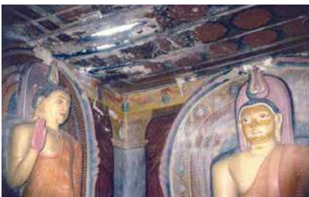
Figure 8. Damage to the decorated ceiling
