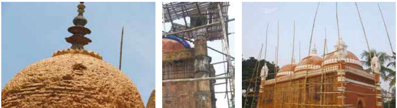
During conservation of Nayabad Mosque
