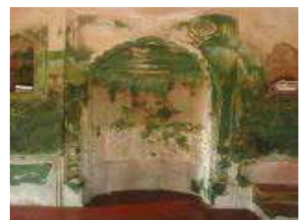
The inner side and outer side of the mosque were infected with salinity, algae and fungi.
