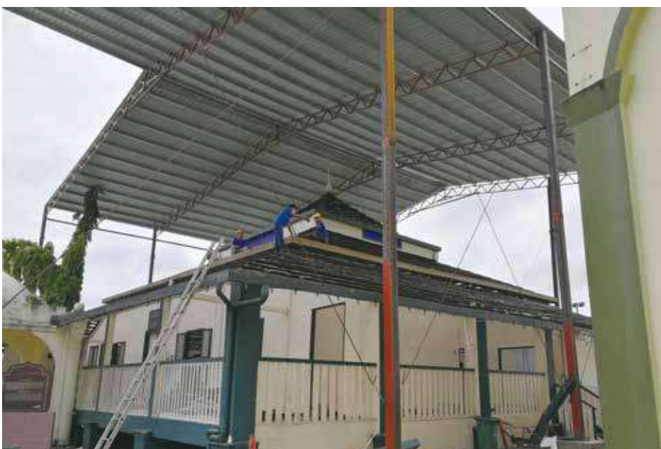
The scaffold roof was the temporary roof system installed at Al Qadim Mosque, supported by steel columns that were secured by bolts and nuts to concrete bases on the ground. The steel columns were also stabilized with cable tie bracing.
