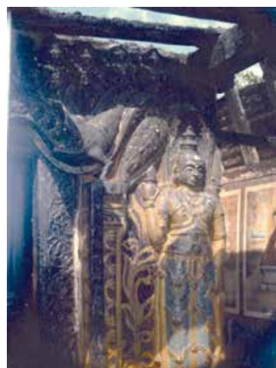
Figure 10. Damage to murals, paintings and statues
