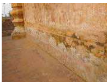
The inner side and outer side of the mosque were infected with salinity, algae and fungi.
