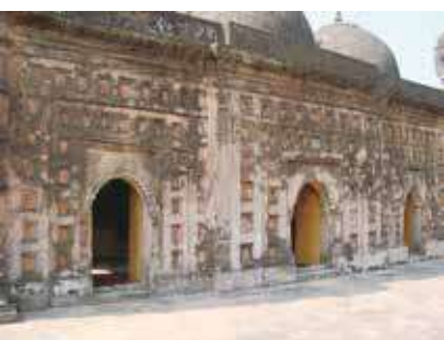
The inner side and outer side of the mosque were infected with salinity, algae and fungi.
