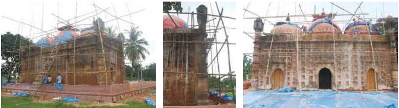
During conservation of Nayabad Mosque
