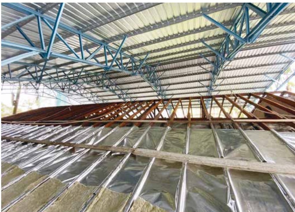
View of the temporary roof system at the Curator's House before the installation of new belian (ironwood) roof shingles
