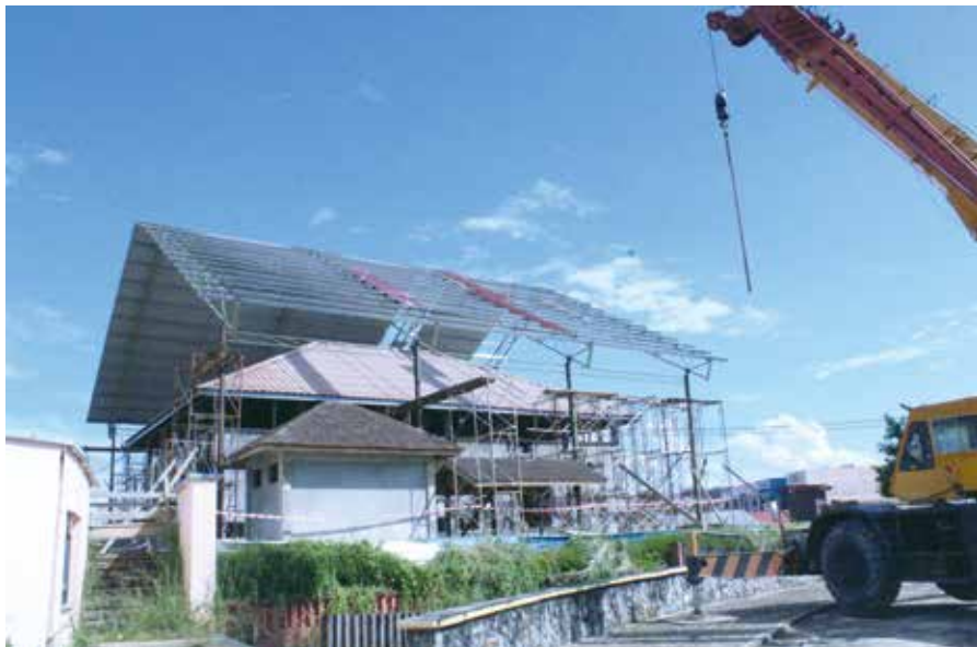
Due to site constraints, a mobile crane was used in the installation of the temporary roof system at Fort Emma.
