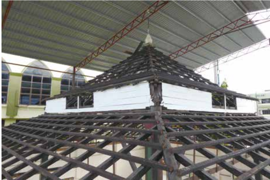
A temporary roof 16 metres high was erected to protect Al Qadim Mosque when the new roofing material was installed to replace the old roof.
