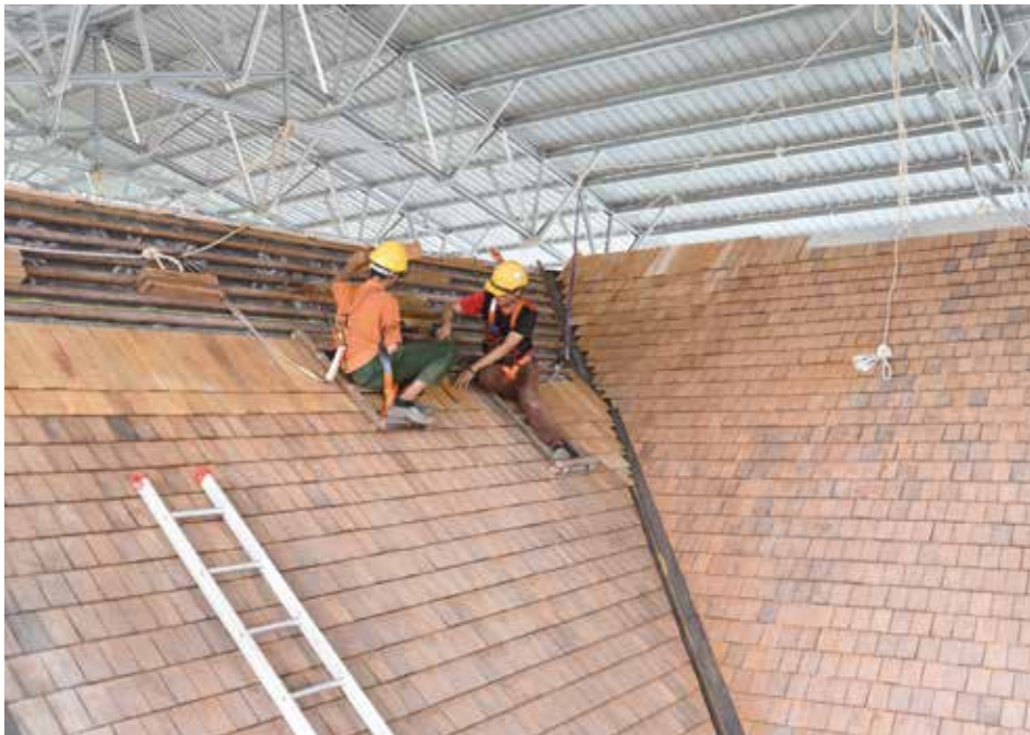
Roofers conveniently laid belian (ironwood) roof shingles under the temporary roof at the Old Sarawak Museum.
