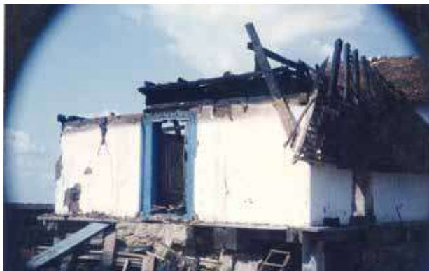
Figure 4. After fire destruction
