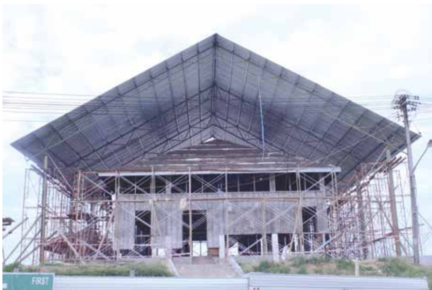
A frontal view showing scaffold roof system that covered Fort Emma, giving full protection to the fort from adverse weather conditions during the installation of belian (ironwood) roof shingles
