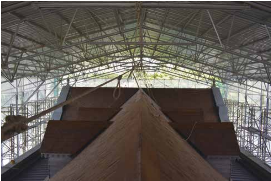
At a height of 14.6 metres, the temporary roof at the Old Sarawak Museum provided a conducive and comfortable work environment.
