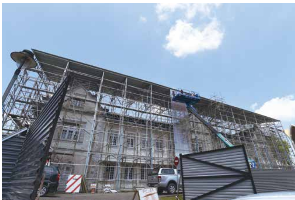
Installation of the temporary roof system at the Old Sarawak Museum
