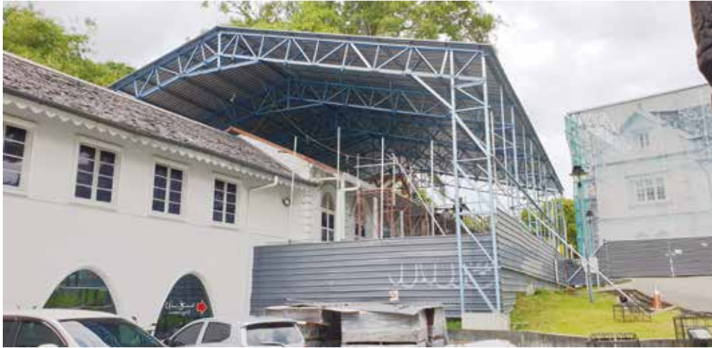
The temporary roof system at the Curator's House provided a high degree of versatility, protection, and encapsulation. The Old Sarawak Museum is located on the far right.
