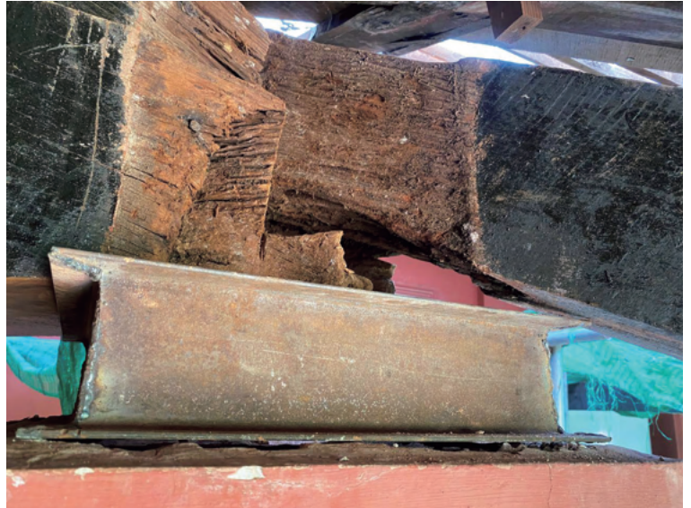
Figure 5(a,b): Dismantle the bricks of the column to remove rot of the timber and reinforce at the junction of components
