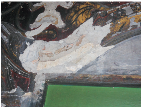
Fig.17. Rendering plaster had broken off from the Dragon Arch ( Makara Torana ) - (wall no. A2)
