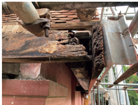
Figure 1-3: Damage to the timber structure inside and outside the roof
