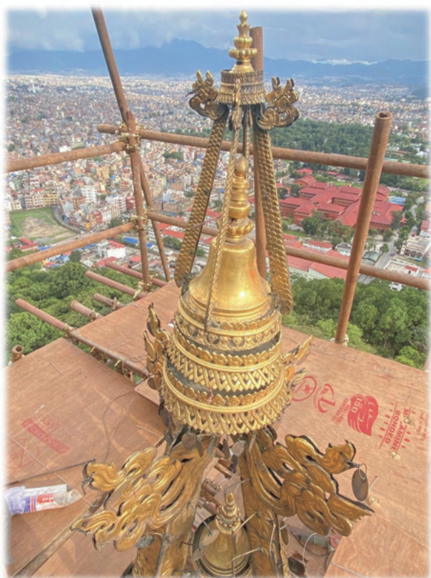
Reinstallation of repaired gajur. Source: FSMC
