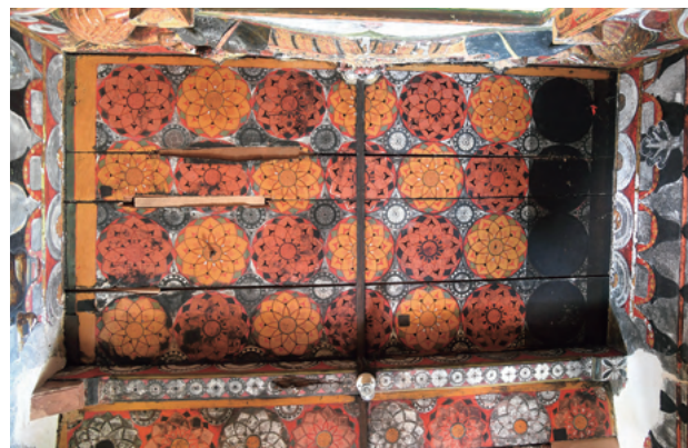
Fig.24. After chemical cleaning (wooden ceiling)
