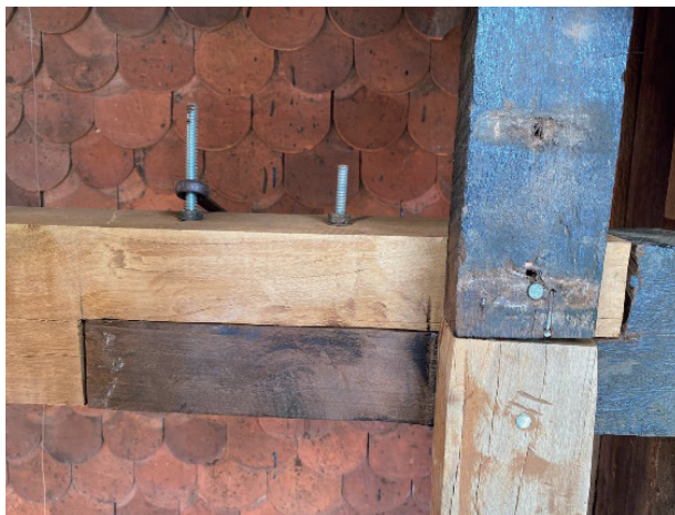
Figure 6(a,b,c): Replacing parts and linking between new and old timber structure
