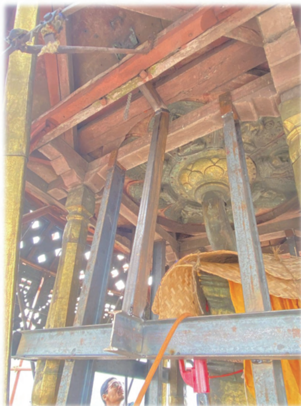
Supports for the other parts of the stupa Source: FSMC
