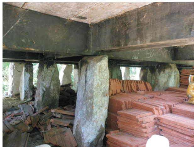
Fig.20. Before cleaning - stone pillars and wooden beams - under the base of the image house
