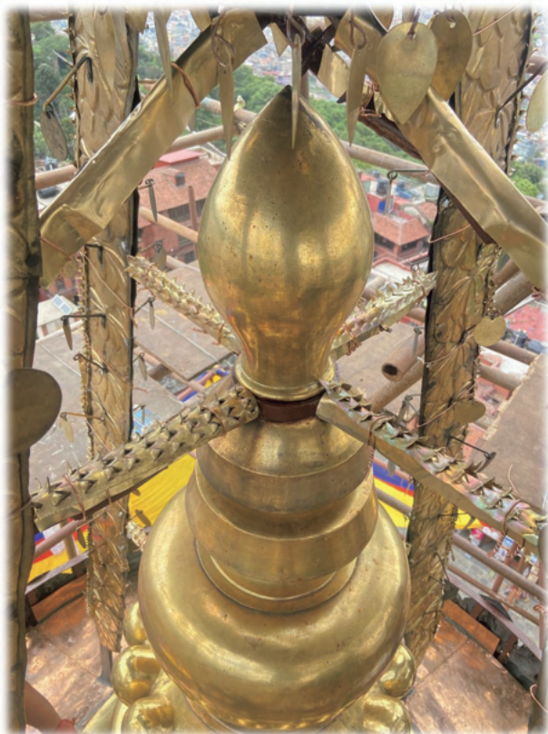
Supports for the gajur during reinstallation Source: FSMC
