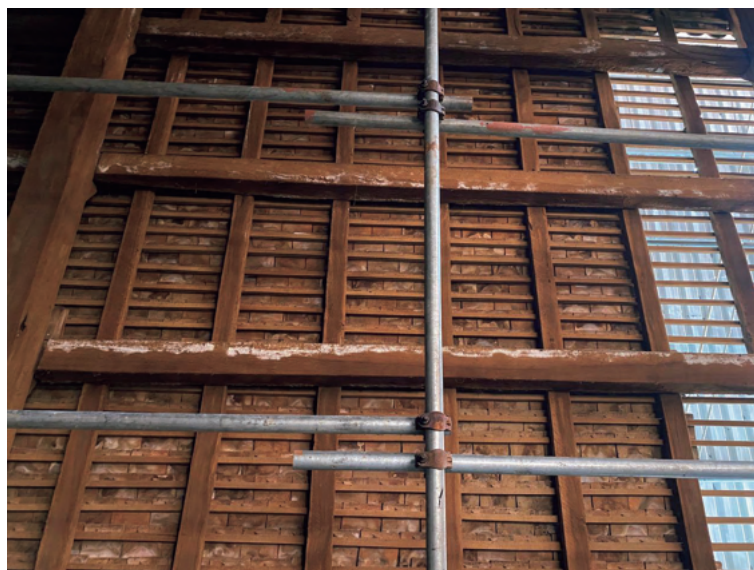
Figure 4(a,b): Mold on the timber of the roof
