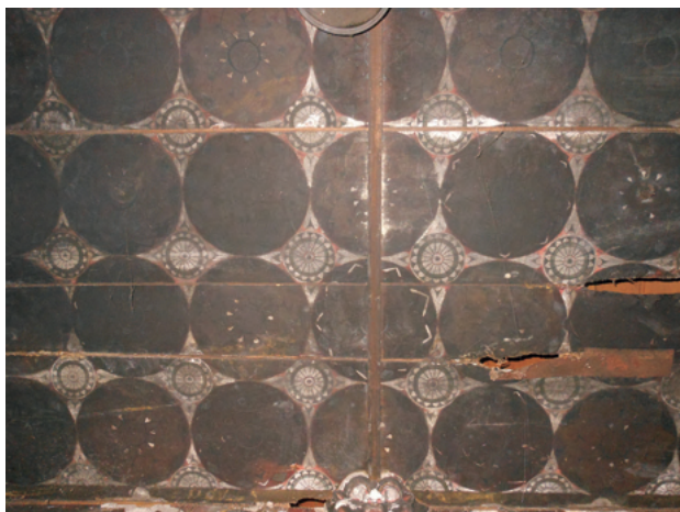
Fig.15. Wooden ceiling before chemical cleaning
