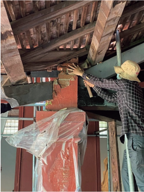
Figure 5(a,b): Dismantle the bricks of the column to remove rot of the timber and reinforce at the junction of components
