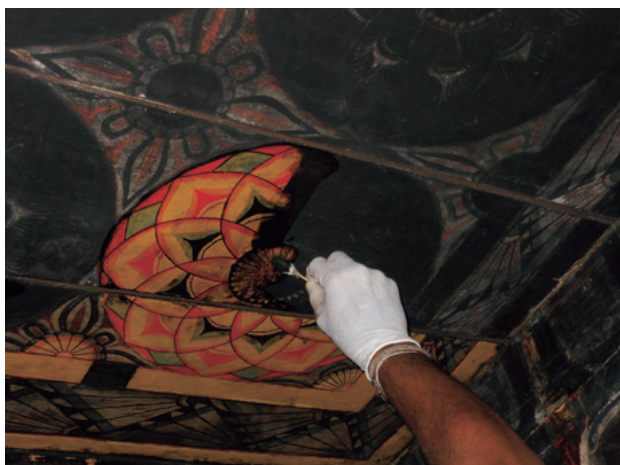
Fig.23. Chemical cleaning for removing soot. (Wooden ceiling no. 4)
