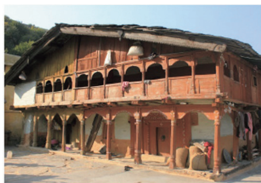
Traditional timber dwellings can still be found in the rural settlements along the Yamura Valley. The chief building materials comprise of river stone, slate stone, teak/deodar wood and adobe.
