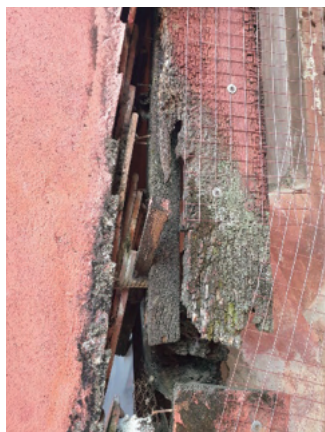
Figure 1-3: Damage to the timber structure inside and outside the roof
