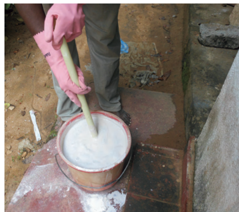
Fig.22. Preparation of paint receiving plaster
