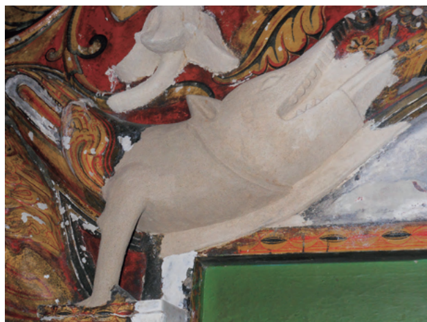
Fig.26. During consolidation of the Dragon Arch ( Makara Torana ) by using lime plaster
