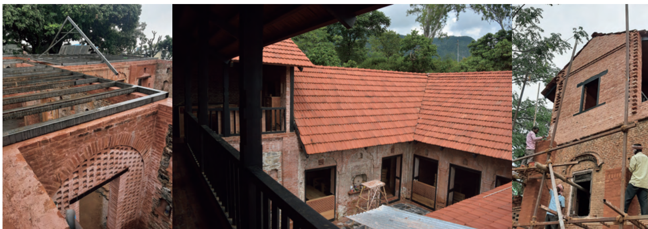
Fig. 8 a, b & c. Images of the structure while roofing and buttressing works were in progress.
