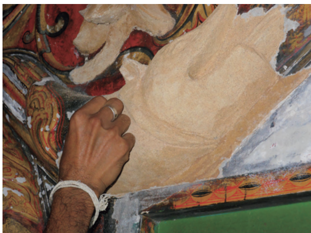
Fig.25. During consolidation of the Dragon Arch ( Makara Torana ) by using clay plaster
