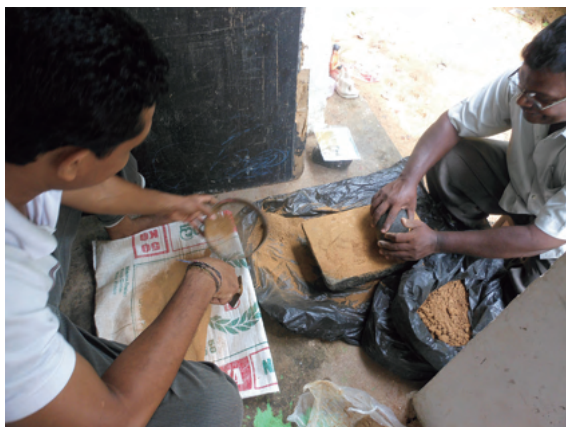
Fig.21. Preparation of clay plaster
