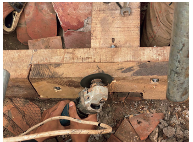
Figure 6(a,b,c): Replacing parts and linking between new and old timber structure
