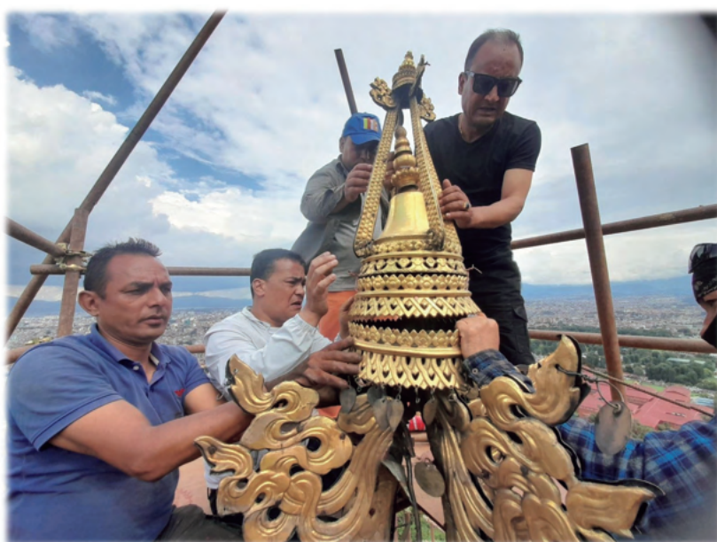
Reinstallation of gajur by craftsmen. Source: FSMC
