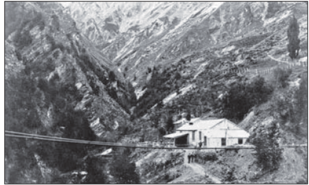
Figure 6. New Main Shaft ca. 1900 (?). Location of the Anglo-American Brush Corporation Electric Motor which powered the winding gear (Source: Petchey 2006:25 & Hocken Library, Dunedin ).
