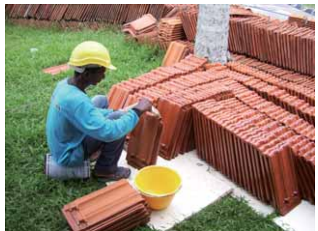
The existing Marseilles tiles were brought down to the ground where each tile was inspected, cleaned and salvaged. The cleaning process involved both dry and wet cleaning techniques
