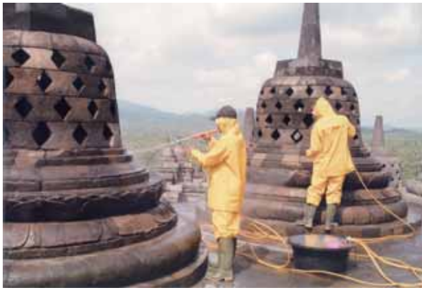
Photo 8. Wet cleaning on the main stupa
