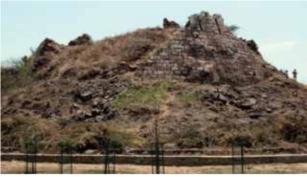
Bastion, before conservation
