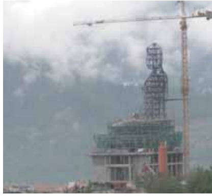
Steel frame structures before fixing panels
