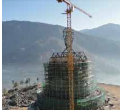
Steel frame structures before fixing panels
