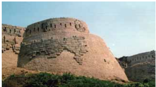
Bastion, after conservation
