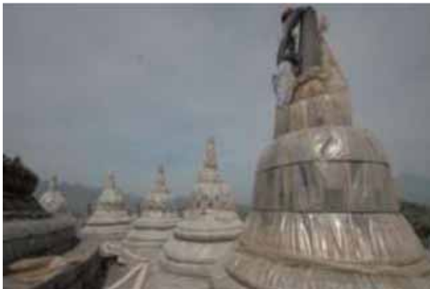
Photo 10. The cleaned stupa covered with plastic
