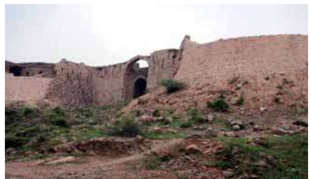
Gate, after conservation
