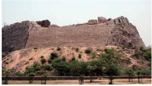
Bastion, after conservation
