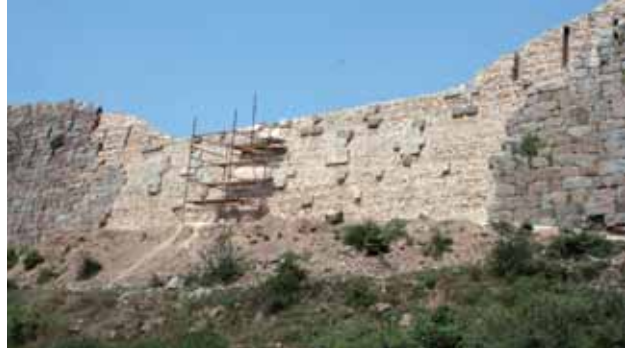
Bastion, after conservation
