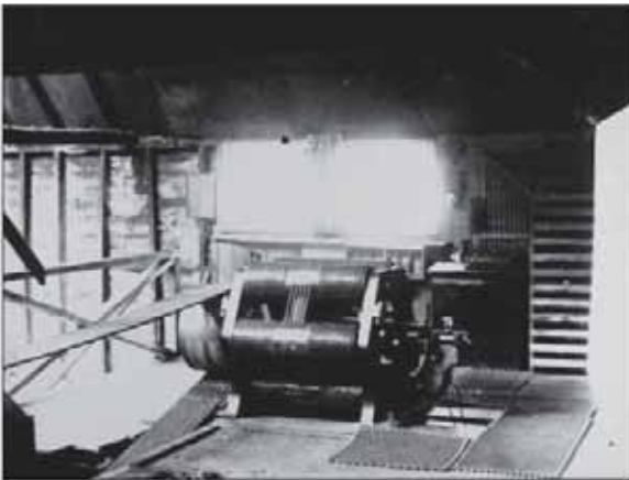
Figure 20. The Anglo-American Brush Corporation Electric Motor at Bullendale. Top: as one of the electric motors looked in 1886 (Source: Petchey 2006:15 & Lakes District Museum, Arrowtown); Bottom: the dismantled motor at the New Main Shaft. The parts are in good condition. Note the native Beech trees which have grown through gaps in the discarded motor parts (Photo: Matthew Schmidt).
