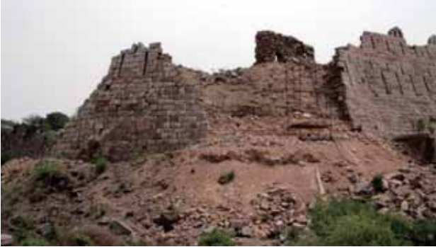
Bastion, before conservation
