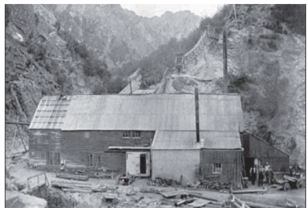
Figure 4. Phoenix (Achilles) Battery ca. 1887 when its stampers were powered by electricity (Source: Petchey 2006:32 & Hocken Library, Dunedin). Compare with Figure 11. The rock crusher is the top of the photograph and the remains of the battery house in the foreground.
