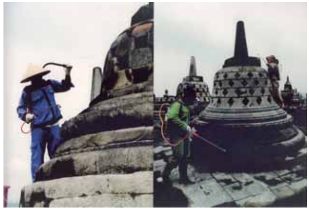
Photo 9. Wet cleaning on the main stupa
