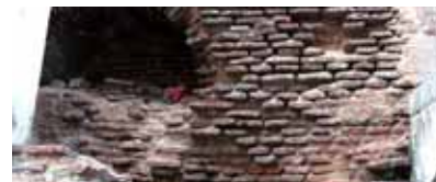
Fig. 21: Sanding of mortar in brick masonry
