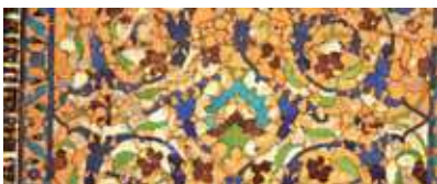
Fig. 18: Exfoliation of glaze from the terracotta body of the tile is the most common damage type on the glazed tiles.
