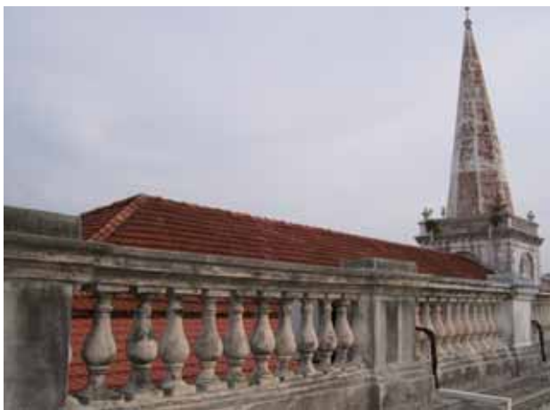
The condition of the pitched roof, balustrades, bell tower and spire before restoration
