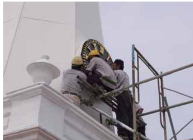
A working replica of 1.27-meter clock was fixed onto the north side of the spire
