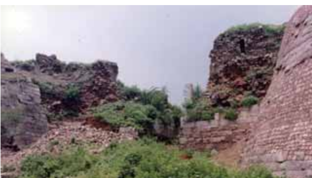
Entrance, in damaged condition
