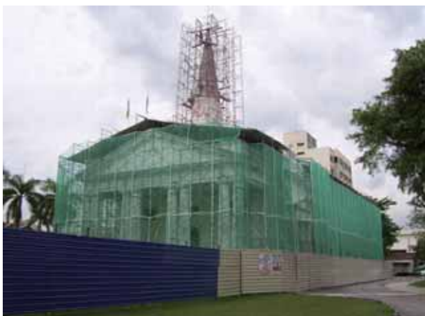
Throughout the restoration work, temporary roofing was installed above the existing pitched roof to ensure that the roof structures were protected from severe rainfalls
