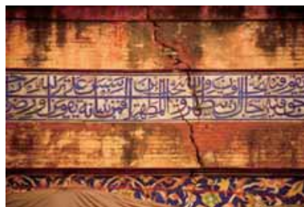
Fig.14: Major crack in the wall above the northernmost archway of the main prayer chamber facing
