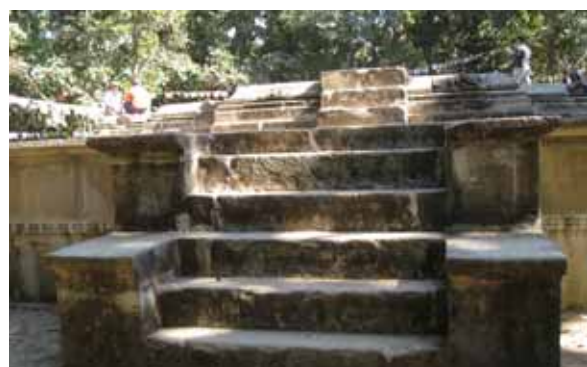
Firing Bays in the Fort, Rasuwagadhi (A Medieval Period Fort)
