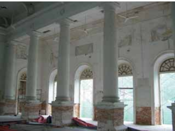
Crumbled lime plaster had to be removed from the lower part of the walls and at the base of the columns which were infected with salt attack and rising damp
