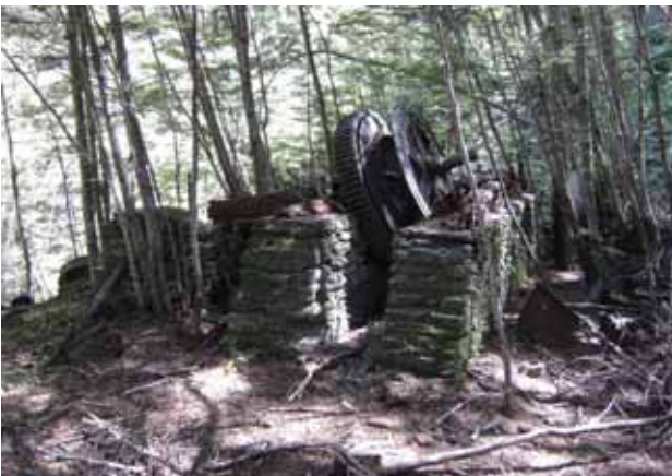
Figure 21. The winding gear structure at the New Main Shaft. Gearing has slipped off the rotten support timbers and onto the structural stonework causing the stonework to bow.
