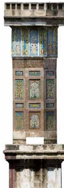
Fig. 7: The southern face of the southeastern minar shows the detail of kashikari and exposed brick work. Detailed investigations show the major damages to the kashikari towards the north side.
