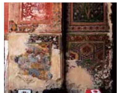
Fig.15: Rising damp in the main prayer chamber has damaged the fresco paint.
