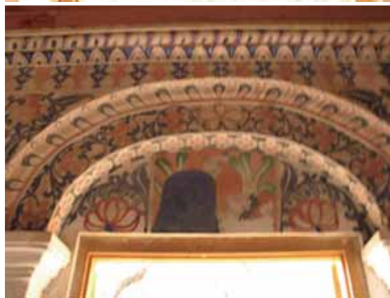
The painted arch at Gallengolla Vihara before and after restoration
