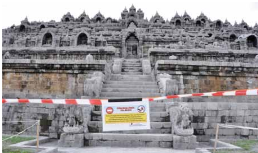
Photo 14. Installation of a prohibition sign to the temple building
