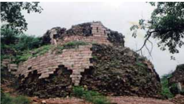
Bastion, before conservation
