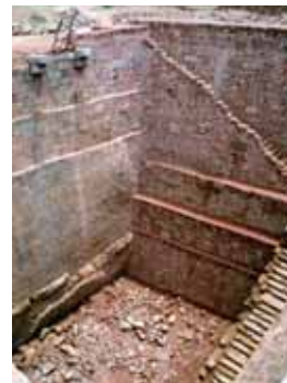
Stepped well, during conservation
