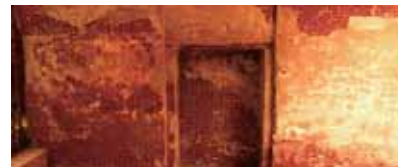
Fig. 17: Efflorescence on the rendered surface (tazzakari) of the wall in the southern section of calligrapher ' s bazaar.
