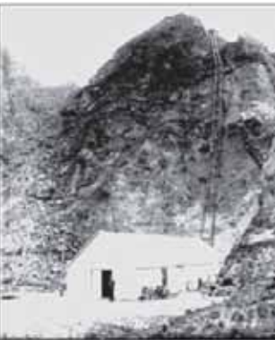
Figure 18. The hydroelectric power scheme at Dynamo Creek photographed in ca. 1900(?). The penstocks can be seen as well as the powerhouse building (Source: Petchey 2006:39 & Lakes District Museum, Arrowtown).
