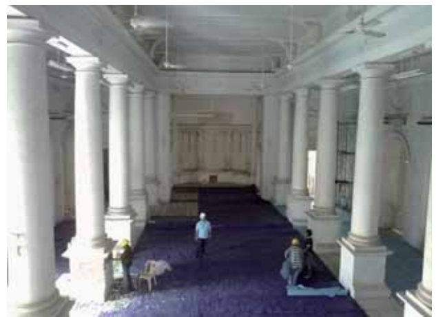
The interior view of the church showing the nave, aisles and altar with two rows of Roman Doric columns during restoration
