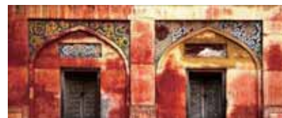
Fig. 19: Fading of surface render (tazzakari) on the northern façade of hujra walls in the courtyard.
