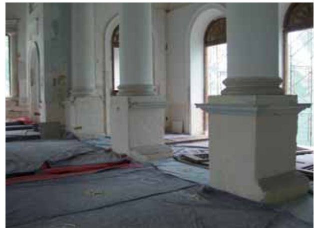
Salt attack was treated through the salt desalination process using a poultice technique called Cocoon before carrying out the injection of a chemical damp-proof course
