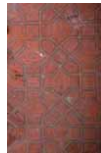
Fig.11: Brick floor pattern in the upper level of the courtyard
