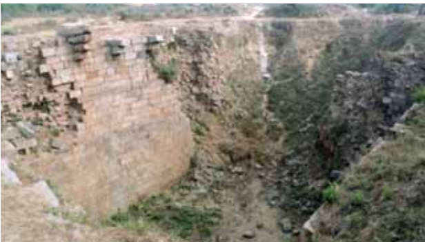
Stepped well (Baoli) in damaged condition
