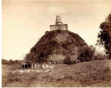
Jatavana stupa before conservation
