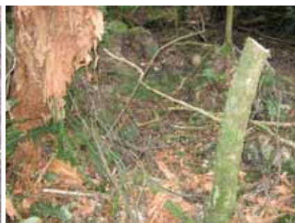
Figure 21. The stone structure which may have been a roofed hut, at the top of the lower pond. A large tree is growing out of the stonework (left in photograph) with saplings and ferns growing out of other areas (see also Figures 11 and 12) (photo: Matthew Schmidt).
