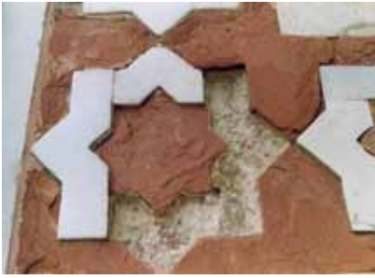
Moderate weathering of top surface of base stone and deadening of mortar: Restored Akbar's Tomb
