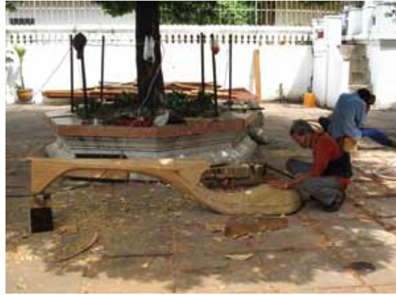
Figure13 : Engraving the new architectural ornament by traditional craftsmen
