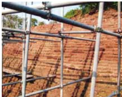
Sandagiriya brick work at 10 m level
