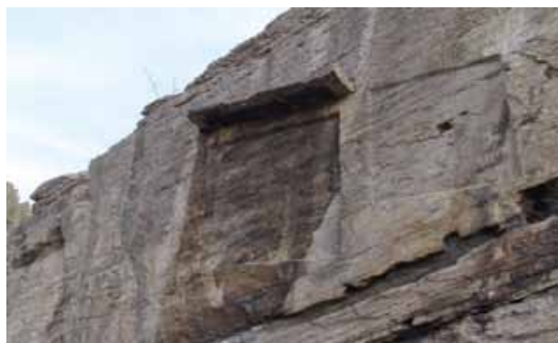
The stone leaking-proof shelf, remains of Tang dynasty
