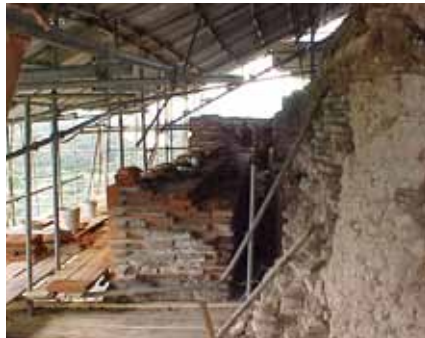
Ancient and new brick layers at the cube, Jatavana stupa
