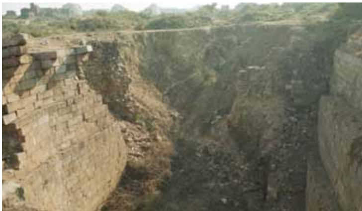
Baoli at Tughluqabad Fort in damaged condition
