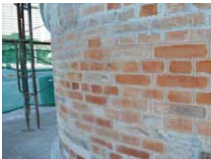
Close-up view of the newly fixed bricks on the wall (reddish in colour)
