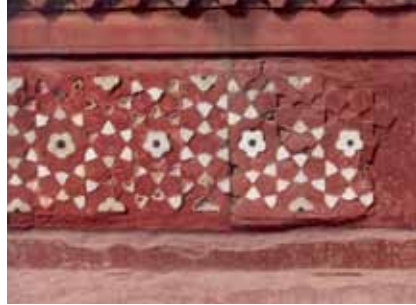
Weathered base and missing inlay pieces, during restoration base stone was replaced and grooved: Itimad-ud-Daula's Tomb
