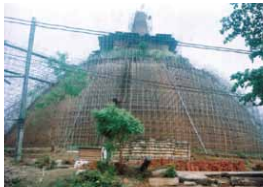
Abhayagiri during conservation (2)
