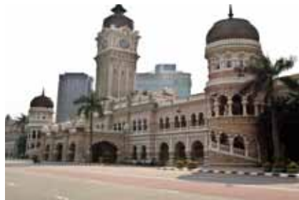
The building front façade with its immense 41.2 metre (135 feet) clock tower, central porch, three copper domes topped with a copper chhatra; and different forms of arches (key hole, ogee, pointed and horseshoe).
