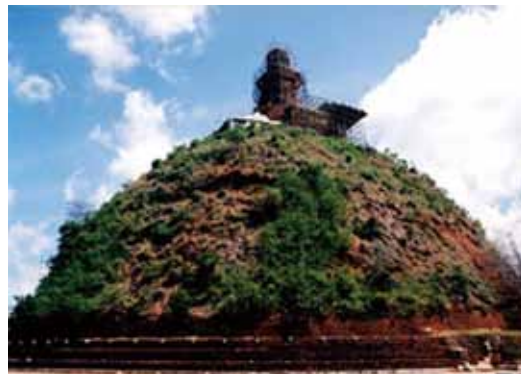
Abhayagiri during conservation (1)
