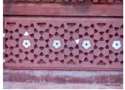
Weathered base and missing inlay pieces, during restoration base stone was replaced and grooved: Itimad-ud-Daula's Tomb
