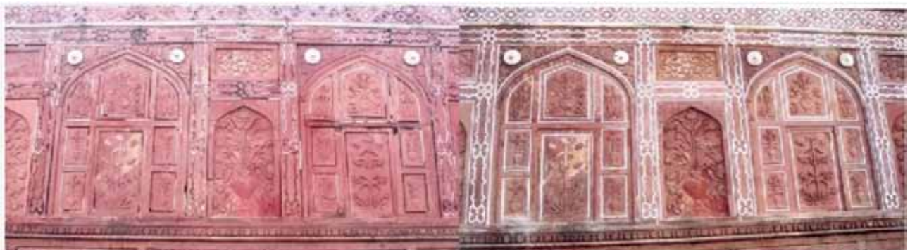
Restoration of missing inlay pieces: Riverside wall, Taj Mahal
