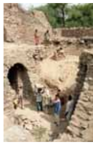
Baoli at Arab-ki-Sarai (during work)
