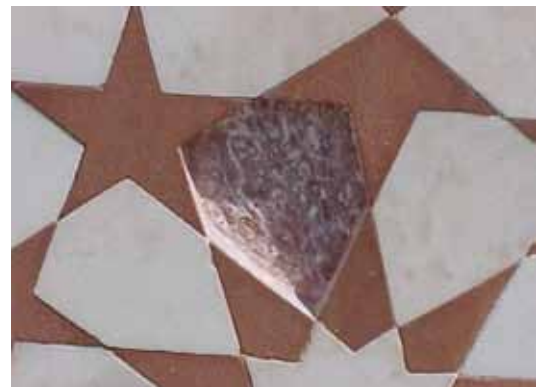
A missing inlay piece before restoration
