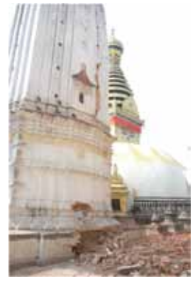
Northern damaged part of the temple
