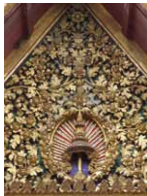
Figure 6 : Gable of Ubosot before restoration, decorated with gilded stucco and colour glass mosaic
