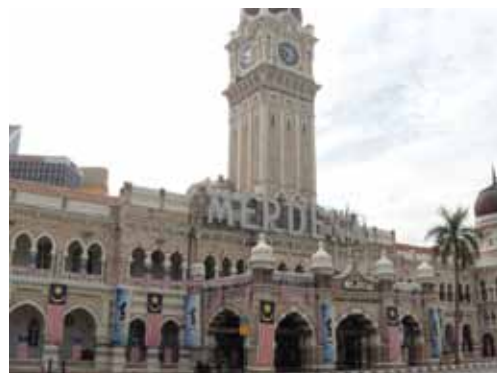
The front façade of the building before restoration
