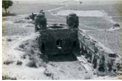
Baoli at Munirka, in dilapidated condition and filled with debris
