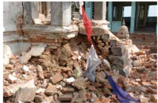
The foundation close to main entrance in southern part
