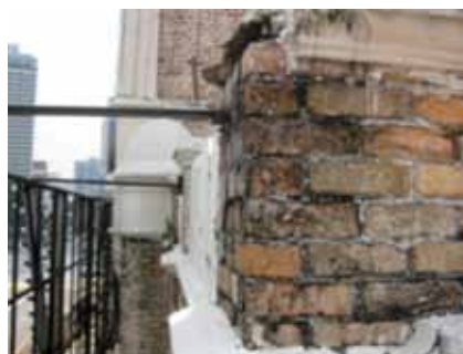
Surface damage on the brickworks
