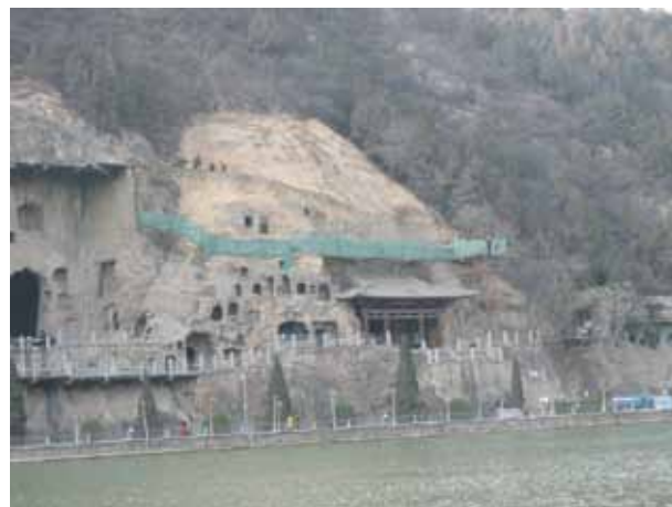
The water-leaking project of caves
