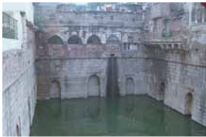
Baoli at Ghiaspur (Nizamuddin), before conservation
