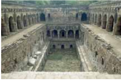
Rajon-ki-Bain ( Baoli ), in damaged condition and filled with debris
