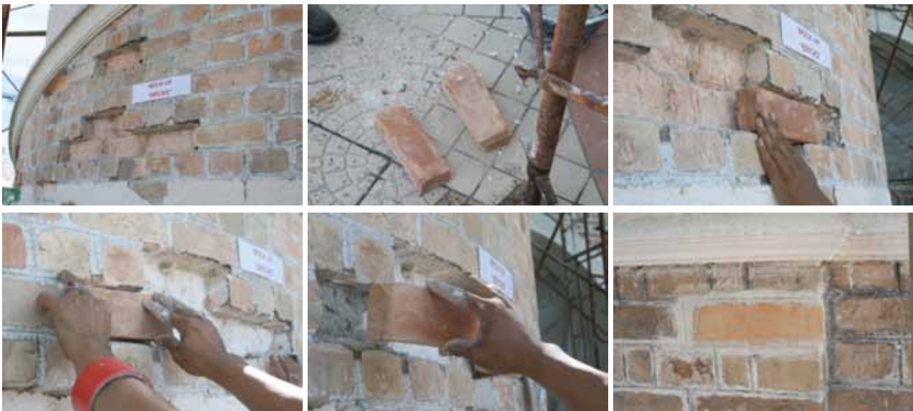
The sequence of brick replacement on the wall
