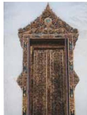
Figure 7 : Window of Ubosot before restoration; Gable of Ubosot before restoration, decorated with gilded stucco and colour glass mosaic; Wooden pane, decorated with gilded and colour glass mosaic
