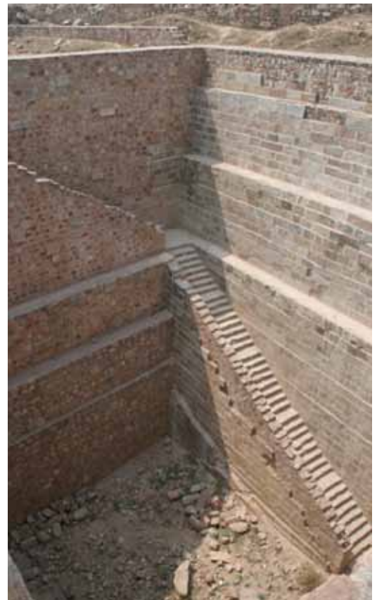
Baoli at Tughluqabad Fort, during conservation
