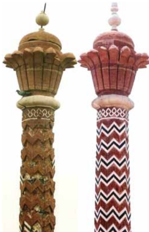
Weathered base and missing inlay pieces, during restoration base stone was replaced and grooved: Itimad-ud-Daula's Tomb
