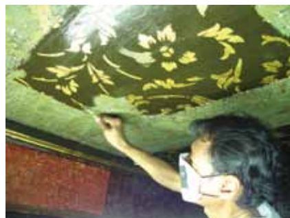
Figure10 : Tracing for the original decoration of ceiling, inside Ubosot, light green layer
