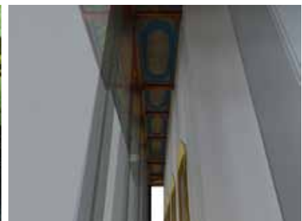
Figure 11 : The simulated perspective of the original decoration of corridor ceiling, gilded stencil pattern on blue colour
