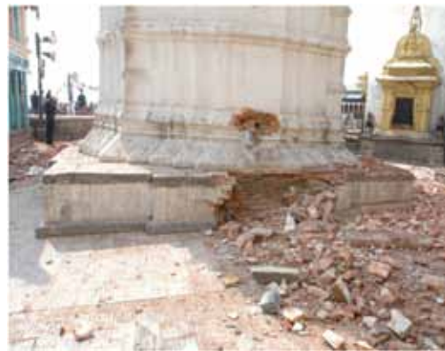
Damaged in the northern lower part of the temple
