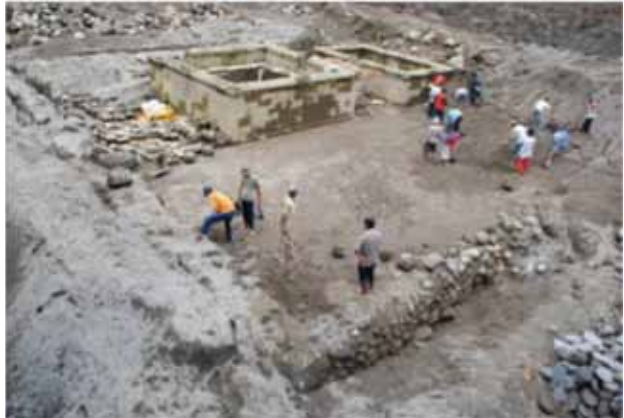
Figure 11. Excavation of yard after eruption of Mount Merapi
