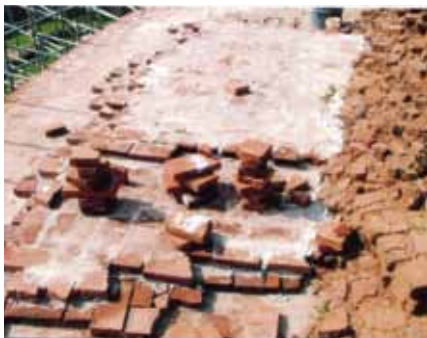
New bricks are being laid at Sandagiriya stupa.
