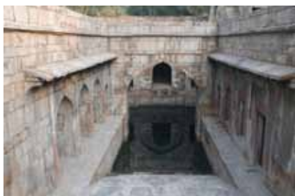
Baoli at Red Fort, after conservation
