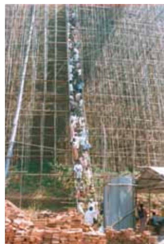
Material transport using manpower at Abhayagiri
