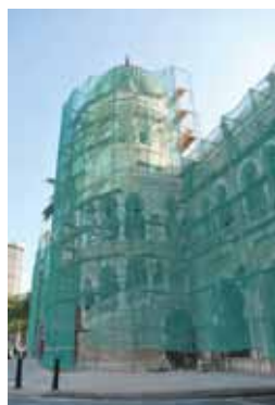
During the façade treatment, safety nettings were fixed on the scaffolding to provide protection from falling debris.
