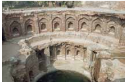
Baoli at Kotla Firoz Shah, after conservation
