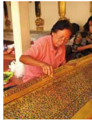
Figure15-16 : Restoring wooden panes by traditional craftsmen
