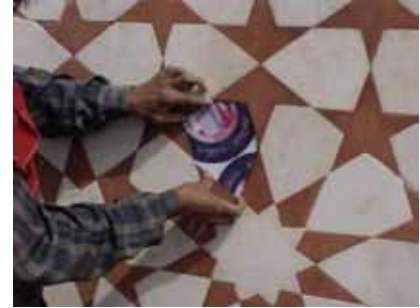
Checking the size of tin format with the missing one
