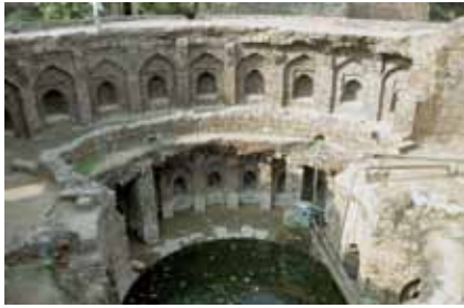
Baoli at Kotla Firoz Shah in damaged condition
