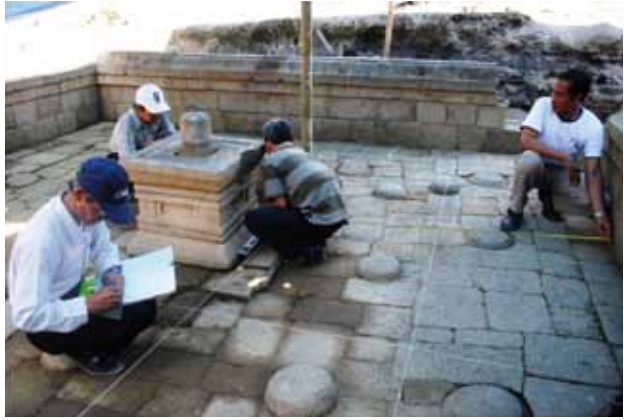
Figure 7. Measurement and drawing for technical study
