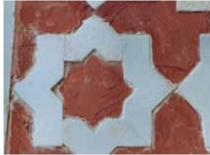
Moderate weathering of top surface of base stone and deadening of mortar: Restored Akbar's Tomb
