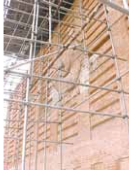
Restoration of mouldings, Jatavana stupa cube
