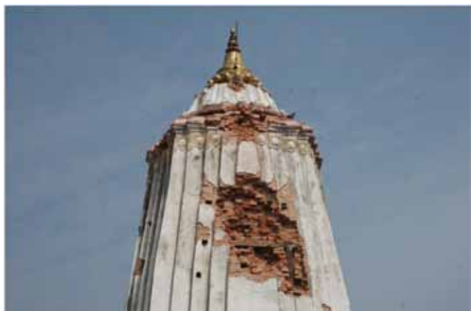
The southern upper part damaged by thunderbolt
