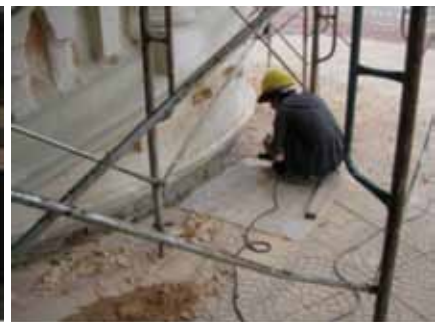
Chemical injection of damp-proof course
