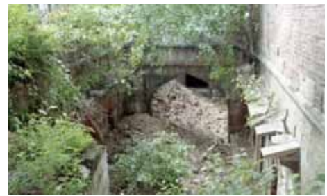
Baoli at Red Fort in dilapidated condition
