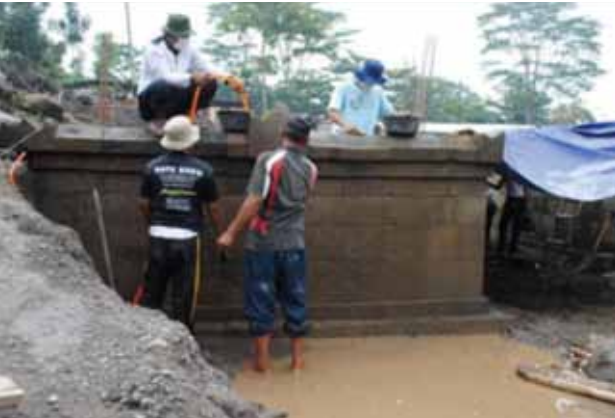
Figure 10. Cleaning of the temple wall
