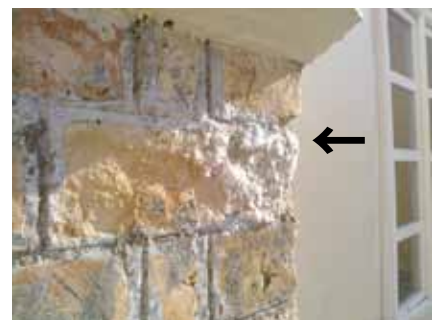
Salt contamination (primary efflorescence) on the brickworks
