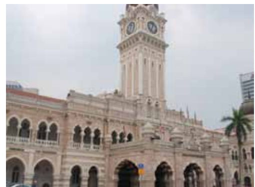
The new look of the building front façade after restoration. All electrical wirings, power cables, light bulbs, blocked letterings and signages on the building façades were carefully removed.
