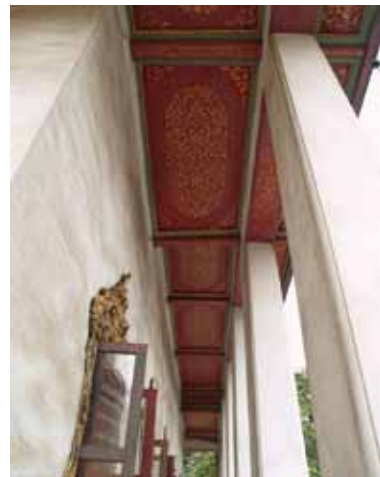
Figure8 : Corridor ceiling of Ubosot before restoration, decorated with gilded stencil pattern on red colour
