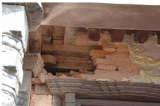
Damaged-above the main entrance gate of the temple
