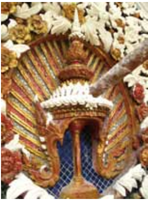
Figure14 : Restoring the stucco on the gable by using traditional lime
