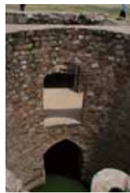
Baoli at Arab-ki-Sarai (during work)
