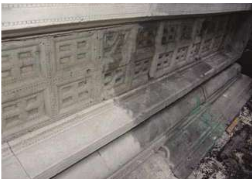
The coral stone of the mosque, showing the condition before and after pressure-water cleaning
