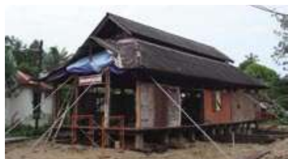
During restoration work, all new extensions were demolished including the front porch and toilet.
