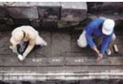
Marking stones before dismantling, June 2009
