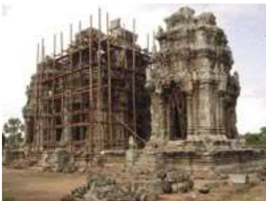
In progress of shoring up of the three principle towers
