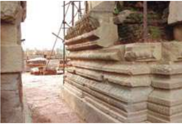
Stone base of Duong Long tower (after excavations)
