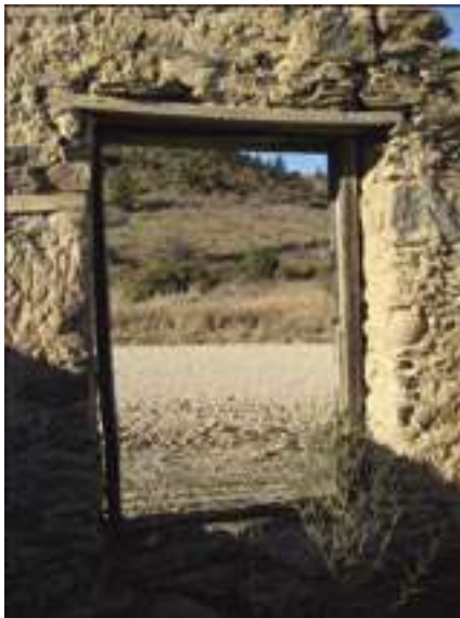
Figure 9. Window of bakery viewed from inside the structure looking out onto Oxford Street. In the 19th century, the schist stonework was set using a mud/lime mortar.
