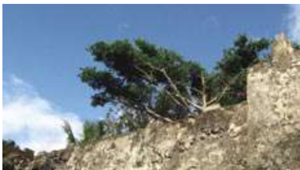
Vegetation growth in some parts of the Baluarte thick walls
