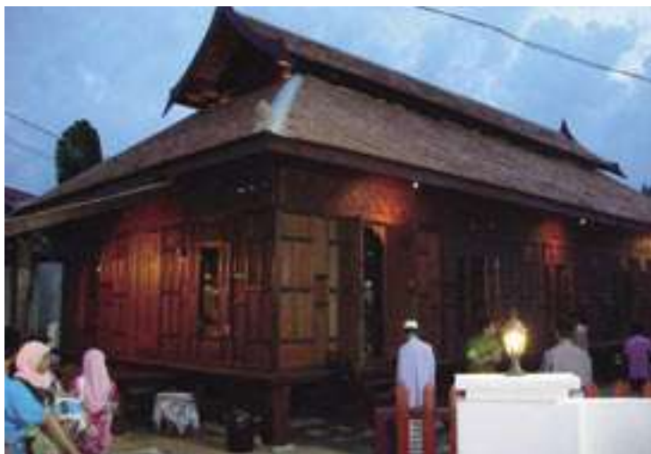
The Kedai Mulong Old Mosque after restoration featuring its new roof styles based on the original design
