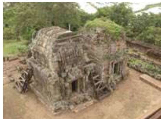
Other towers after shoring up
