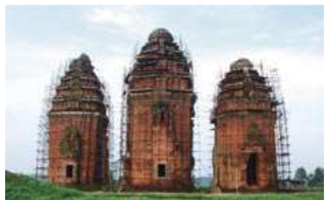
Duong Long tower (after excavations)
