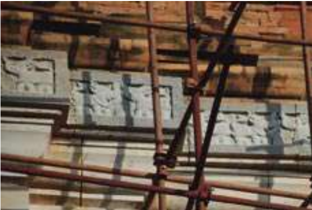
Restoration of the relief on the roof of Duong Long tower
