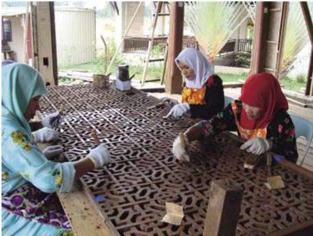
Local villagers were invited to be involved in the restoration of timber lattice panels. Such community involvement creates greater awareness on preservation and conservation of heritage properties.
