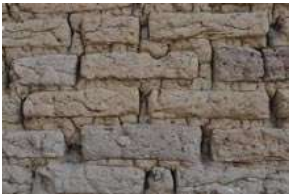
Picture 1, 2: Clay used for private house construction, Duong Lam village - Hanoi
