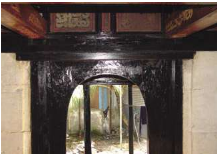
The ceiling of the mosque: conservation treatment was done on half, and the other half shows the state before conservation.
