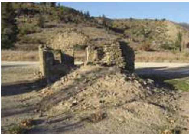
Figure 7. Bendigo Bakery viewed from the back of the structure looking towards Oxford Street and the goldfield in the distance. The collapsed structure at the back of the bakery is believed to be where the oven was located. This mound is also made up of debris bulldozed onto the site over the years. The mound will be investigated during the stabilisation works.
