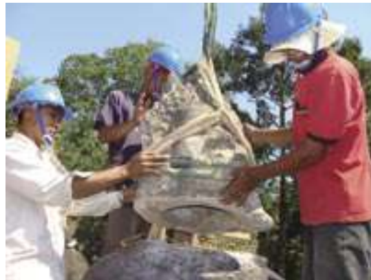
The cement head of Demon was removed
