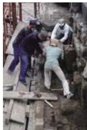
Dismantling filler stones, June 2009
