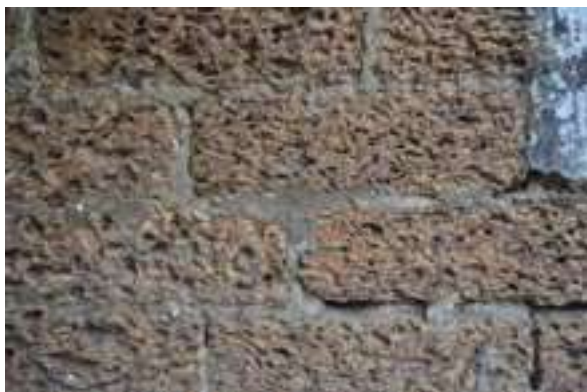
Picture 3: Laterite used for private house construction Duong Lam village - Hanoi
