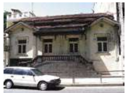
Typical Street House of British Period — House along Trincomalee Street, Kandy
