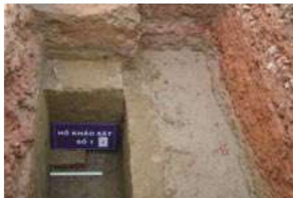
Picture 5, 6: The consolidation of foundation by laterite, clay, sand, lime, and brickbat Can Chanh Palace – Imperial City – Hue Citadel
