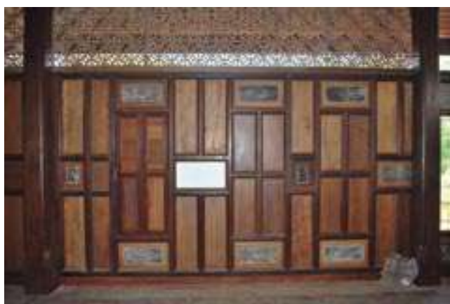
Timber walls, lattice panels and columns after restoration. The original black and gold-colour panels on the wall were revealed after scraping off the existing paint.
