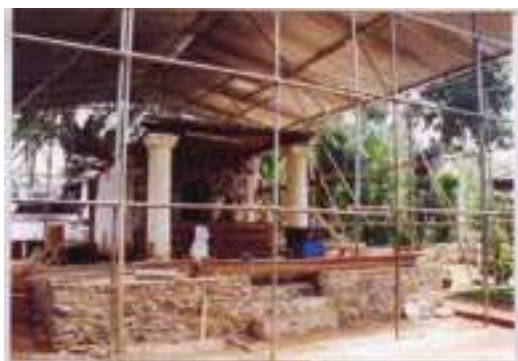
Temple building being conserved by the Central Cultural Fund – Katudeniya Vihara
