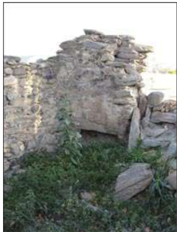
Figure 8. Collapsing chimney on the back wall of the bakery viewed from the interior. On the right of the photograph was where the entrance to the oven used to be.
