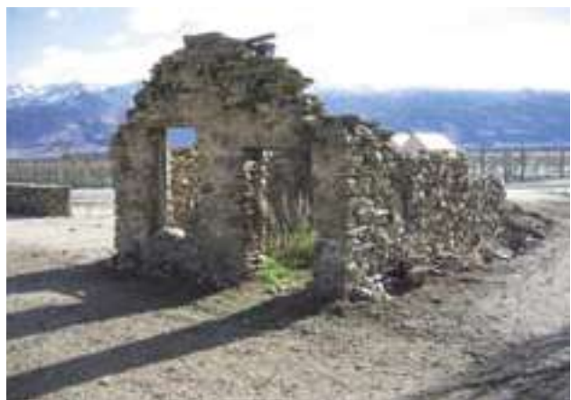
Figure 5. Bendigo Bakery ruins. The vineyards in the background lie over the old township. The footprint of the building is the new DoC Historic Reserve, the surrounding land being in private ownership (photograph: Matthew Schmidt).
