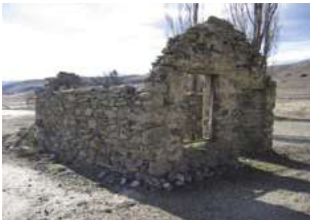
Figure 6. Bendigo Bakery ruins. More vineyards lie behind the building (photograph: Matthew Schmidt).
