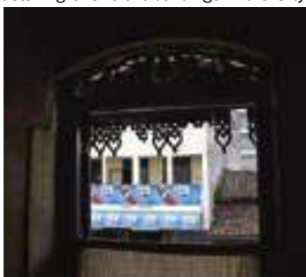
Deteriorated timber window and Valance Board
