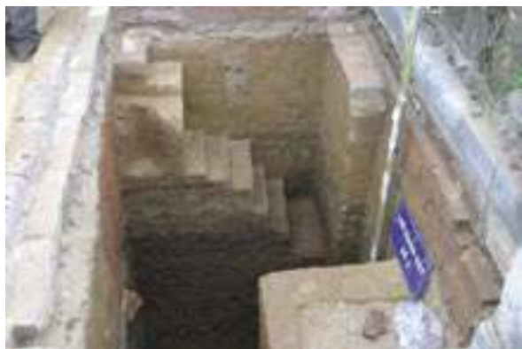
Picture 5, 6: The consolidation of foundation by laterite, clay, sand, lime, and brickbat Can Chanh Palace – Imperial City – Hue Citadel
