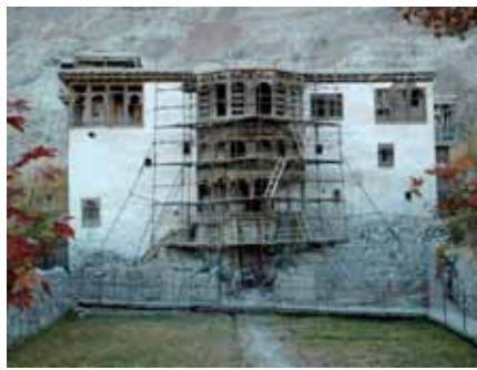
Fig. 2. North view of Khaplu Palace with main entrance wooden loggia under restoration
