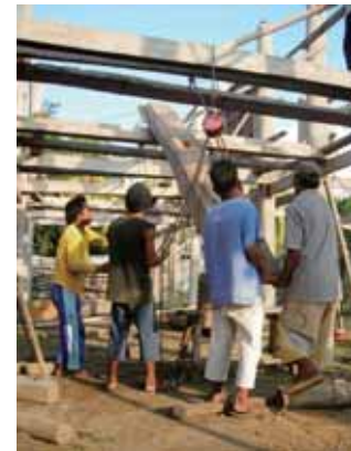
Moving of the main beam by a pulley, 2008
