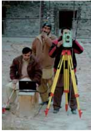
Fig. 11. Lifting and pulling back the loggia to a stable state is being closely monitored with total station
