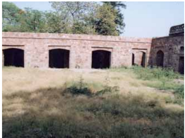
Damaged cells, Arab Sarai (after conservation)
