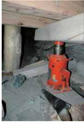
Fig. 12. Lifting of loggia to a stable state with the help of hydraulic jacks
