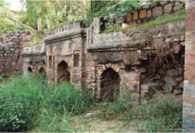
Mosque, Arab Sarai (before conservation)
