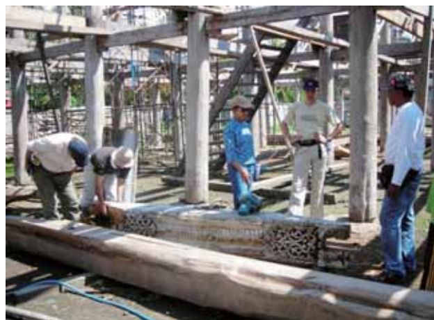
Inspection of the main beam before reinstalling, 2008
