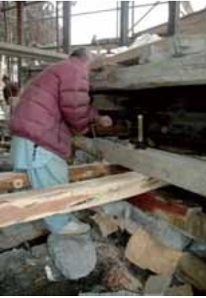
Fig. 10. Traditional construction techniques are being implemented during the restoration of loggia
