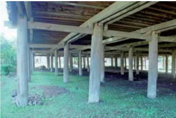
The poles of the building leaned to westward.
