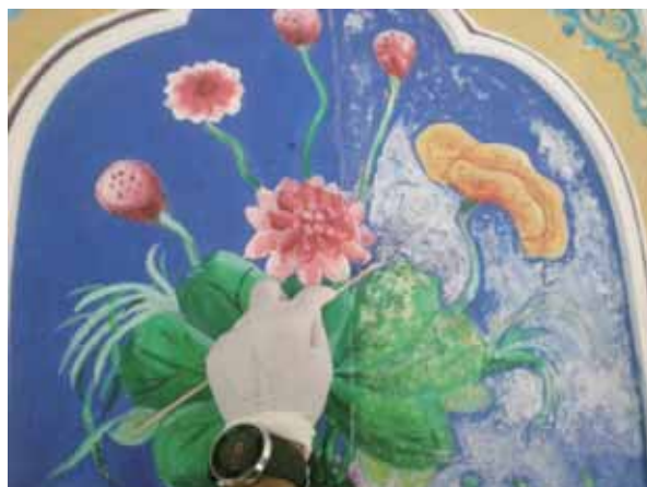
The wet cleaning technique involved the application of cotton tips and chemical solutions to remove the new layers of paints.
