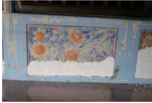
Paper pulp technique was applied to areas which had high level of moisture content.
