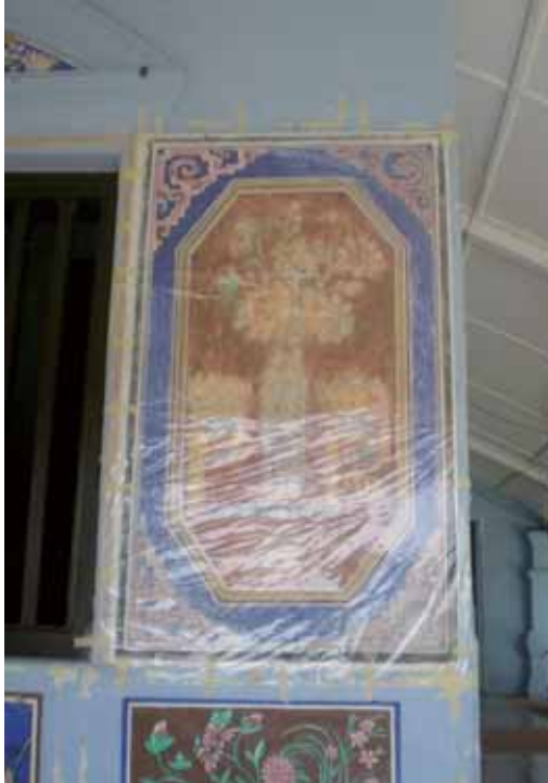
Plastic sheets were temporarily used to protect the wall murals from dust and rain
