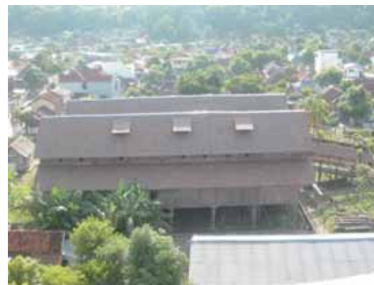
Restoration work viewed from above, 2010
