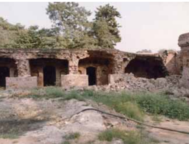
Damaged cells, Arab Sarai (before conservation)
