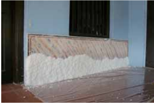
Paper pulp technique was applied to areas which had high level of moisture content.
