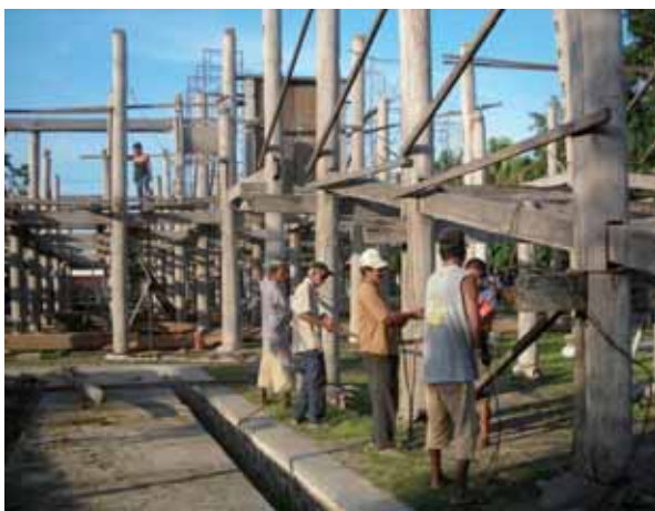
Enforcement of the main poles, 2008
