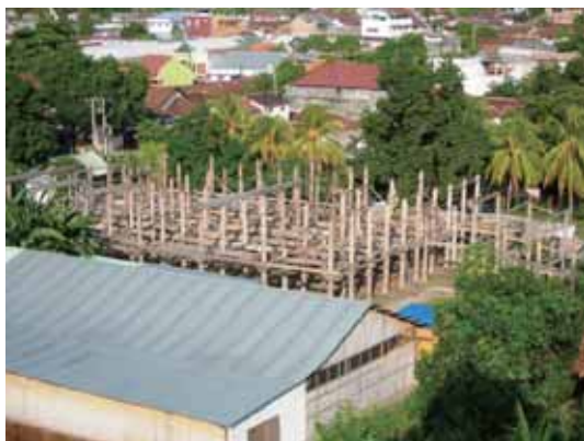
Restoration work viewed from above, 2008
