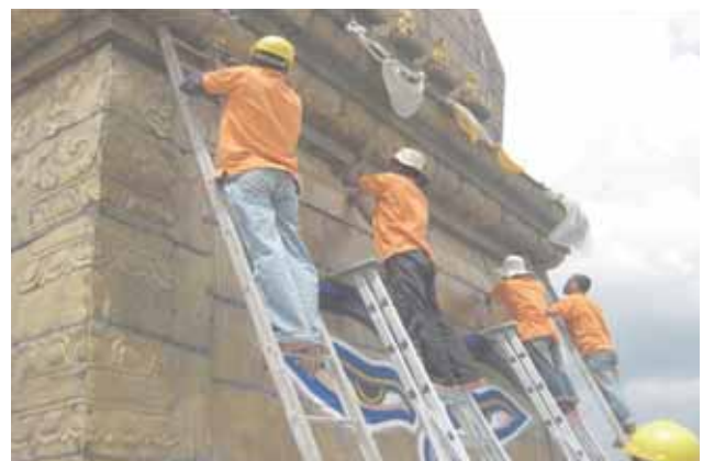
Removing copper sheets for gold gilding
