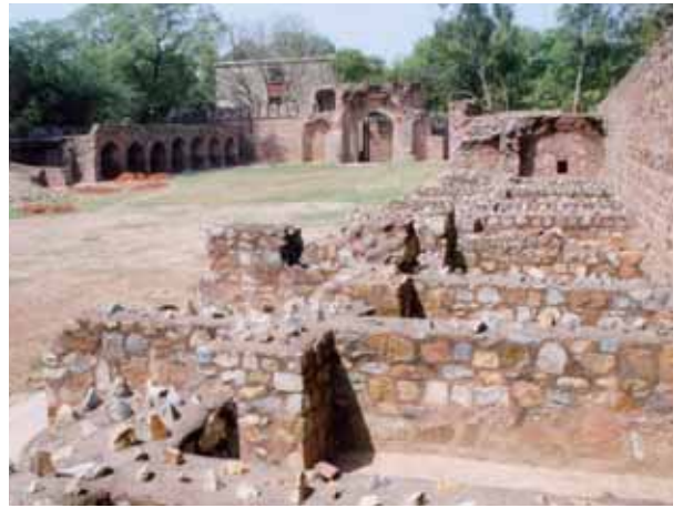
Damaged cells at Arab Sarai (a general view)
