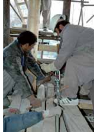
Fig. 13. Turning buckles are being used to pull back the tilted loggia
