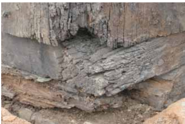
The deteriorated wooden parts of hermika
