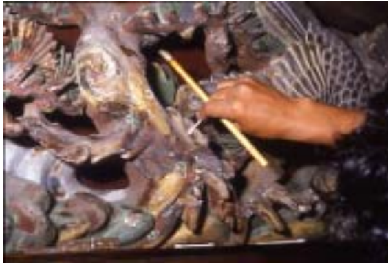
Fig.6 Working for preventing exfoliation
