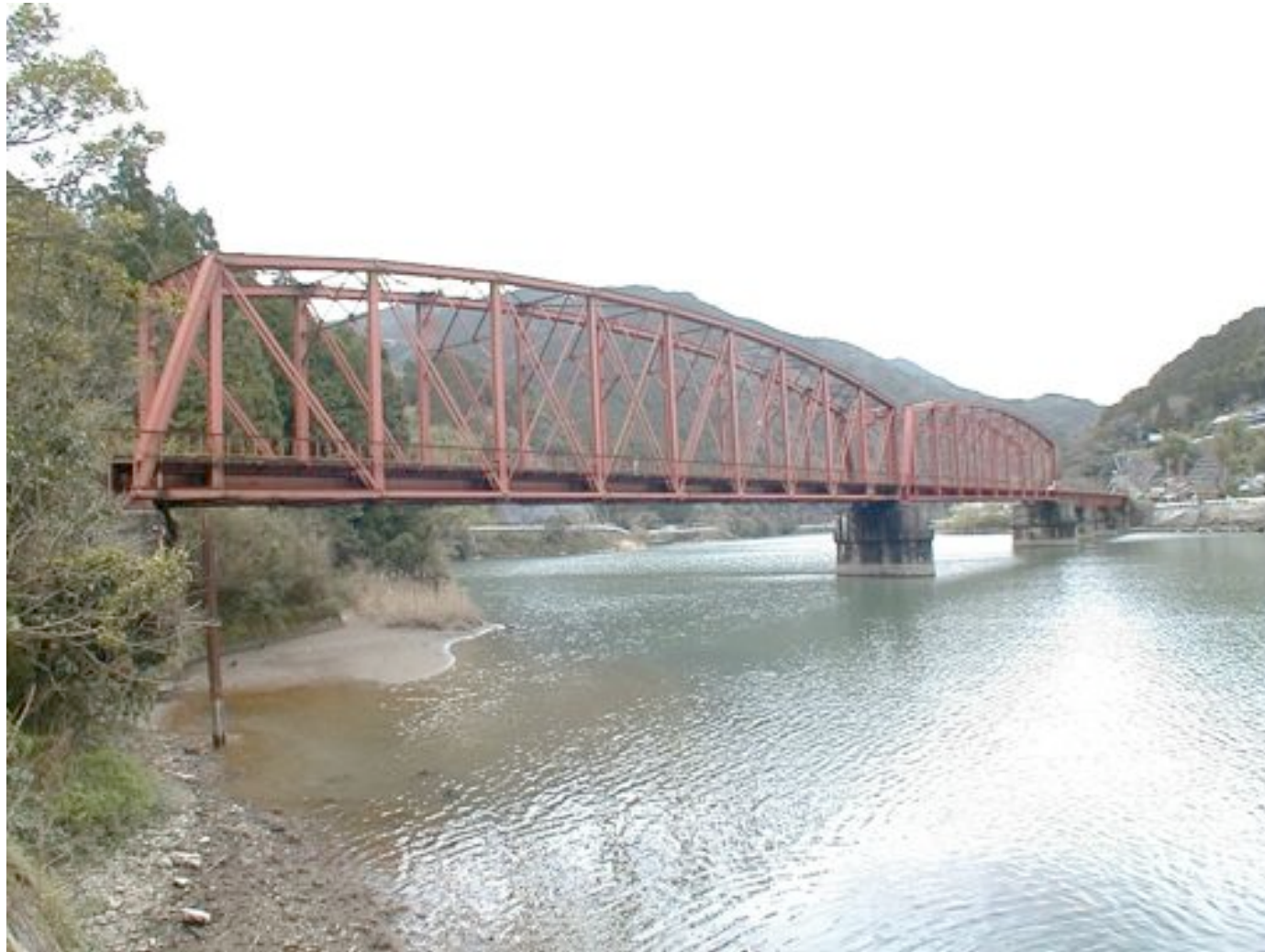
A bridge of Hisatsu Railway Line (Kumamoto, Japan)
