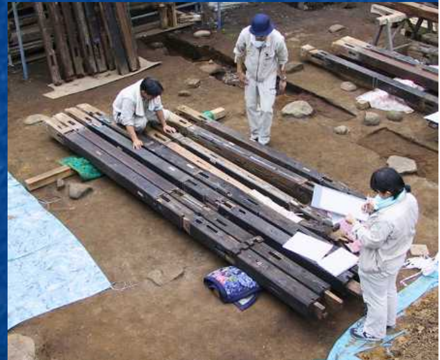
Training program for chief engineers Restoration survey at a repair site for a private house
