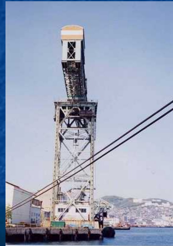
Hammerhead crane at Mitsubishi Heavy Industries Inc. Nagasaki Shipyard
