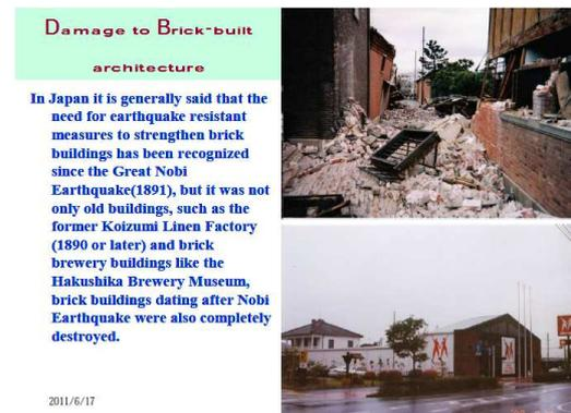
Fig. 22 Damage to Brick-built buildings
