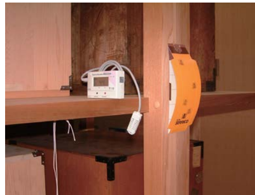
Temperature/humidity monitor (left) and pest detector (right)
