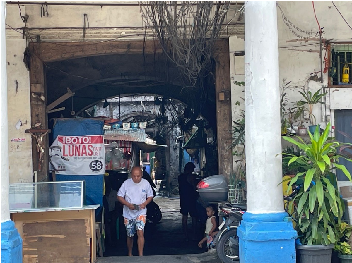
The technical documentation team cannot access the site safely because of threats from tenants.
