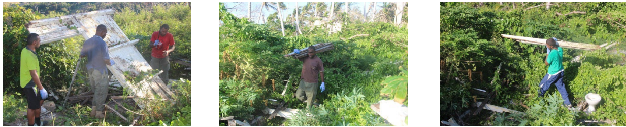
Dismantling the building structures. Images credit: Fiji Museum
