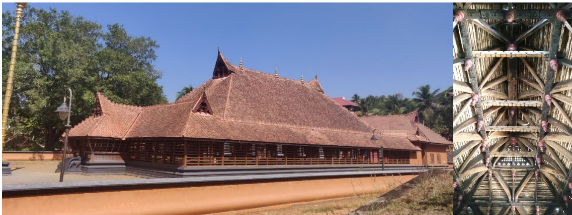
Figure 3. Koothambalams, traditional performance theatres of Kerala, and their timber roof joinery details
