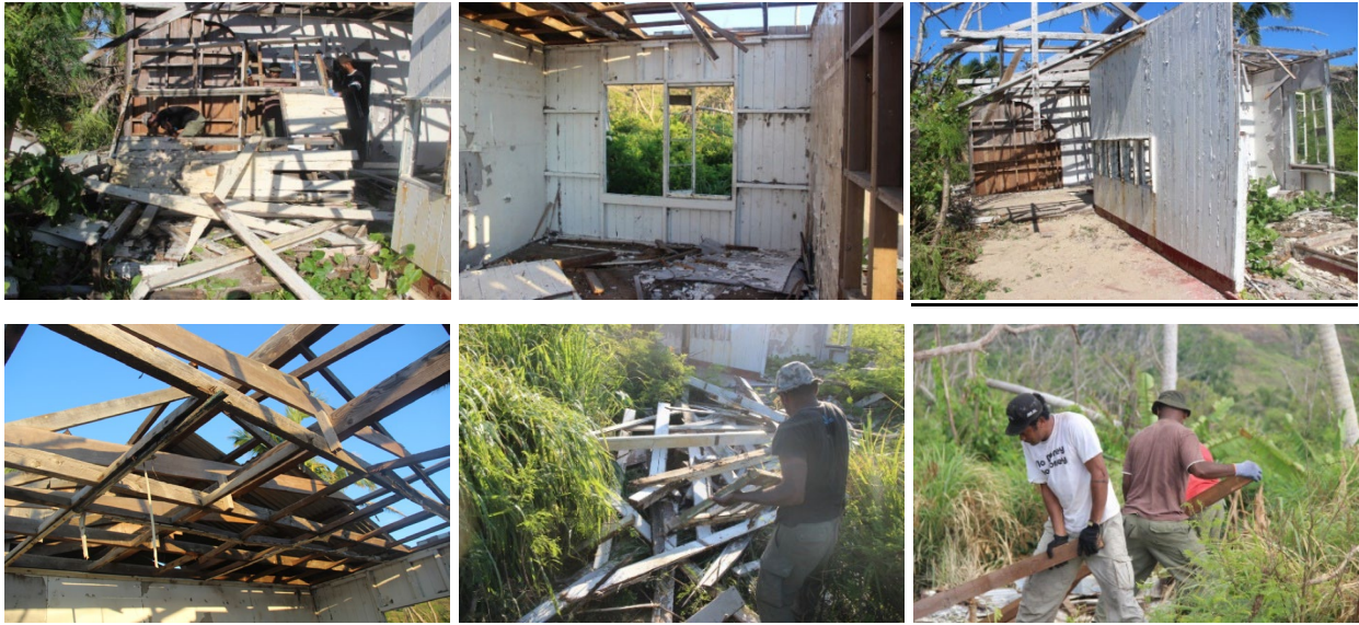
Site B building structure. Images credit: Fiji Museum
