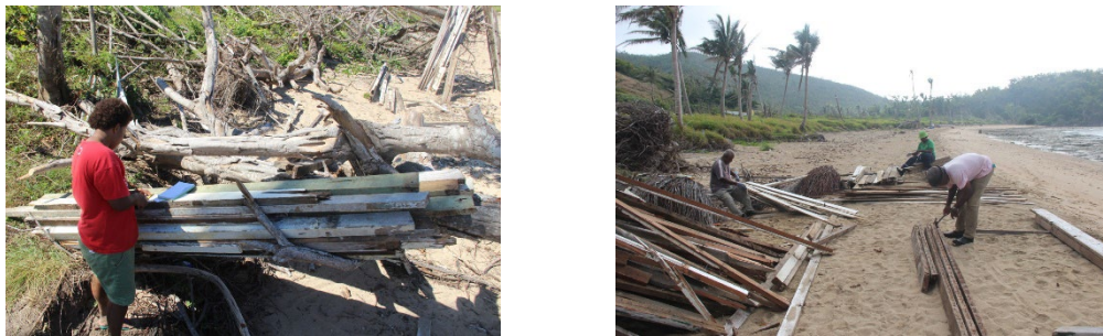
Measuring, extracting nails, piling the timbers according to their sizes. Images credit: Fiji Museum
