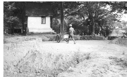
Filling soil in excavated pits
