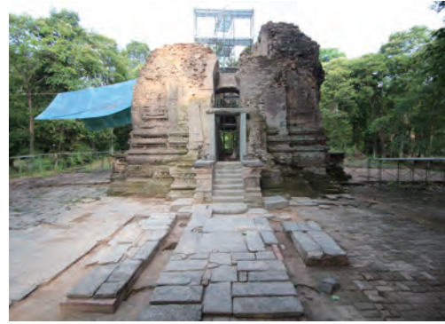
塔東面（修復後） East face of tower (after restoration)
