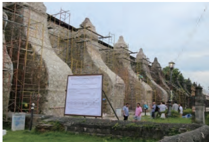
パオアイ教会の外壁の清掃 Cleaning of exterior walls of Paoay Church
