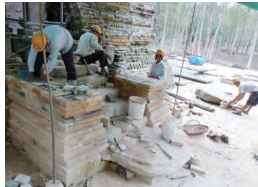
塔北面（修復中） North face of tower (under restoration)
