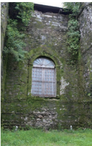
パオアイ教会の外壁 Exterior walls of Paoay Church
