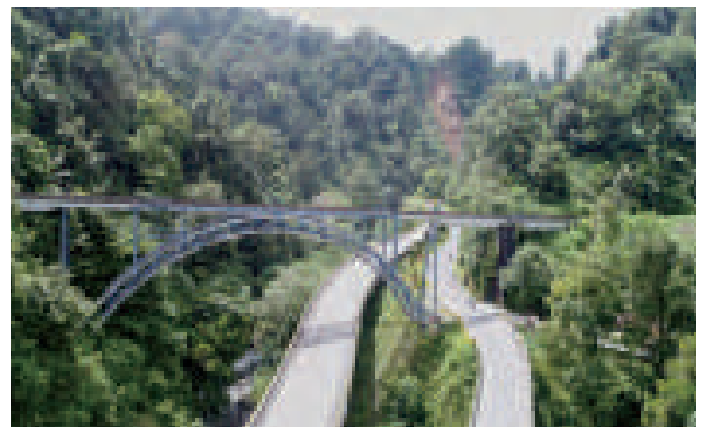
Fig.3 エリアB：鉄道施設と土木構造物 Area B: Railway Facilities and Engineering Structures
