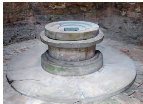
塔台座（修復後） Pedestal of tower (after restoration)
