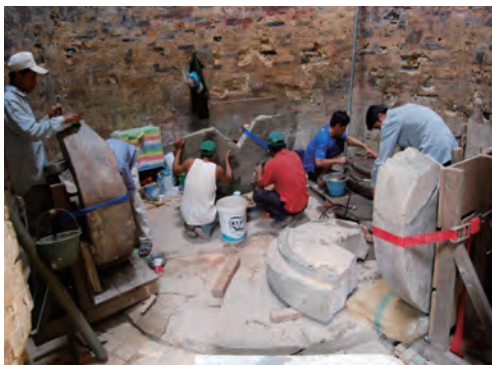
塔台座（修復中） Pedestal of tower (under restoration)
