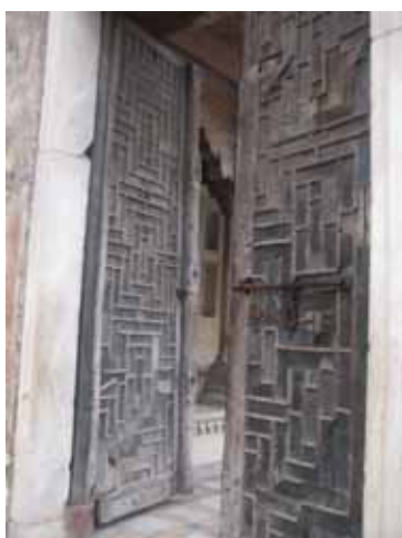
FIGURE 8,9. Old wooden door eroded by physical and chemical effects
