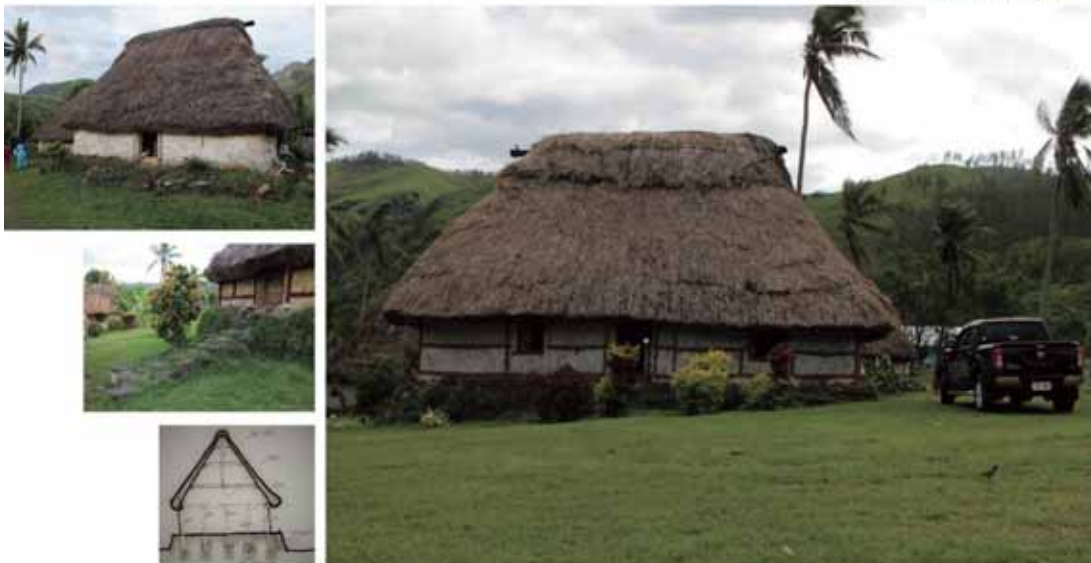
These houses were not damaged and were used for the community meetings and to host the damage assessment team for 2 days
