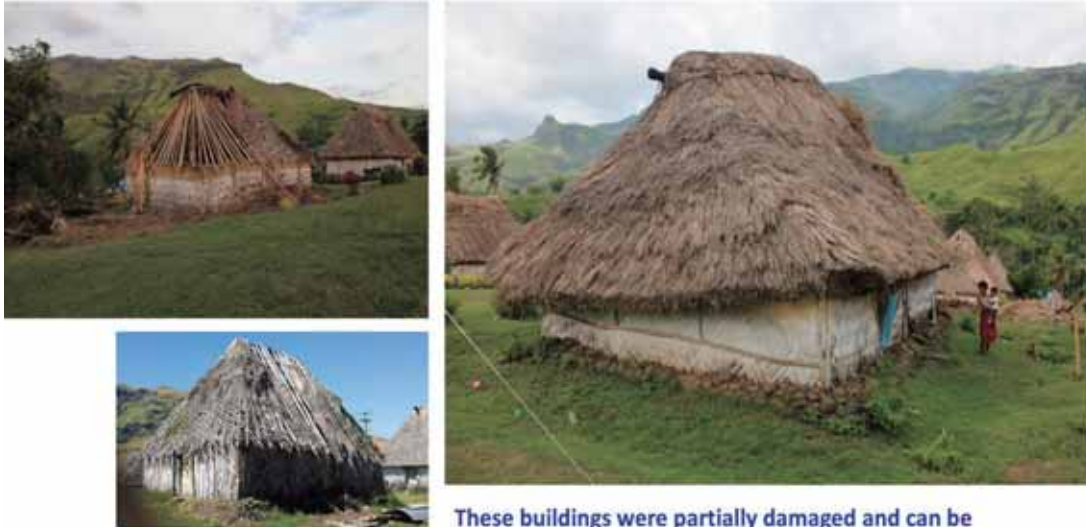
These buildings were partially damaged and can be repaired.
