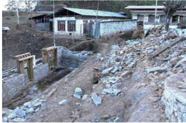
FIGURE 4. Construction of a Drasha (residence of a monk)
