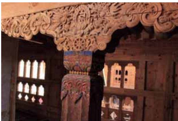
FIGURE 10. Preservation of old timber component
