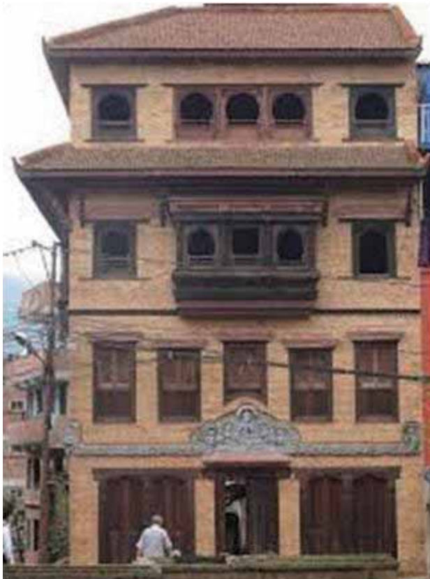
A traditional preserved house: after renovation
