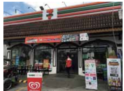
FIGURE 19. 7/11 Store (new construction)
