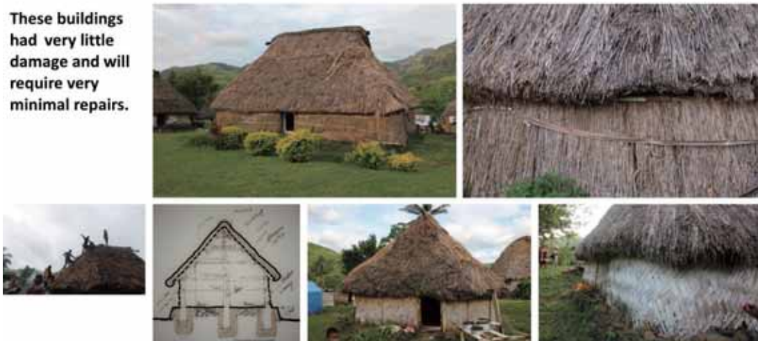
FIGURE 7. Black coded houses – Houses that had minor damage and require very little repair.
