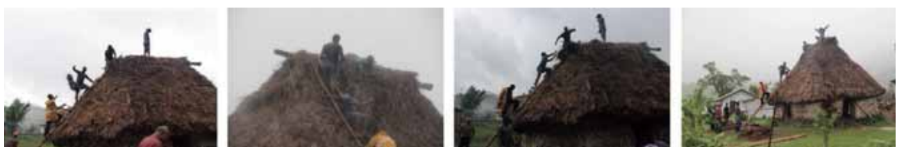
FIGURE 13. Maintenance works in Navala village.
