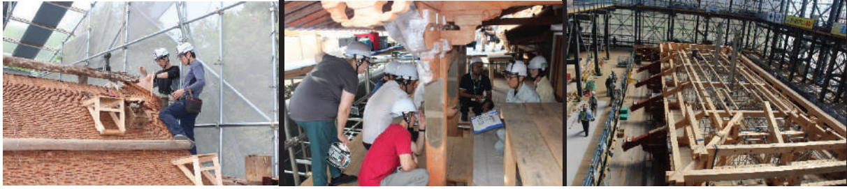
Fig.1 Site inspection of restoration projects
