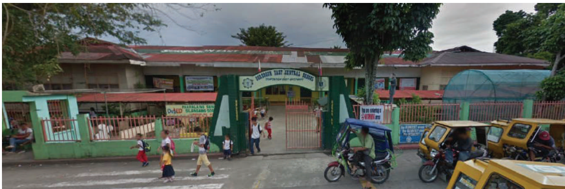
Fig.7 Pre-restoration panoramic view of the Sorsogon East Central School Gabaldon Building, showing the cramped site space
