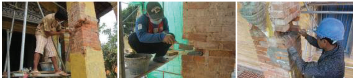
Fig.46–48 Repairing brick pillars
