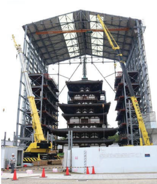
Fig.3 Well-organized restoration site of Yakushi-ji Temple original pagoda
