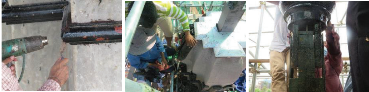
Fig.13 Restitution of the roof top of the Museum building 2018 (©NMC)
