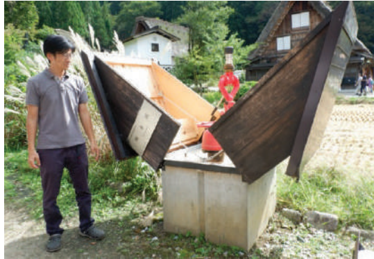
Small building storing fire extinguishers in Shirakawa village
