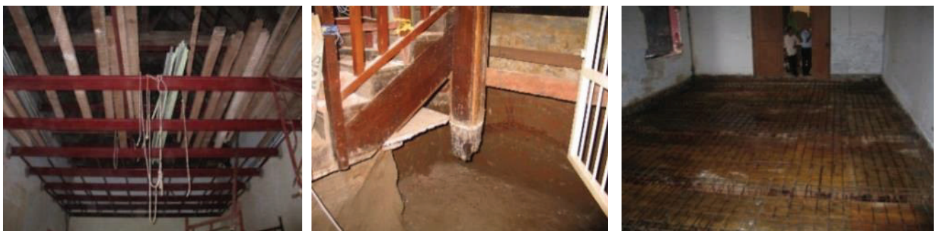
Fig.4 Renovation of the exhibition hall in 2006 (©NMC)
