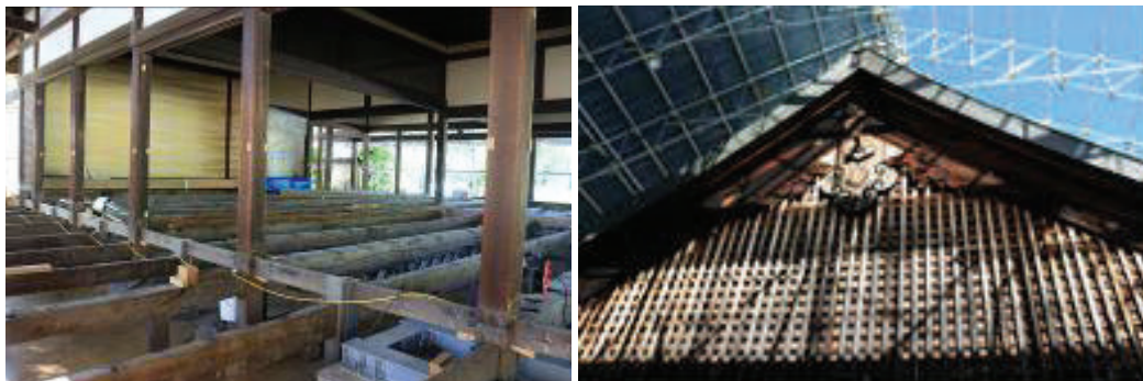
Restoration site at Toshodai-ji Temple
