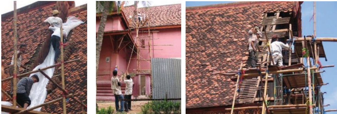
Fig.6 Repairing the roof top, 2008 (©NMC)
