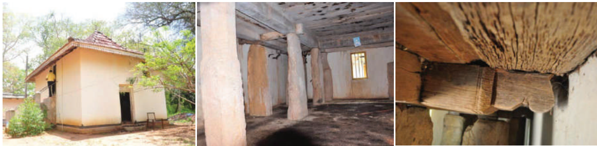
Fig.5 Modified tampita vihara and its current interior condition
