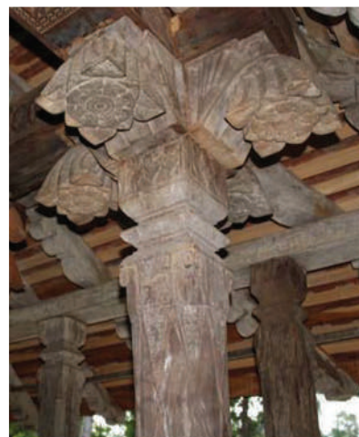
Fig.2 (Left) Section and isometric view of pekada (Right) Carved pekada at Panavitiya Ambalama
