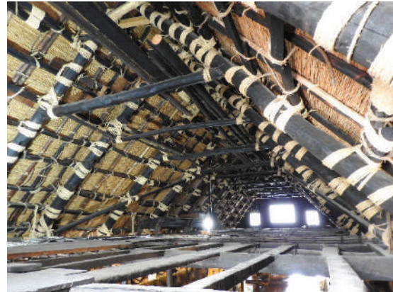
Fig.4 Roof structures at Shirakawa village,Gifu
