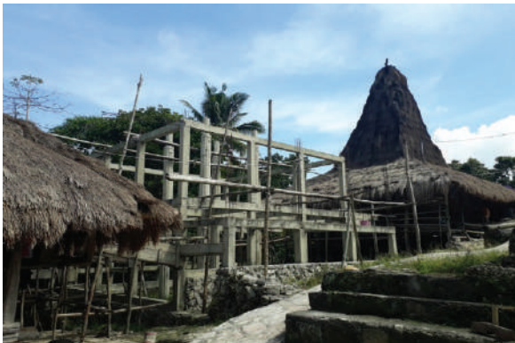
Left: Traditional houses in Sumba using concrete instead of bamboo columns and beams
