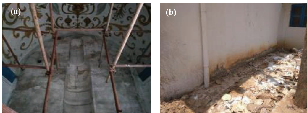
Figure 8. (a) The altar after removal of the wooden panels, and (b) the exterior wall of the altar
