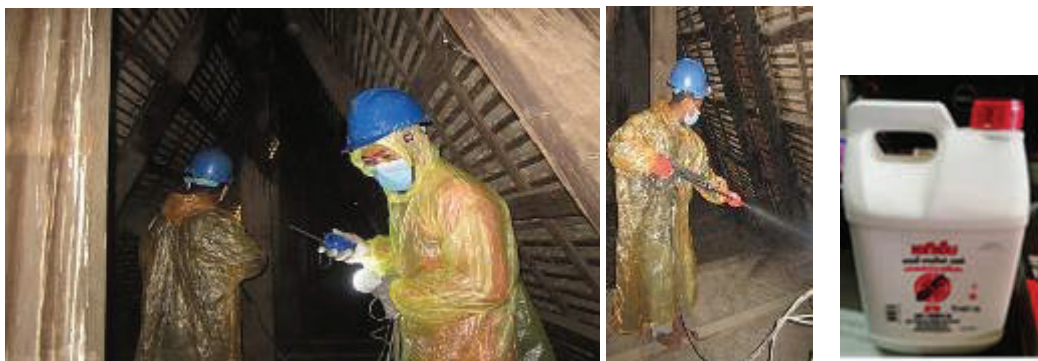
Fig.37–38 Removing termites from the wooden structure Fig.39 Poison for removing termites
