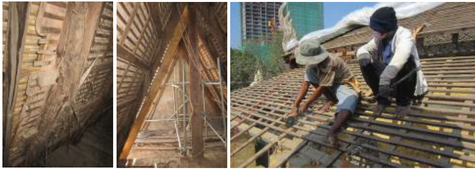
Fig.40–42 Repairing the damaged wooden structure of the temple
