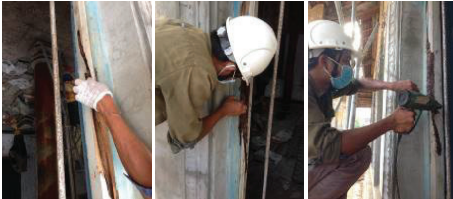
Fig.43–45 Restoring wooden portions destroyed by termites
