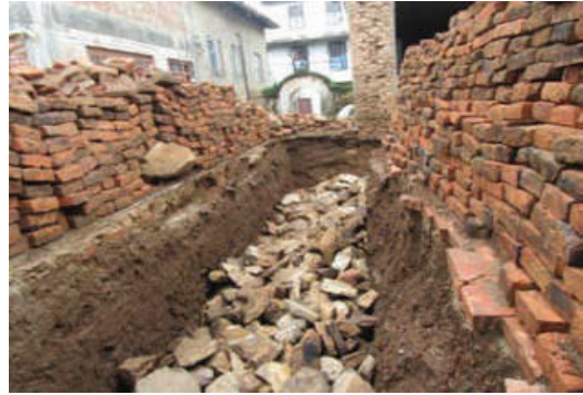
Fig.5 Exploration of the foundation
