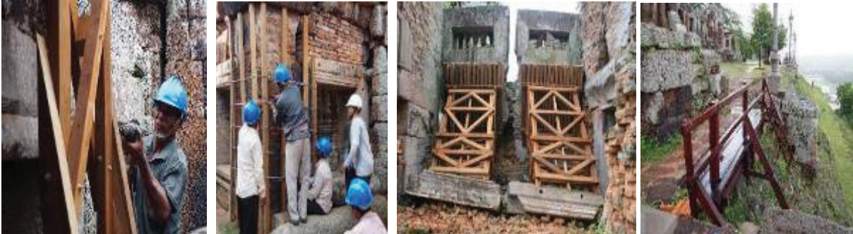
Fig.16–19 Emergency work on monuments
