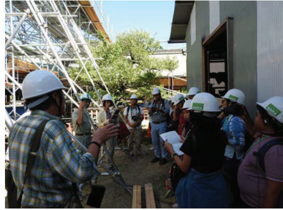
Fig.2 observation Restoration and field study at Toshodai-ji Temple (Nara city)
