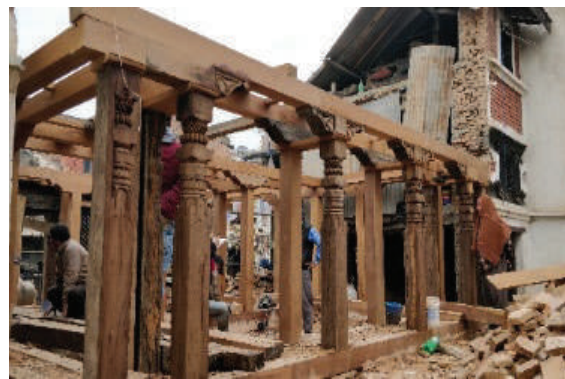
Fig.6 Thams (posts) and nidals (beams) are erected
