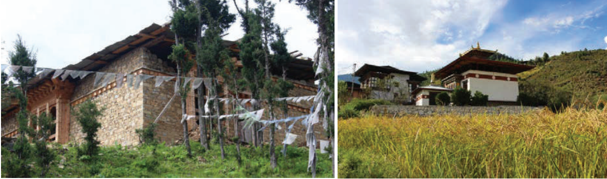
Fig.4 Reconstruction in progress (left) and major alteration to the design (right)
