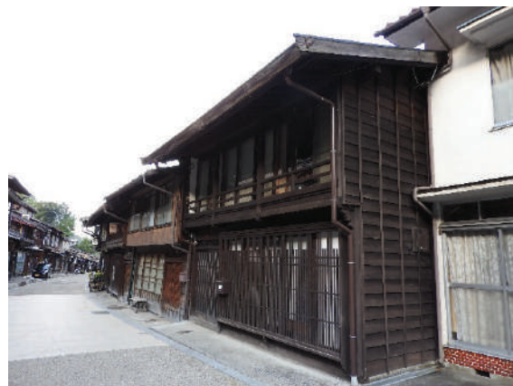
Fig.6 façade of group traditional building, Shiojiri-shi Narai ,Nagano
