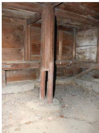
Fig.1 Left: Tenman Shrine used as case site for documentation and evaluation during the training course Right: Evidence of change (survey traces) seen in the base of pillar.
