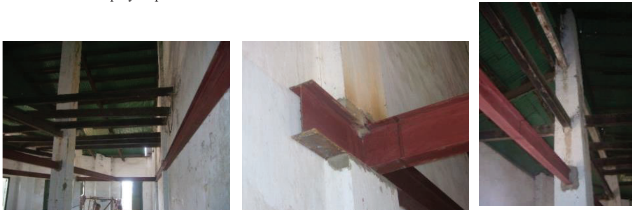
Fig.8 Stabilizing a structure to be dismantled, colonial building in Kampot, 2014
