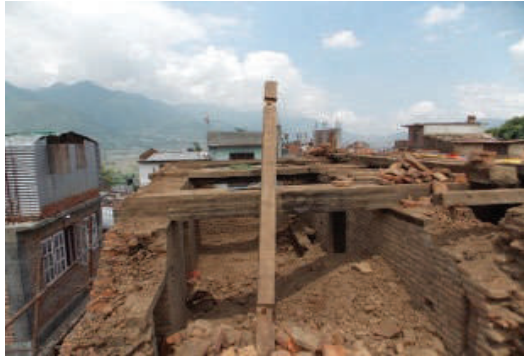
Fig.4 Disassembly in progress
