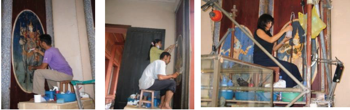
Fig.5 Repair and repainting of a window of the National Museum, 2006 (©NMC)
