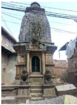
Fig.8: Damaged Shakyamuni Buddha during earthquake
