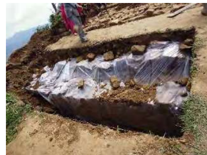
Fig.2: Back filling of trench after documentation
