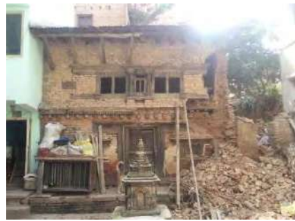
Fig.9: Bihar during earthquake
