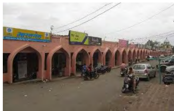
Figure 5: Unsympathetic interventions done by government agencies under a development scheme
