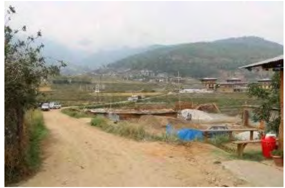
New modern structure under construction
