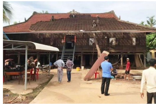
Fig.2 Dismantling Process
