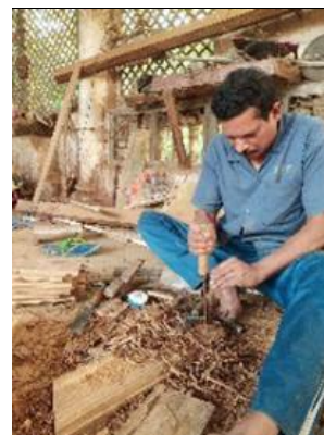
Carpenters reproducing missing wooden posts
