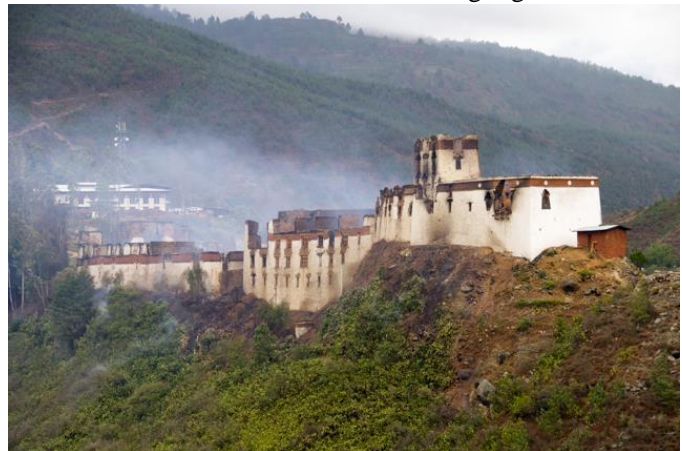
Photo 2. Aftermath of the tragic fire incidence.
