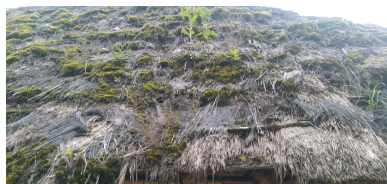
Figure 3- Uma Lulik Darlau Aimet and Berhunu with plants growth on the top of Roof in Manutasi, Ainaro; Source: SEAC, 2019
