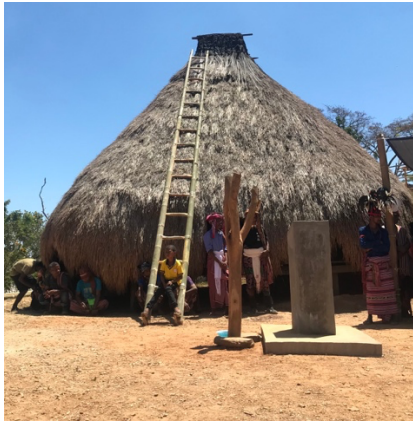
Figure 1-Uma Lulik with the type of ground floor, in Aileu; Source: SEAC, 2021
