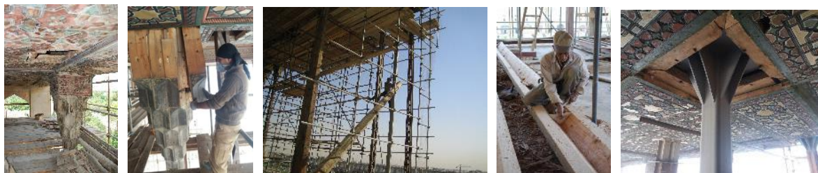
Picture 4, 5, 6, 7, 8: Restoration and strengthening of wooden columns (source: Meidan Emam World Heritage Office archive)
