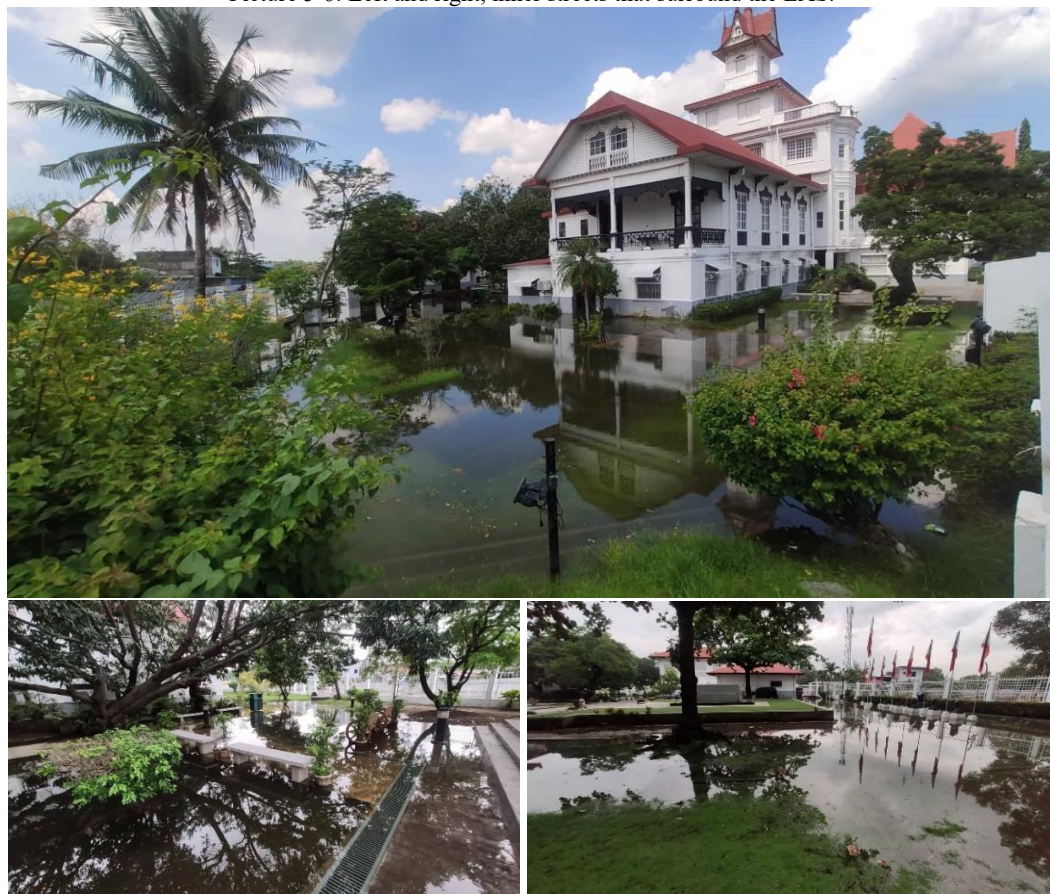
Picture 7-9: EAS complex flooded by high tide (July 2022)
