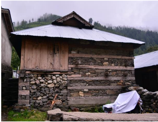
Figure 4 The rear elevation with the horizontal wooden beams and stone infill.
