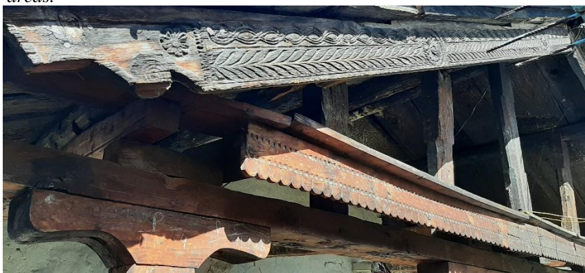
Fig 11. and Fig 12. Apart from construction of the structure, a remarkable level of wood carving and ornamentation can be found in the door frames, brackets, pillars, panels and other parts of the structure in deodar wood which comprises of mostly of geometrical patterns.
