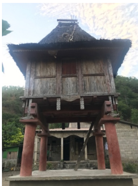
Figure 3Uma Lulik Latuloho with pillars cemented and painted, in Camea Dili/Capital, originated from Tutuala-Lautén; Source: SEAC, 2022
