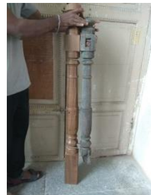
Carpenters reproducing missing wooden posts
