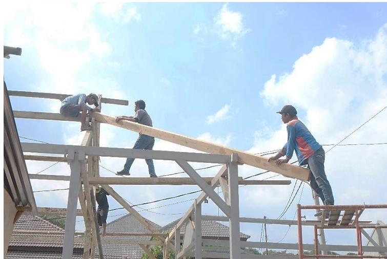
Picture 4. skillful workers demonstrating replacement of new rafter Source: Galih Nagari, 2018
