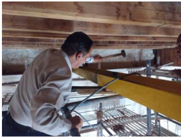
Additional support of I sections added to the system of wooden beams
