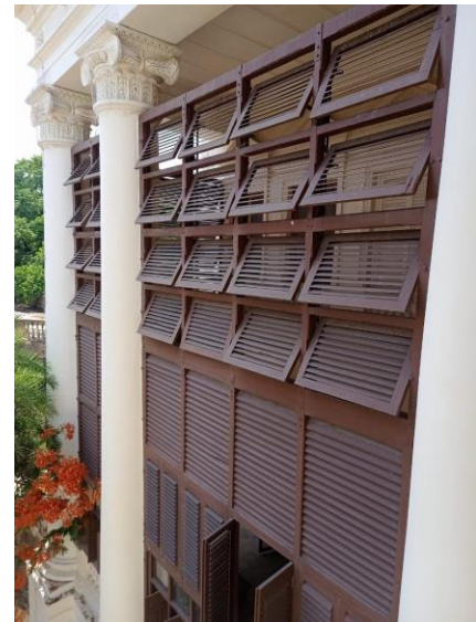
Louvers Southern facade
