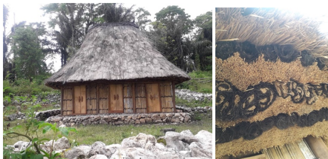
Figure 6 The seven alternating layers of grass and tali metan/arenga pinnata palm ( tua metan or tali metan in Tetun), in Ossu Viqueque ; Source: SEAC,2018;
