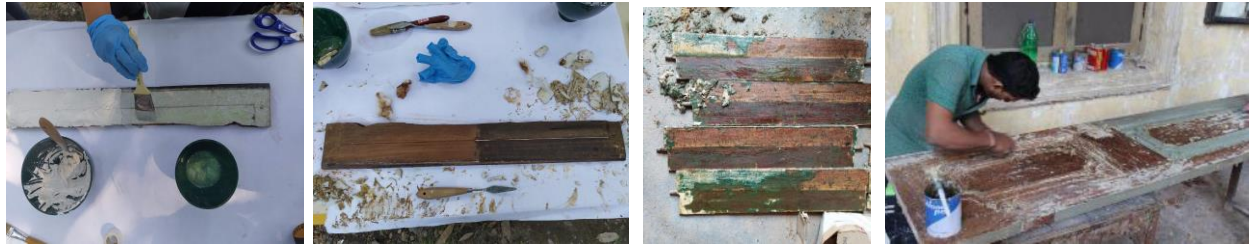
Different techniques used for removing multiple pain layers
