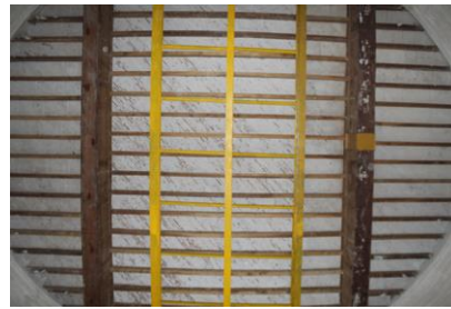
Additional support of I sections added to the system of wooden beams
