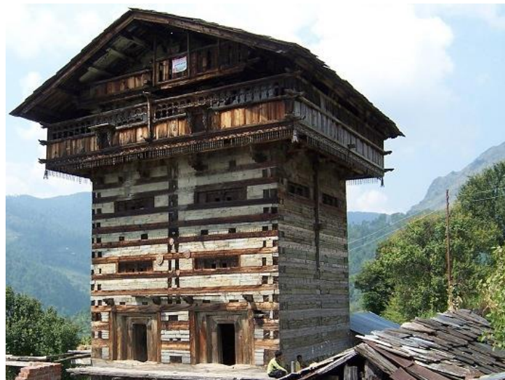
Figure 7 Five storied high Koti Banal structure at Koti village of Uttarakhand (Ref : Rautela, P., et.al.: Housing Report: Timber-reinforced Stone Masonry (Koti Banal Architecture) of Uttarakhand and Himachal Pradesh, Northern India. World Housing Encyclopedia
