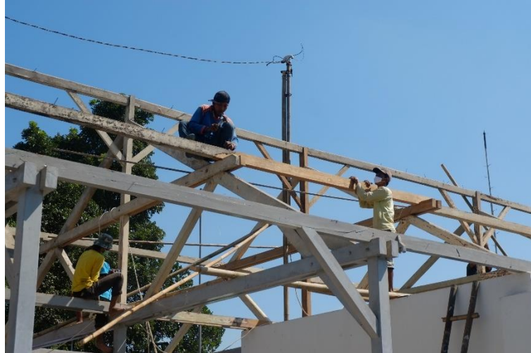
Picture 3. skillful workers demonstrating replacement of new girder Source: Galih Nagari, 2018
