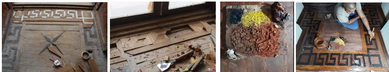
Process of restoration of a parquet border
