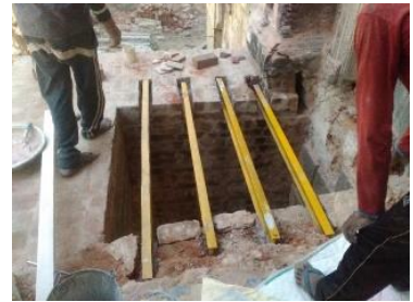
I sections being used to replace
