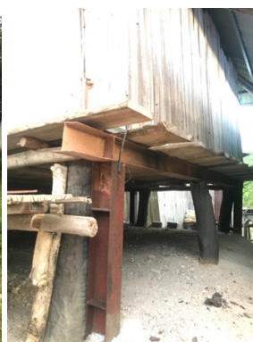
Figure 1Uma Lulik Asumeta with the roof used by Zinc and its column support by the Iron, in Camea Dili; Source: SEAC, 2022;
