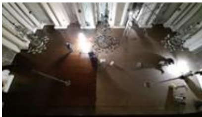
Process – Finishing layer of flooring
