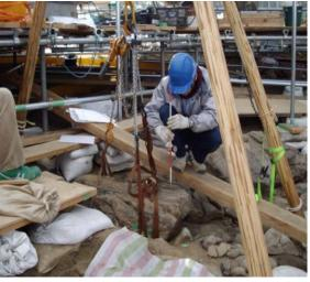
② After reinstallation of the stones has been completed, the gaps surrounding the stones are filled with clay.
