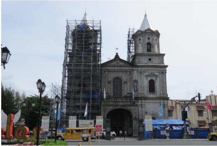
Image 2 The HRP under conservation works (Photo by © ETFFI).
