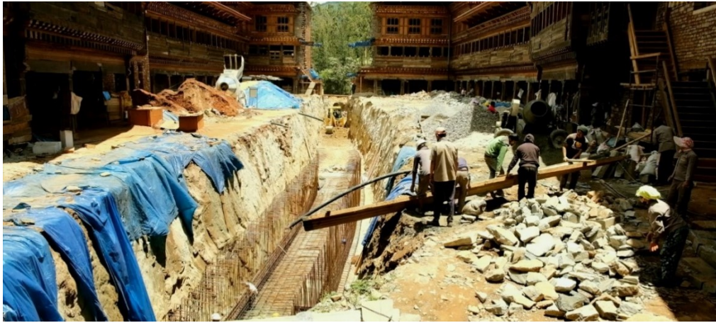
Figure 8. Construction of the service tunnel. Source DCHS
