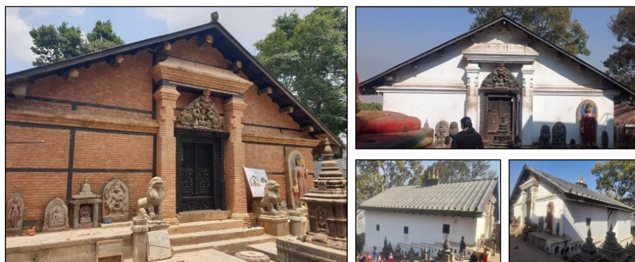
SHANTIPUR TEMPLE : After Rehabilitation
