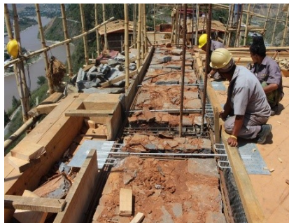
Figure 6. Installation of Wangdue latch Source: DCHS
