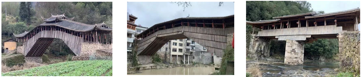
Figure 3. Xuezhai Bridge (left), Wenxing Bridge (middle) and Wenzhong Bridge (right) after reconstruction
