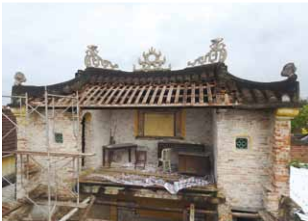
Flaked mortar walls were removed.
