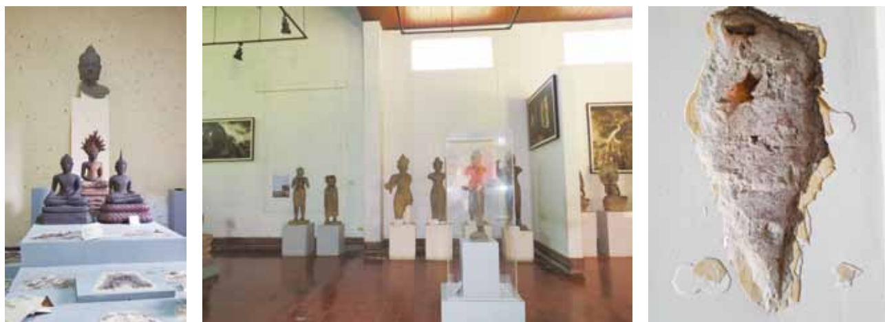
Fig. 6: Dirty wall due to pigeon droppings and peeling mortar
