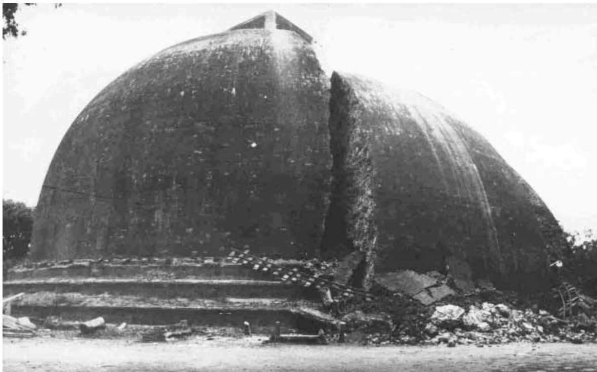
Failure of the restored dome of Mirisawetiya Stupa – Second attempt in the eighties
