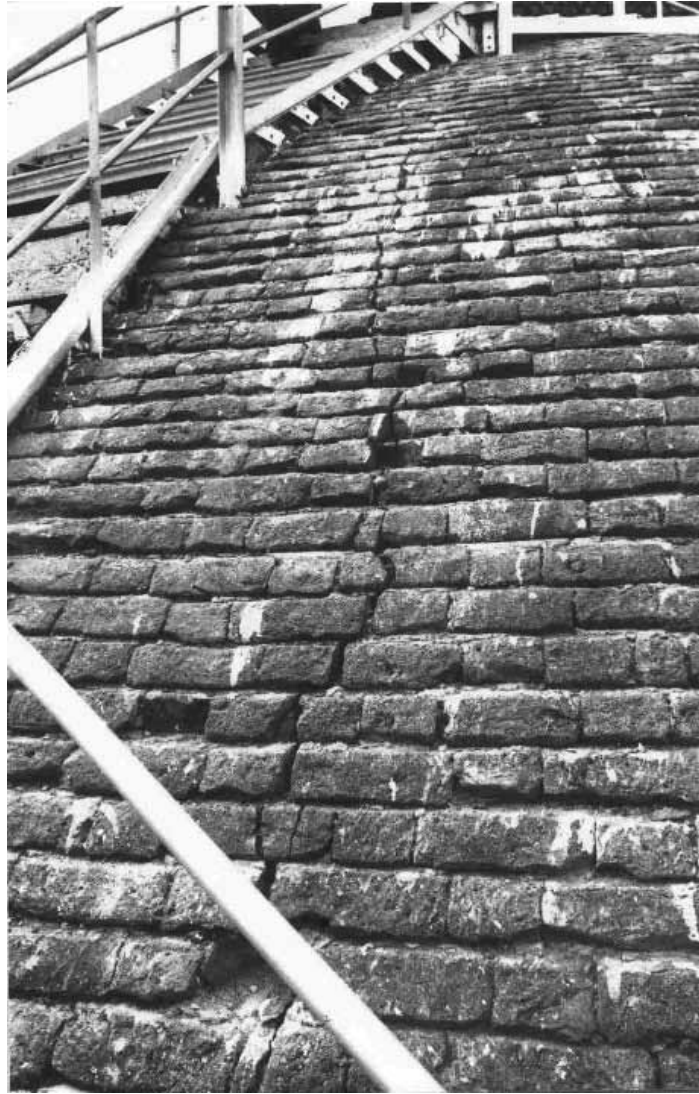
Cracks that appeared on the dome of Mirisawetiya before the failure
