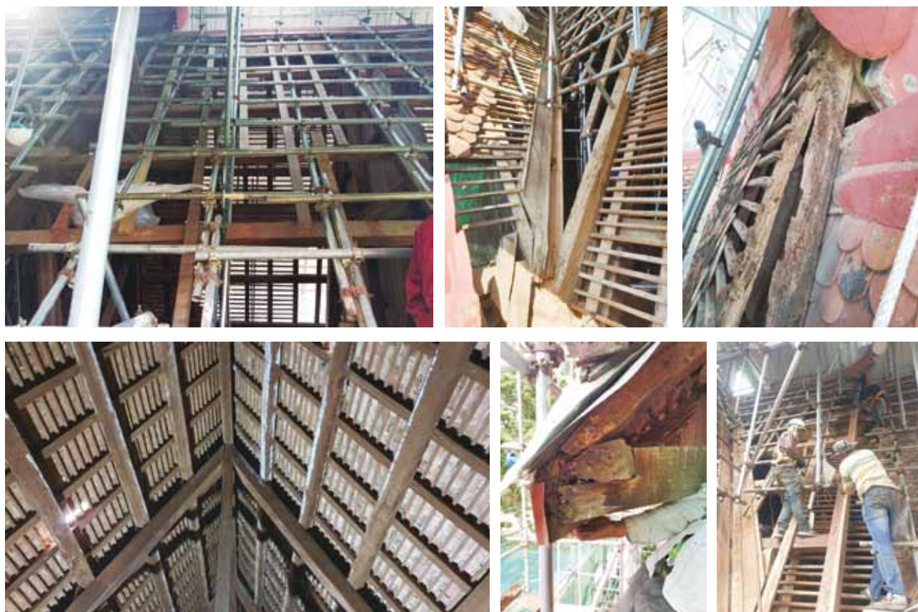
Fig. 5: Damaged timber
