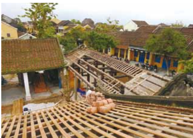
Restoring the communal house's roofs
