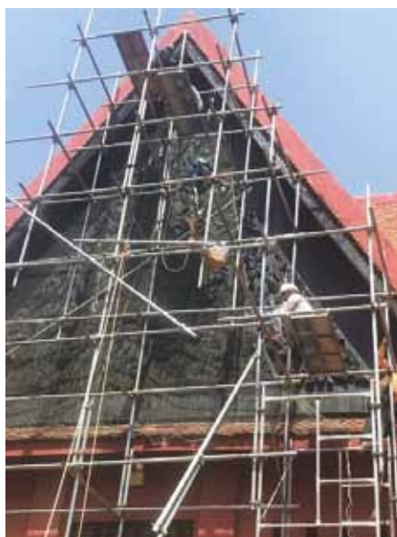
Fig. 2: Installation of pigeon bars under the pediment
