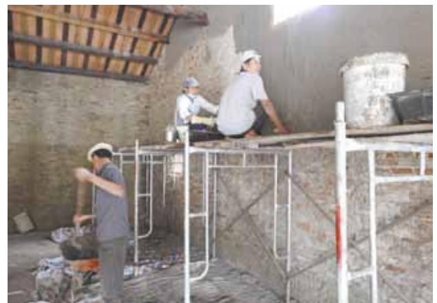
Rendering the walls with lime mortar
