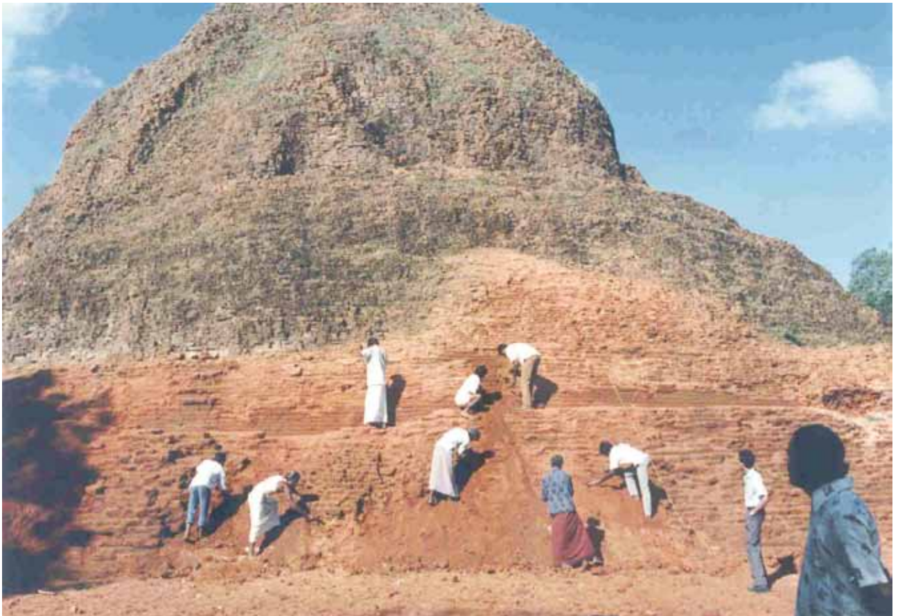
All loose ancient brickwork was carefully removed.
