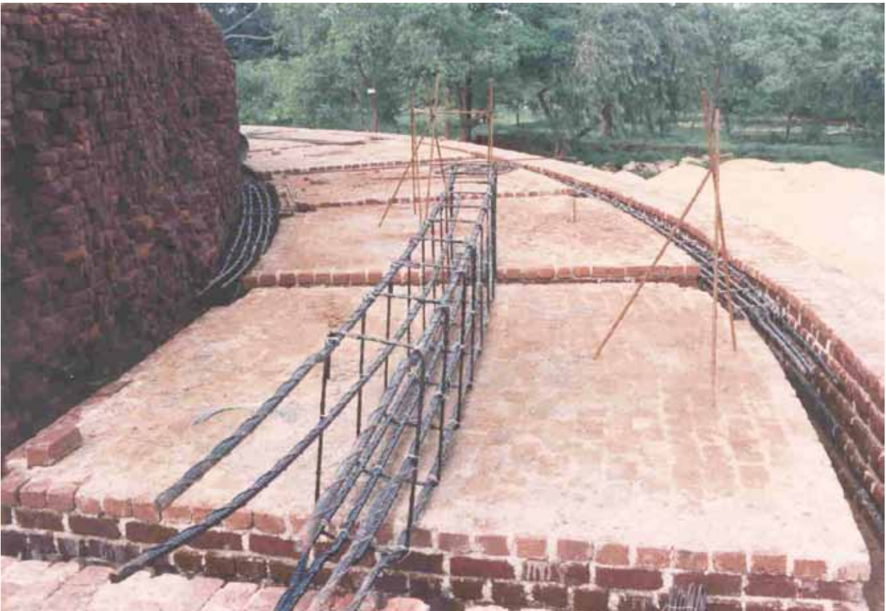
Prior to the casting of reinforced concrete rings
