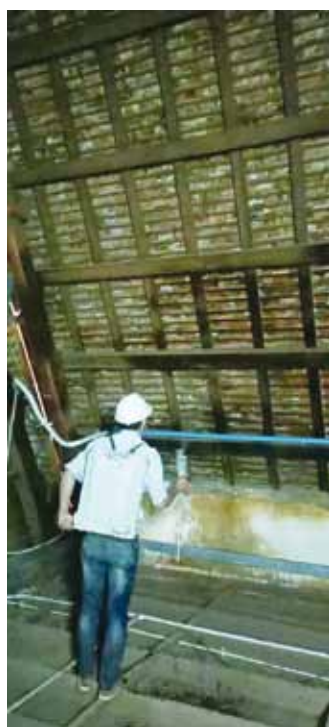
Fig. 3: Termite treatment
