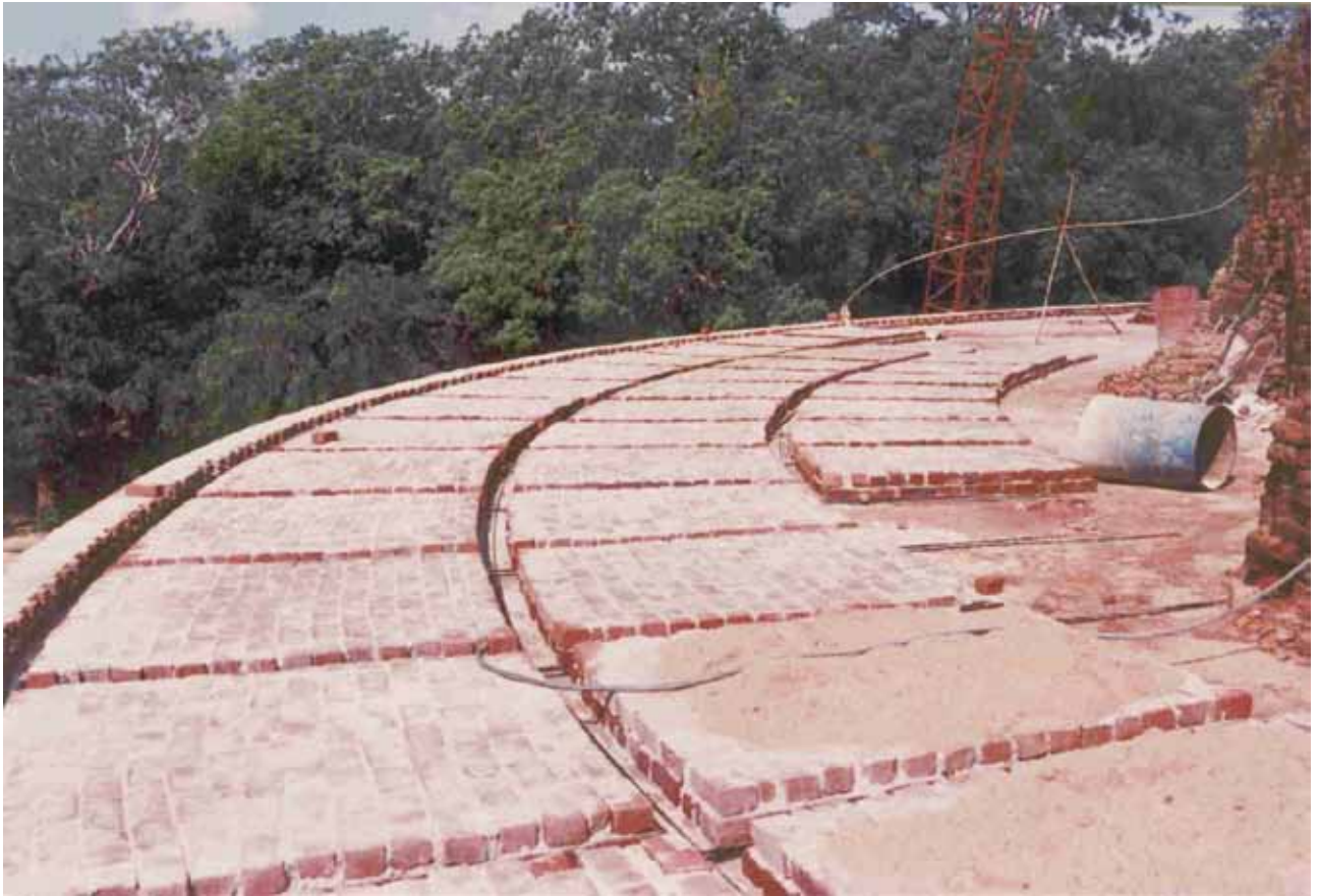
Prior to the casting of reinforced concrete rings
