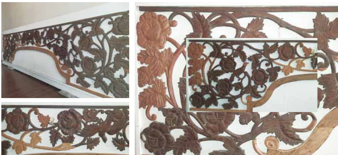
The restoration of the missing parts of a wooden calado with floral, leaf, and bird motif ornamentation was part of their project. The composition was completed based on the remaining existing parts. The wood material used is narra, considered as one of the hardest local woods.
