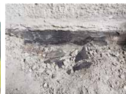
Condition prior to restoration: There were traces of damp roofing used during the 1950s rehabilitation that had contributed to further deterioration of the walls.
