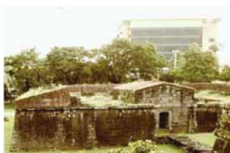
Condition prior to restoration: There were traces of damp roofing used during the 1950s rehabilitation that had contributed to further deterioration of the walls.
