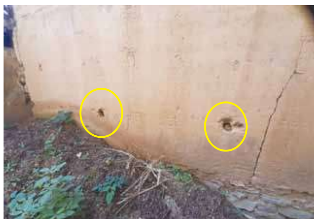
Fig. 5. Left: Photos showing evidence of hanger holes with wood remnants. Right: Plan showing the direction and location of hanger hole remnants
