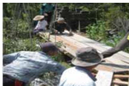
Figure 9. Manufacturing stone sliding boards made of wooden
