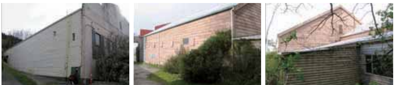
Figure 4. Exterior photographs of the hall (south, north and west/back walls) showing its weather board construction and alterations over time, such as pressed steal cladding replacing the weatherboards on the south side of the building and the lean-to added on to the west (back) wall (source: Guy Williams & Assoc's).
