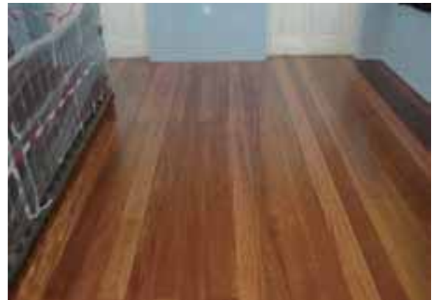
Timber floorboards at upper floor were carefully removed, inspected and replaced with new timber of similar size and species to retain the building authenticity.
