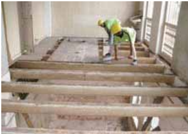
Timber floorboards at upper floor were carefully removed, inspected and replaced with new timber of similar size and species to retain the building authenticity.
