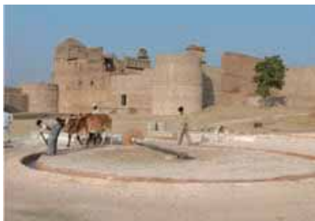
Preparation of mortar using ancient technique
