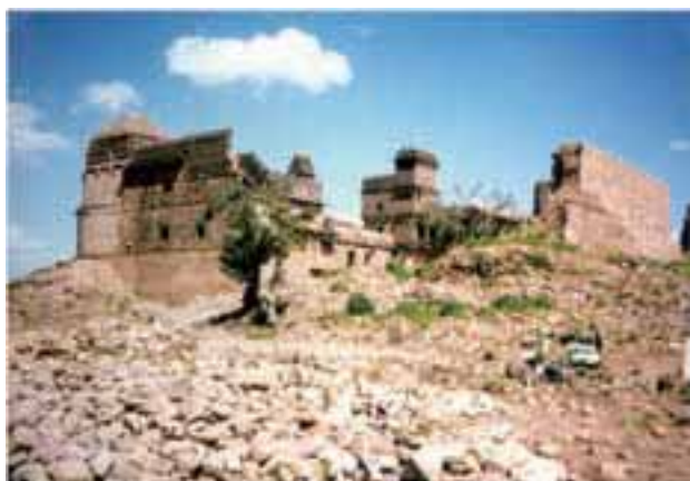
Navkhanda Mahal in damaged condition
