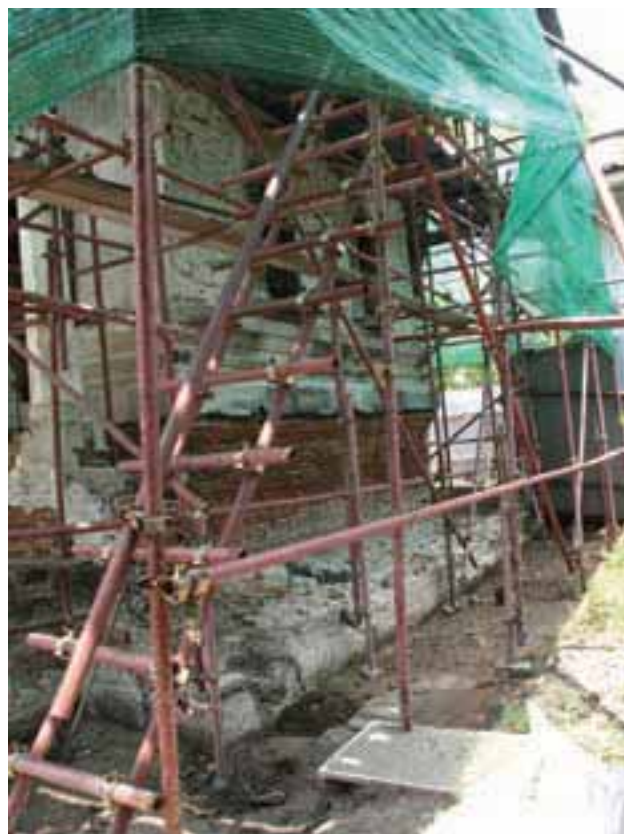
Figure 8: The remaining base structure of disappeared corridor, the brick patio and the gutter after finishing the excavation in the west.
