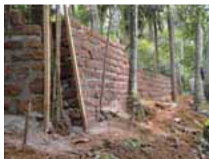
The southeast bastion during restoration
