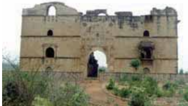
Koshak Mahal before conservation
