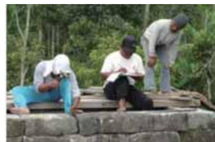
Figure 8. Marking activities / stones registration before dismantling
