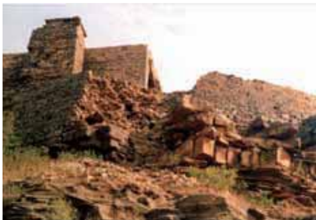
Fallen fortification walls of the Fort
