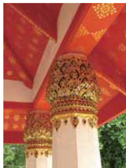
Figure18: The decoration of lotus shape capital after finishing the restoration.
