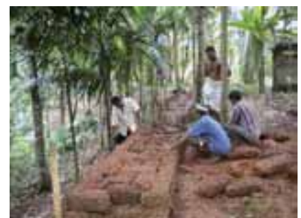
The southern wall during restoration
