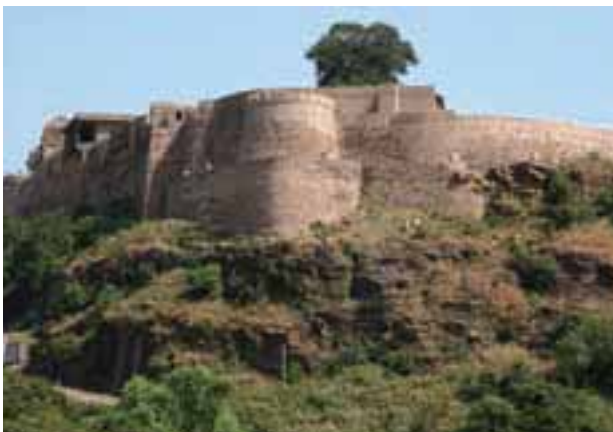
Fortification walls after restoration
