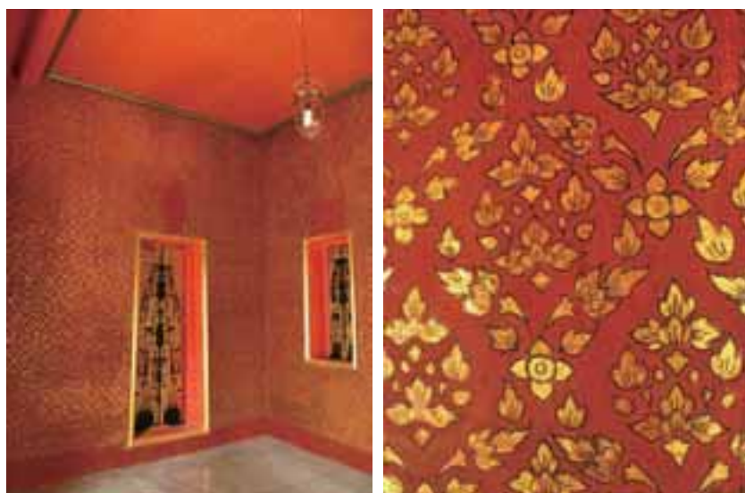
Figure17: The Tripitaka hall after finishing the restoration, (a) interior view, (b) decoration detail of gilt painting.
