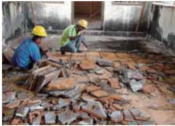
Damaged terracotta floor tiles at upper floor were replaced with the new ones of similar type, material and size as the original.
