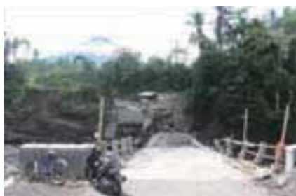
Figure 3. Bridge / Check Dam interrupted by a stream of cold lava and Mount Merapi in the background
