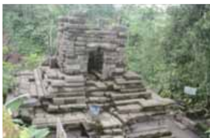
Figure 6. Conditions of the temple before dismantling
