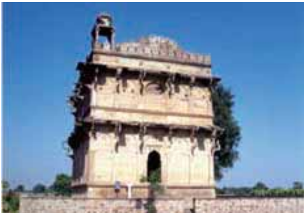
Shahzadi ka Roza before conservation
