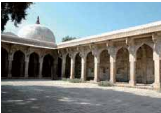
Jama Masjid after removal of lime plaster
