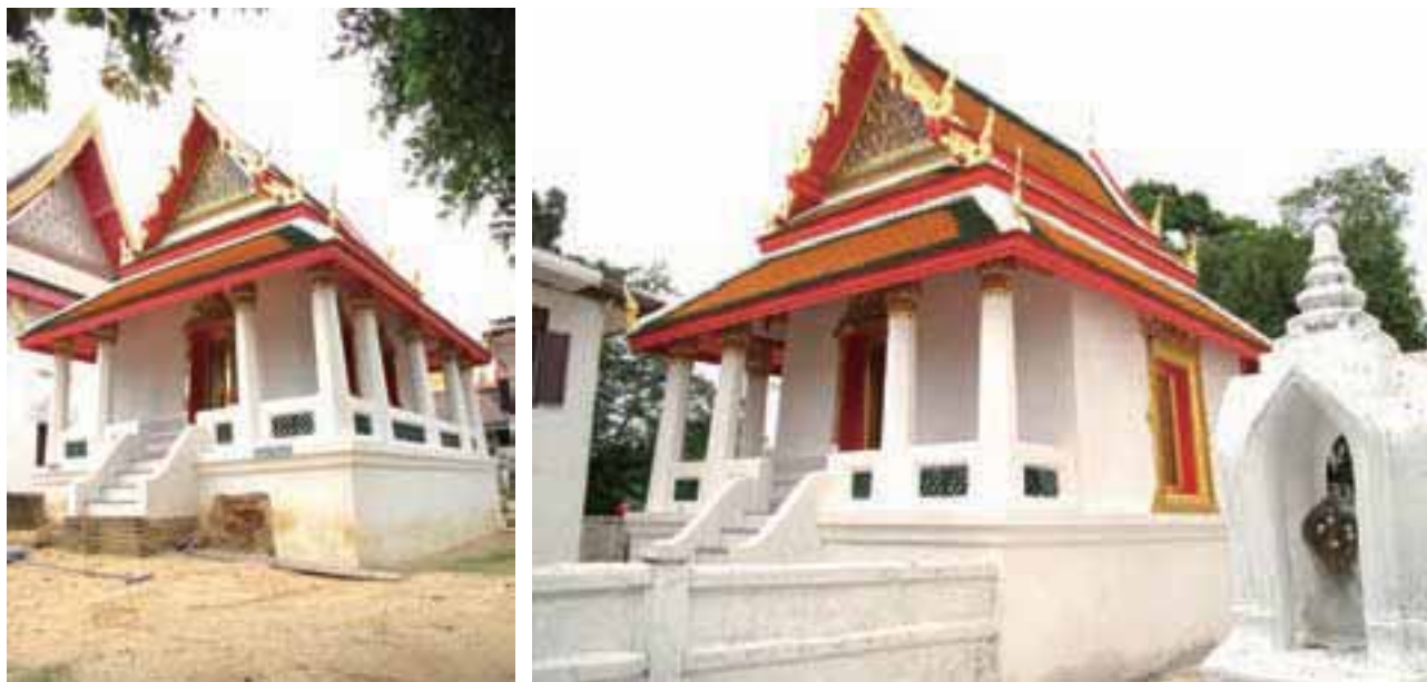
Figure16: The Tripitaka hall after finishing the restoration, (a) the ruin of the extended platform was covered with sand in order to protect damage and stay for restoration in the future. (b) View from the south.
