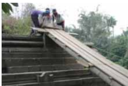
Figure 10. Dismantling activities by using board sliders; stones are tied to prevent damage.
