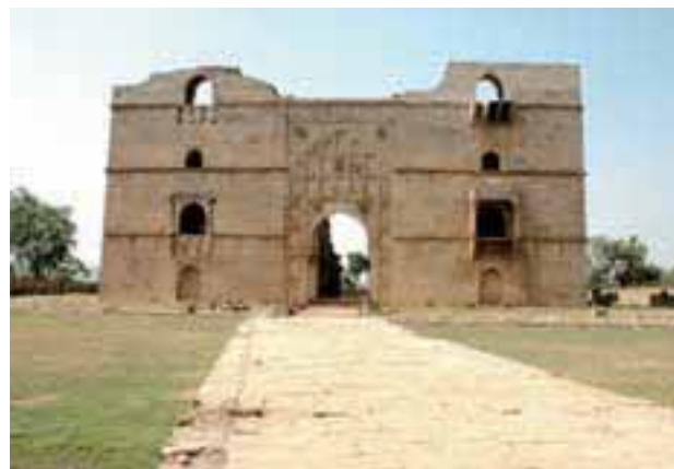
Koshak Mahal during conservation work
