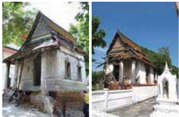
Figure 1: Exterior existing condition of The Tripitaka hall in the preliminary survey: (a) the north, (b) the south
