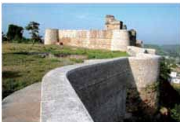
Navkhanda Mahal after restoration
