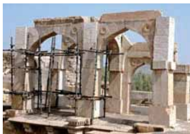
The arch of Koshak Mahal during conservation work
