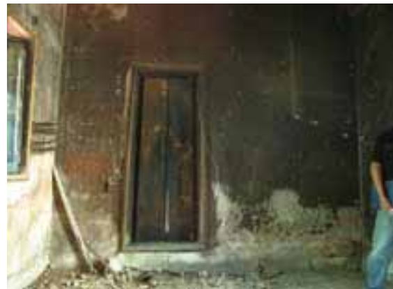
Figure 2: Interior existing condition of the Tripitaka hall in the preliminary survey.
