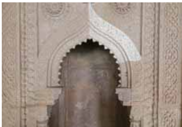
A part of an arch in Jama Masjid is left half done (covered with lime plaster) for reference.
