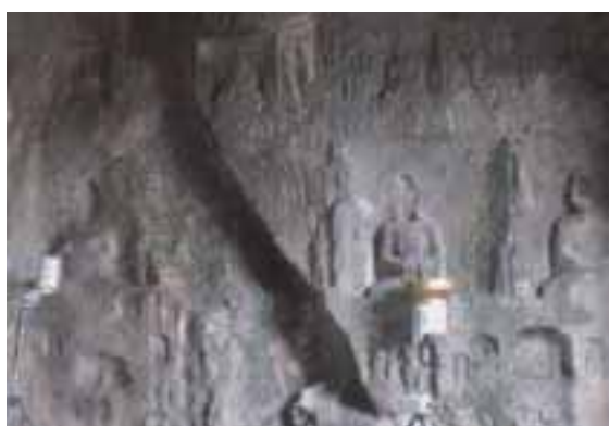
Fig. 3. Leaking water running through cracks on the north walls inside the Ludong Cave
