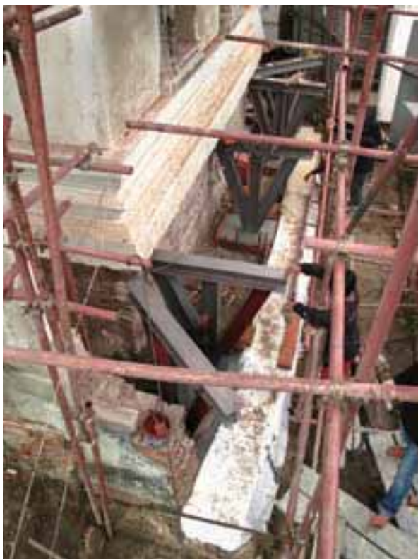
Figure 13: The new structure, I-shape steel, in the west corridor reconstruction. The original remaining structure was protected by the textile to conserve it in the existing state before starting reconstruction.
