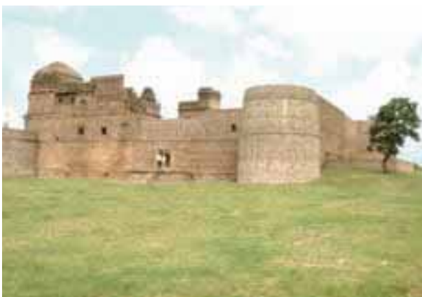
Navkhanda Mahal after conservation and restoration
