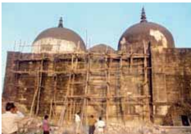
The rear view of Jama Masjid before conservation
