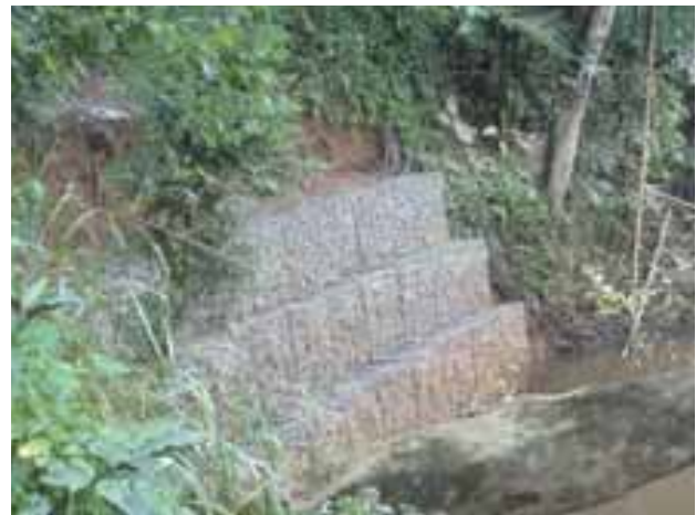
Gabion wall, constructed to prevent erosion
