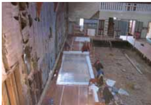
Figure 20. The work area during recovery (source: Guy Williams & Assoc's)
