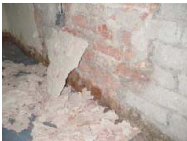
The poultice is left to suck up all the mineral salts over the period of at least 2 weeks. It becomes dry like a cardboard mould before it can be peeled off and disposed.
