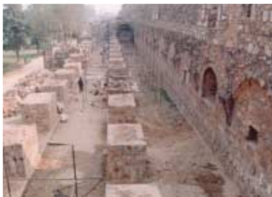
Raising of pillars in R.R. Masonry
