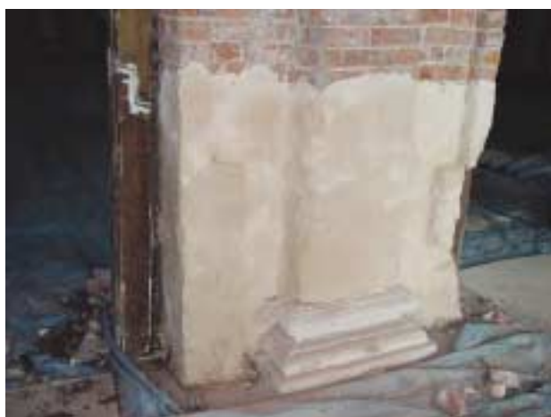
The Cocoon method uses creamy paste, in a form of poultice, to solve the problem of salt contamination mainly in the masonry walls, pilasters and columns.
