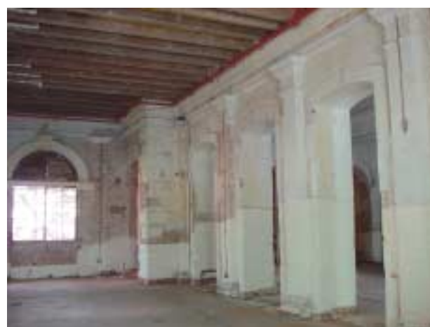
The Cocoon method uses creamy paste, in a form of poultice, to solve the problem of salt contamination mainly in the masonry walls, pilasters and columns.
