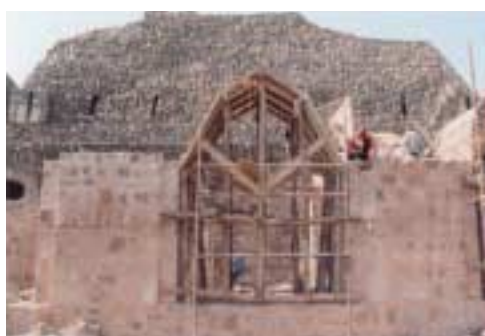
Wooden frame to obtain the shape of arch
