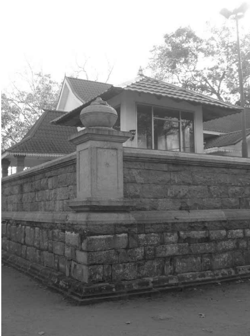
Conservation of the stone retaining walls of the terraces of the sacred Bodhi-tree at Anuradhapura. The upper section of the retaining wall is restored using stone work reproduced with mechanized-systems.
