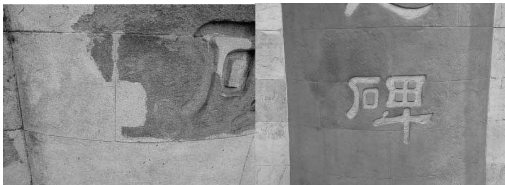
Fig. 2: restoration details after 10 years exposure (taken in 2010, left) and new staining (taken in 2011)
