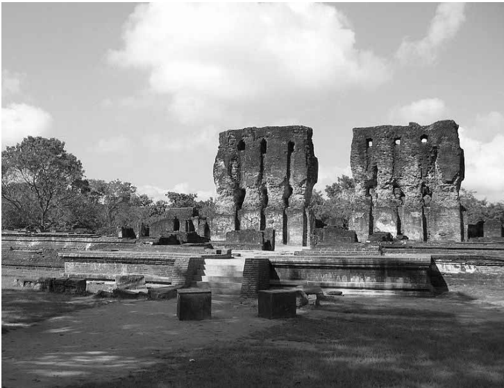
Parakkramabahu Palace, Polonnaruwa (12 th century AC). Note the vertical crevices and the holes of the brickwork indicates the vertical wooden reinforcements and the horizontal floor beams respectively.
