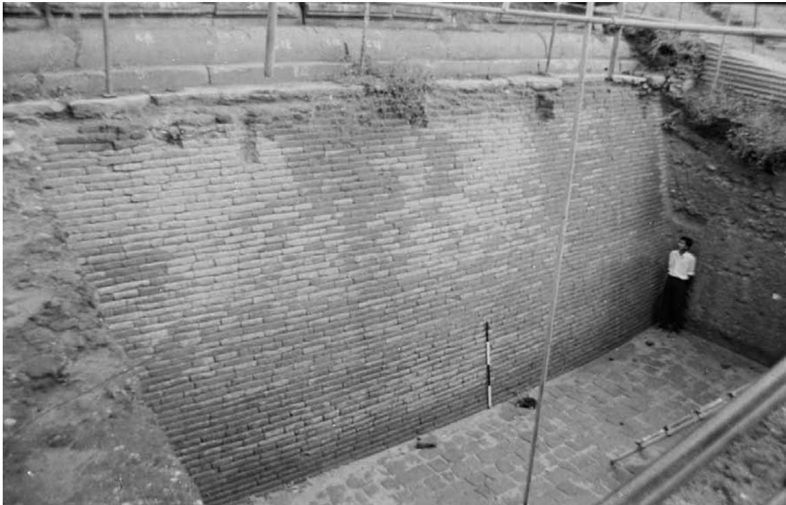
Foundation of Jetavana stupa
