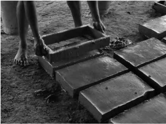
Process of preparing green bricks
