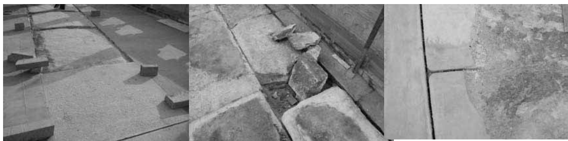
Fig.6: Methods to restoration (from left to right: replacement, piece-in and re-profile)
