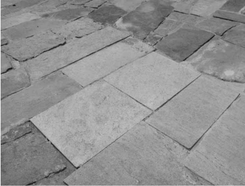
Stone paved terrace of Mirisaveti stupa showing the filling of voids and missing stone work with machine-cut stones
