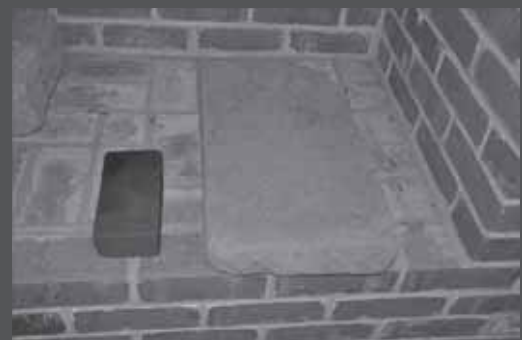
Comparison of ancient brick (450x225x50 mm) with modern brick (212x106x56 mm)
