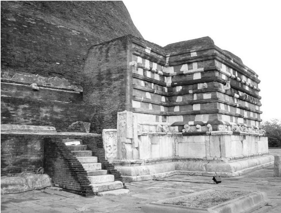
Stone frontispieces of Jetavana stupa showing the filling of voids and missing stone work with brick work
