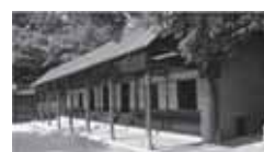
Left: Façade of Seonhyangjae (a study building of Youngyeongdang, Changdeokgung, Seoul, Historic site no. 122). Right: A detail of its side. By using brick, a brick artisan has imitated a gable of wooden architecture.
