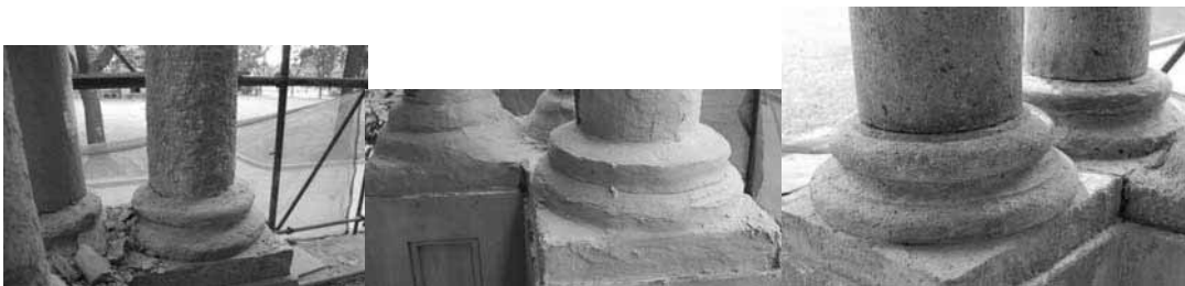
Fig. 9: Desalination before restoration in Shanghai
