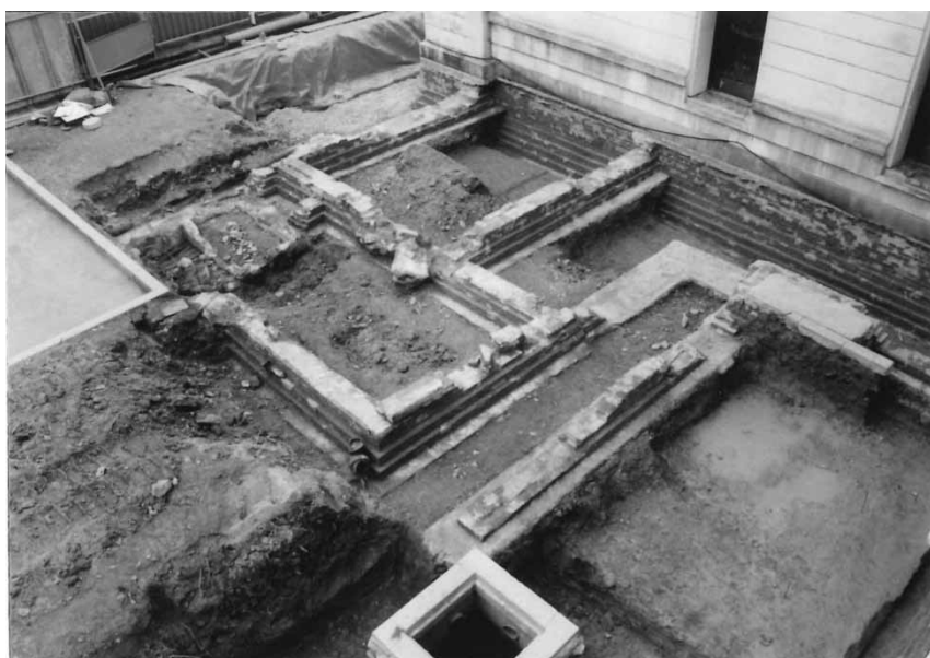
Photo 5: Brick foundation of back brattice found in excavation survey
