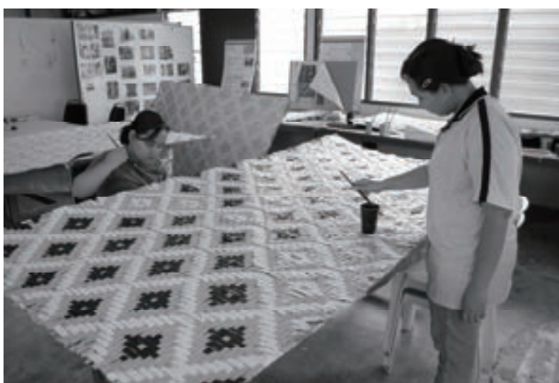
Local villagers were involved in repainting the bamboo-weaving panels.
