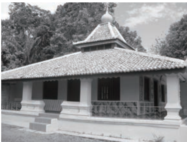
The Old Macap Mosque was designed symmetrically with two-tier roof structures and a small domed roof
