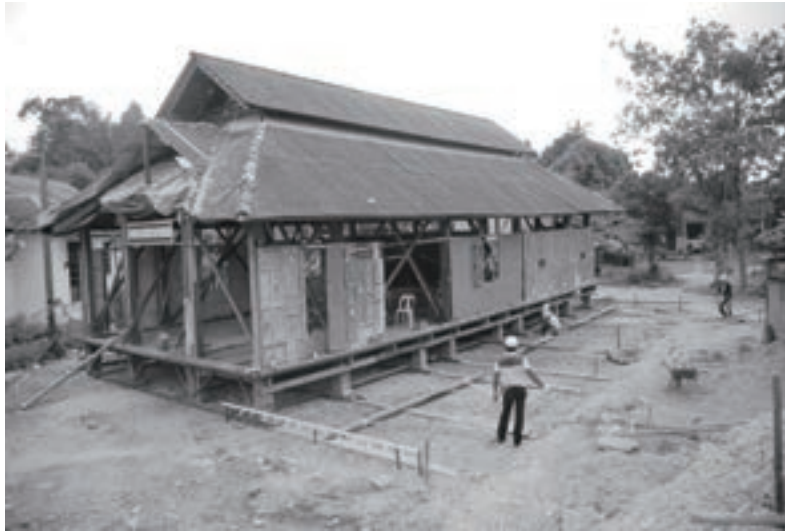
The Kedai Mulong Old Mosque was repositioned to its new location of 25 feet distance away
