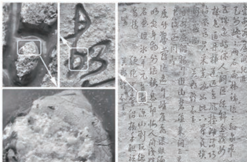
Figure 8. Accelerated deterioration caused by thick coatings
