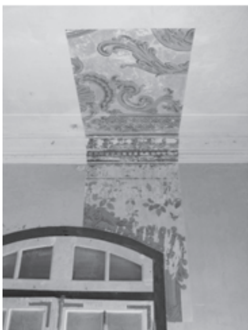
Decorative details covered by the lime mortar layers
