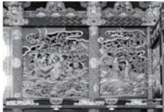
Fig.7. Chudei-shitaji base coat seen in initial coloring material analyses revealed that it is a coloring base coat material composed of green verditer, whiting and brass powder.
