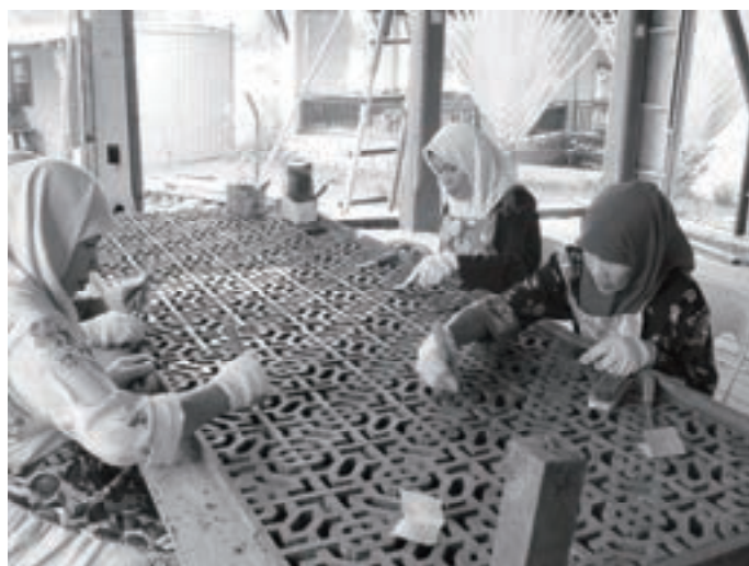
Local women were engaged in repairing the timber lattice panels of the mosque
