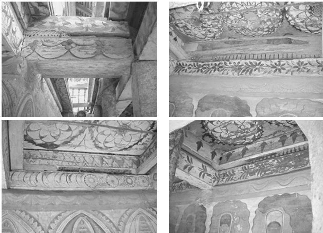
Decayed Beams
