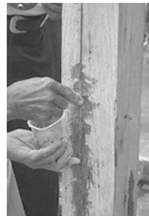
Patching with wood powder
