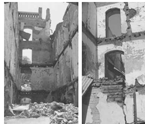
The gutted palace, no wooden elements remaining
