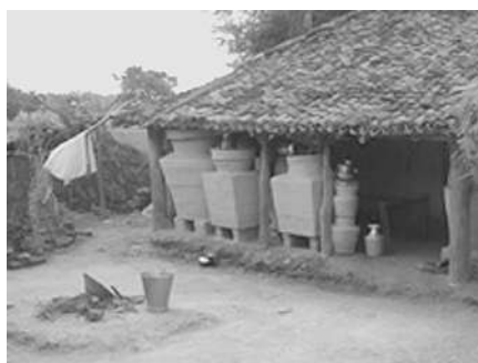
Traditional building form with wooden posts and tile roof in villages surrounding Lumbini
