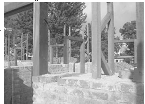
New construction with timber reinforcement
