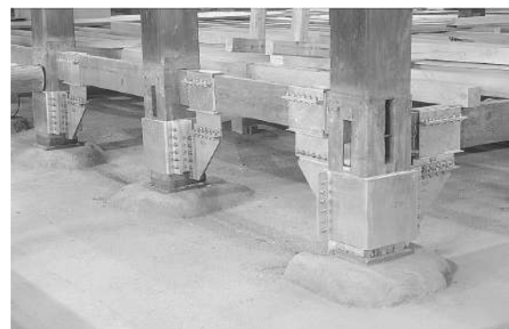
Fig. 10 Beam-column joint dampers
