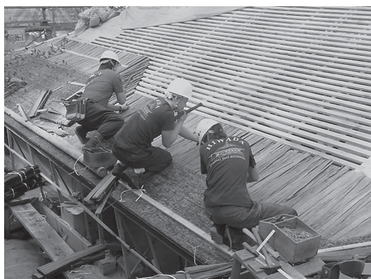
Fig. 5 Roofing with cypress bark, a “Selected Conservation Technique”
