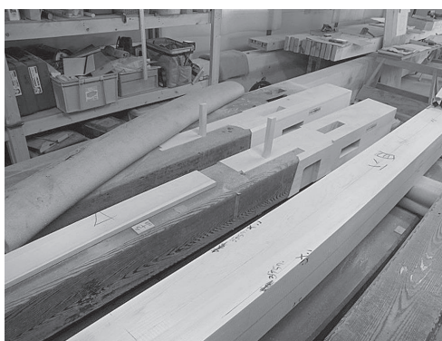
Fig. 4 Repair of wooden posts with traditional woodwork joints (Japan)
