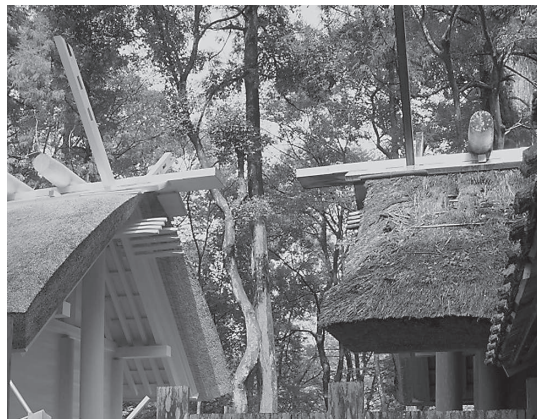
Fig. 2 Thatched roof buildings of Ise Shrine; 20 year old building to the right and newly rebuilt building to the left
