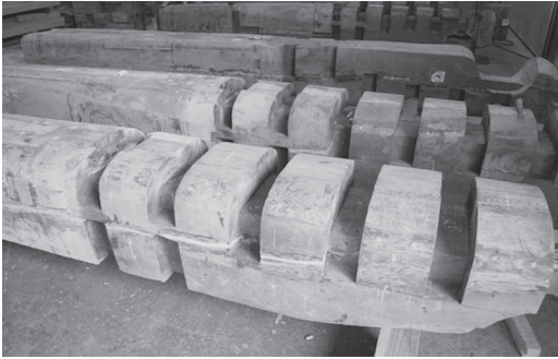
Reinforcement of cracks of the 1st floor girders by using special epoxy resin
