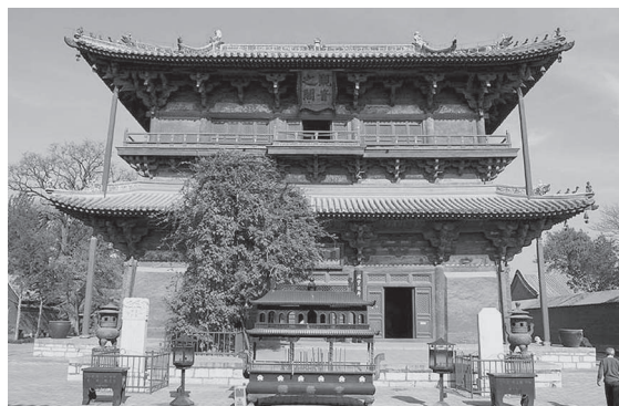
Figure 2 The eave-supporting pillars of Guanyin Pavilion in Dulesi Temple is the supporting structures added during renovation by later generation.
