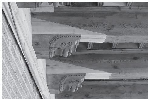
Fig. 3 Timber-to-timber repair of wooden beams (Palacio del Condestable, Spain)
