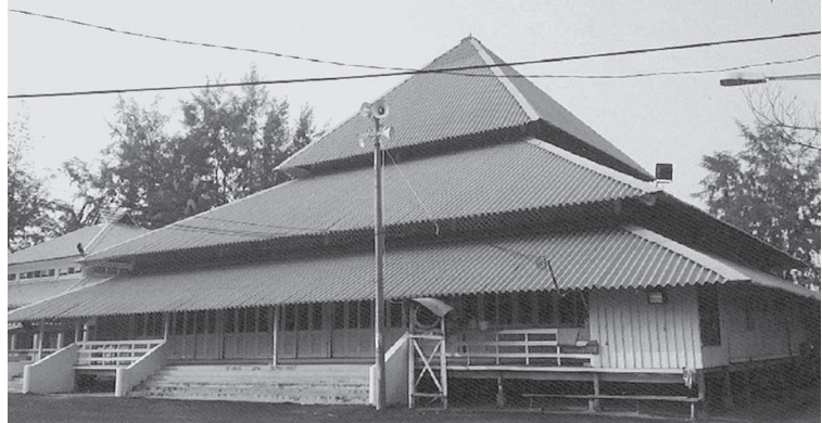
Mosque – Kg Dal mosque (L) and Meru mosque (R). Ventilation an important architectural feature in the hot tropics is seen here through woven bamboo walls of Kg Dal mosque. Often layered roof as in Meru mosque and structures on stilts provide ventilation
