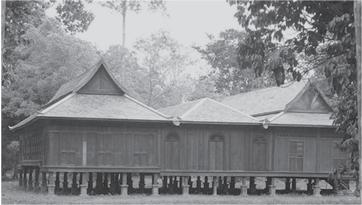
Rumah Kelantan – 12 pillar house has 3 roofs for main house, middle and kitchen. The roof is usually made of singgora tiles. Note the house is raised on a partially concrete pillar
