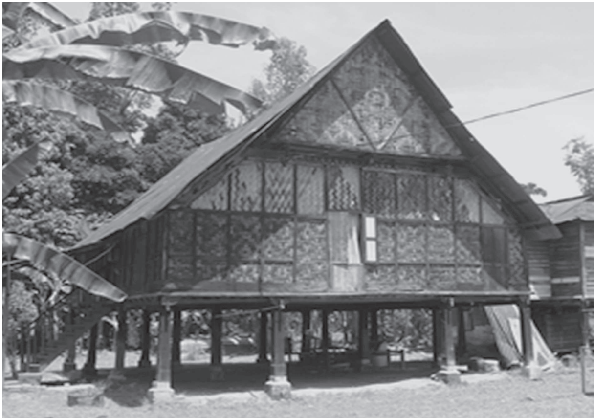
Rumah Perak – Rumah Kutai has large sloping roof and the walls are partially or completely of woven bamboo, and low concrete stumps support the pillars that raise the house above ground
