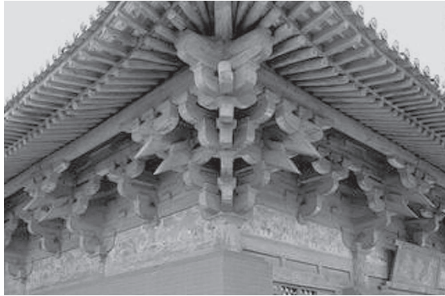
Figure 3 The brackets of later generation in the main hall of Country Guarding Temple in Pingyao, Shanxi which follow the Five Dynasties system
