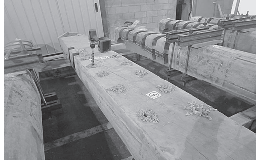
Reinforcement/compression pressing of cracks and then making holes for bolting work of the 1st floor girders
