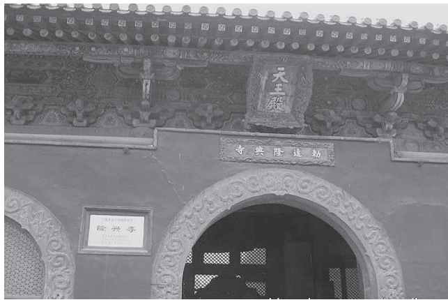
Figure 4 The brackets of the hall of Longxing Temple in Hebei have brackets from both Song Dynasty and Qing Dynasty
