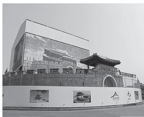
Paldalmun Gate covered with steel-frame prefabricated housing (Photographed on Mar. 27, 2012)
