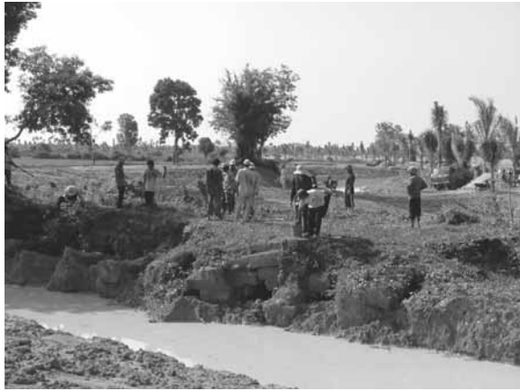
The bridge after clearing the bio-vegetation
