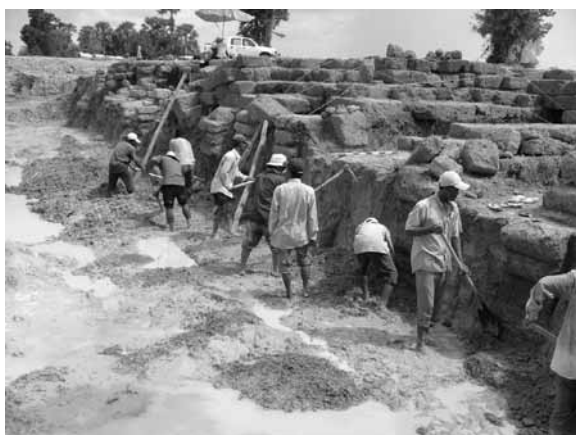
Blockages caused by accumulated soil in the bridge's drainage
