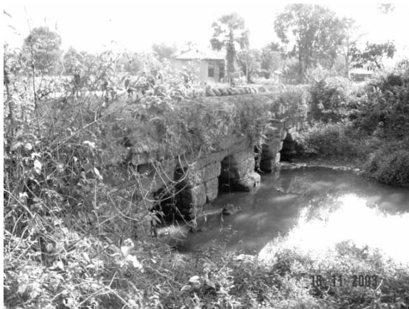
Before excavation bridge's embankment
