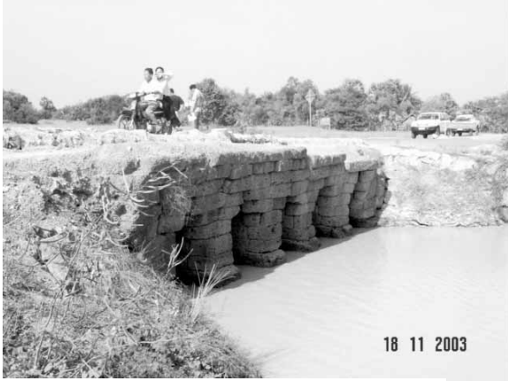
Before excavation bridge's
