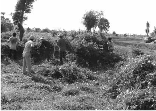
Clearing the bio-vegetation covering the bridge
