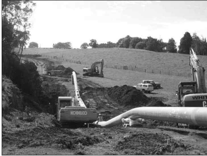
Figure 5: Installation of gas pipeline, Tikorangi, New Plymouth Photo: Jo Wylie, 2006
