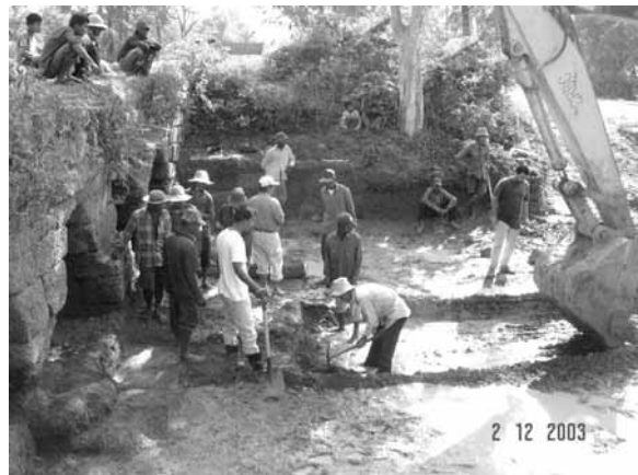
Excavated to determine the limit of the pavement and embankment step
