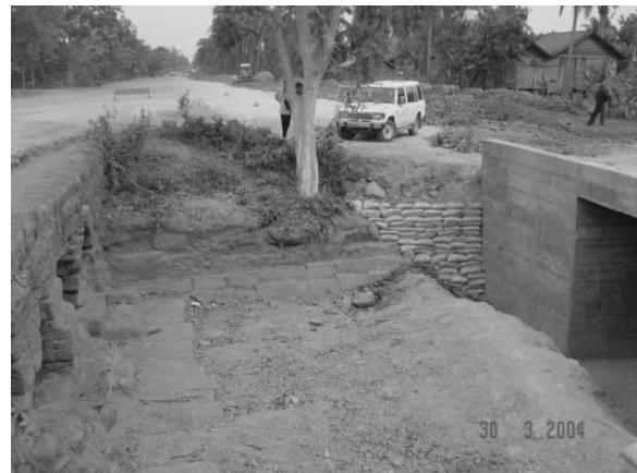
A new bridge already constructed
