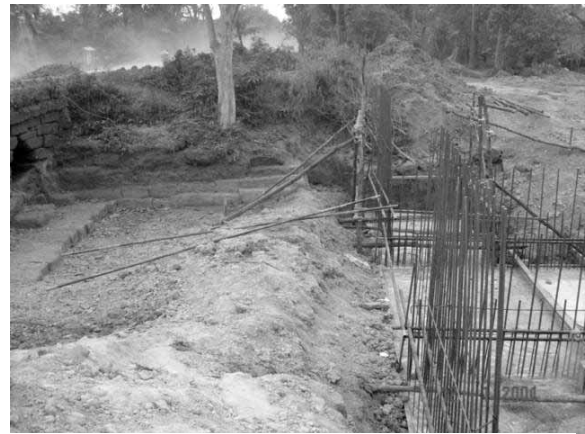
A new bridge was built 1.5m from the ancient embankment
