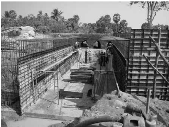
A new bridge being constructed
