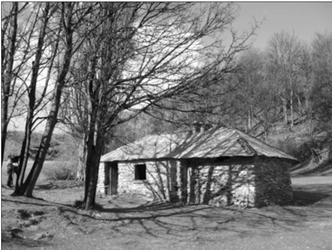
Figure 47. Bakery before restoration. (photo: Matthew Schmidt).
