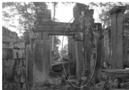
Pl. 14 JSA's reinforcement (wire wrap)
