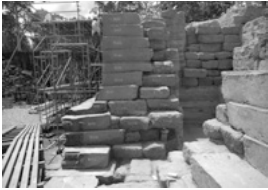
Pl.17 Detected laterite structure at northwest corner
