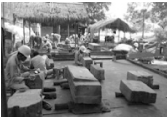
Pl. 23 Repairing sandstone components
