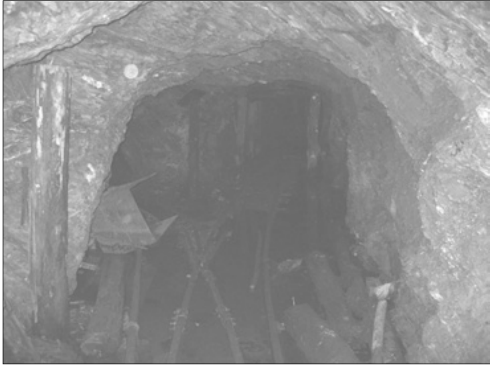
Figure 22. Scheelite and gold mine at Glenorchy, Otago. Original support timbers, mining cars and rail lines can be seen (photo: Matthew Schmidt).
