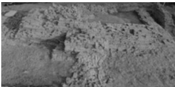
Structure No. 8B
