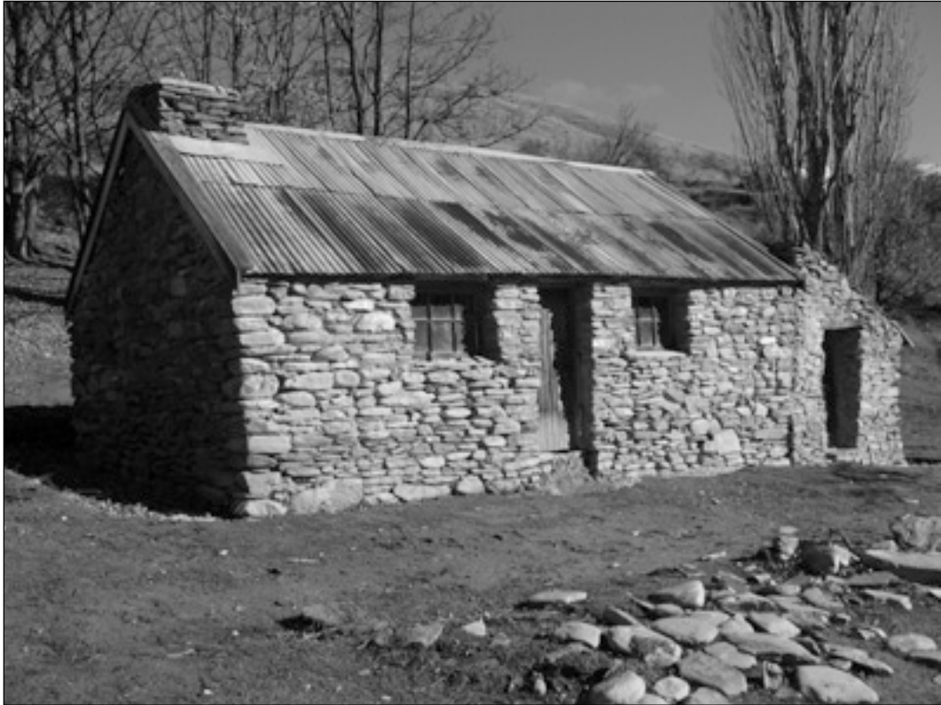
Figure 46. Needham's Cottage after restoration.(photo: Matthew Schmidt).
