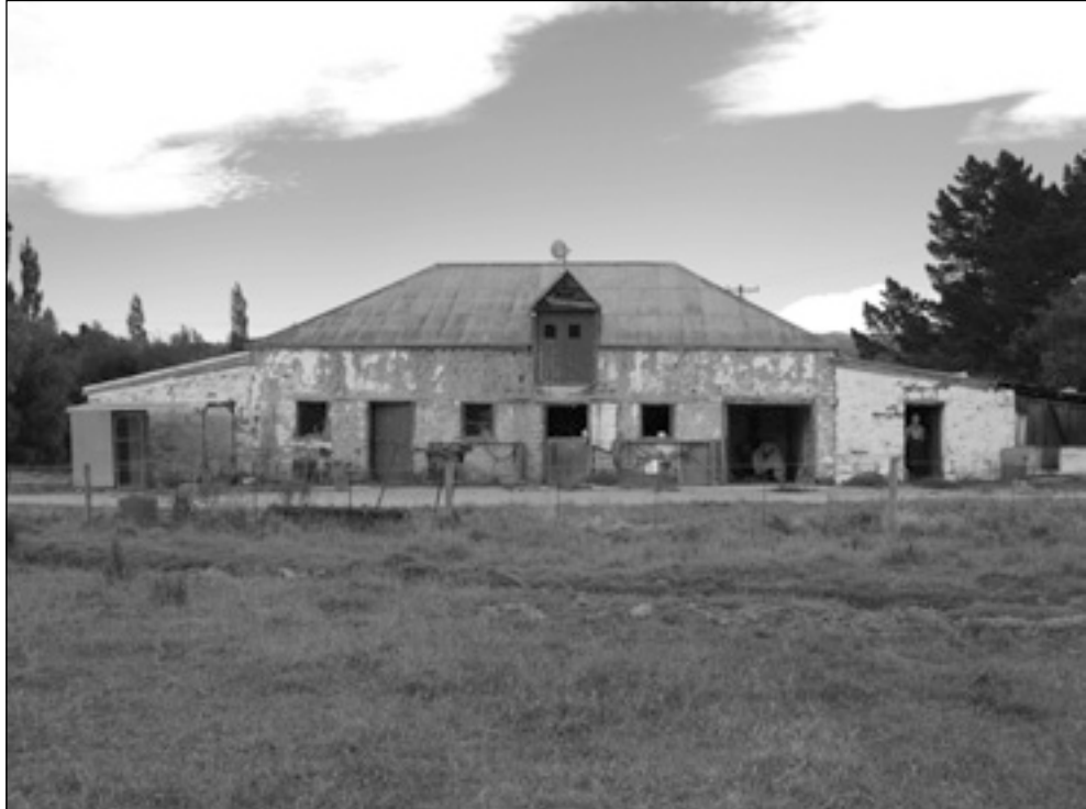
Figure 27. Mud brick stables and store built ca. 1871, Lauder Pastoral Lease, Central Otago. (photo: Matthew Schmidt).
