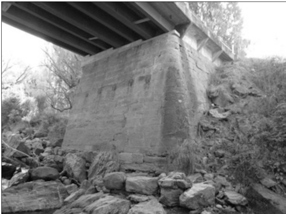
Figure 29. 19 th century stone bridge piers, Roaring Meg, Kawarau Gorge, Central Otago. (photo: Matthew Schmidt).
