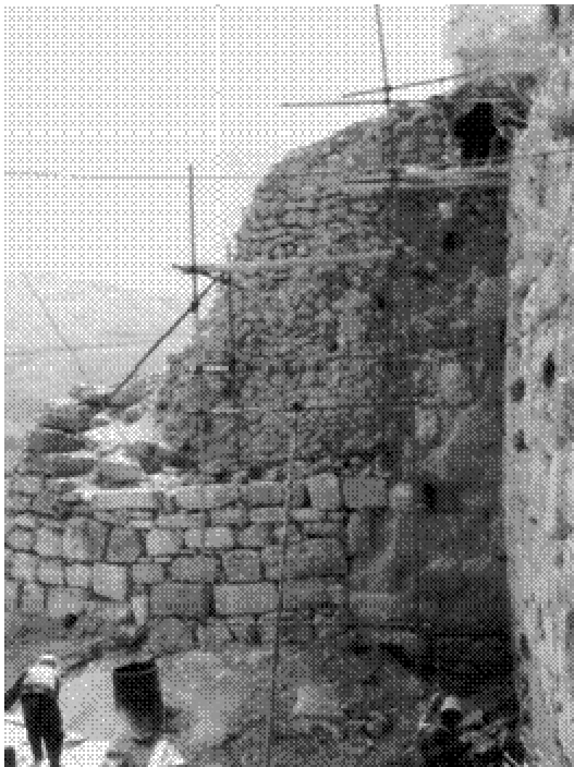
Figure12. Consolidation and stabilization of the ruined parts of the rampart
