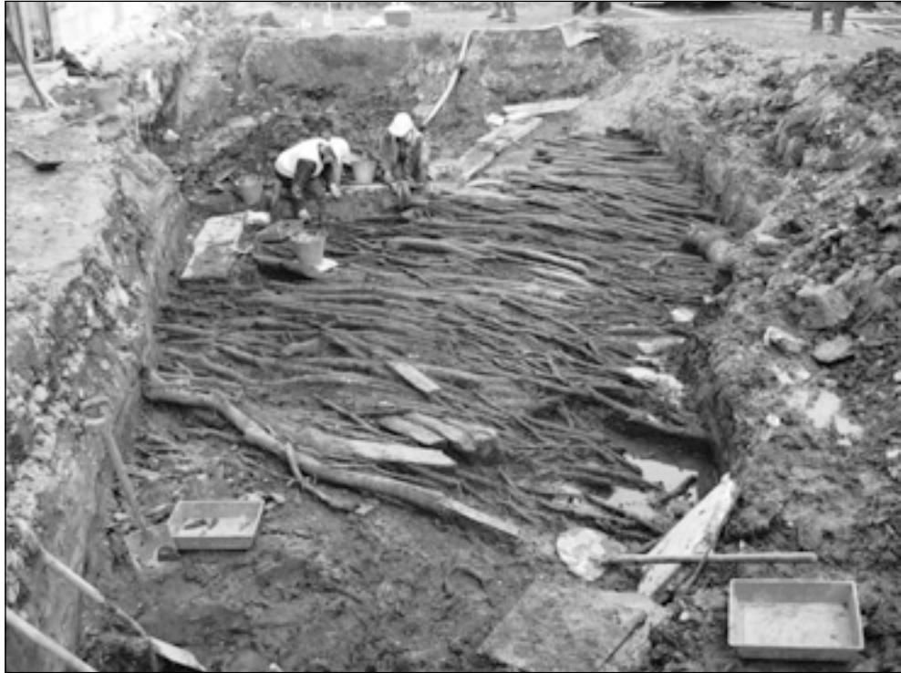
Figure 36. Corduroy (wooden) causeway from the 1850s when Europeans first settled Dunedin. The causeway was buried in wet pug/clay conditions 1.8m below the current road surface. (photo: Owen Graham).
