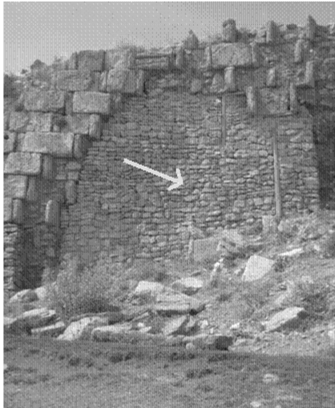
Figure7. Consolidation and stabilization of the ruined parts of the rampart
