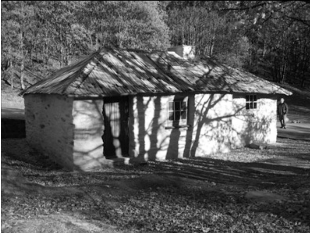
Figure 48. Bakery after restoration works. (photo: Matthew Schmidt).
