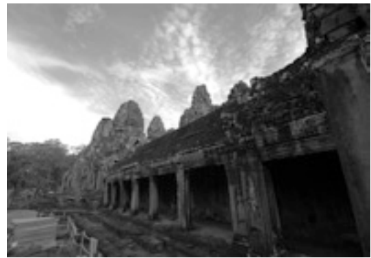
Pl. 4 Recent condition of the Inner Gallery
