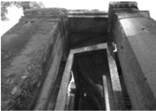
Pl. 13 EFO's reinforcement (concrete cement)
