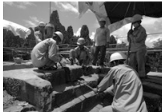
Pl. 22 Dismantling activities of southwest
