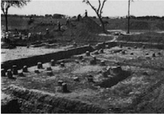
Fig. 13 Foundations under excavation.
