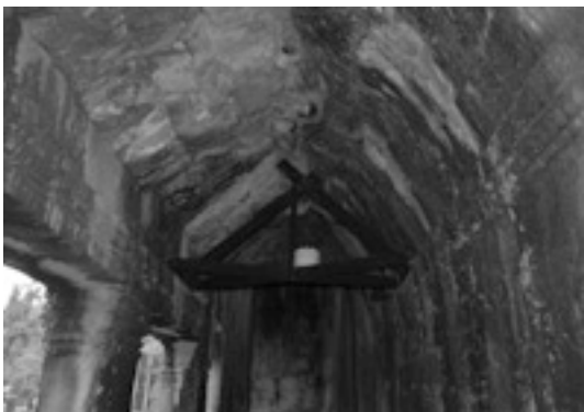
Pl. 15 JSA's reinforcement (wooden truss)
