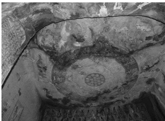
Picture 9. Leaking water on the Wanfo Cave roof
