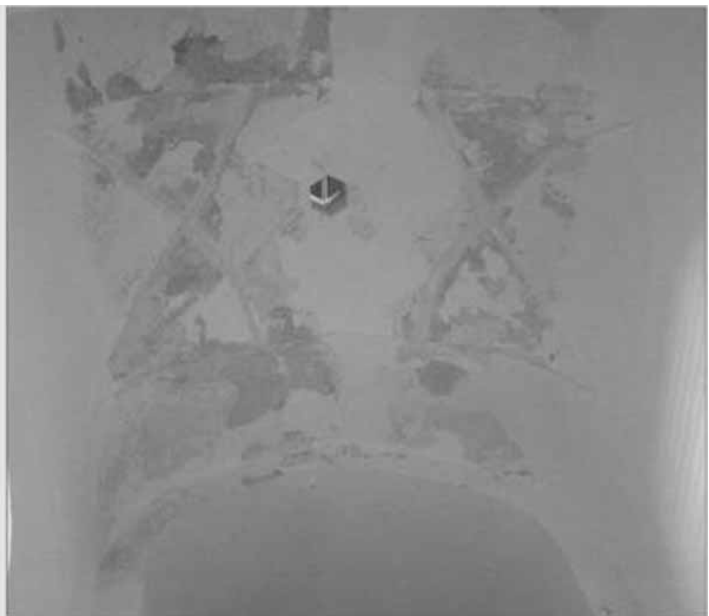
Damp ceiling even after installation of a water resistant shield
