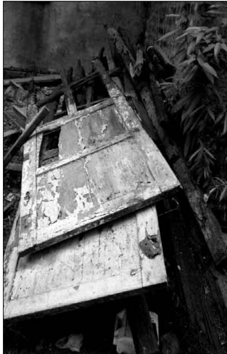
Figure 14. Original doors and beams from St Michael's Church, showing evidence of burning
