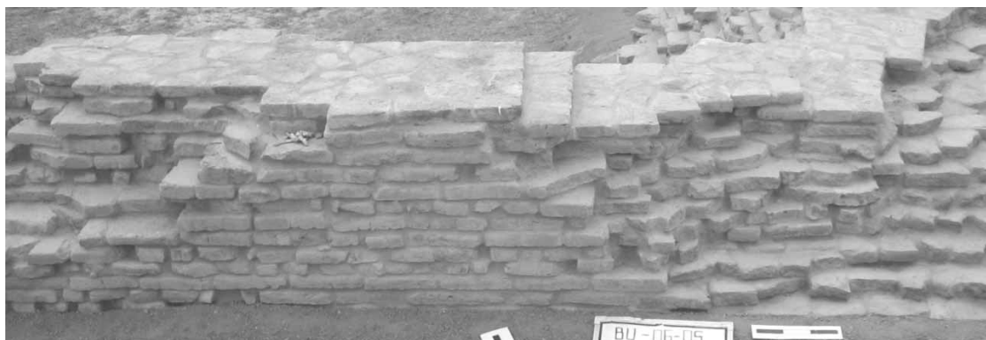
Fig. 8 A protective layer on the surface of the top part a wall, Mausoleum 4
