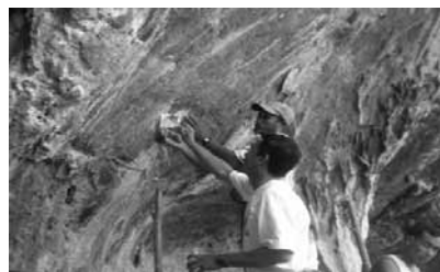
Cleaning of lime whitewash with chemical solution
