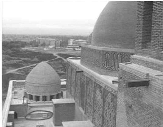
Water resistant shield forming an extraneous layer
