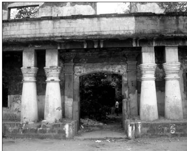
Figure 15. Original columns west of the church, made of plaster over brick (Photo by Elle Lim)
