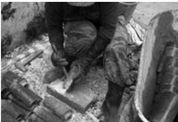
Fig. 19 Cement mortar previously adhering to the roll tiles was carefully chipped off by hand
