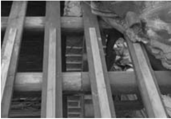
Fig. 13 Local section of rotted purlins replaced by new timber
