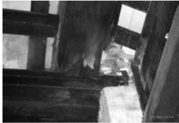
Fig. 16 I-section steel lintels between the brick piers
