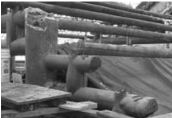
Fig. 3 Timber frame components with of loss structural capability were replaced by matching timber poles
