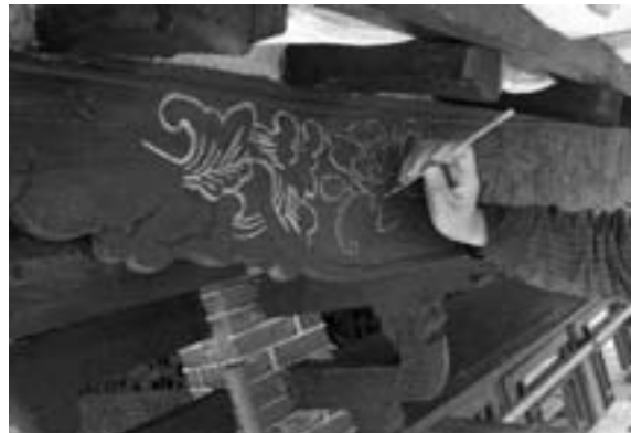
Fig. 28 Restoring grooves painted in "gilt thread drawing"
