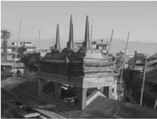
Metal pinnacle ( gajur ) support ( bhangī ) and wooden planking before jhingati laying on the roof
