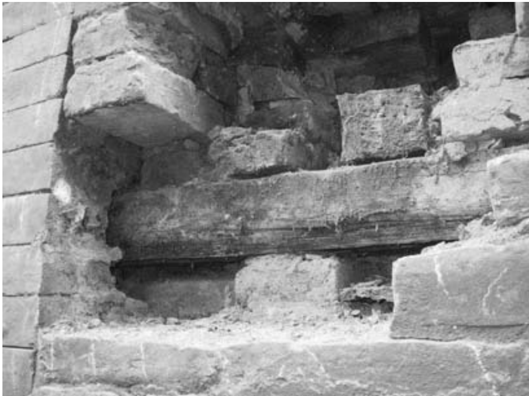
Decayed tie timber seen in a wall panel test
