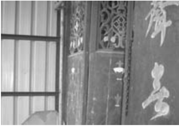
Fig. 29 The existing timber doors with lattice patterns are in good shape with little sign of fracture or rotting
