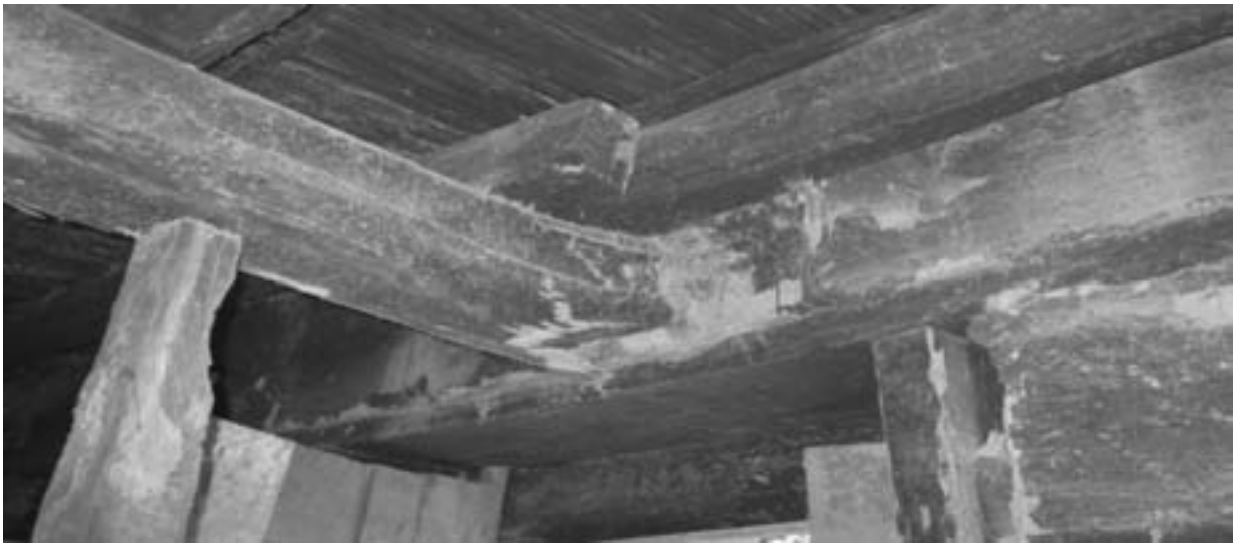
(Fig.5.1) Timber decay
