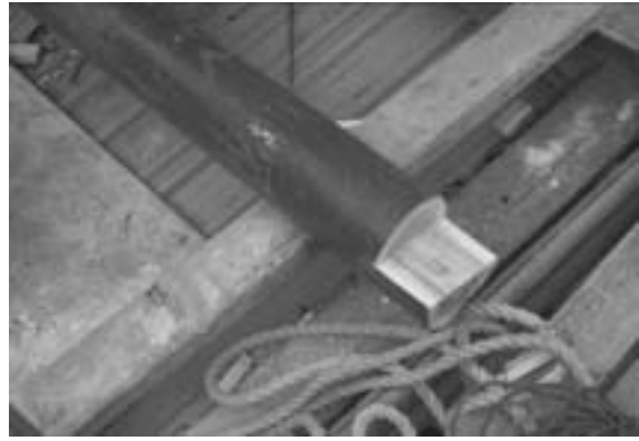
Fig. 14 Local section of rotted purlins fitted back to the main member by traditional crafted joints
