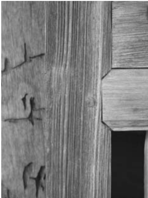
Examples of deterioration of rumah pencu caused by insects, ultraviolet light, fungi and humidity
