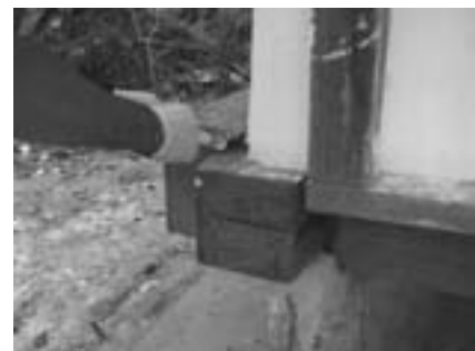
Fig. 50 Applying insecticide
