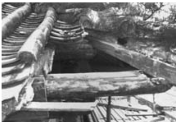
Fig. 11 Occasional sections of overhanging purlins are found to have rotted
