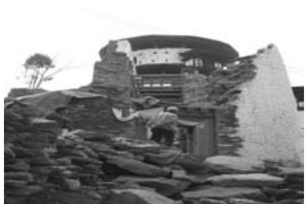
(Fig. 5.3) Poor bonding and bulging
