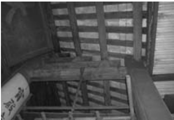
Fig. 1 Supporting the roof of the Main Grand Hall is a Lingnan style lifting-beam with strut-column timber frame
