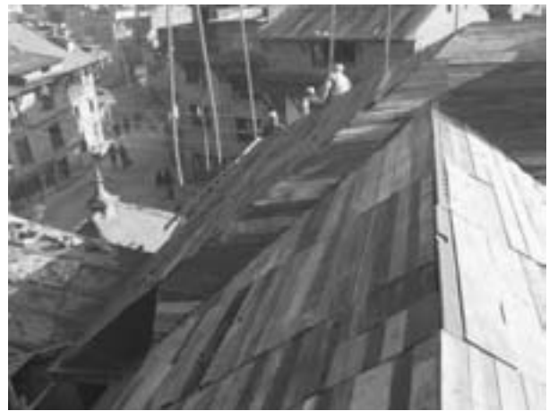
Metal pinnacle ( gajur ) support ( bhangī ) and wooden planking before jhingati laying on the roof
