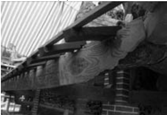
Fig. 27 The rotted corners of the eaves board were repaired in situ
