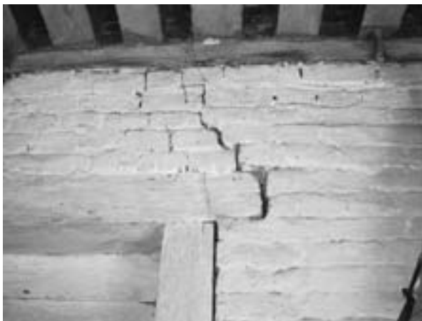
Wall cracks seen in the interior and exterior walls of the dyochhen
