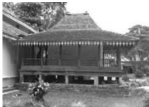
Figs. 34-37 Timber frame as the base to the entire image house
