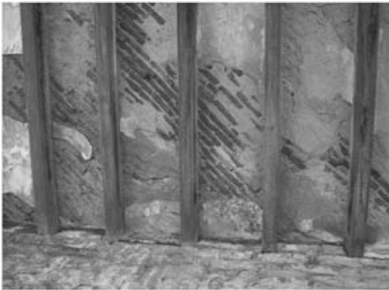
Fig. 17 Madras terrace roof with wooden secondary beams and bricks laid at an angle, partially deteriorated due to water seepage
