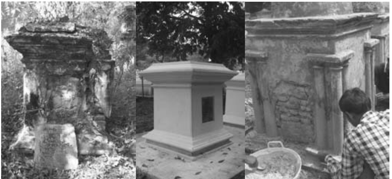
Fig. 23-25 Restoration consisting of vegetation removal, masonry reconstruction/consolidations, lime plastering in coarse and fine lime mortar, restoring lime plaster embellishments and stone plaques for 300 tombs in a cemetery
