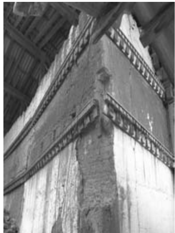
(Fig. 5.4) Erosion due to weathering
