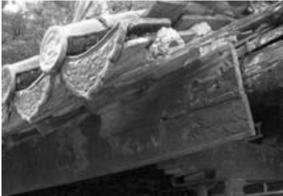
Fig. 25 The existing eave board was covered with dirt and mould at the start of project
