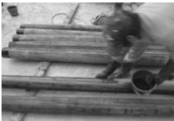
Fig. 5 Timber frame painted with two layers of raw tung oil until soaked wet just like the traditional method
