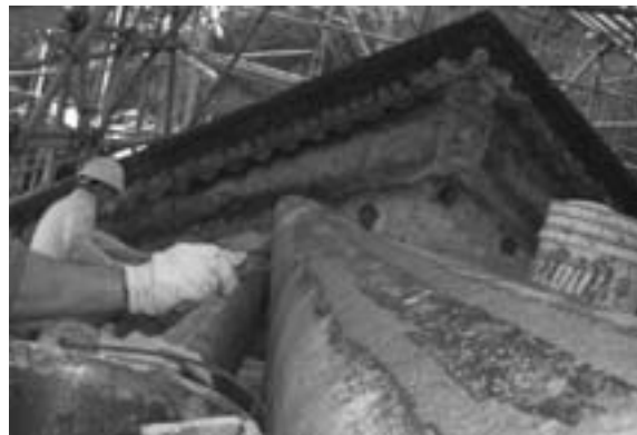
Fig. 4 Filling up the gaps with wood blocks and chips mixed with resin
