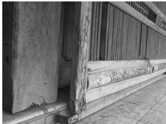
Examples of vandalism ( left ), and damage from ultraviolet light, humidity, and insects ( right )
