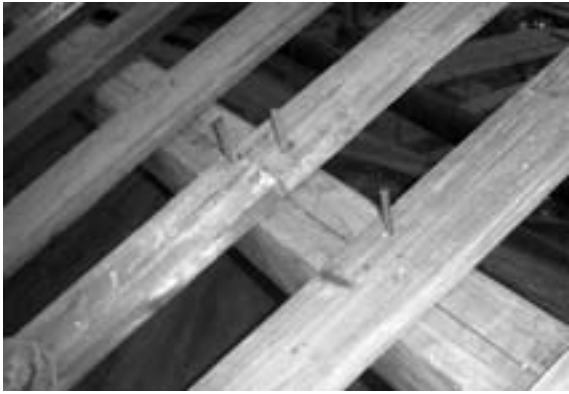
Fig. 21 The team re-introduced a Lingnan traditional technique of fixing with bamboo nails
