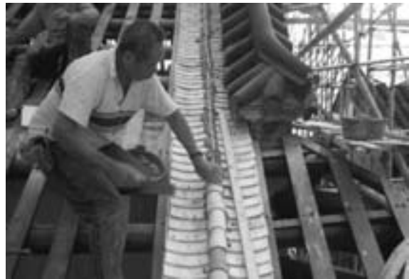
Fig. 18 Using continuous rows of interlocking cylindrical tiles to cover the joint between rows of pan tiles
