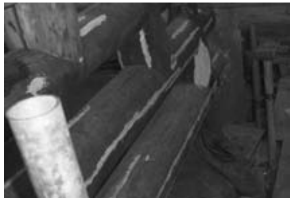
Fig. 2 Timber frame with minor damage was repaired while remaining in place
