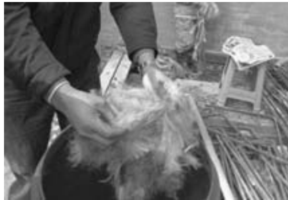
Fig. 34 The method of hemp-mixed lime plaster was eventually tested and applied
