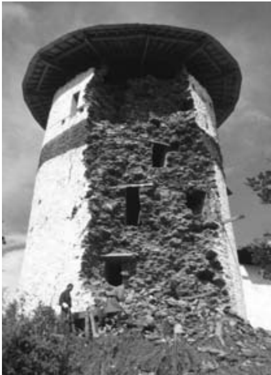
(Fig. 5.3) Poor bonding and bulging
