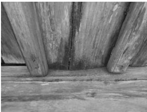
Damage to a the ceiling due to leaking water ( left ), and to a sliding door from climate and human factors ( right )
