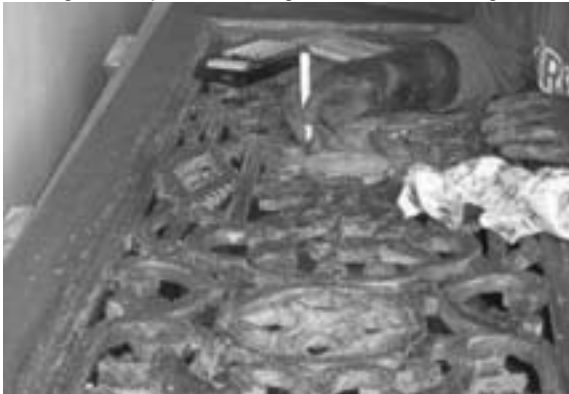
Fig. 31 Workers applied diluted chemical paint remover on the wood surfaces
