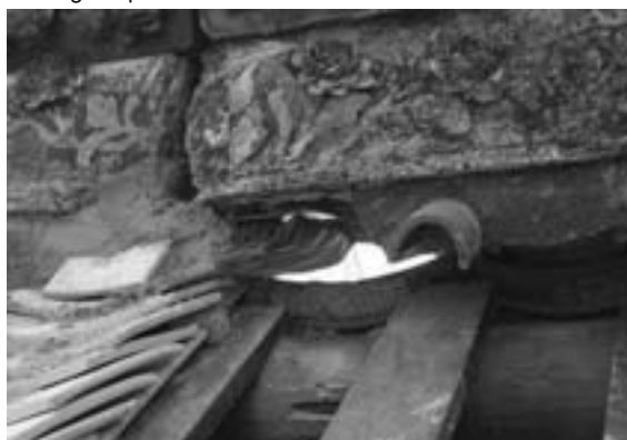
Fig. 12 A major fracture at the middle of the ridge decoration
