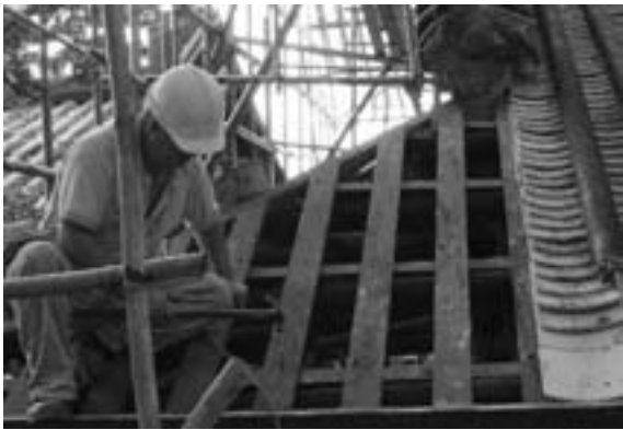
Fig. 17 The roof is the traditional Lingnan "single roll, single pan" tile construction
