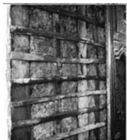
Fig. 22 Structure of mural painting at Dalada Maligawa (Prematilleke and Colombage, 2000)
