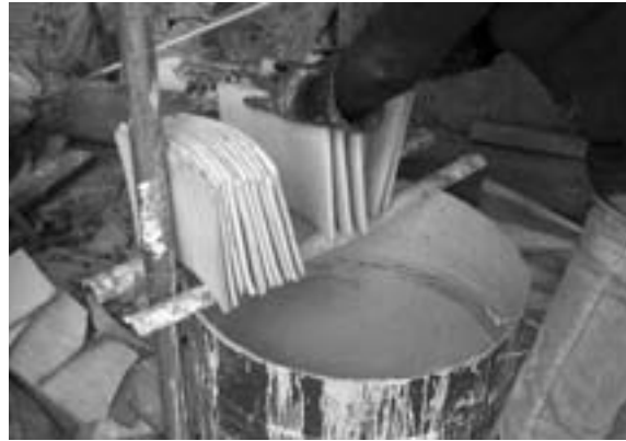
Fig. 24 The salvaged pan tiles were soaked in lime water for up to three times until they appeared white
