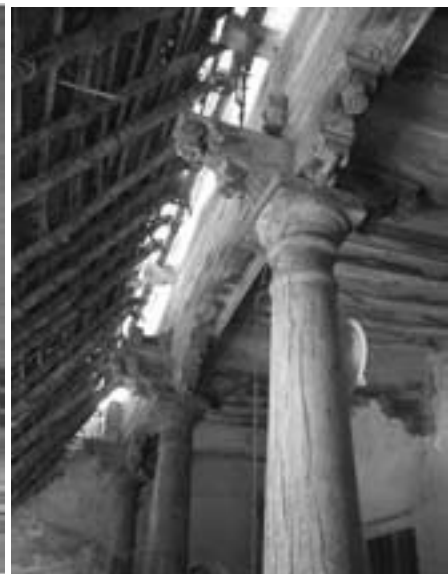
Fig. 18 Wooden columns, carved brackets and beams, in a historic house
