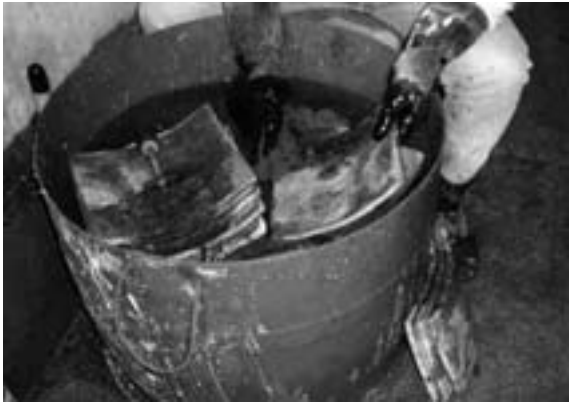
Fig. 23 The salvaged pan tiles were selected, and then thoroughly cleaned of bird droppings and mould
