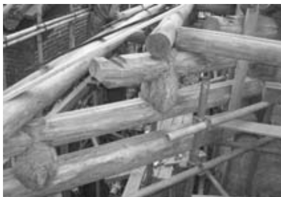
Fig. 6 Replacing part of the timber structure with new members using traditional carved jointing
