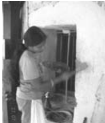
Fig. 46 Filling the rendering
