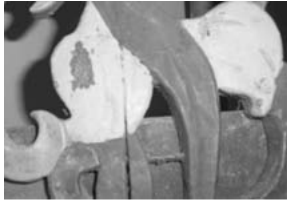
Fig. 30 Cracks and chipped-off corners to be repaired by traditional filling of wood dust mixed with mortar
