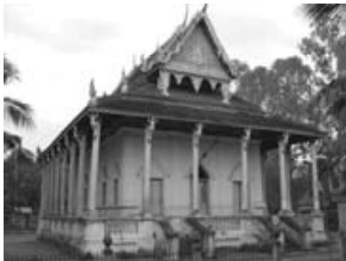
Fig. 16 Ancient prayer hall with a roof structure of wood and core of bricks
