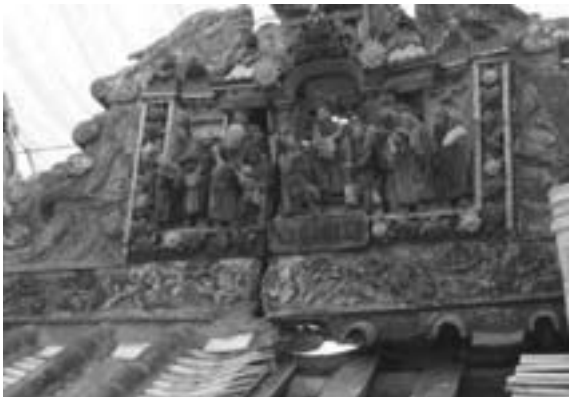
Fig. 33 A major fracture is found in the middle of the group of Si-wan glazed ceramic
