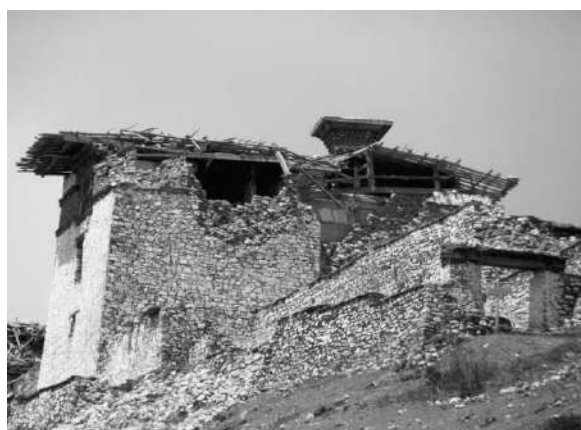
Fig. 6 Lingzhi Dzong, damaged by an earthquake. Photo: DCHS
