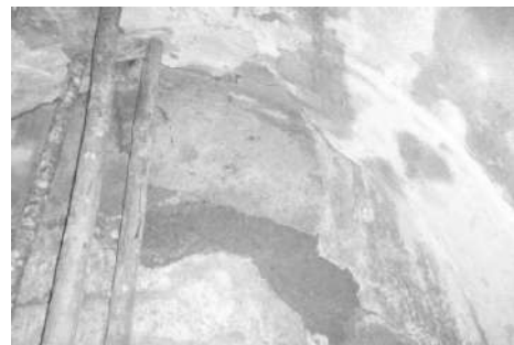
Cracks on mortar
