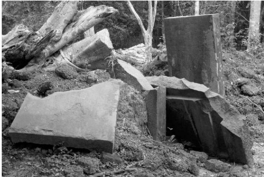
Fig. 8: The outer west gopura 's doorframe at Prasat Yeai Poan broke due to a large tree (2011)
