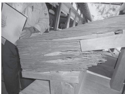
Cross section of roof at Kasuga-taisha Shrine Nara
