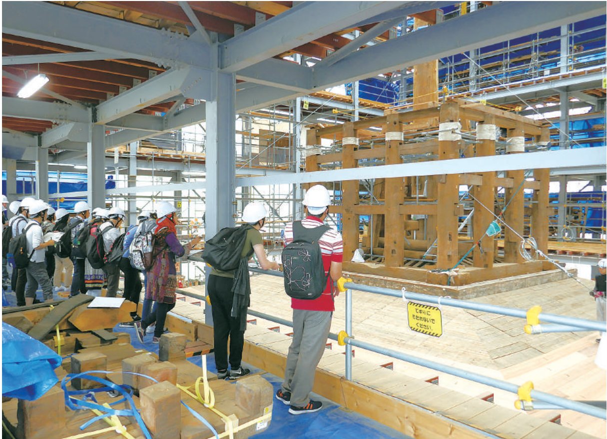
Observation of total dismantling repair work of the east pagoda in Yakushi-ji Temple (Assembling the members to original position)
