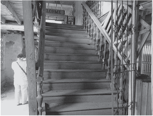
Fig. 10. Old wooden stair. Though worn out from use, it is still functional. It will be dismantled and reinstalled after repair and restoration.
