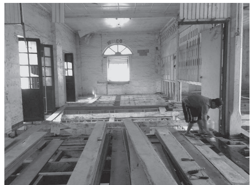
Fig. 15. Wooden floor planks being dismantled for rehabilitation, cleaning and treatment
