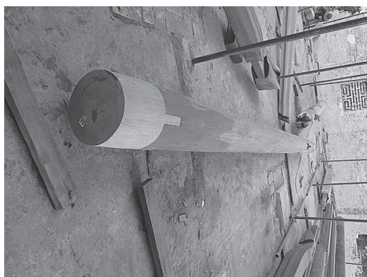
Fig. 9. The replaced end of a pillar (HMCC, 2014)
