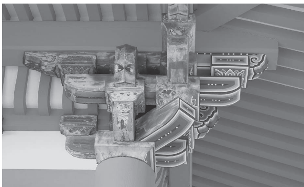
Left: Bracket complex: original painting partly preserved Right: Re-roofing work of the main hall
