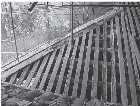
Fig. 7. Deformed roof system (HMCC, 2014)
