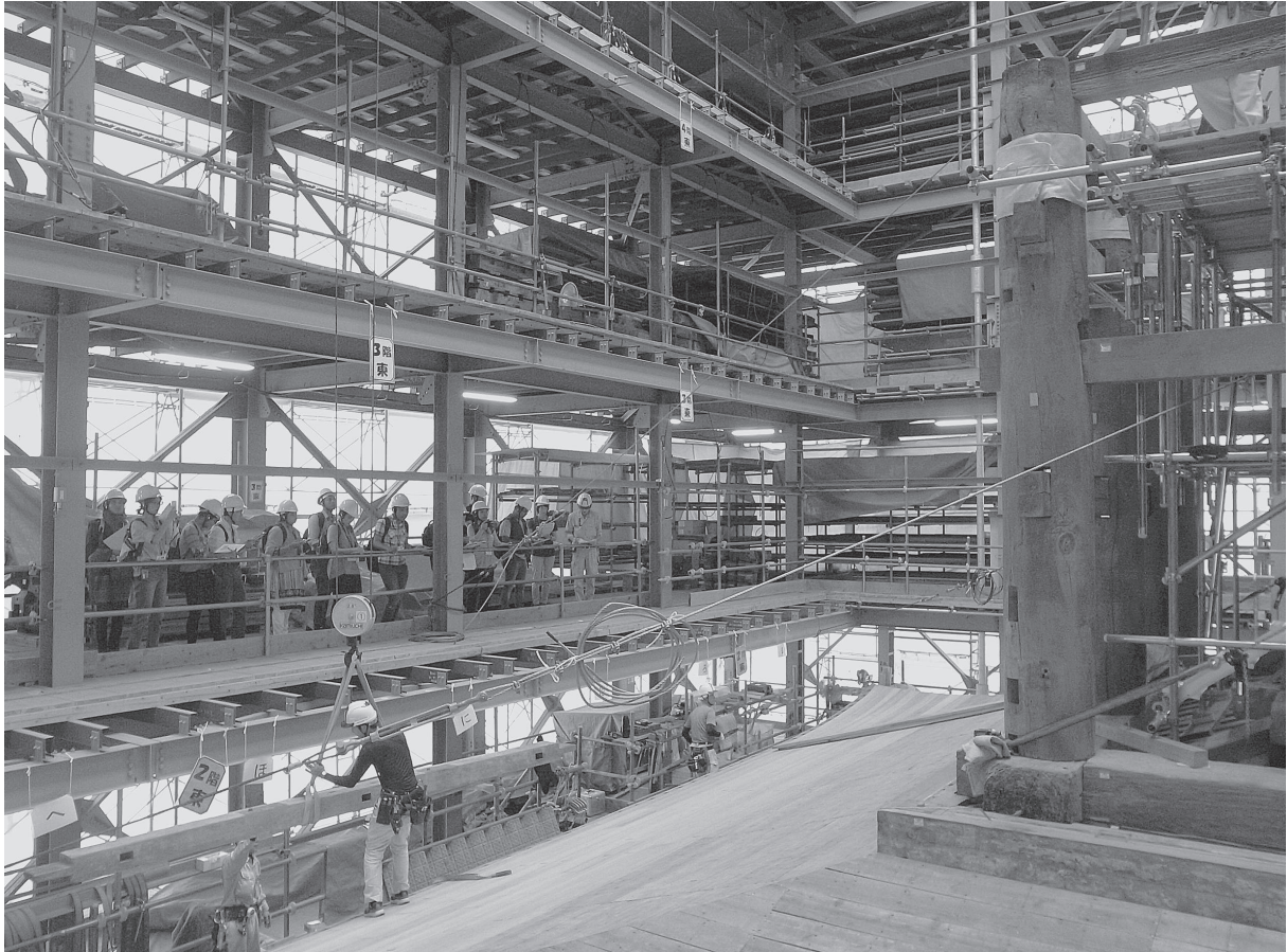
Observation of total dismantlement work of east pagoda at Yakushi-ji Temple
