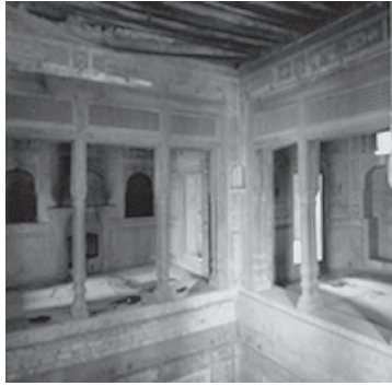
Fig. 7. Deteriorated timber roof due to water seepage and termite attacks
