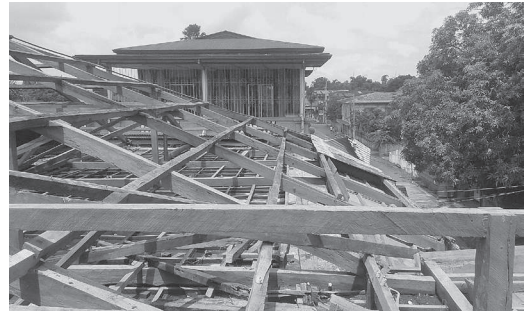
Fig. 17. Part of the roof showing wooden trusses and purlins being repaired after the corrugated GI roofing was dismantled for replacement
