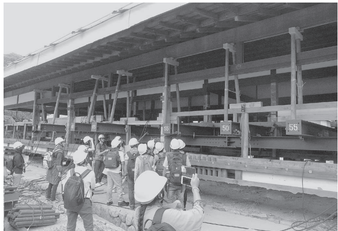
Left: Mr Kaneko instructing damaged survey of wooden members
