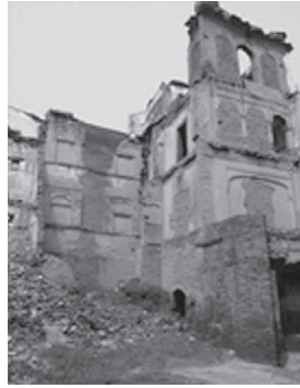
Fig. 8. Missing wooden doors, roof and jharokhas
