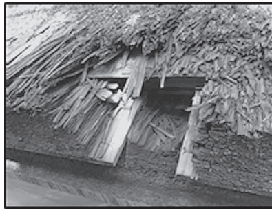
Picture: Roofing with cypress bark
