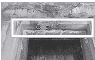
Deterioration due to salt from the concrete support
