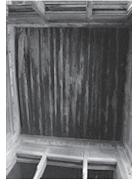
Fig. 9. Decayed wooden beams and columns
