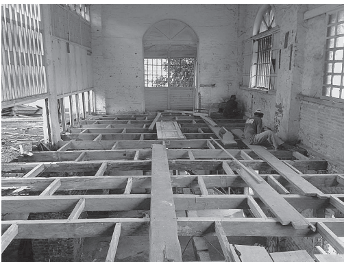
Fig. 14. Wooden floor joists and bridging on the second floor of the building undergoing repair
