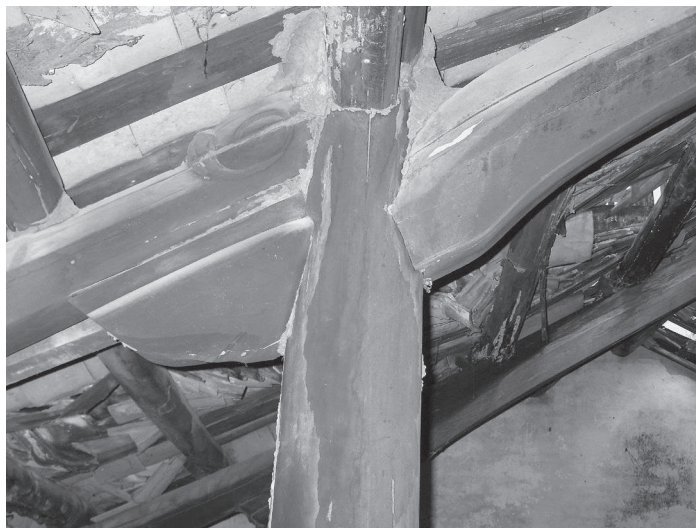
Figure 3. Traditional decorative woodwork decayed due to termite infestation (photo by the author)
