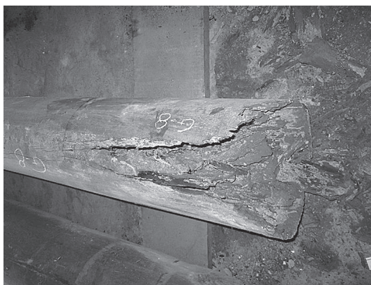
Fig. 5. The end of a degraded pillar (HMCC, 2014)
