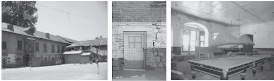
Figure 1. (Left) Front façade of the house. (Center) Structural crack observed in the basement. (Right) Billiards room, Khatamband ceiling damaged and replaced with wooden planks. (photos by the author)
