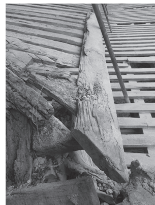
Fig. 8. Deformed roof system (HMCC, 2014)
