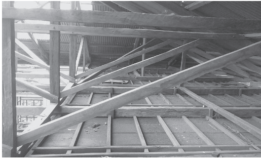
Fig. 16. Truss members and ceiling joists of the roofing. Many of the truss members are still intact and need only minor repairs and rehabilitation.
