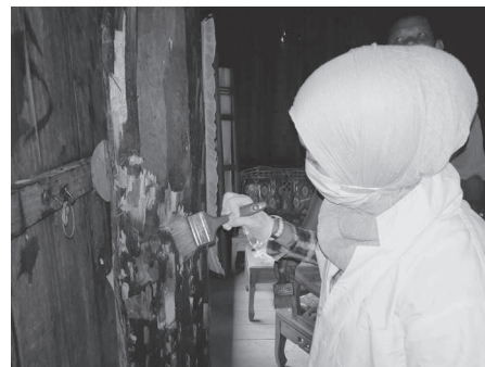
Fig. 6. Application of tobacco and cloves for cleaning and pickling wood in rumah gadang Rosma Syarif, Sumpur district, Tanah Datar Regency, 2016
