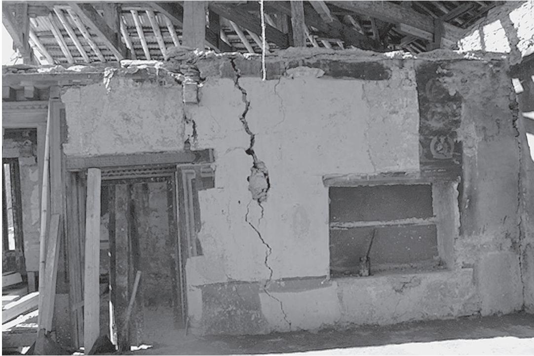
Figure 6. The structural walls and timber components are interlinked. Wogmin Lhakhang at Phajoding.
