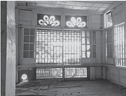
Fig. 12. View of the interior of the balcony. Many wooden parts in this section of the building are already dilapidated.
