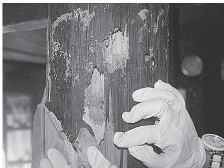
Fig. 5. Wood damage caused by termites in rumah gadang Rosma Syarif, Sumpur district, Tanah Datar Regency, 2016
