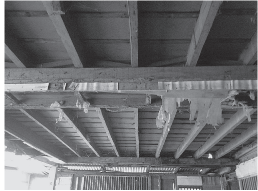
Fig. 11. Wooden girders and floor joists of the second floor, shown here with dilapidated members
