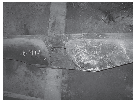
Fig. 6. Beams suffering from termites (HMCC, 2014)
